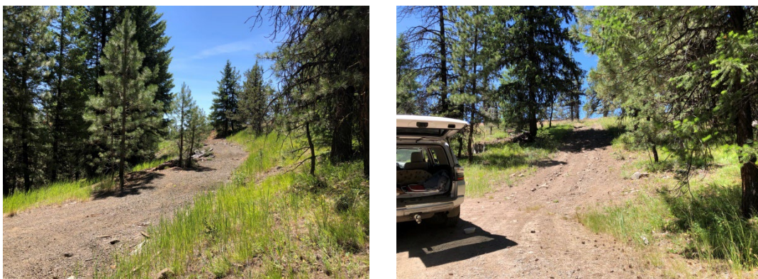
Figure 11. 30-500 road at its legal end. Breached berm in the left picture that is well driven and a go around road in the right picture. This breached road allows unauthorized motor vehicle access to another 2 miles of closed road in the headwaters of Peterson Creek and a network of roads and trails that extends to Dry Porter Creek.
