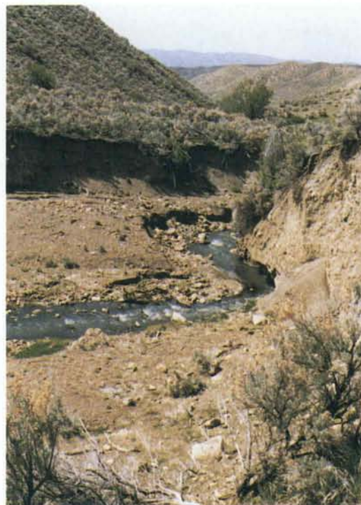
Vertically unstable stream channel.
