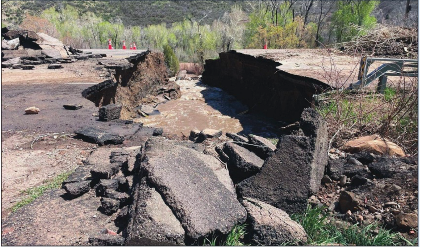
Colorado Highway 133 collapsed between Paonia and Somerset May 3 when the culvert below failed and opened what CDOT called a sinkhole.
