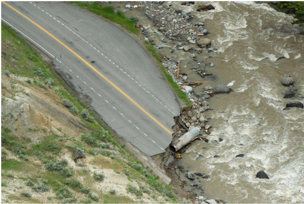
A broken culvert rolls out from underneath a washed out section of North Entrance Road on the Gardner River in Yellowstone National Park on June 19.
