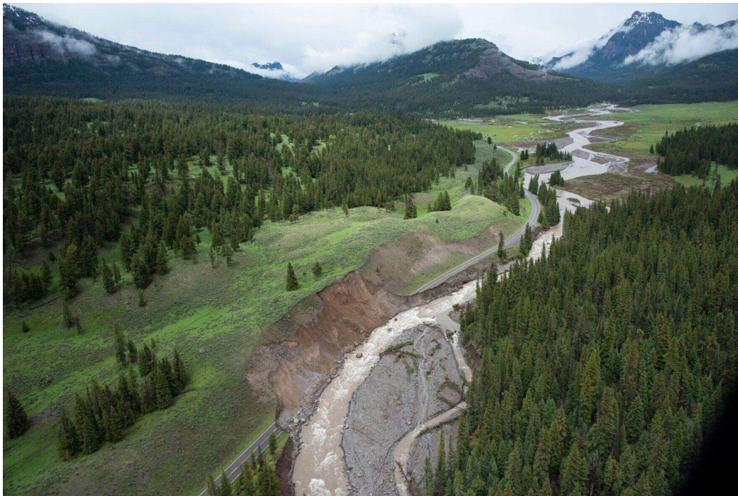
Sections of Northeast Entrance Road are washed out due to flooding on Soda Butte Creek on June 19 in Yellowstone National Park. Samuel Wilson, Bozeman Chronicle, Report for America
