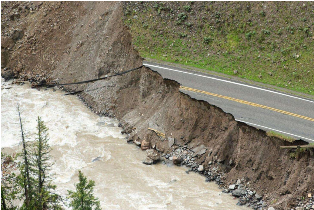
A section of utility lines are exposed in a washout of Northeast Entrance Road next to Soda Butte Creek in Yellowstone National Park. Samuel Wilson, Bozeman Chronicle
