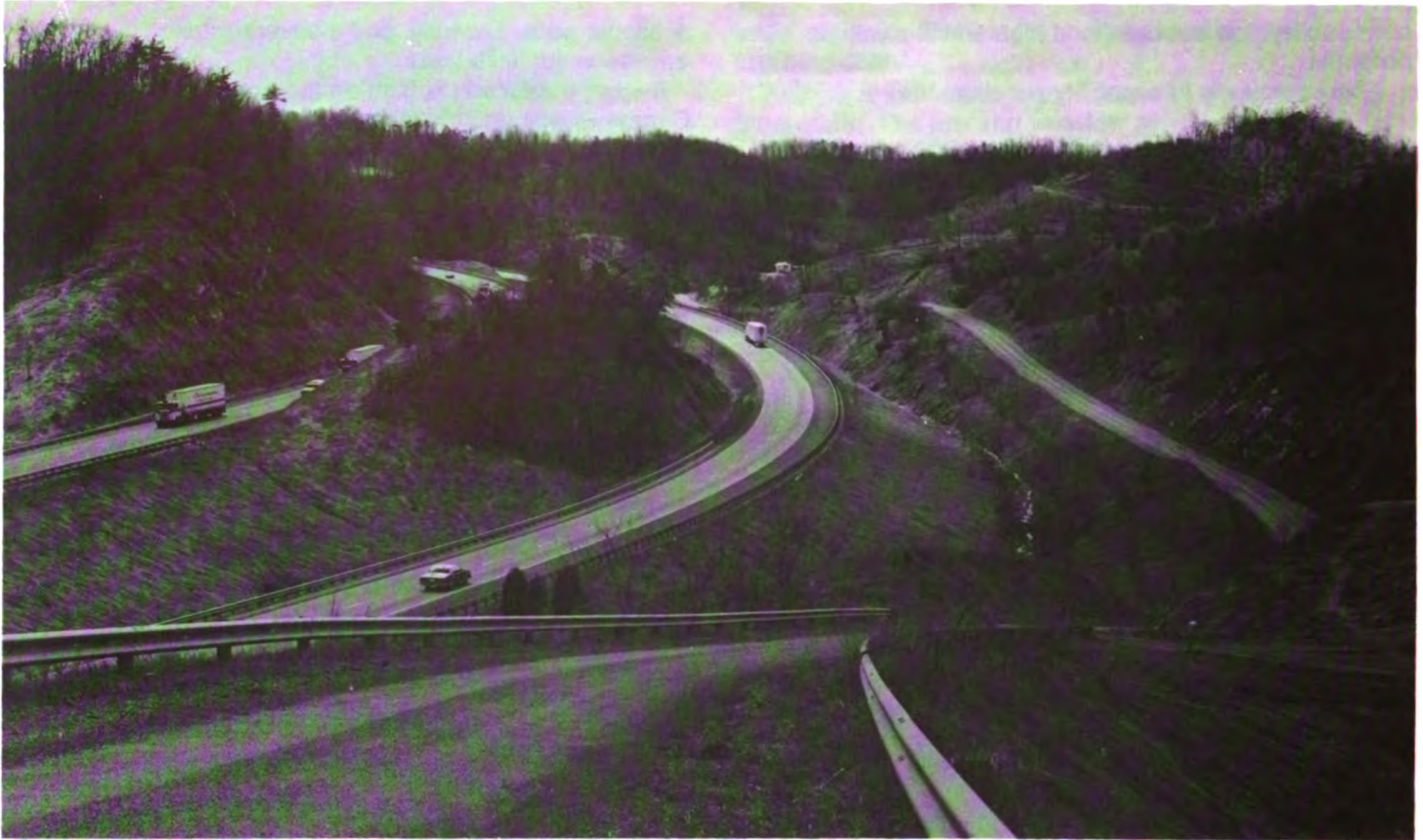
Figure 7.—Slope and shallow depth to bedrock limit excavation during highway construction, and slope and low strength limit the use of the Caneyville-Opequon-Rock outcrop complex, 25 to 60 percent slopes, as a source of roadfill.
