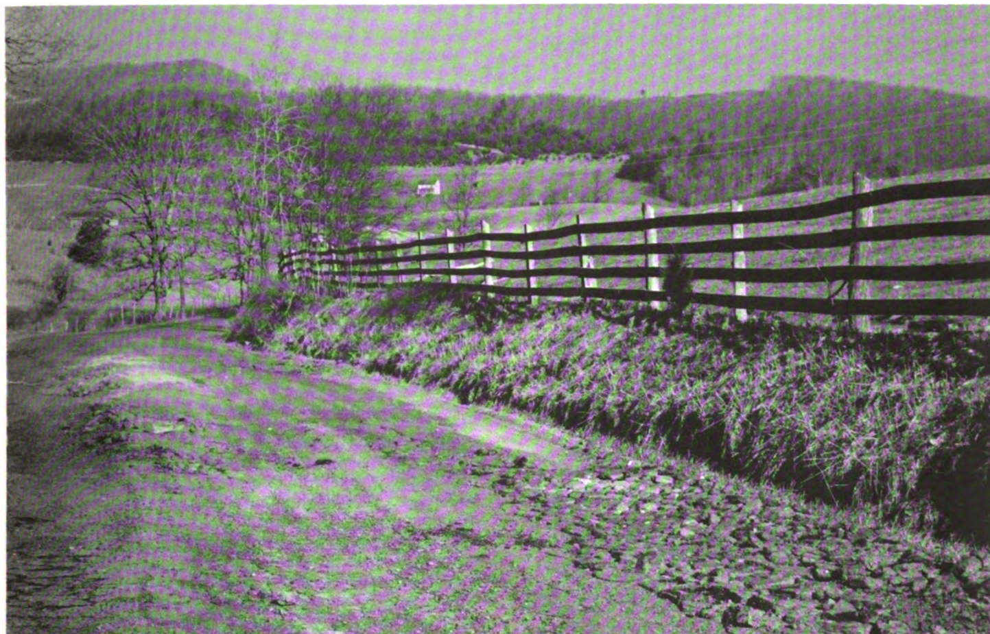
Figure 9.—Frost heaving on Guernsey silt loam, 2 to 7 percent slopes, causes disintegration of pavement.
