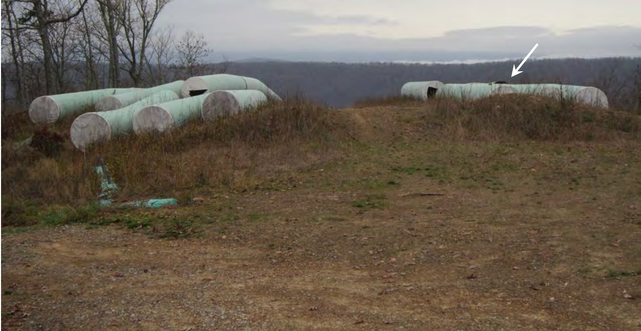
Figure 3. Photograph of pipes in the Jefferson National Forest adjacent to Forest Service Brush Mountain Road, taken from the road and looking toward the northwest. Holes in two of the pipe cappings are visible in the photo. The white arrow points to the top section of another pipe located behind those in the foreground that does not have a capping.
