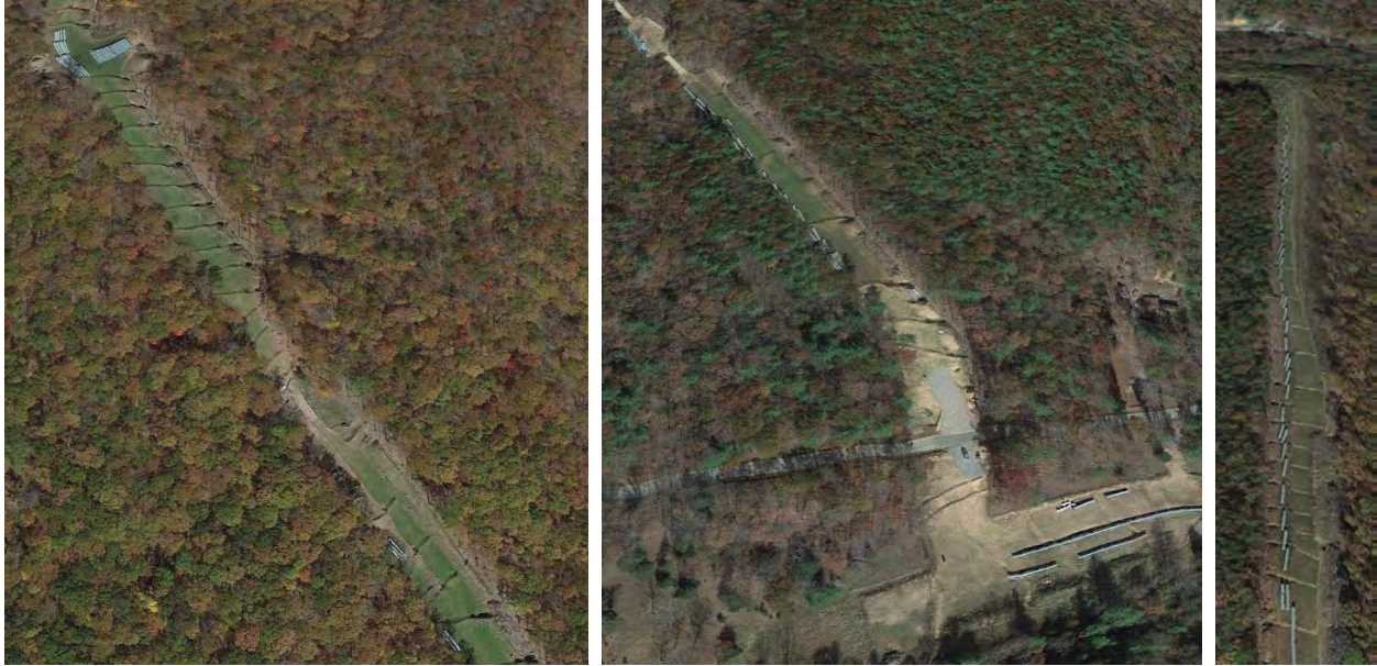
Figure 1. Google Earth imagery of pipes exposed to the elements in Jefferson National Forest on the upper southeastern slope of Sinking Creek Mountain (left), the lower segment of that same slope and adjacent to Craig Creek (middle), and the northwestern slope of Brush Mountain (right). Imagery is dated 11/2019.
