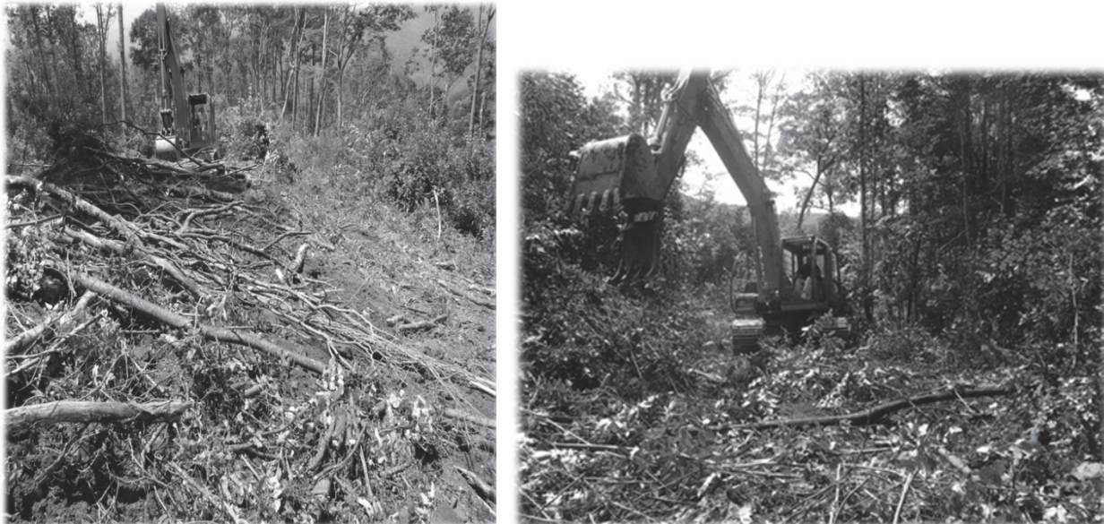
Figure 20. Farmers Branch Timber Sale in harvest unit 4 (left) and Eagle Fork Timber Sale unit 2 (right) subsoiling to reduce soil compaction and detrimental soil disturbance from skid roads and landings
