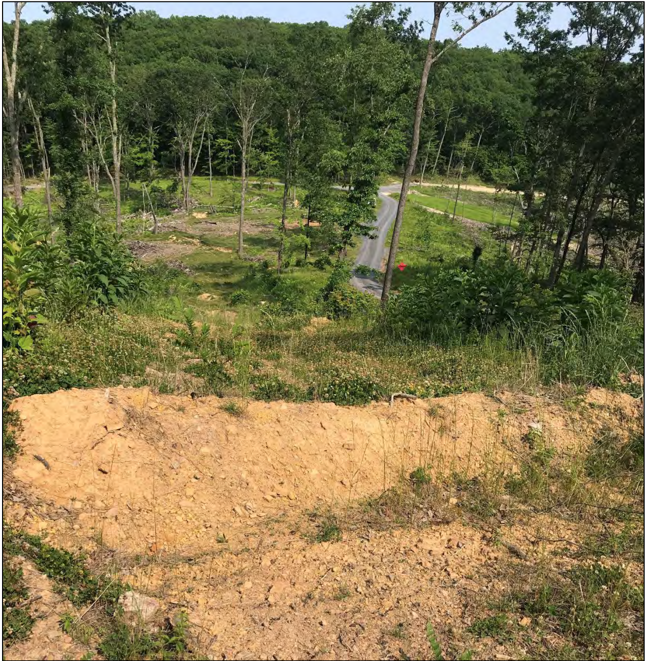
Figure 7 View of waterbar on skid road (bladed) in the Little Mountain Unit #3.
