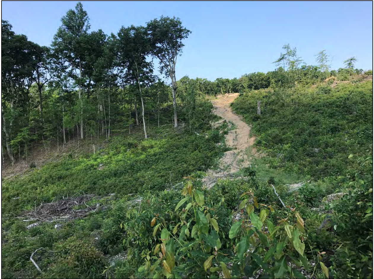
Figure 5 View of skid trail (bladed) with surface erosion in Porter's Mill Unit #7.
