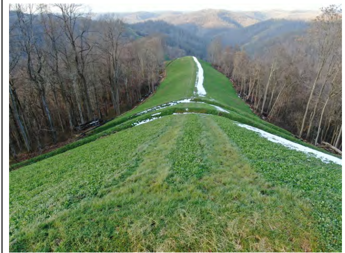
Spread A – The slope breakers along the ridge were functioning as designed (December 29, 2020) – MP 1.7 – Acceptable
