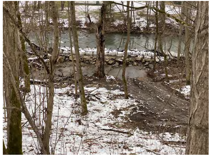
Spread G – This is the upstream sandbag placement of the new non-Project related work. Water this side of the sandbags is the same as the uppermost sinkhole from 2019 (December 28, 2020) – MP 200.6 – Communication
