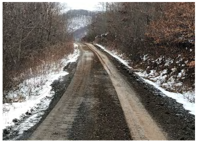
Spread E – The access road was recently plowed and cinder added to the road base for traction. Per Mountain Valley, the road was plowed by the non-Project related powerline company working in this area utilizing the same access road (December 29, 2020) – MP 143.6 – Communication
