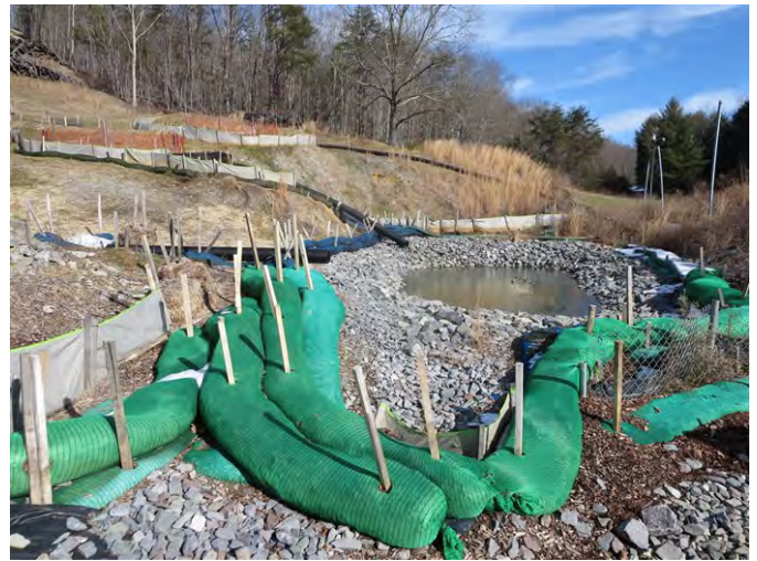
Spread F – Multiple temporary erosion controls were installed (December 30, 2020) – MP 194.7 – Acceptable
