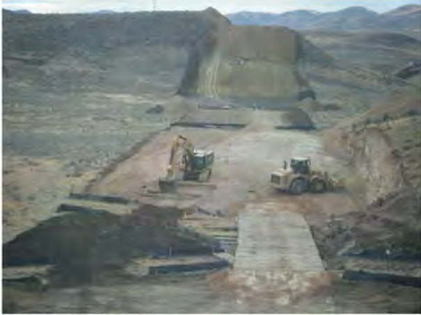
Figure 6. Backfilled crossing. This figure is available in colour online at wileyonlinelibrary.com/journal/rra
