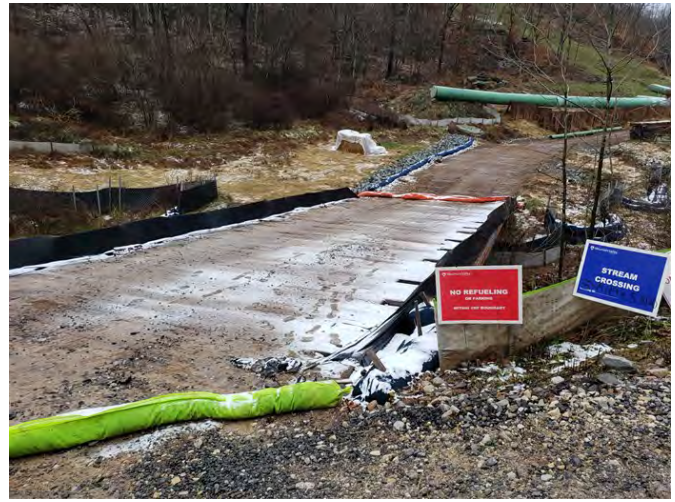
Spread A – No issues noted at stream S-A120 (January 2, 2021) – MP 6.7 – Acceptable
