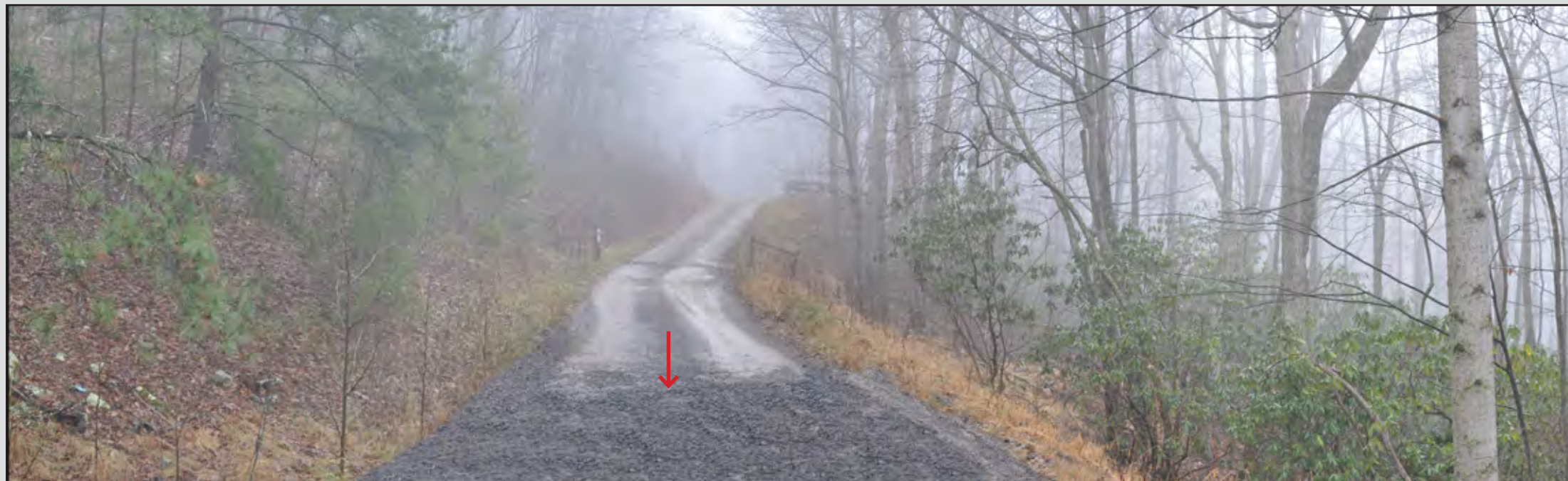
Post Construction - From this location modifications to the gravel in the roadway would be apparent in the immediate foreground where culvert upgrades would occur.
