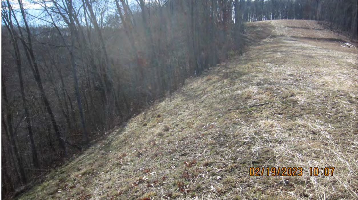
The pictures above show that MVP has removed all the silt fences and silt sock from this area. This will be a problem if the resume construction. You will see why when I file my complaint in a couple of days.
