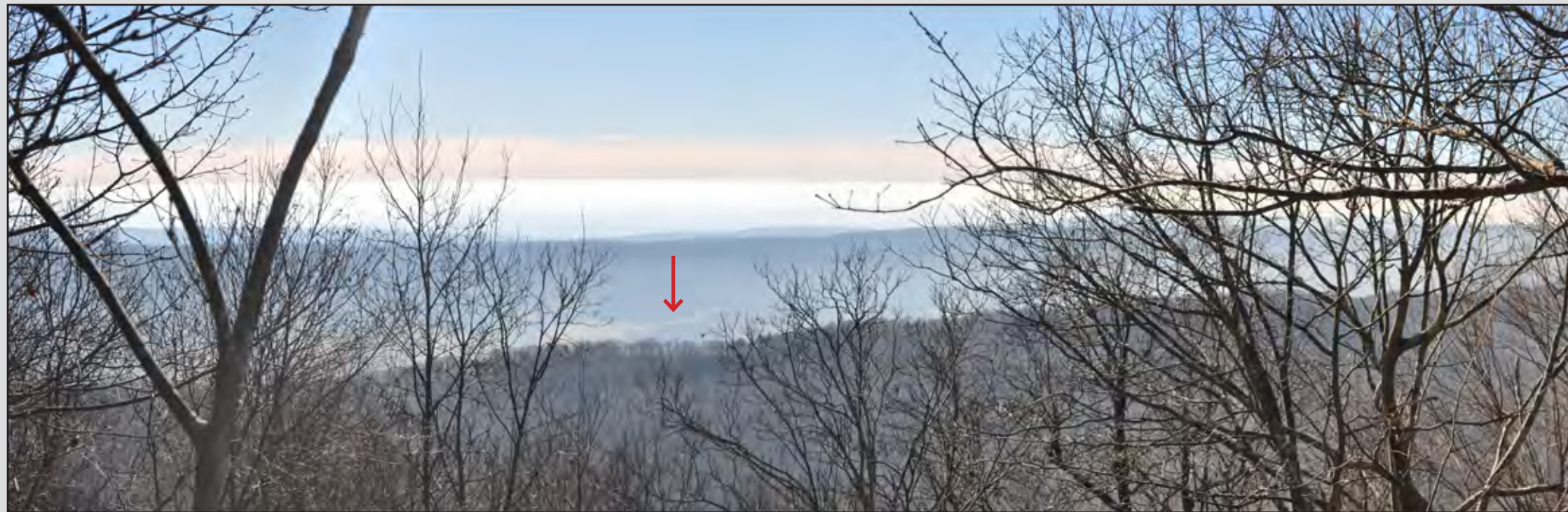
Post Construction - The proposed pipeline would cross along the base of Sinking Creek Mountain approximately 2.25 miles from an overlook located east of the Kelly's Knob overlook. The red arrow indicates where the proposed pipeline would be visible crossing in front of Sinking Creek Mountain. The proposed pipeline where it crosses over Peters Mountain is not visible from this viewpoint.
