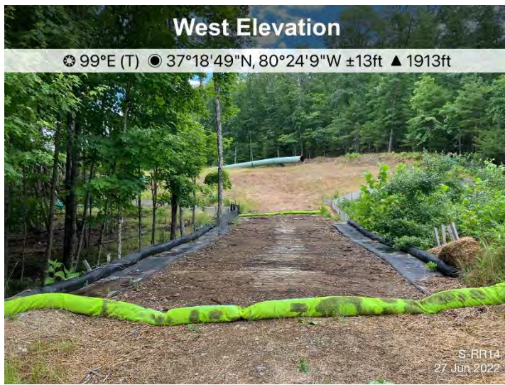
Figure 3: Designated crossing S-RR14, ESC's are in place and functioning.
