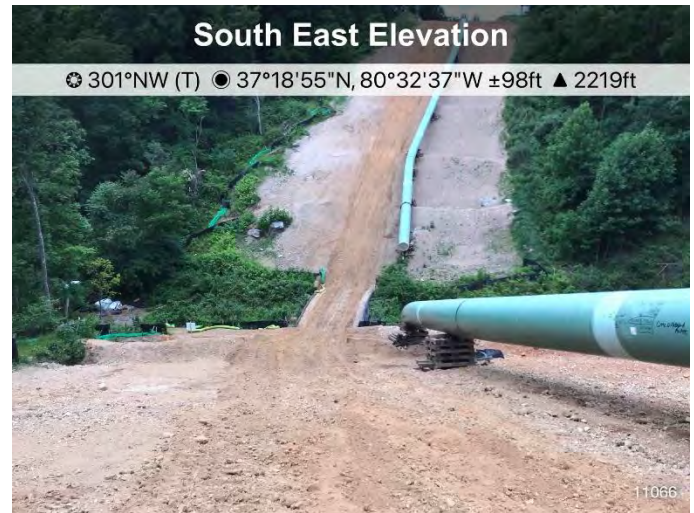
Figure 2: St11066 pipe has been strung and ECD's are in place.
