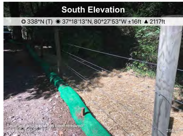
Figure 2: Escaped sediment and gravel has been removed and the area has been stabilized.
