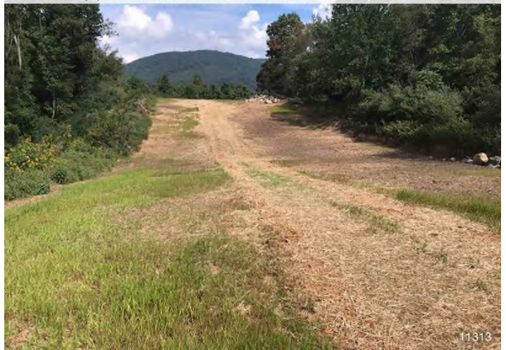
Figure 4: STA 11313+00 – Controls in place and functioning properly. Area stabilized with straw.
