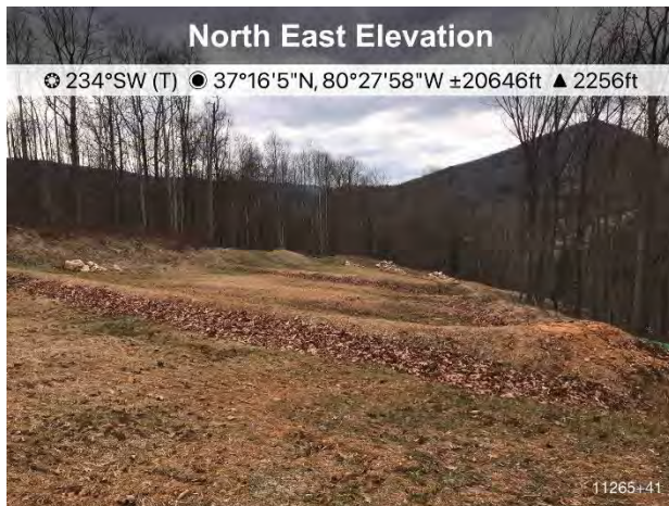
Figure 3. St11265+41 area is stabilized and ECD's are in place.
