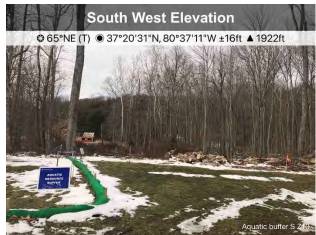
Figure 4: Aquatic Buffer for S-Z13, ESC controls were in place.
