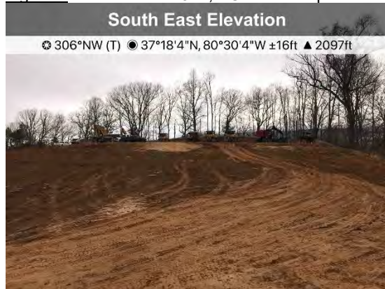
Figure 1: Near ATWS 1347, ECD's are in place.
