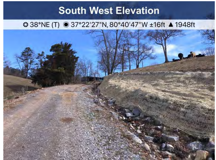
Figure 2: Blanket matted remains installed at AR GI- 234
