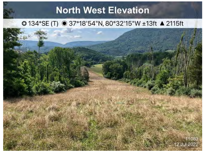
Figure 2: St11083, ECD's and stabilization are in place
