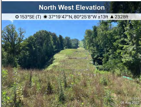
Figure 1: St11531 ECD's and stabilization are in place.
