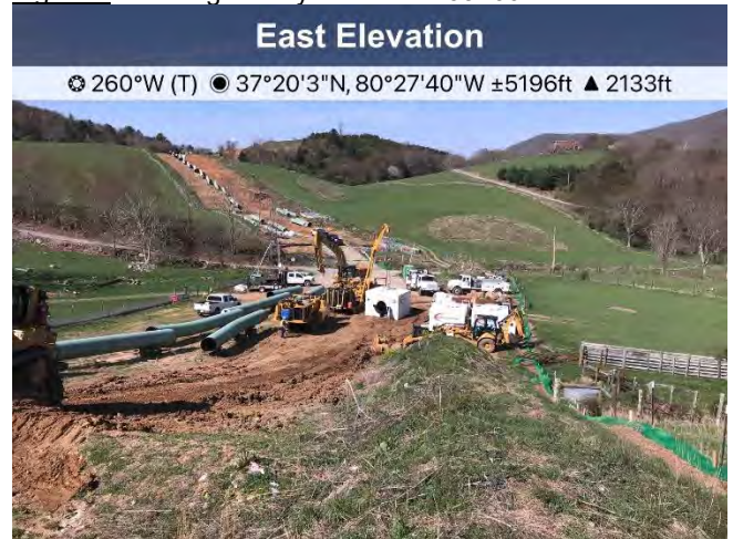
Figure 2: Welding activity near St11493+00.
