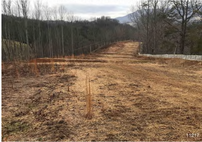
Figure 3: STA 11601+00 – Controls in place functioning properly. Area stabilized with straw.
