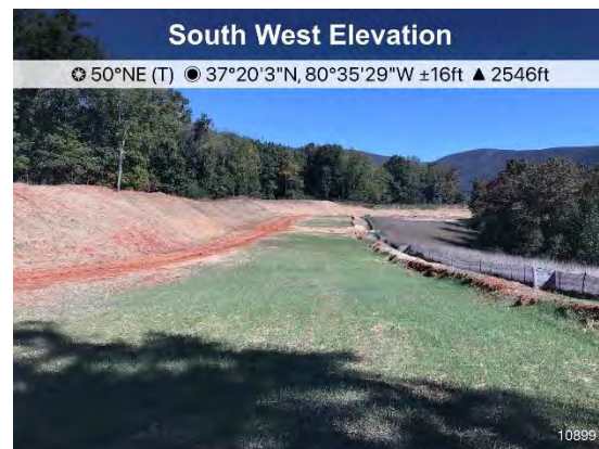
Figure 4: St 10899 area is stabilized and ECD's are in place.
