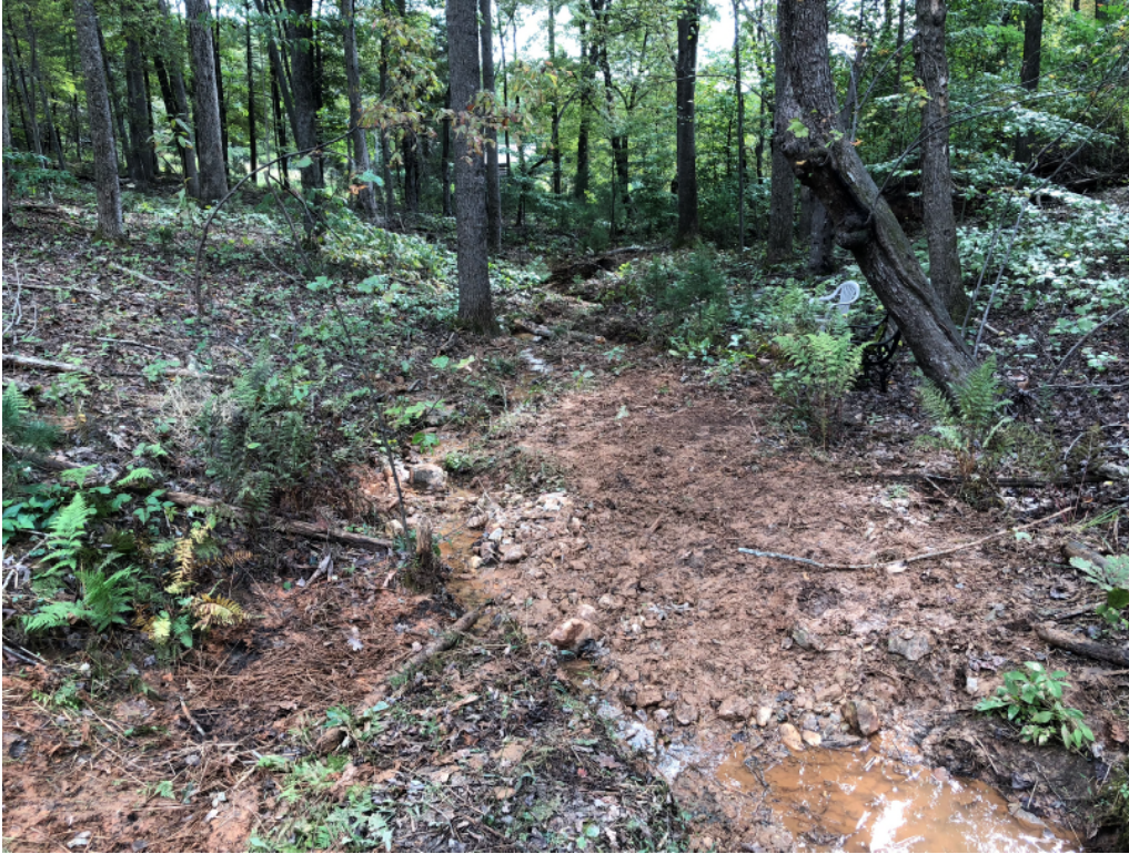
Photo 3: Sediment in stream and on banks at edge of RoW; Depth = 0.5-2" Orientation: Downstream
