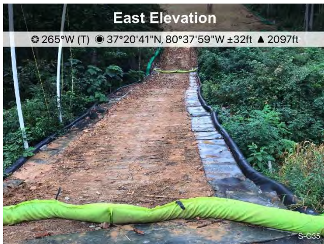
Figure 3: Designated crossing S-G35, ECD's are in place and functioning.
