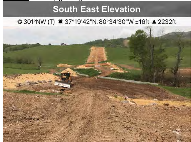
Figure 4: Actively grading near St10955
