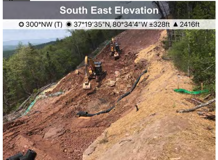
Figure 2: Active installation of CWD near St10977.
