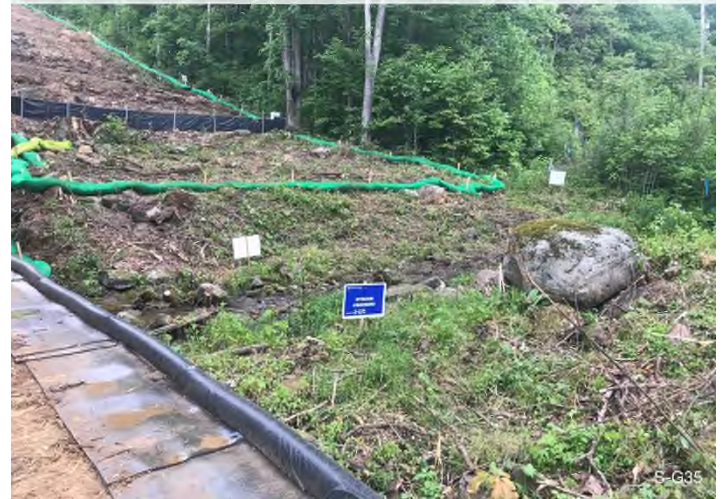
Figure 4: Stream S-G35 – Controls in place and functioning properly. BRG: 303°NW (T) LAT: 37.344790 LON: -80.633358 ±32ft ALT: 2124ft
