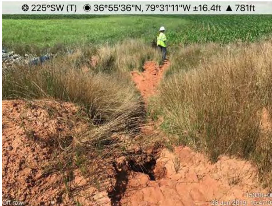
Figure 10 - Sediment deposits off ROW onto a farm field, near UT to Harpen Creek, June 28, 2019, DEQ Inspec. Rpt. Spread I, Source: DEQ
