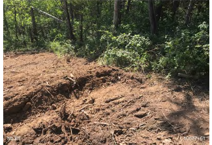
Figure 2: STA 10677+61 – Topsoil waterbar does not have end-treatment.
