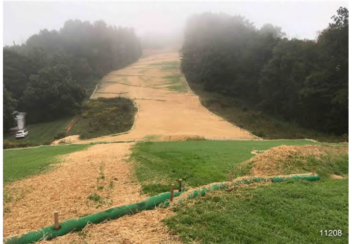
Figure 4: STA 11165+72 – Re-stabilize stockpile.
