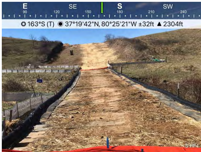
Figure 1: Designated crossing S-PP4, ESC's are in place and functioning.
