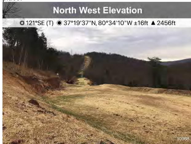
Figure 3: St10968 area has been stabilized and ECD's are in place.
