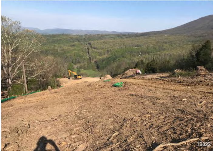
Figure 3: STA 10840+70 – Temp. topsoil WB does not have end-treatment.
