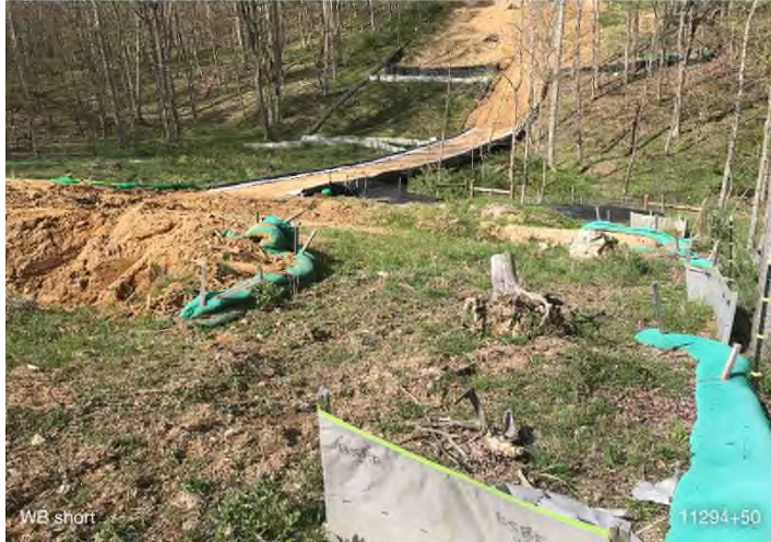
Figure 3: STA 11286+00 – Slope drain does not have outlet protection.
