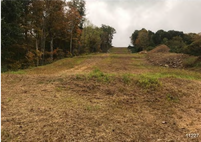
Figure 1: STA 11227+00 – Controls in place and functioning properly. BRG: 121°SE (T) LAT: 37.310555 LON: -80.516159 ±33914ft ALT: 1814ft
