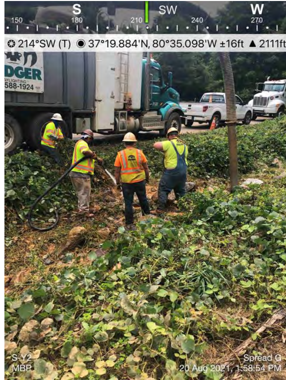
Figure 28 - Workers using a pressure washer and pump truck in an attempt to remove sediment deposited in Doe Creek from MVP worksites. August 20, 2021. Action Log ID 5068. Source: MBP
