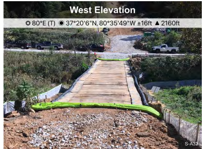
Figure 2: Designated crossing S-A32, ECD's are in place.
