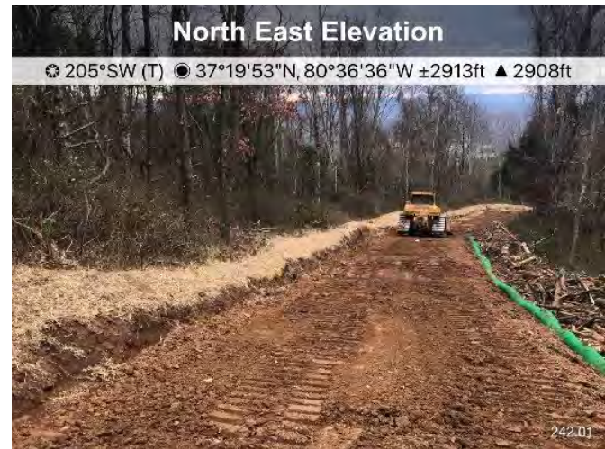
Figure 2: Construction of AR GI 242.01, ECD's have been installed.
