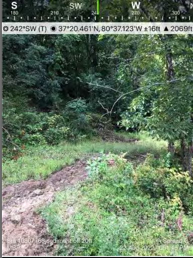
■ Figure 5: St10807+68 sediment has escaped off LOD.
