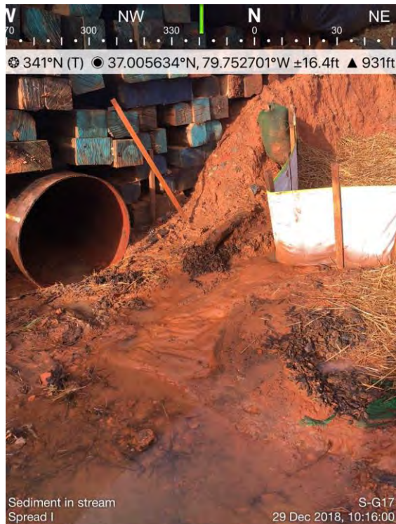
Figure 4 - Sediment deposited in UT Blackwater River, December 29, 2018, Action Log ID 1562, Source: MBP
