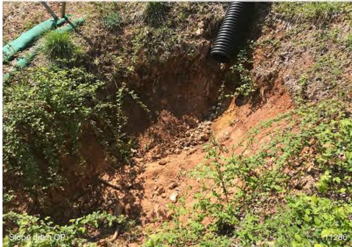
Figure 3: STA 11286+00 – Slope drain does not have outlet protection.
