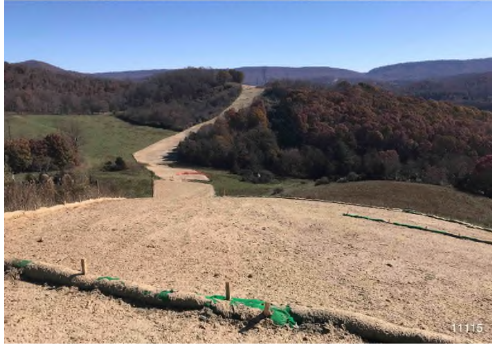
Figure 4: STA 11151+00 – Controls in place and functioning properly. Area stabilized with straw.
