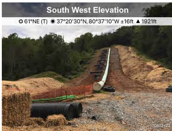
Figure 3: St 10803+20 ECD's are in place.
