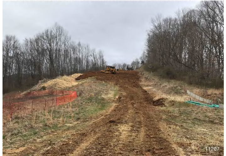
Figure 2: STA 11207+00 – Controls in place and functioning properly. BRG: 333°NW (T) LAT: 37.303751 LON: -80.506530 ±16ft ALT: 1957ft
