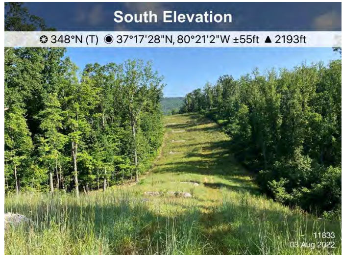
Figure 4: St11833, ECD's and stabilization are in place.
