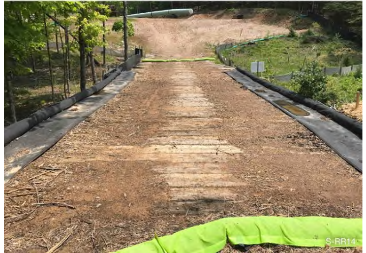
Figure 2: Stream S-RR14 – Controls in place and functioning properly around S-RR14 BRG: 110°E (T) LAT: 37.314042 LON: -80.402567 ±2805ft ALT: 1897ft
