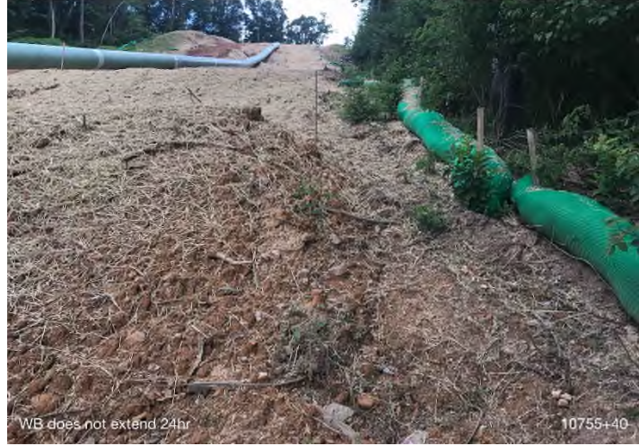
Figure 7: STA 10755+40 – Waterbar does not extend full length of the ROW.
