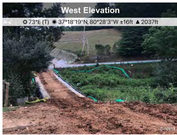
Figure 3: Designated crossing S-NN11
