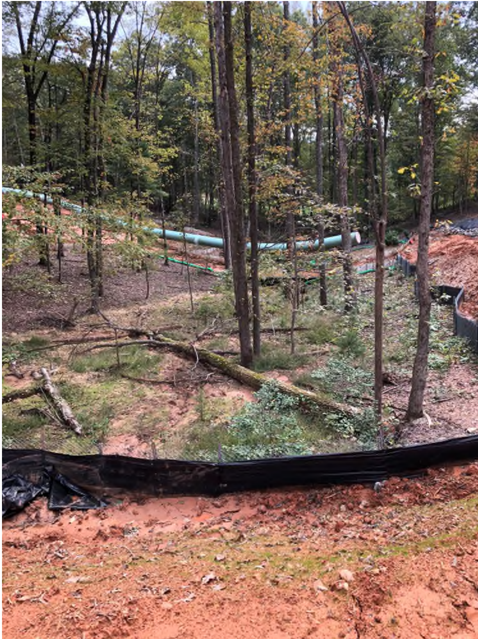
Photo 4: Overview of stream crossing and sediment within forested buffer Orientation: SE
