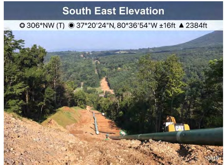
Figure 4: St 10818 ECD ongoing maintenance
