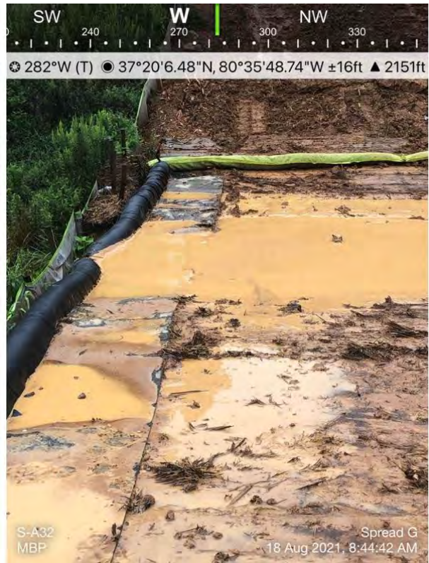
Figure 31 - Sediment deposited in UT Doe Creek, August 18, 2021, Action Log ID 565, Source: MBP
