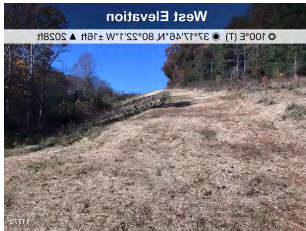
Figure 3: St11770 ECD's are in place and area is stabilized.
