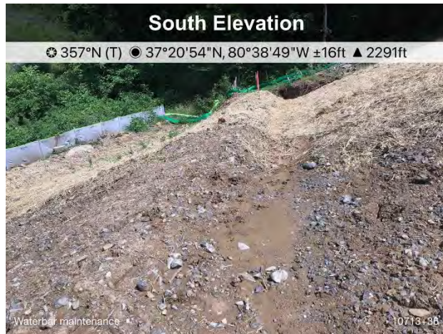
Figure 1: St10713+36 sediment in flow path
