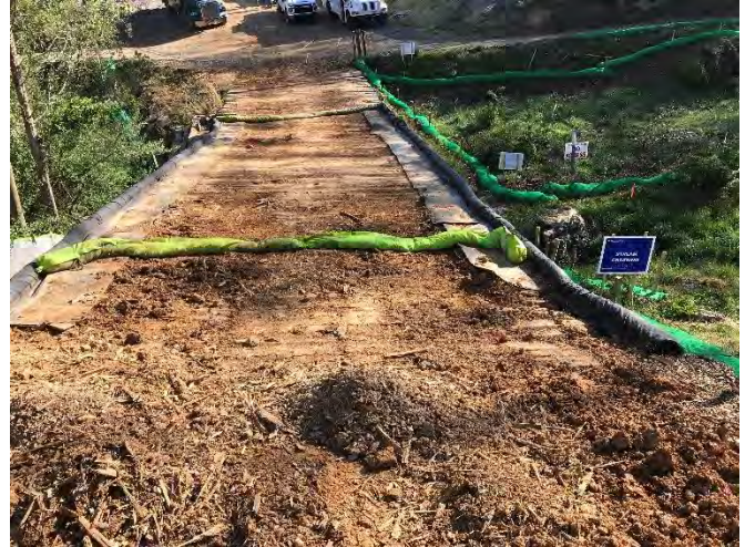
Figure 2: Designated crossing S-NN11, ECD's are in place.
