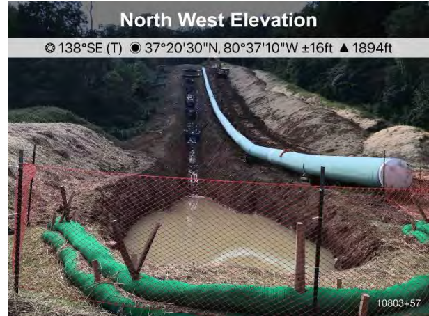
Figure 2: St 10803+57 ECD installed at base of trench.
