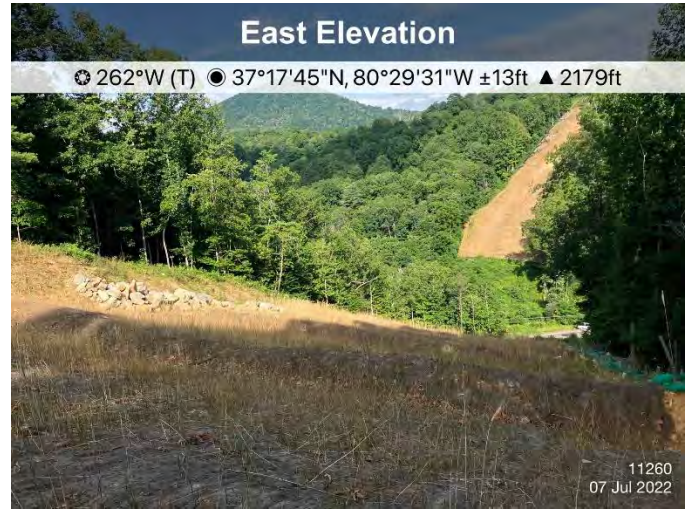
Figure 2: St11260, ECD's and stabilization are in place
