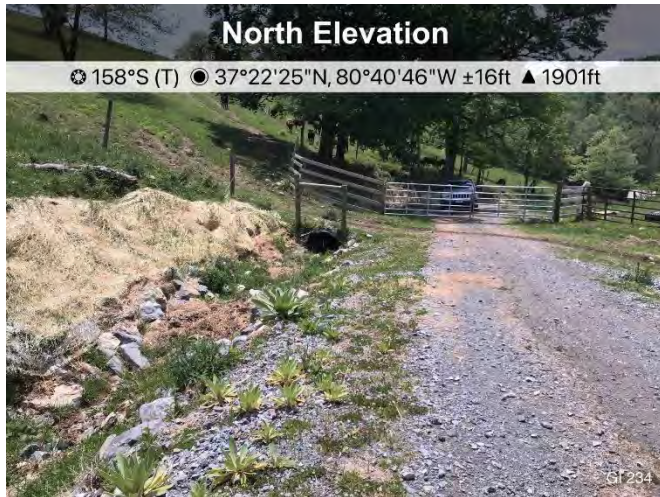
Figure 1: Access road GI 234 matting remains installed.
