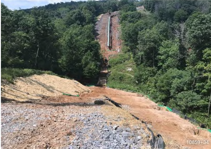
Figure 1: STA 10859+34 – Controls in place and functioning properly. BRG: 310°NW (T) LAT: 37.337414 LON: -80.604308 ±16ft ALT: 2326ft
