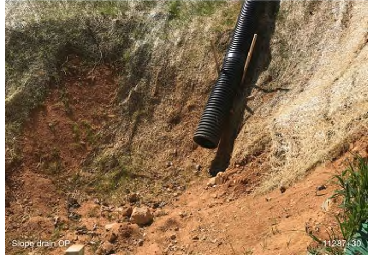
Figure 4: STA 11281+75 – Slope drain does not have outlet protection.
