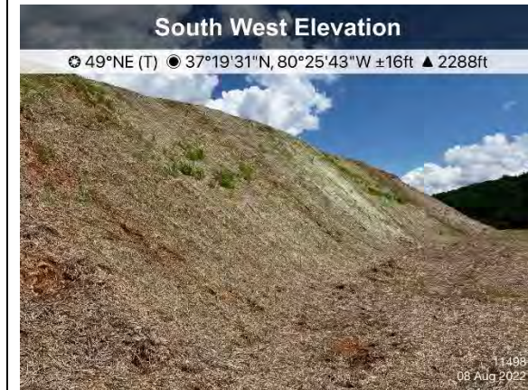
Figure 2: St11498, ECD's and stabilization are in place.
