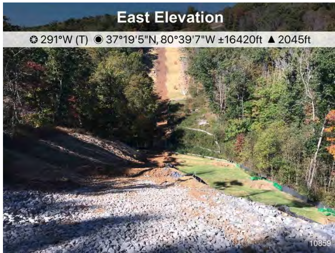
Figure 1: St 10859 ECD's are in place and area has been stabilized.
