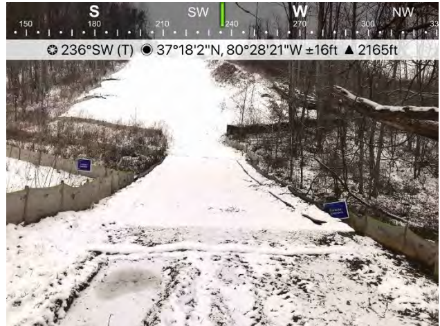
Figure 4: Designated crossing S-NN12 ECD's are in place.
