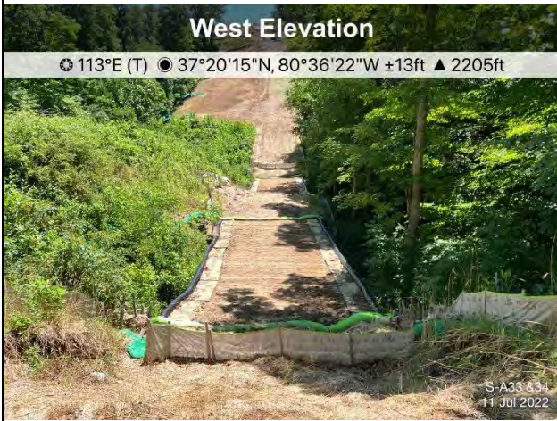
Figure 3: Designated crossing S-A33&34, ECD's are in place.
