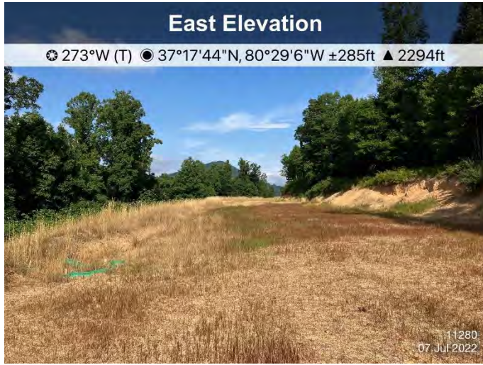
Figure 1: St11280, ECD's and stabilization are in place.
