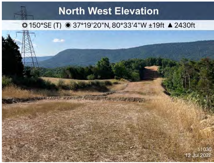
Figure 1: St11030, ECD's and stabilization are in place.
