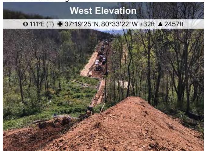
Figure 4: Above designated crossing S-RR5, additional ECD crews are mobilizing.
