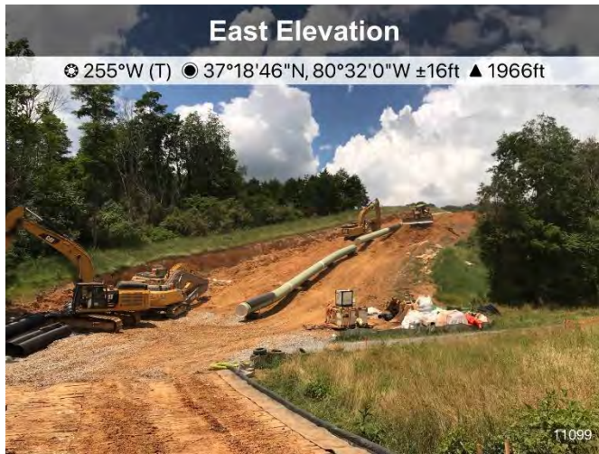
Figure 1: St11099 grading activities, ECD's are in place.
