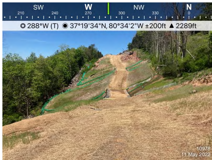
Figure 3: STA 10978+00 – Controls in place and functioning properly. Area stabilized with straw.
