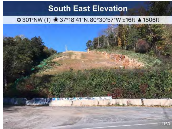
Figure 2: St 11160 Mountain Lake road crossing, ECD's are in place and slope is stabilized.
