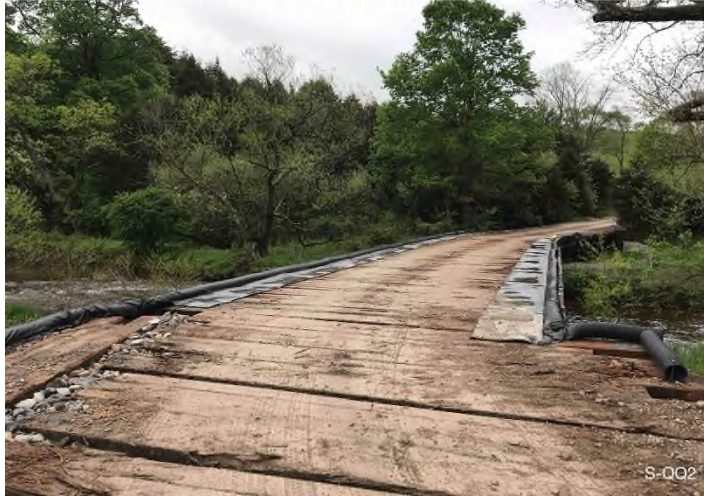
Figure 1: Stream S-QQ2 – Controls in place and functioning properly around stream crossing. (Sinking Creek) BRG: 178°S (T) LAT: 37.333126 LON: -80.431150 ±541ft ALT: 2008ft
