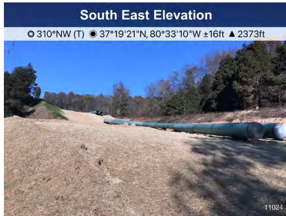
Figure 1: St11024 area is stabilized and ECD's are in place.
