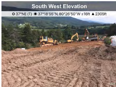
Figure 3: St 11428 on going grading activities and permanent stabilization.
