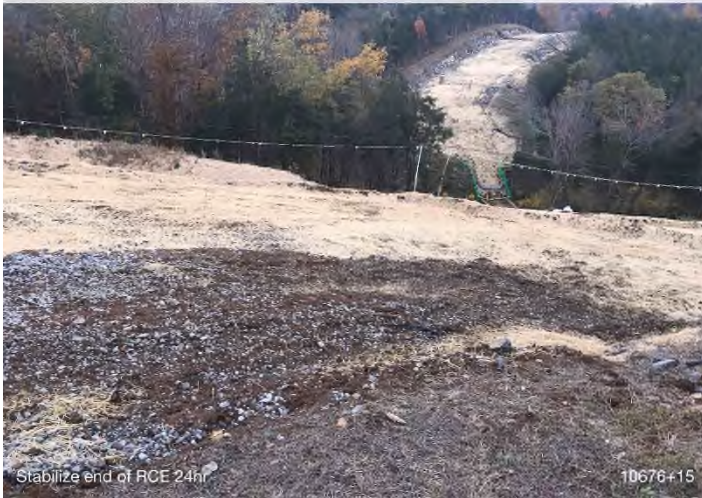
Figure 3: STA 10676+15 – Stabilization needed.
