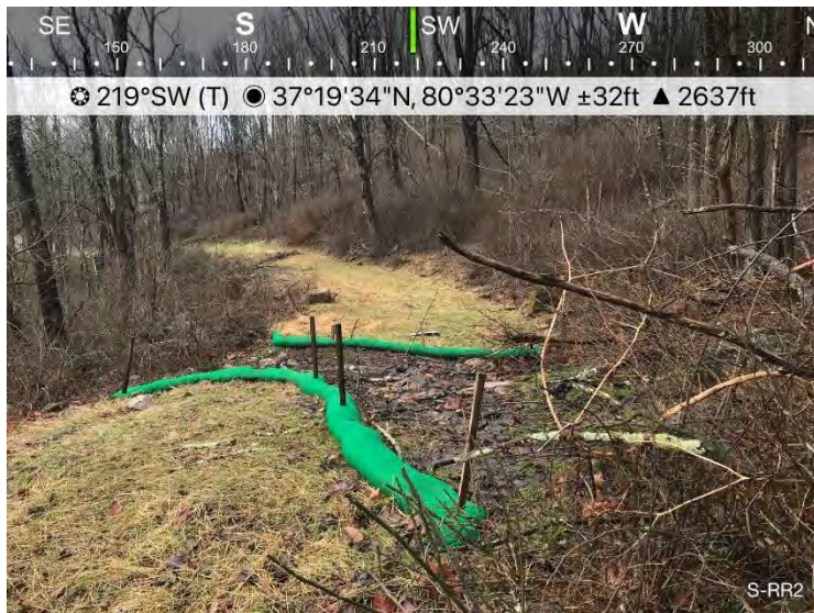
Figure 1: Designated crossing S-RR2, ESC's are in place and functioning.
