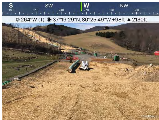
Figure 3: St 11492+87, ECD's are in place and functioning.
