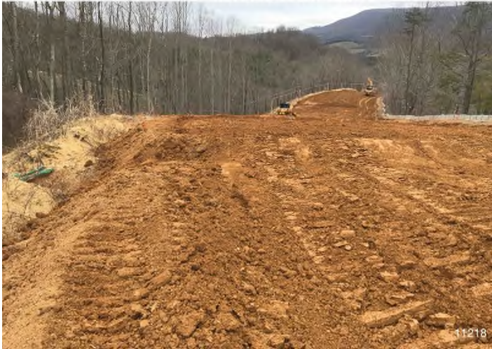
Figure 1: STA 11218+00 – Controls in place and functioning properly. BRG: 300°NW (T) LAT: 37.301381 LON: -80.503930 ±16ft ALT: 2080ft
