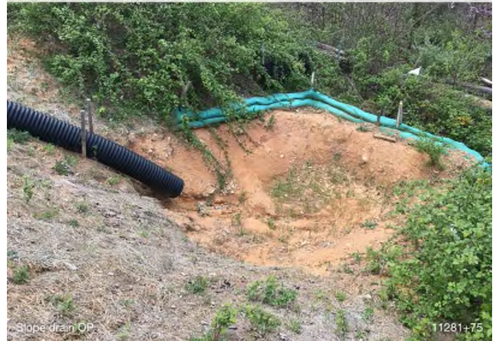
Figure 4: STA 11281+75 – Slope drain does not have outlet protection.
