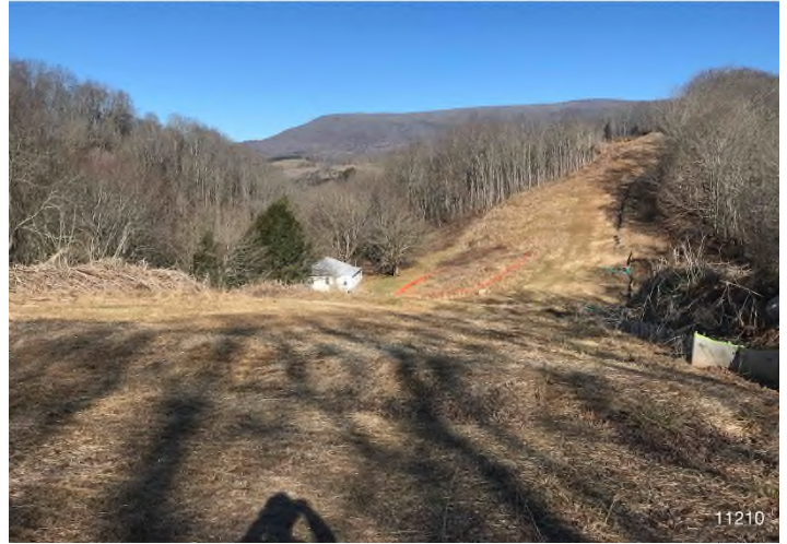
Figure 4: STA 11180+00 – Controls in place and functioning properly. Area stabilized with straw.
