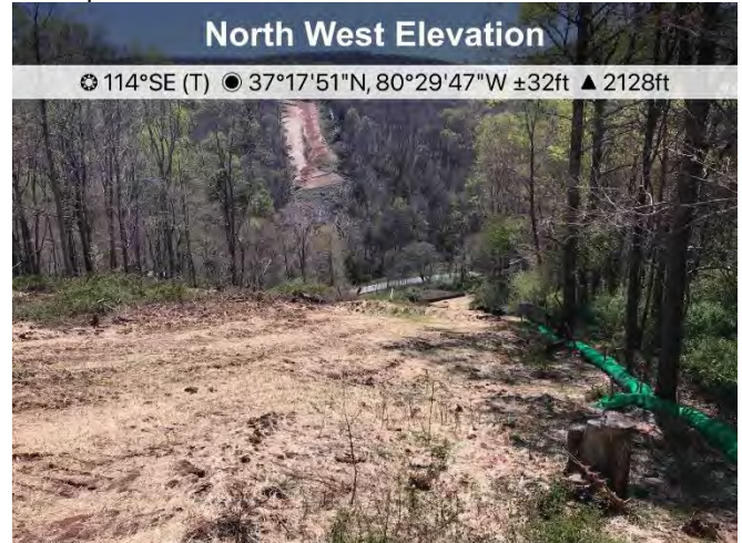
Figure 2: Near St11246+83, area has been stabilized and ECD's are in place.
