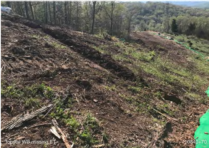
Figure 3: STA 10840+70 – Temp. topsoil WB does not have end-treatment.
