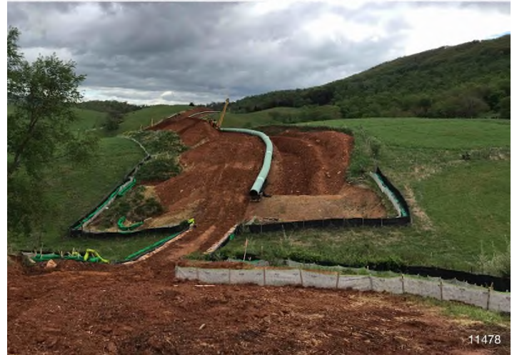
Figure 4: STA 11478+00 – Controls in place and functioning properly. BRG: 65°NE (T) LAT: 37.280701 LON: -80.388092 ±6562ft ALT: 2148ft
