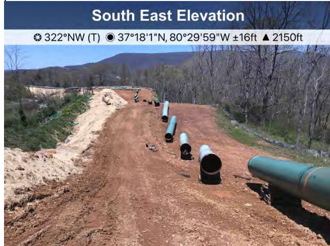
Figure 1: Near St11233, pipe has been strung and ECD's are in place.
