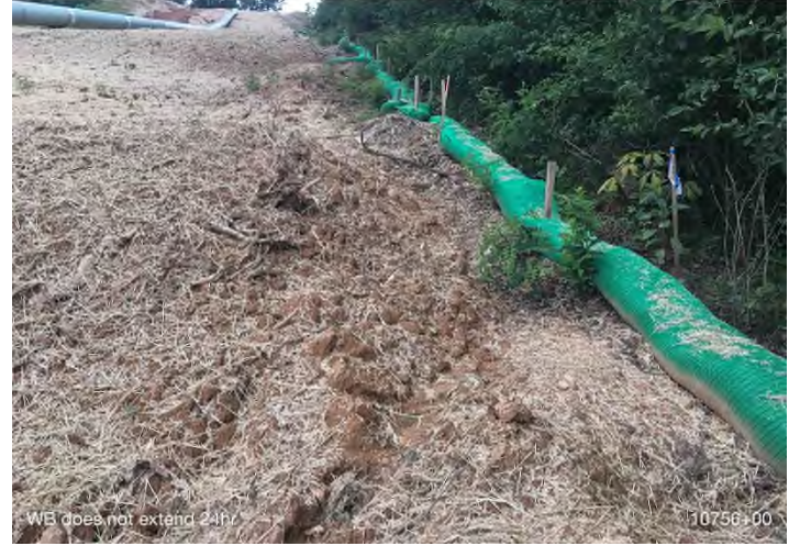
Figure 6: STA 10756+00 – Waterbar does not extend full length of the ROW.
