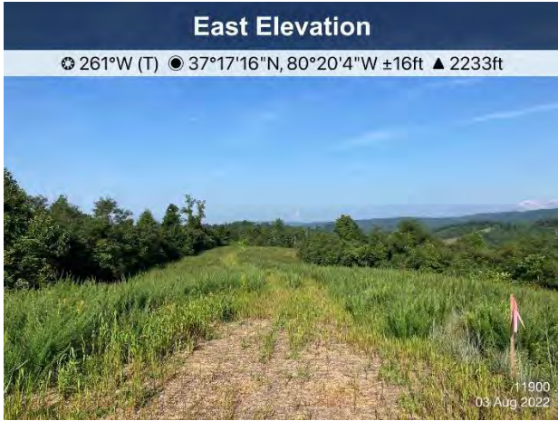
Figure 1: St11900 ECD's and stabilization are in place.
