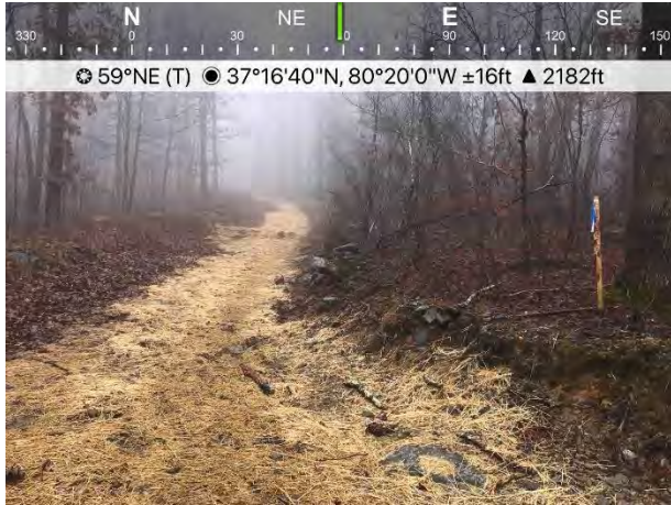
Figure 1: AR –MN266 has been stabilized with mulch.
