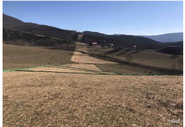
Figure 4: STA 10940+00 – Controls in place and functioning properly. Area stabilized with straw. BRG: 189°S (T) LAT: 37.330028 LON: -80.579988 ±16ft ALT: 2282ft
