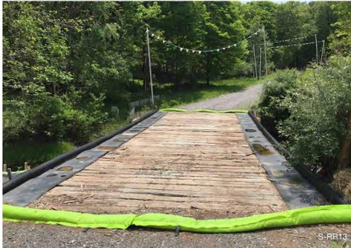
Figure 1: Stream S-RR13 – Controls in place and functioning properly around Craig Creek. BRG: 128°SE (T) LAT: 37.314629 LON: -80.402699 ±16ft ALT: 1878ft
