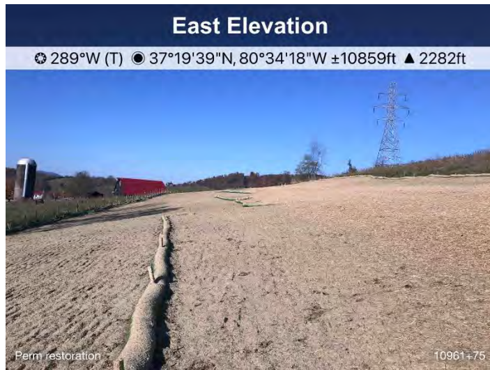
Figure 3: St10961+75 permanent restoration has been applied.
