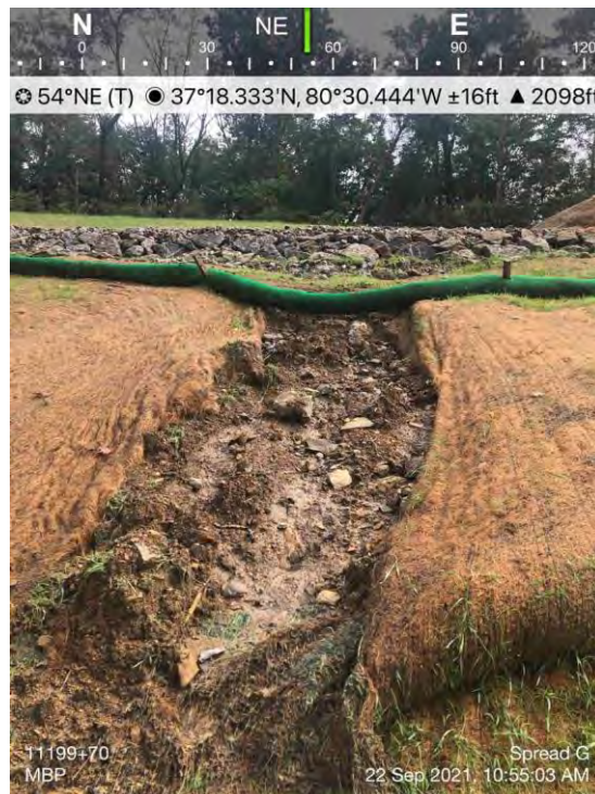
Figure 24 - Compost filter sock undermined near Sinking Creek, September 22, 2021, Action Log ID 5196, Source: MBP
