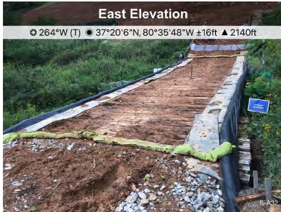
Figure 1: Designated crossing S-A32, ECD's are in place.
