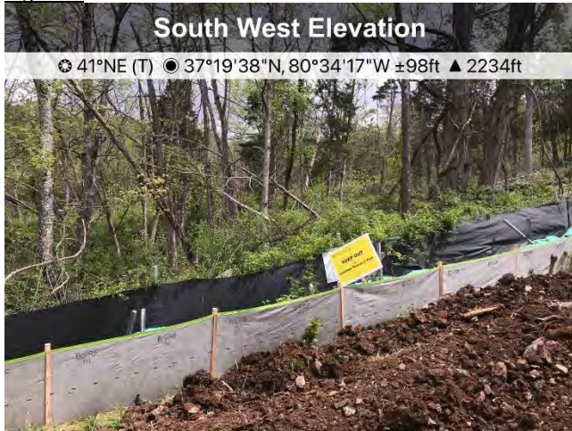
Figure 3: Protected area neat St 10965+51
