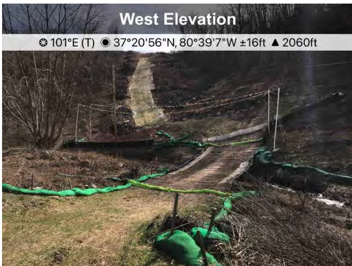
Figure 3: Designated crossing S-G32, ECD's are in place and functioning.
