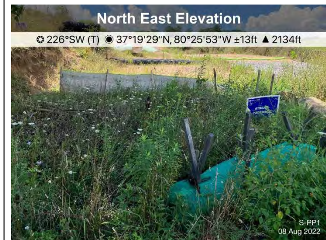
Figure 4: Designated crossing S-PP1, ECD's and stabilization are in place.
