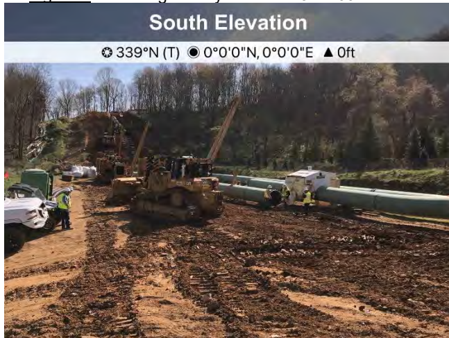
Figure 1: Lowering activity near St11524+00.
