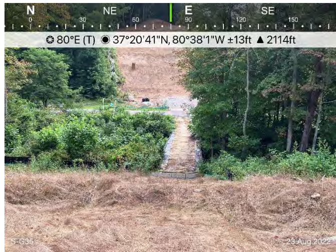
Figure 4: Designated crossing S-G35, ECD's are in place.
