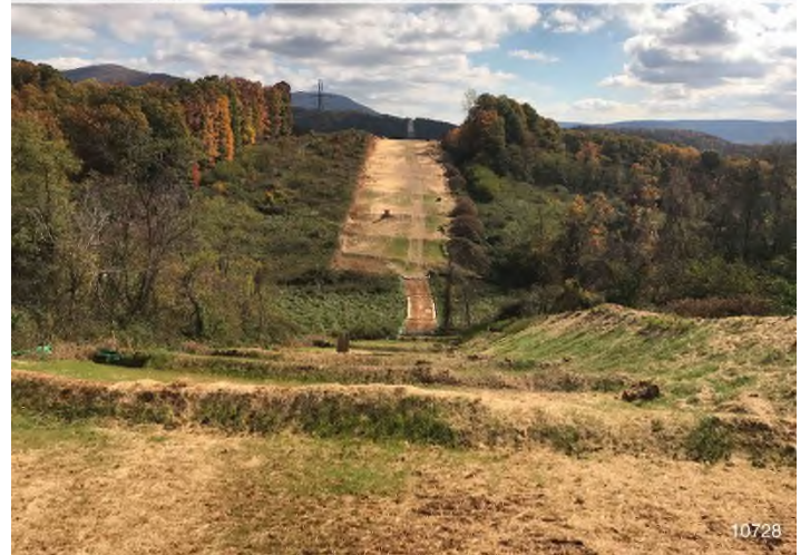
Figure 4: STA 10728+00 – Controls in place and functioning properly. Area stabilized with straw.
