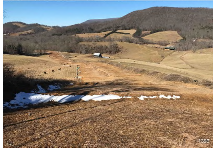
Figure 4: STA 11494+00 – Controls in place and functioning properly. Area stabilized with straw.
