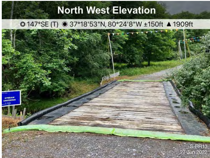
Figure 1: Designated crossing S-RR13, ESC's are in place and functioning.
