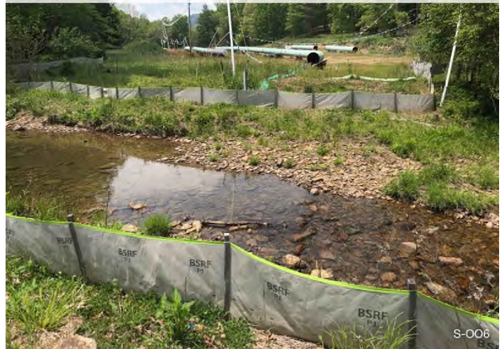
Figure 4: Stream S-006 – Controls in place and functioning properly around Craig Creek. BRG: 261°W (T) LAT: 37.313637 LON: -80.404490 ±16ft ALT: 1901ft
