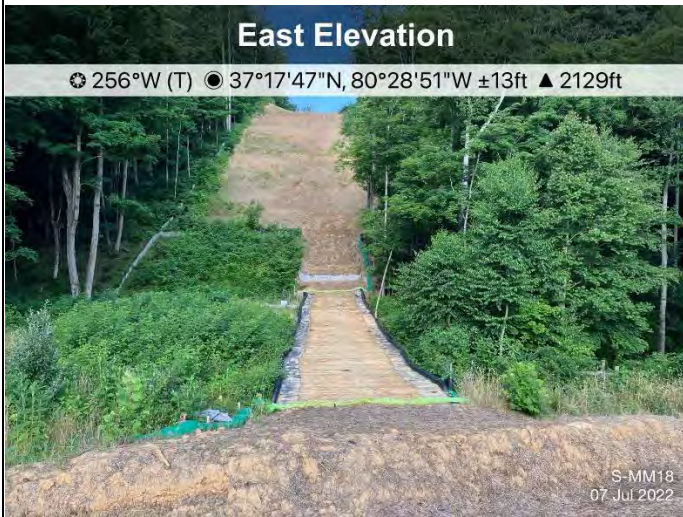
Figure 3: Designated crossing S-MM18, ECD's are in place.
