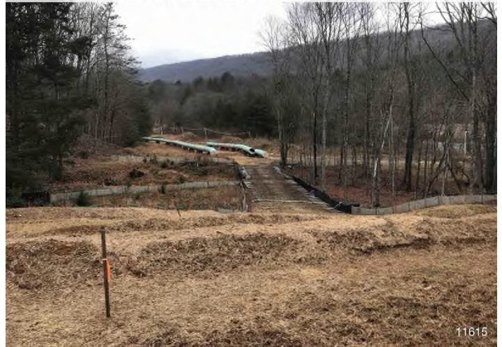
Figure 4: STA 11615+00 – Controls in place functioning properly. Area stabilized with straw.
