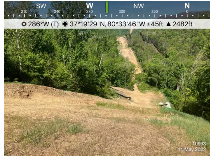
Figure 4: STA 10968+00 – Controls in place and functioning properly. Area stabilized with straw.
