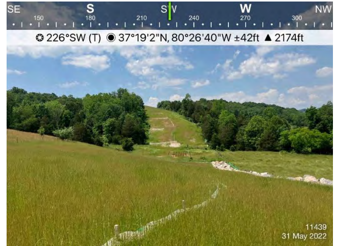
Figure 2: St11439 ECD's and stabilization in place.
