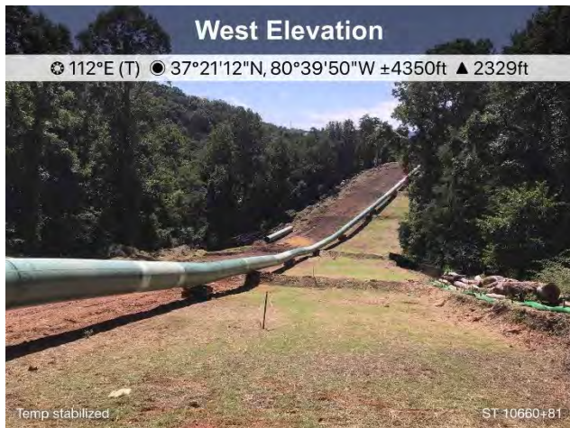
Figure 7: St10660+81 area is temporarily stabilized
