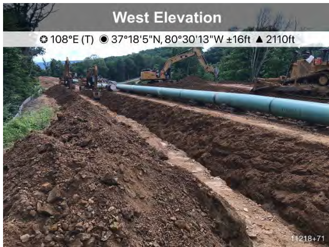
Figure 3: St11218+71 active trenching
