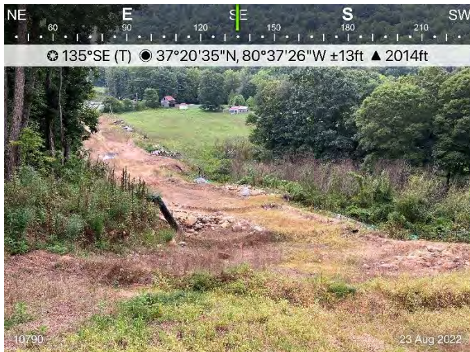
Figure 3: St10790, ECD's and stabilization are in place.
