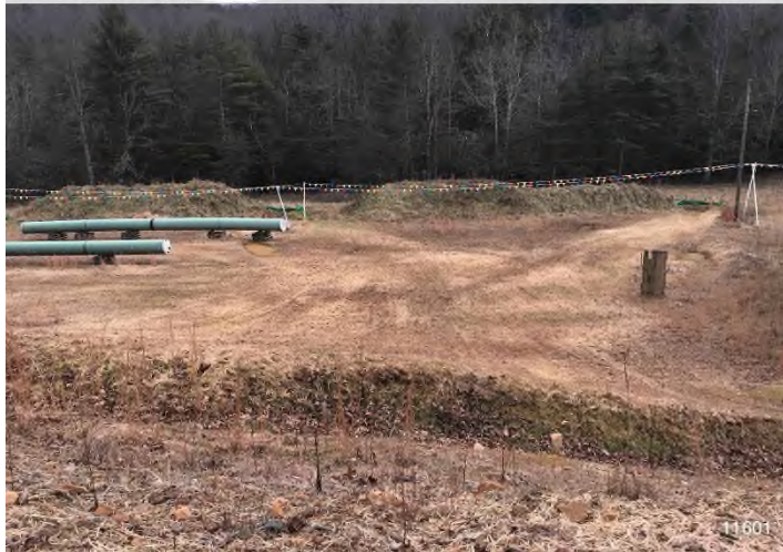
Figure 3: STA 11601+00 – Controls in place functioning properly. Area stabilized with straw.
