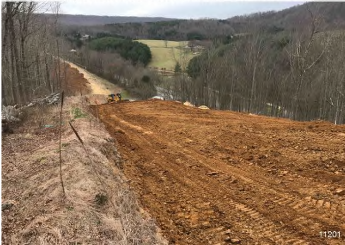
Figure 3: STA 11201+00 – Controls in place and functioning properly. BRG: 184°S (T) LAT: 37.305400 LON: -80.507007 ±32ft ALT: 2000ft
