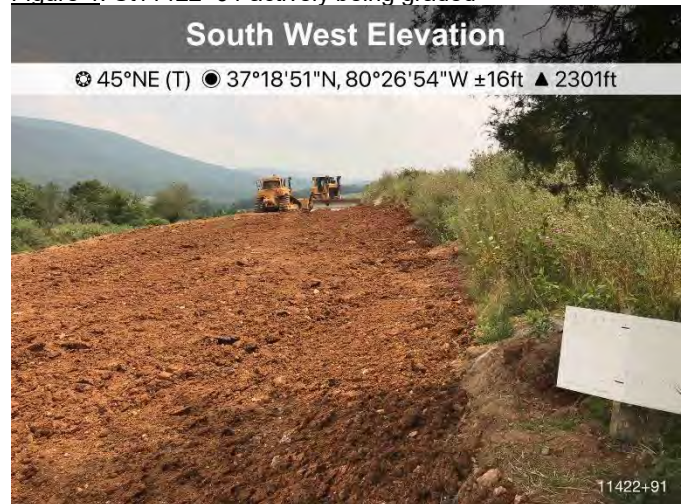
Figure 4: St11422+91 actively being graded
