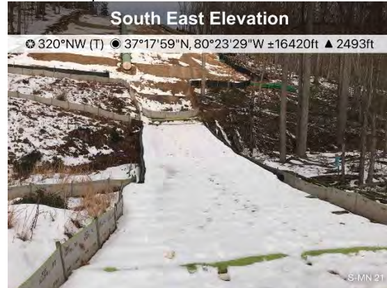
Figure 2: Designated stream crossing S-MN21, ESC controls were in place.
