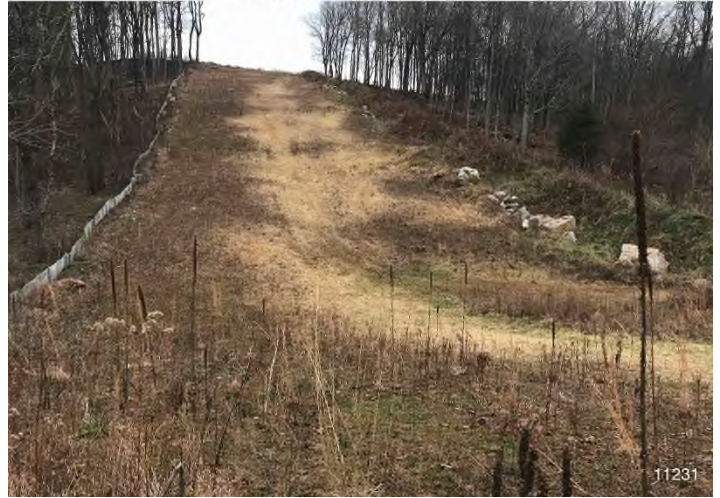
Figure 4: STA 11615+00 – Controls in place functioning properly. Area stabilized with straw.
