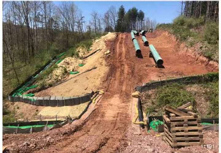
Figure 4: STA 11191+00 – Controls in place and functioning properly. BRG: 319°NW (T) LAT: 37.306628 LON: -80.509749 ±32ft ALT: 2023ft
