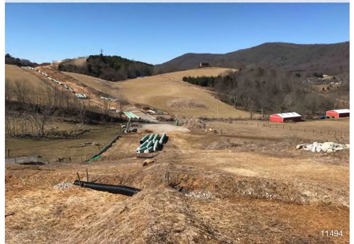
Figure 4: STA 11494+00 – Controls in place and functioning properly. Area stabilized with straw.
