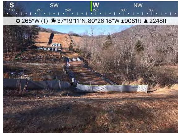
Figure 4: Designated stream S-0013, ECD's are in place.
