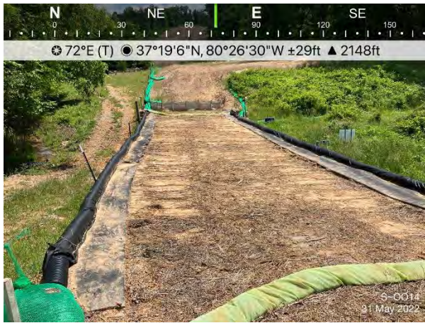
Figure 3: Designated crossing S-0014, ESC's are in place and functioning.
