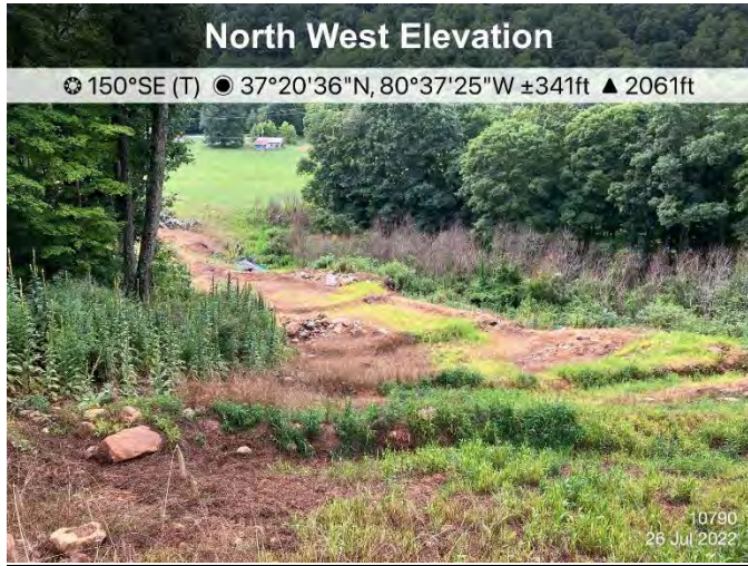
Figure 1: St10790, ECD's and stabilization are in place.
