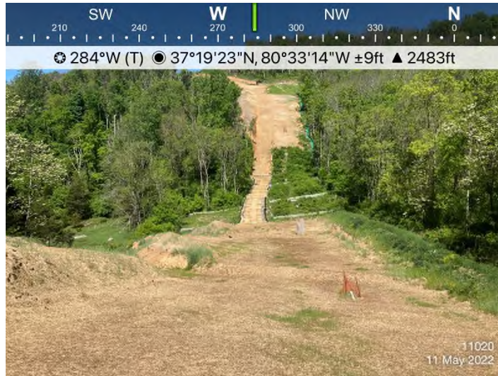
Figure 3: STA 10978+00 – Controls in place and functioning properly. Area stabilized with straw.
