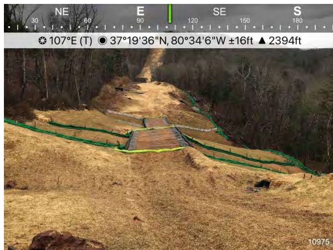
Figure 3: St10975, ECD's are in place and functioning.
