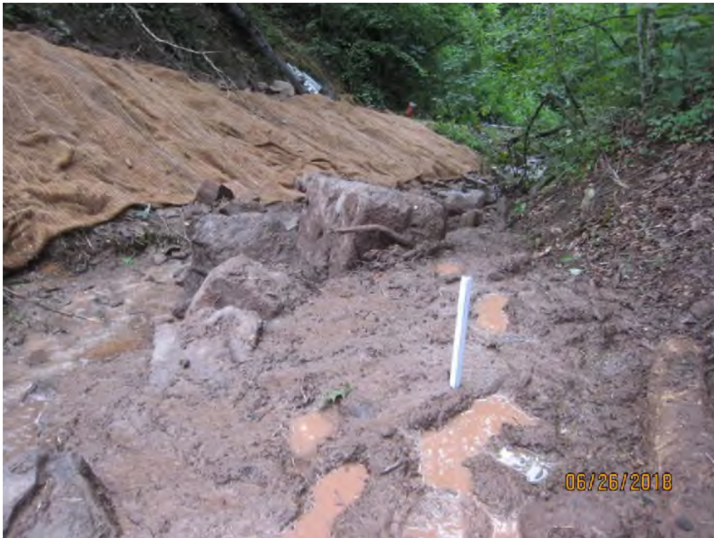
Photo 1: Sedimentation within "Stream 39" ~25' downstream of LOD
