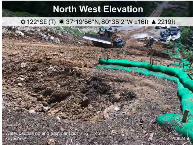
▪ Figure 5: St 10924{+56 water bar end treatment not keyed in
