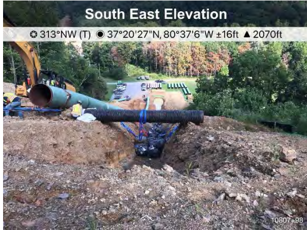
Figure 1: Additional control installed near St 10807+98
