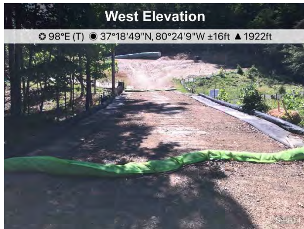
Figure 3: Designated crossing S-RR13, ECD's are in place.
