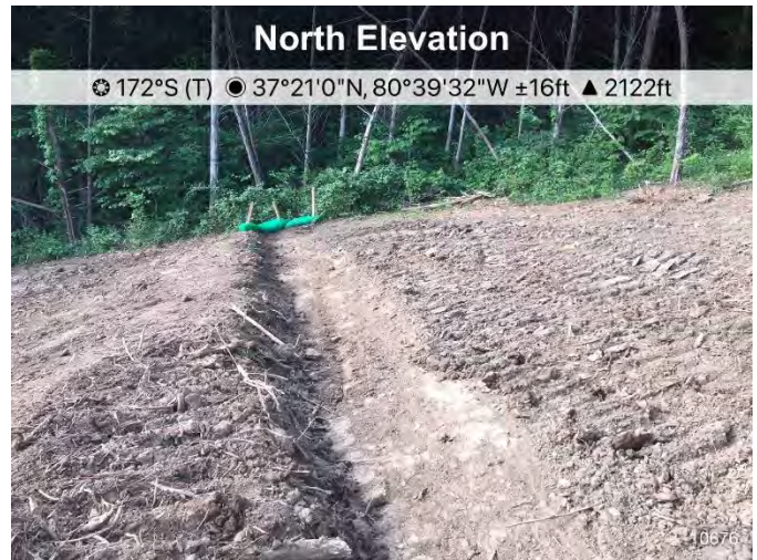
Figure 2: Installation of temporary waterbar at St10676.
