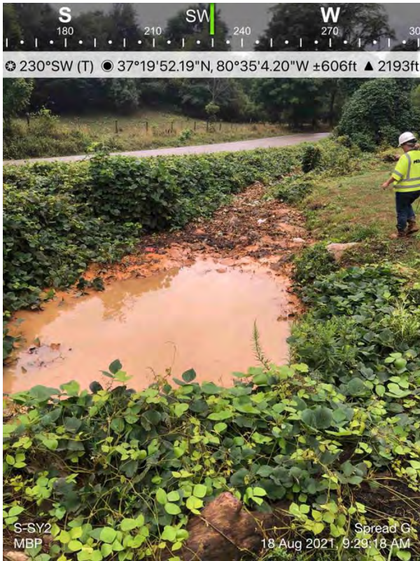
Figure 26 - Sediment deposited in Doe Creek, August 18, 2021, Action Log ID 5068, Source: MBP
