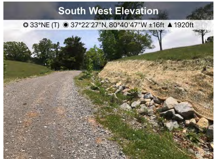
Figure 2: Access road GI 234 matting remains installed.
