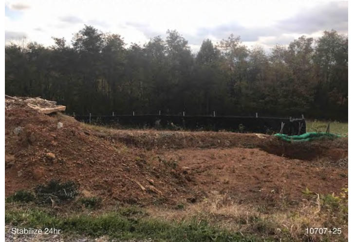
Figure 4: STA 10728+00 – Controls in place and functioning properly. Area stabilized with straw.
