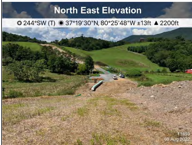
Figure 3: St11493, ECD's and stabilization are in place.
