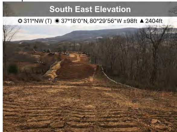
Figure 2: Above St11230+00 ECD's and stockpile stabilization in place.
