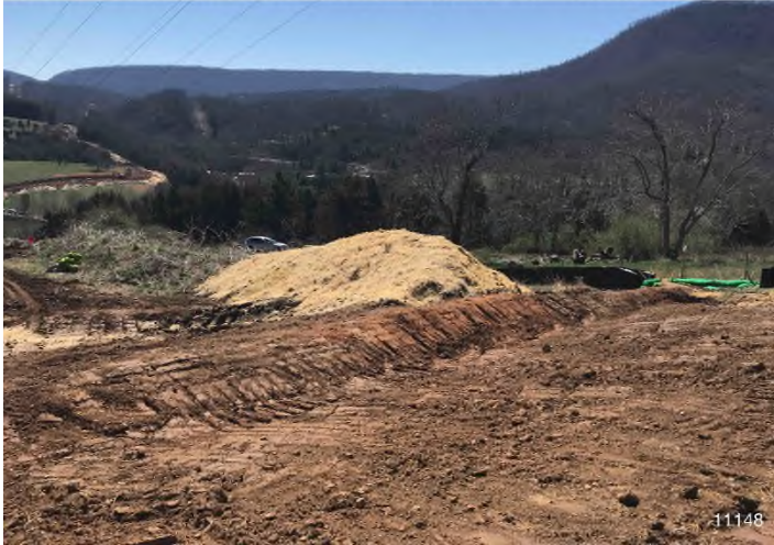
Figure 1: STA 11148+00 – Controls in place and functioning properly. BRG: 153°SE (T) LAT: 37.306572 LON: -80.509770 ±11398ft ALT: 1865ft
