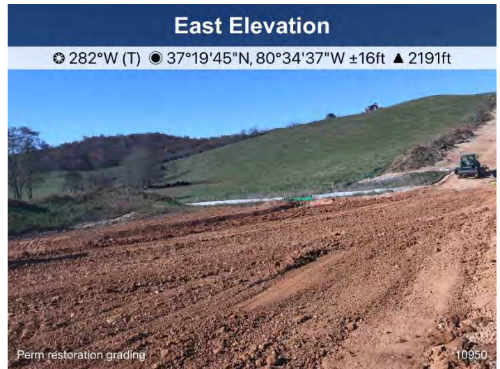
Figure 4: St10950 active restoration grading.
