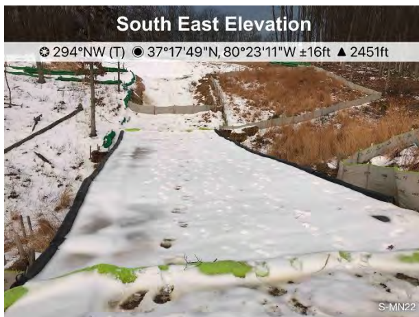
Figure 3: Designated stream crossing S-MN22, ESC controls were in place.
