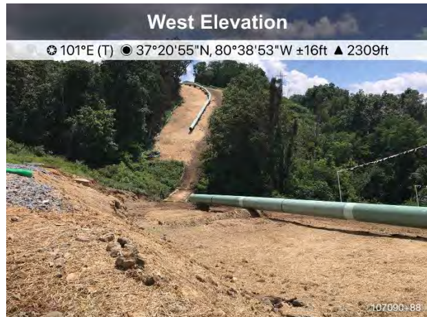
Figure 8: Stabilized area near St10709+88
