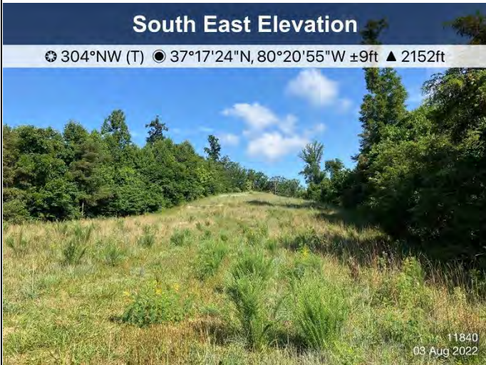
Figure 3: St11840, ECD's and stabilization are in place.
