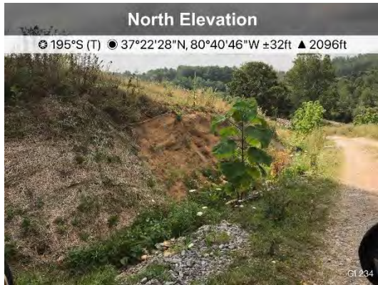
Figure 1: AR GI 234 ditch line
