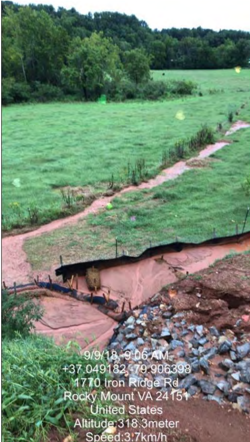
Figure 12 - Sediment off ROW near UT Little Creek, September 9, 2018, Source: citizen observer, accessible at Virginia Pipeline Violations Facebook page
