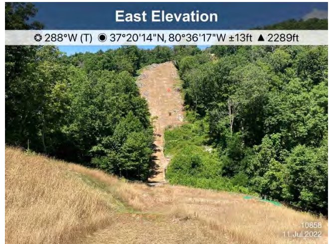
Figure 4: St10858, ECD's and stabilization are in place.
