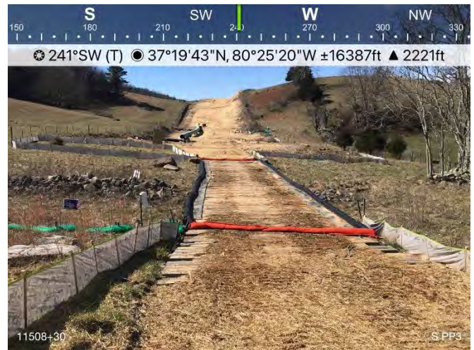
Figure 2: Designated crossing S-PP3, ESC's are in place and functioning.
