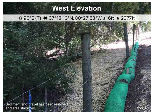
Figure 4: Escaped sediment and gravel has been removed and the area has been stabilized.
