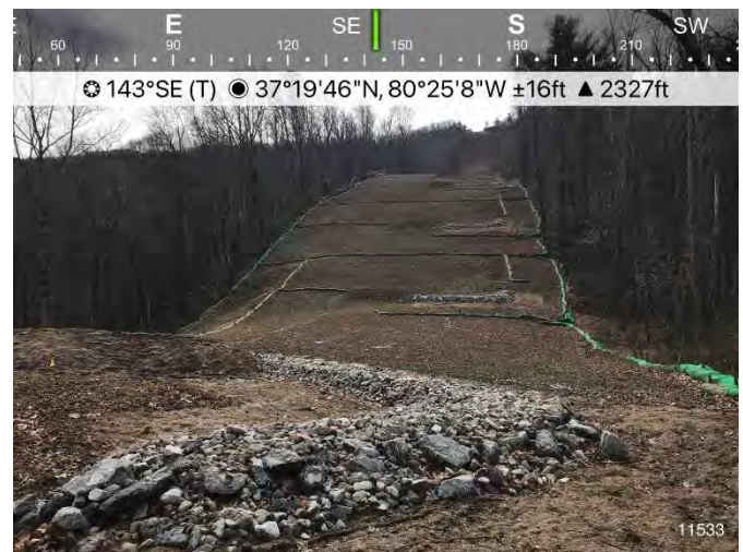
Figure 4: St1 1533, ECD's are in place and functioning.
