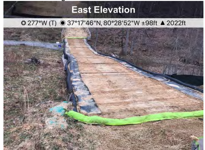
Figure 2: Designated crossing S-MM18, ECD's are in place and functioning.
