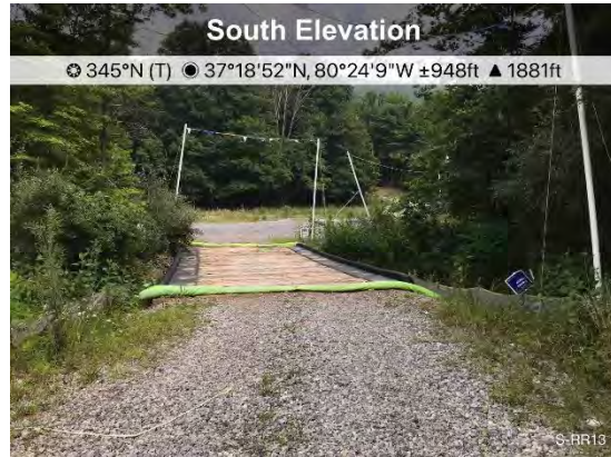
Figure 2: Designated crossing S-RR13, ECD's are in place.
