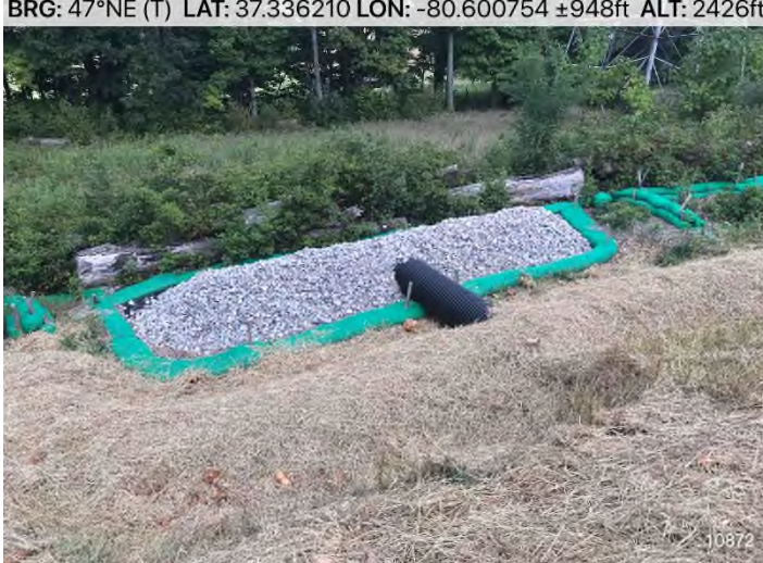
Figure 3: STA 10872+00 – Controls in place and functioning properly. BRG: 47°NE (T) LAT: 37.336210 LON: -80.600754 ±948ft ALT: 2426ft
