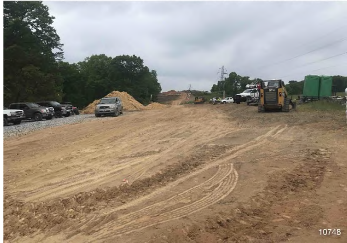
Figure 1: STA 10748+00 – Controls in place and functioning properly. BRG: 321°NW (T) LAT: 37.345255 LON: -80.636571 ±16ft ALT: 2301ft
