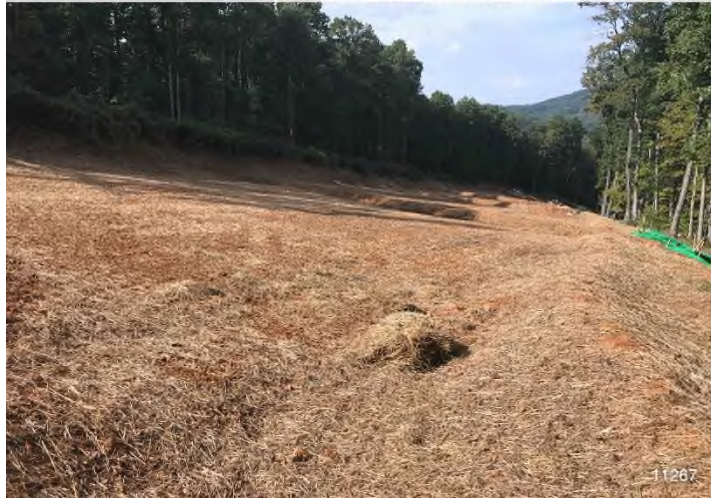
Figure 4: STA 11313+00 – Controls in place and functioning properly. Area stabilized with straw.
