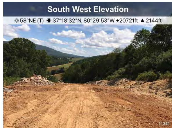
Figure 4: St 11342 ECD's are in place.
