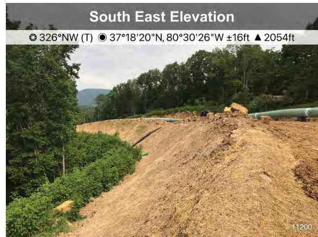
Figure 4: St 11200 stabilized slope
