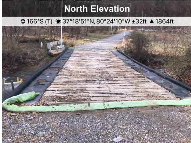
Figure 1: Designated crossing S-RR13, ECD's are in place.
