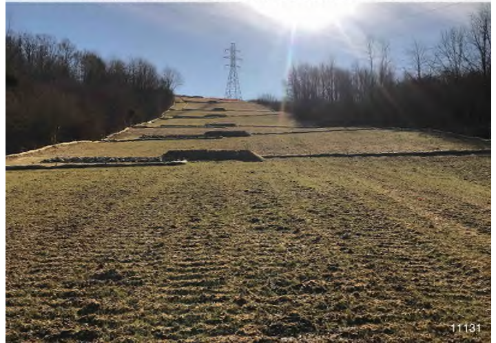
Figure 4: STA 11131+00 – Controls in place and functioning properly. BRG: 133°SE (T) LAT: 37.314253 LON: -80.523731 ±164ft ALT: 2050ft
