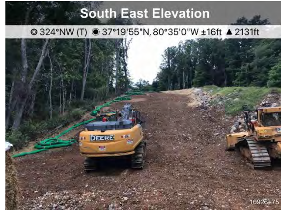
Figure 2: St 10926+75 ECD's are in place.
