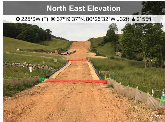
Figure 2: Designated crossing S-PP3, ECD's are in place.
