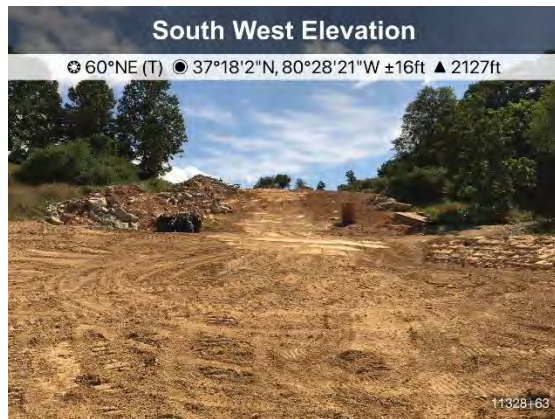
Figure 3: St 11328+63 ECD's are in place.
