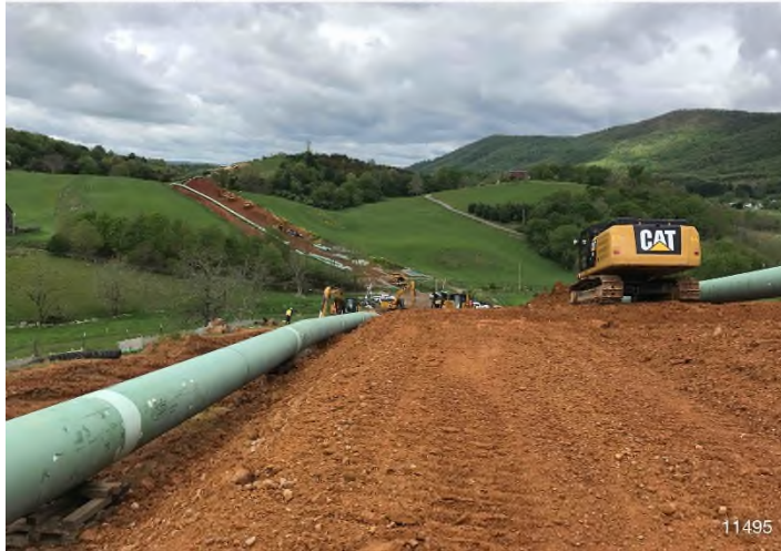
Figure 3: STA 11495+00 – Controls in place and functioning properly. BRG: 230°SW (T) LAT: 37.325289 LON: -80.429496 ±16ft ALT: 2288ft
