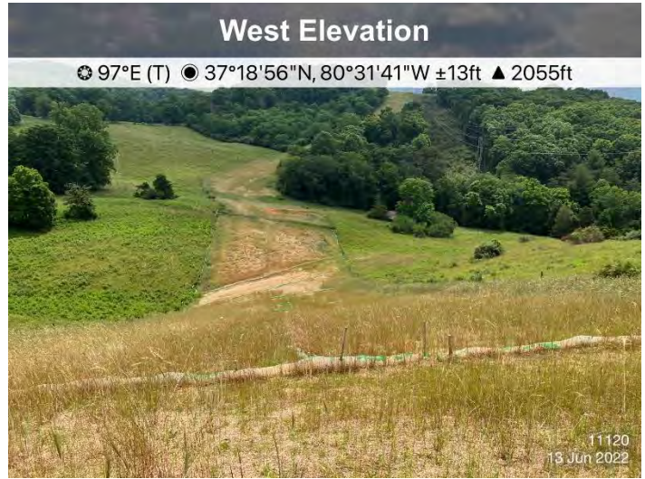
Figure 2: St11120, ECD's and stabilization in place.
