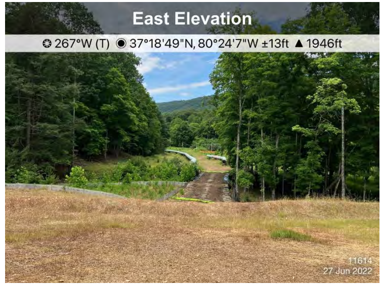
Figure 2: St11614, ECD's and stabilization in place.
