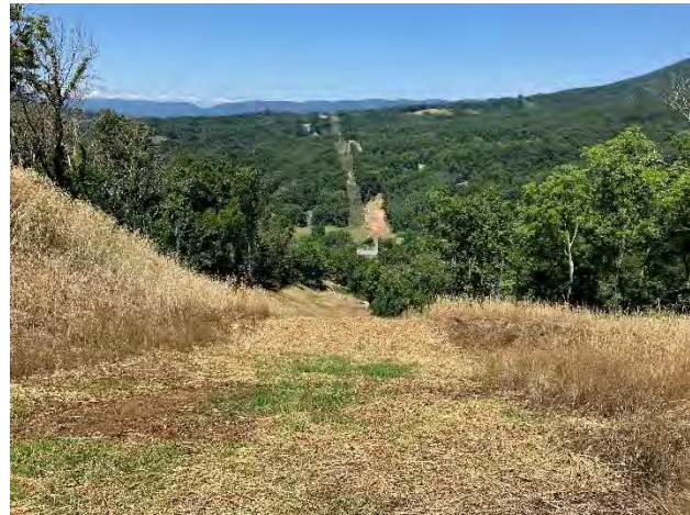
Figure 2: St10819, ECD's and stabilization are in place
