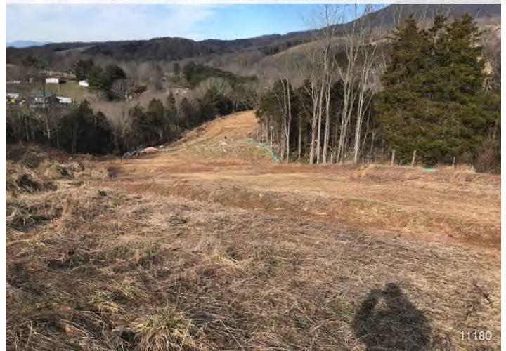
Figure 4: STA 11180+00 – Controls in place and functioning properly. Area stabilized with straw.
