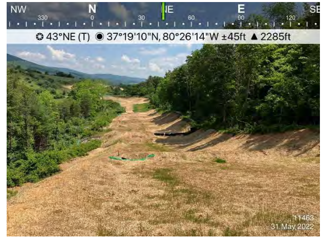
Figure 4: St11463 ECD's and stabilization in place.
