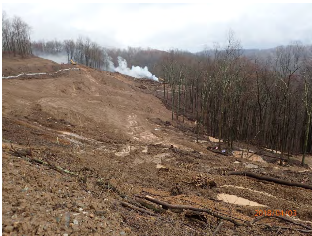
Disturbed area near the reported slip area.
