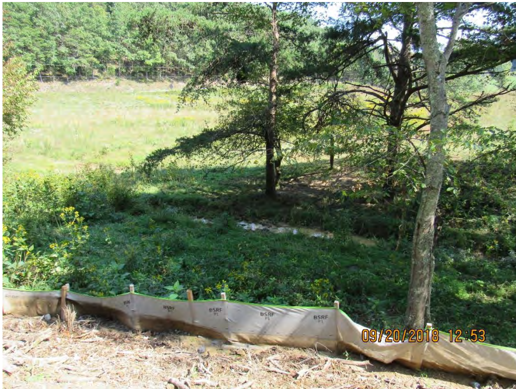
Photo 3: Sediment laden UNT of Painters Run down stream of control failure near station 10270+49
