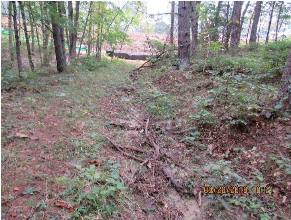
Photo 7: Historic release of controls near station 9617+75 with upgraded controls above Slate Run.
