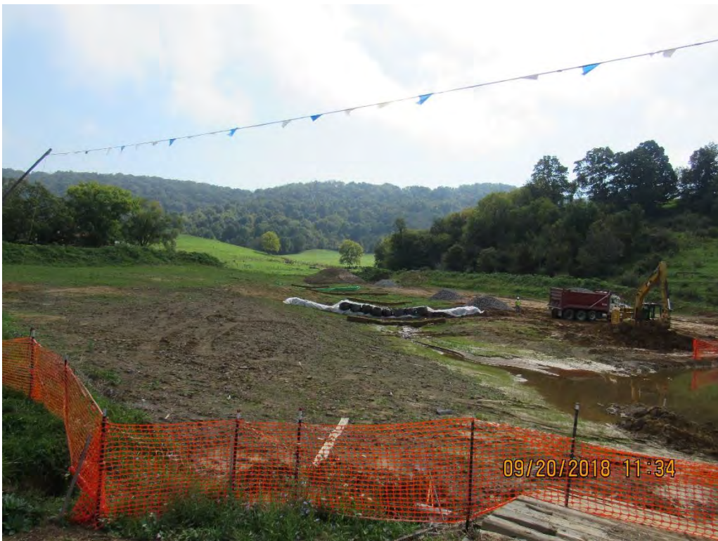
Photo 10: Hurricane Florence storm prep near Lindsie Methodist Church station 10116+46.
