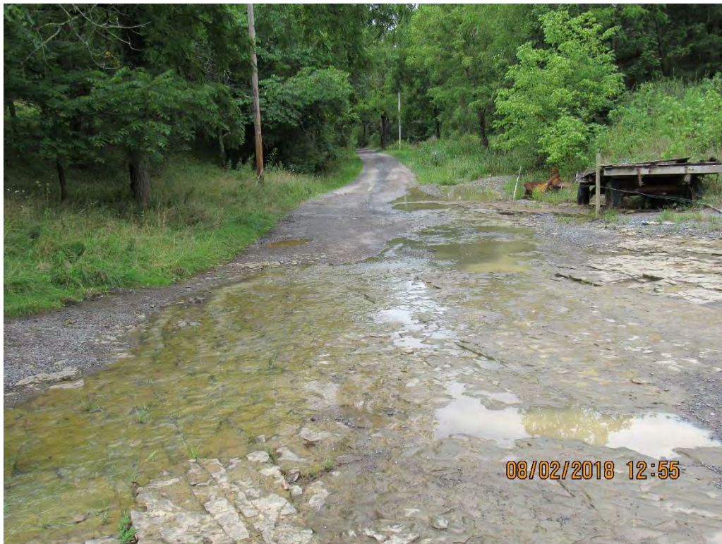
Photo 26: UNT of Hans Creek crossing- exit of stream over Ellison Ridge Road.
