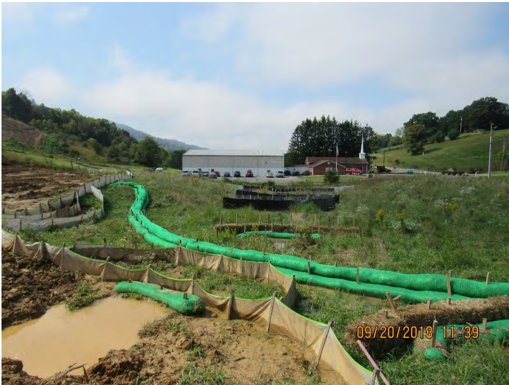
Photo 11: Hurricane Florence storm prep near Lindsie Methodist Church station 10116+46.
