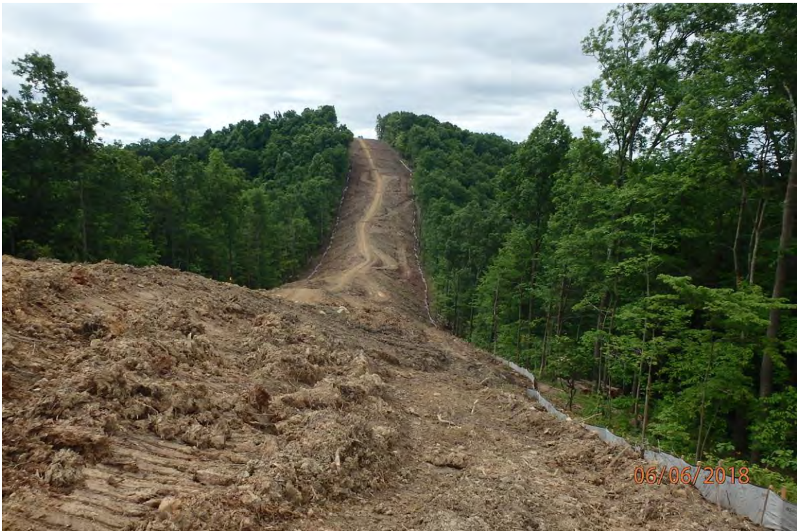
Area adjacent to 498+06 showing controls in place.
