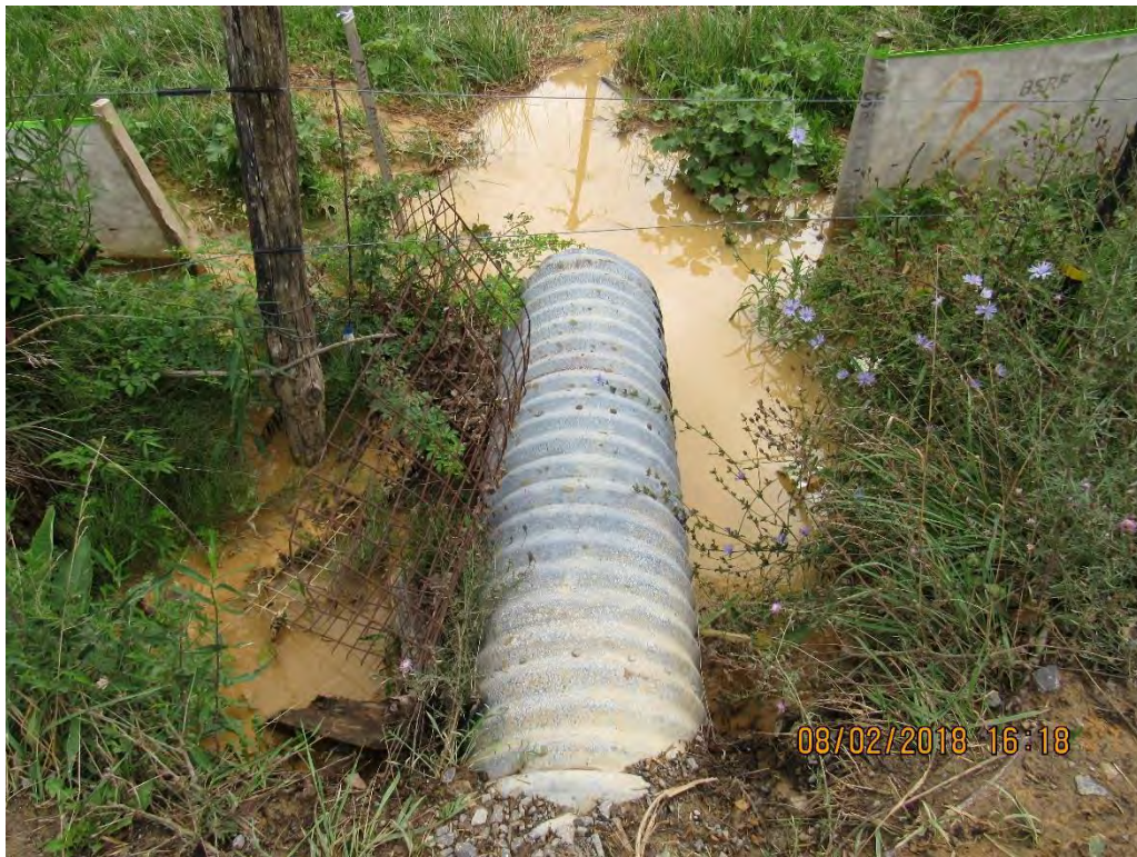
Photo 38: Culvert outlet into wetland area across road from full sump.
