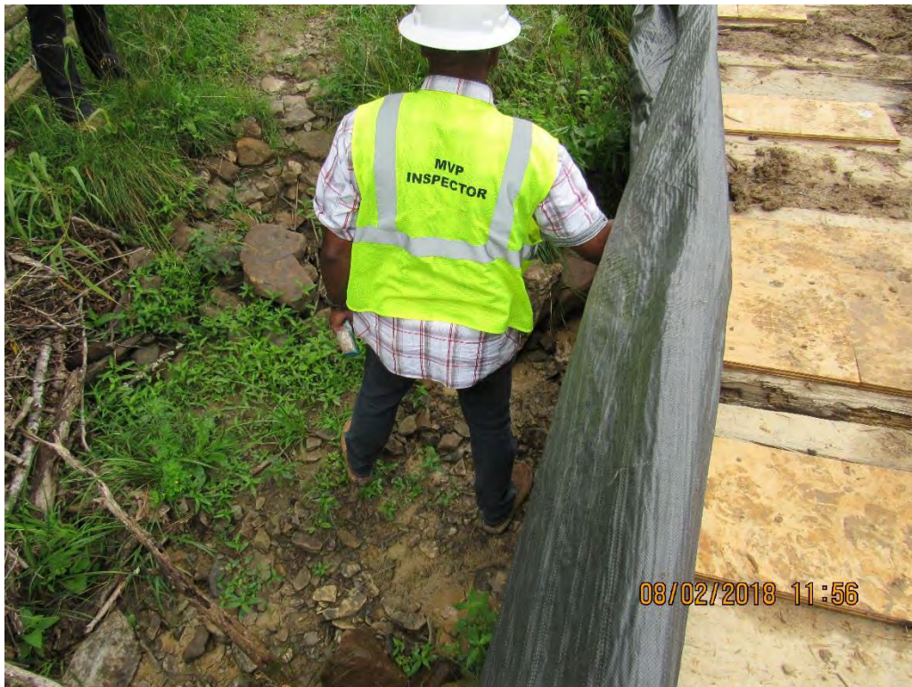
Photo 18: Sediment deposits observed below base of bridge between feet and in front of inspector.
