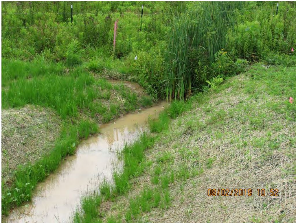
Photo 15: Stoney Creek below sediment plume entering stream in photo 14.
