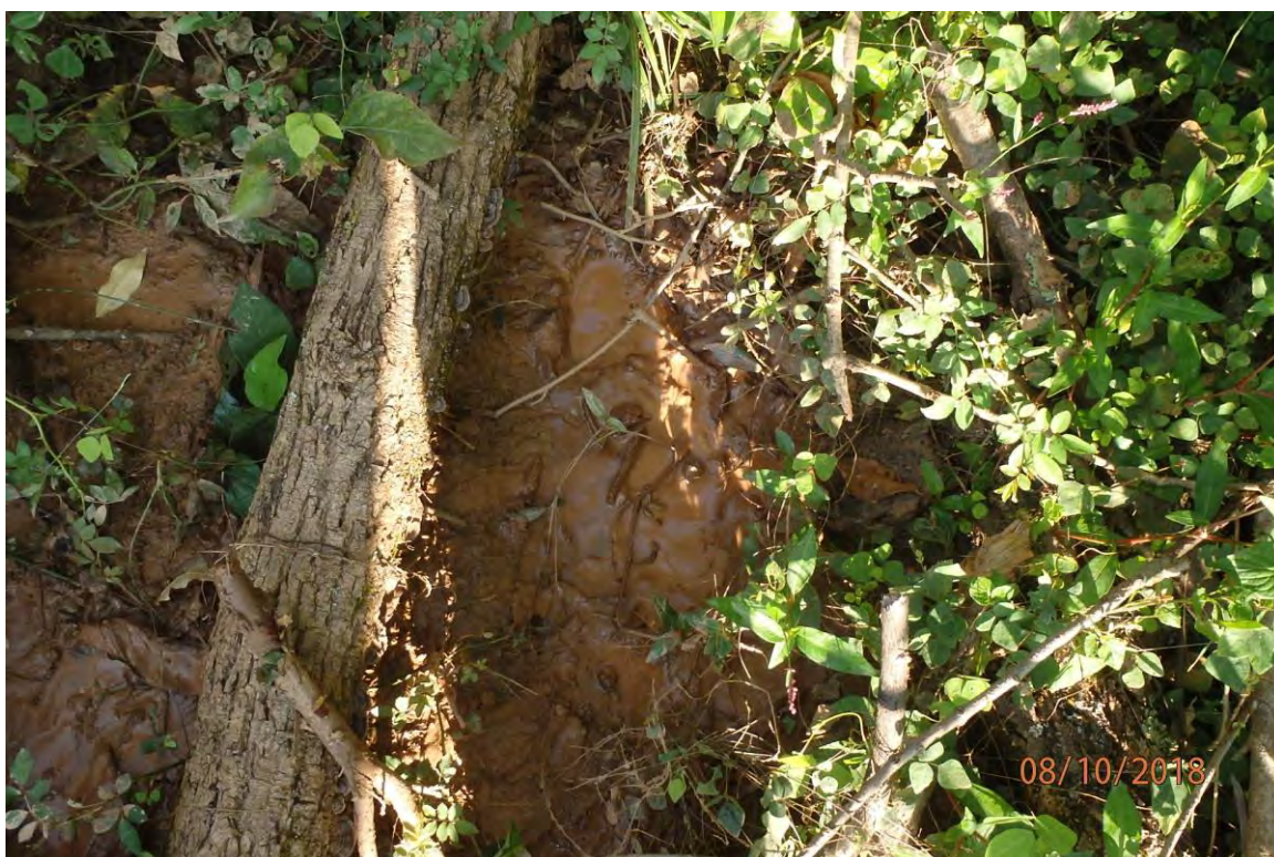
A water bar installed at a steep angle in the Meathouse Fork watershed and the resulting offsite sediment deposits. Deficiencies in site evaluation item numbers 6, 7, 14, 19 & 21 pictured.
