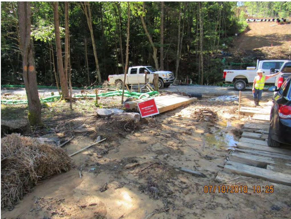
Photo 4: Sediment down gradient of straw bale pile (on right in above photo).
