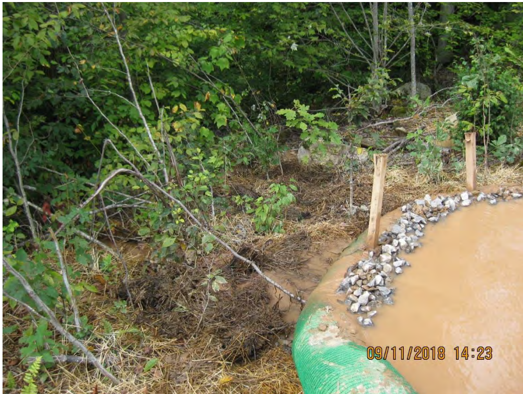
Photo 9: Station 900 (approximately)- outlet of sump below photo 8 with sediment laden water leaving site view down gradient.
