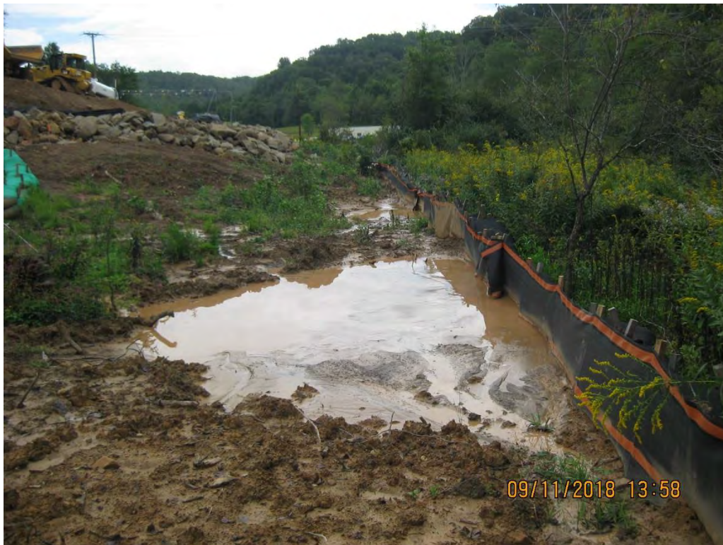
Photo 4: Station 150 (approximately)- controls maintained abating NOV issued 8/13/2018.
