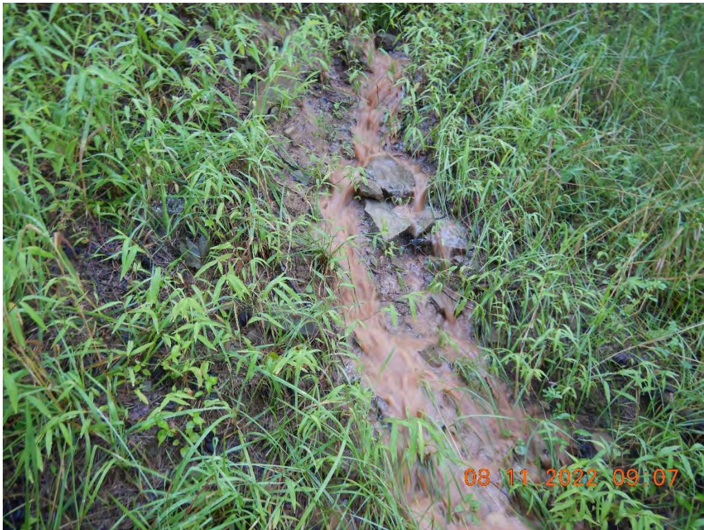
Photo # DSCN2166 – Sediment laden water flowing downslope below and outside of the Mountain Valley Pipeline project.
