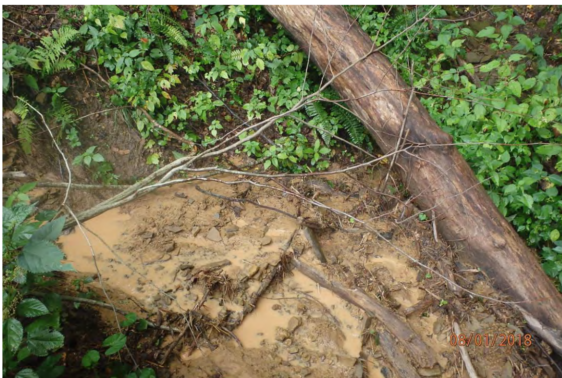
CNA offsite sediment deposits and visible plume in UNT Goose Run (39° 26.100' X 80° 28.4922') originating from site. Deficiencies in site evaluation item numbers 19, 20 & 21 pictured.
