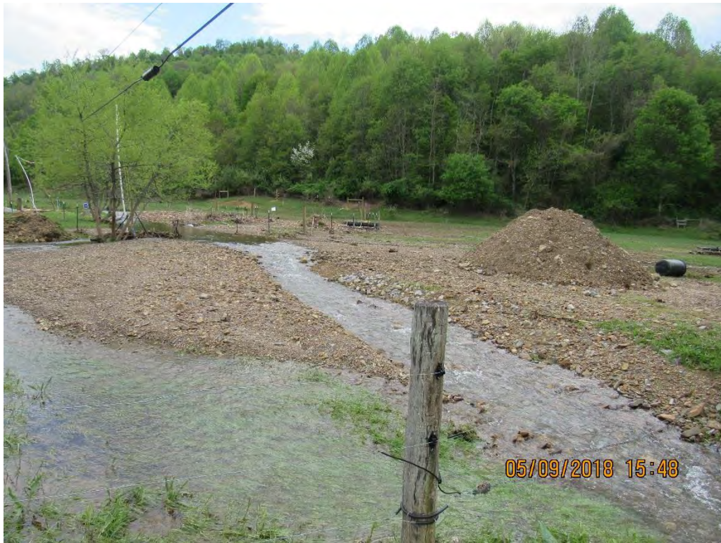
Photo 3: Mr. Laws field (station 10146+32, sheet 9.35)- stream has been partially returned to channel. Rock/soil pile from landowner removing debris to restore to channel.
