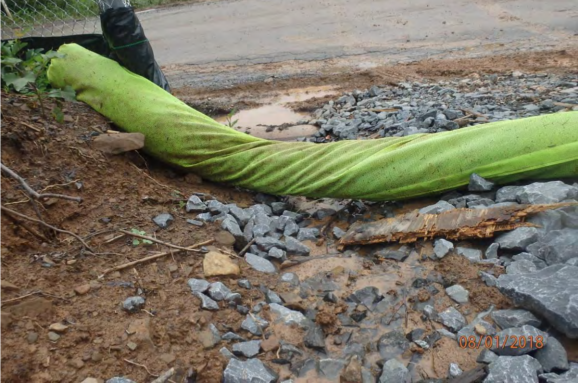
Improperly operated BMP in Right Fork of Big Elk watershed. Deficiencies in site evaluation item numbers 1, 6, 19 & 21 pictured.
