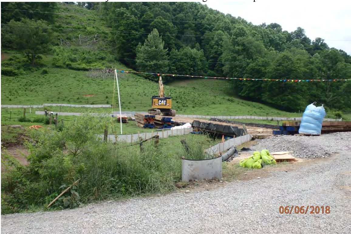
Area adjacent to AR 19 showing BMP installation.
