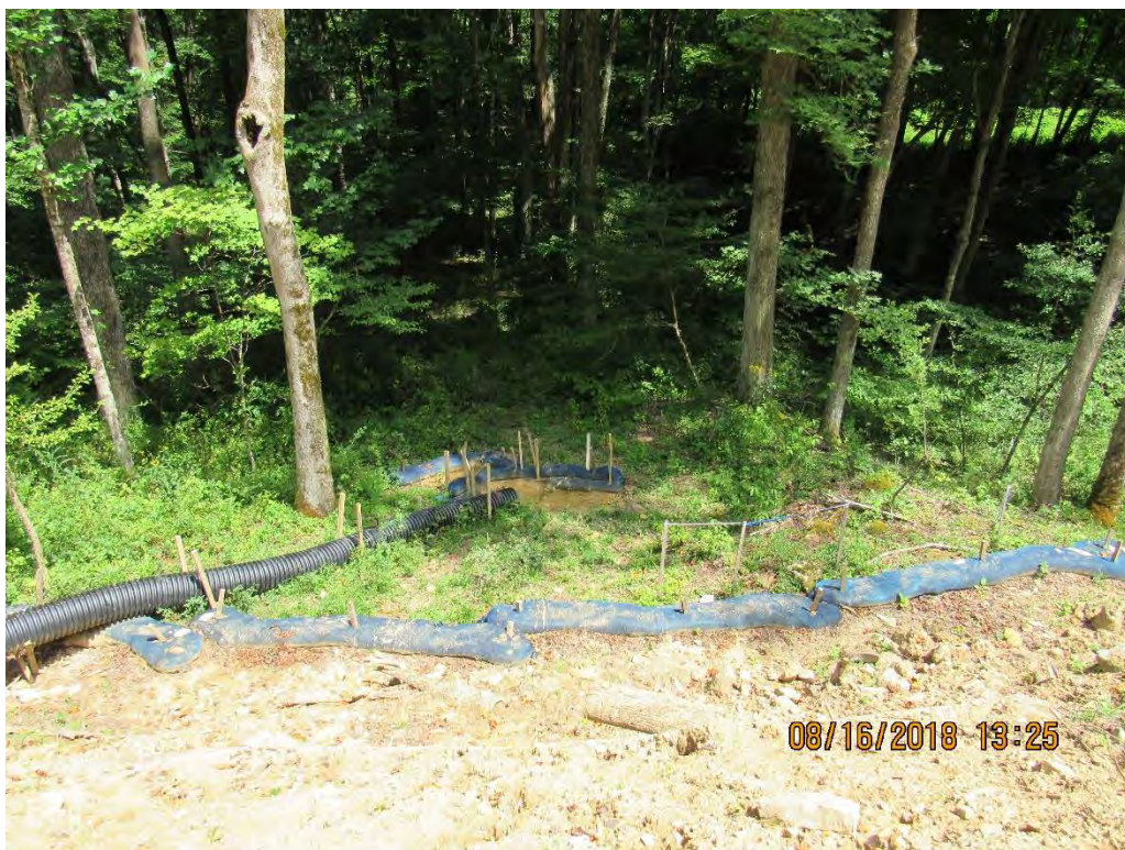
Photo 34: Recommended to lengthen 'J' hooks at end of pipe slope drains at station 6978+70.
