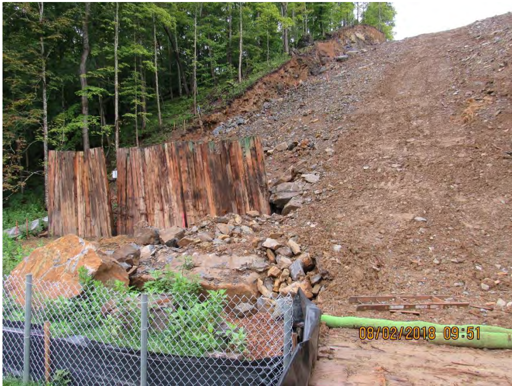
Photo 7: Vertical mats installed to divert rocks from stream.
