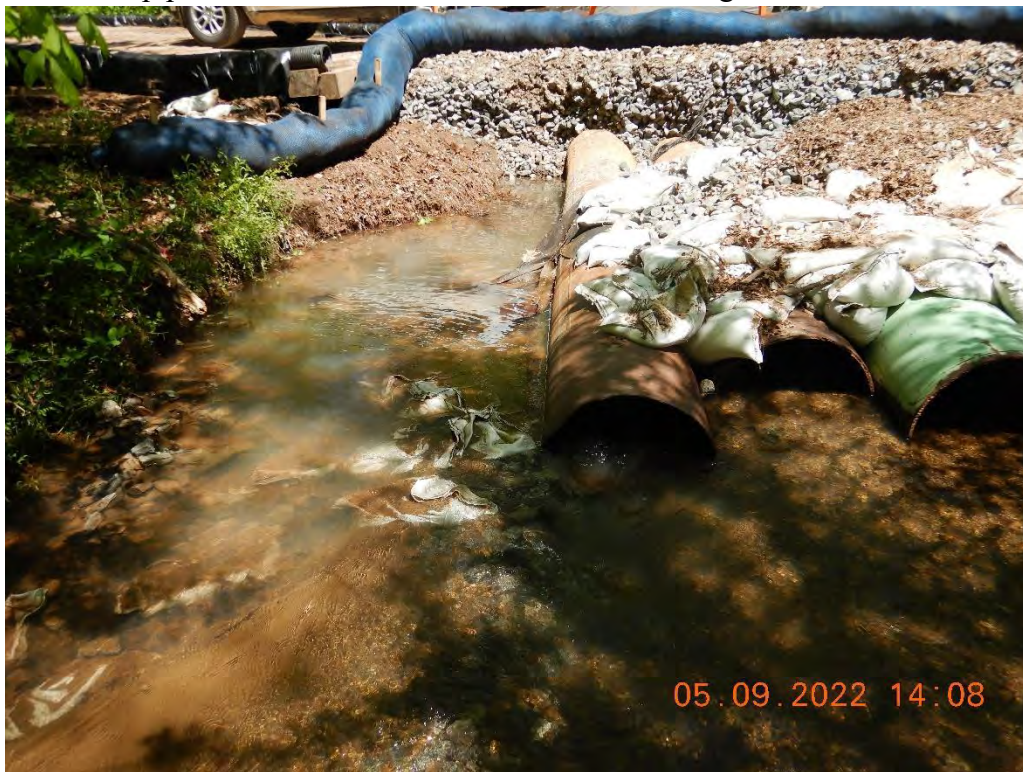
This is a photo showing the flumes that were in place on 5/9/2022.
