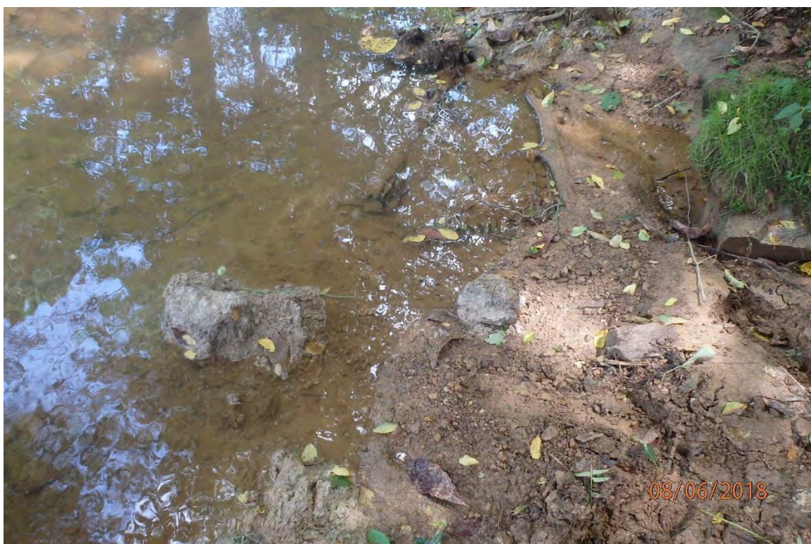
Offsite CNA deposits in Grass Run (39° 20.1127' X 80° 31.3233') that originate from site. Deficiencies in site evaluation item numbers 19, 20 & 21 pictured.
