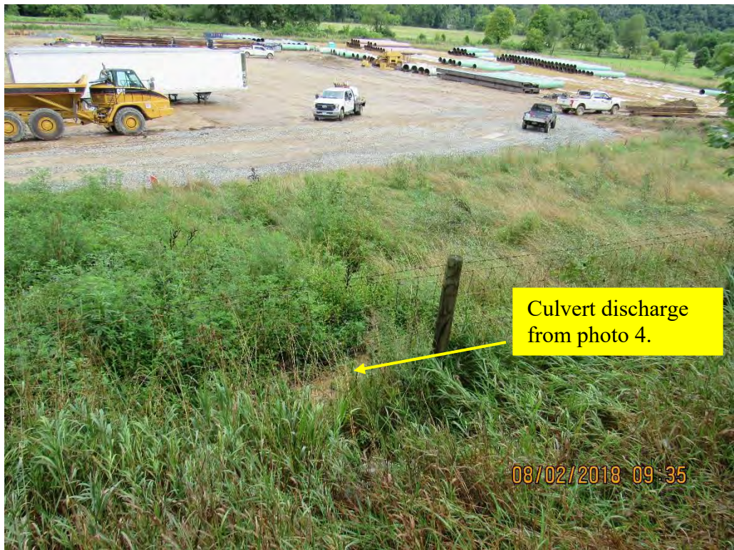
Photo 5: Road side ditch discharging into field upslope of laydown yard, receiving additional treatment prior to release
