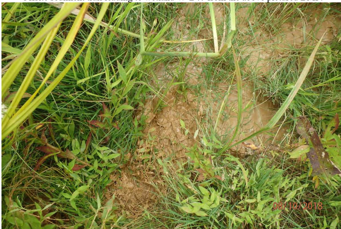
CNA deposits in wetland UNT Left Fork of Freemans Creek (W-B47) (39° 04.744' X 80° 34.904) that originate from site. Deficiencies in site evaluation item numbers 6, 7, 19, 20 & 21 pictured.
