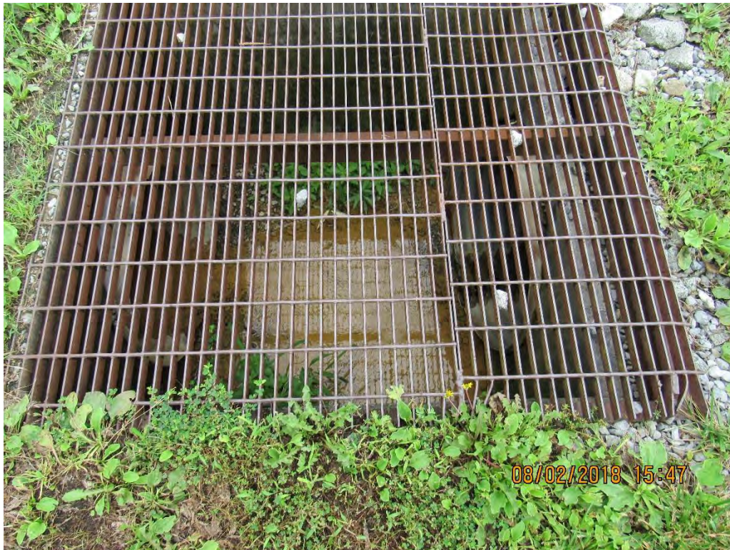
Photo 35: Clear water in drop inlet upstream of culvert (photo 34).
