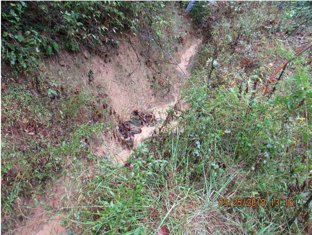
Photo 1: Sediment laden water from sumps near station 3625+00.
