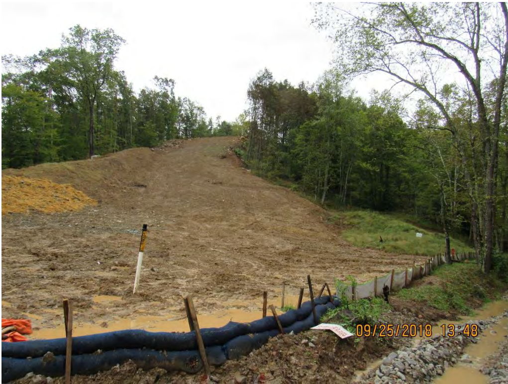
Photo 7: Former area of concern near Barbecue Run at station 3565+00.
