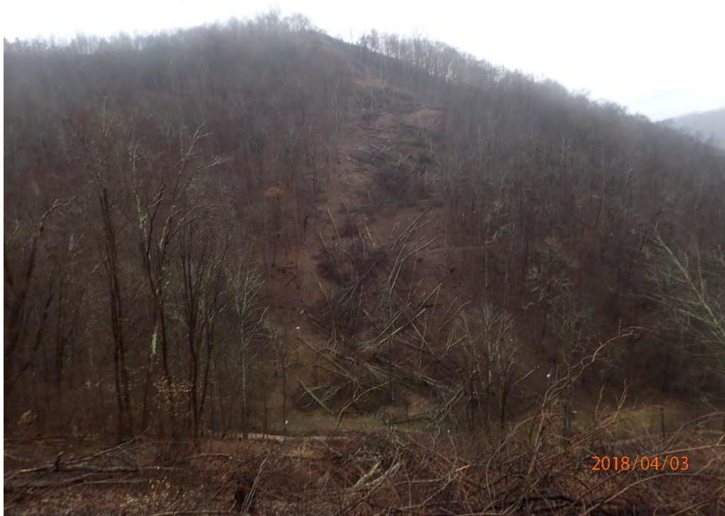
Line clearing off North Fork Road.
