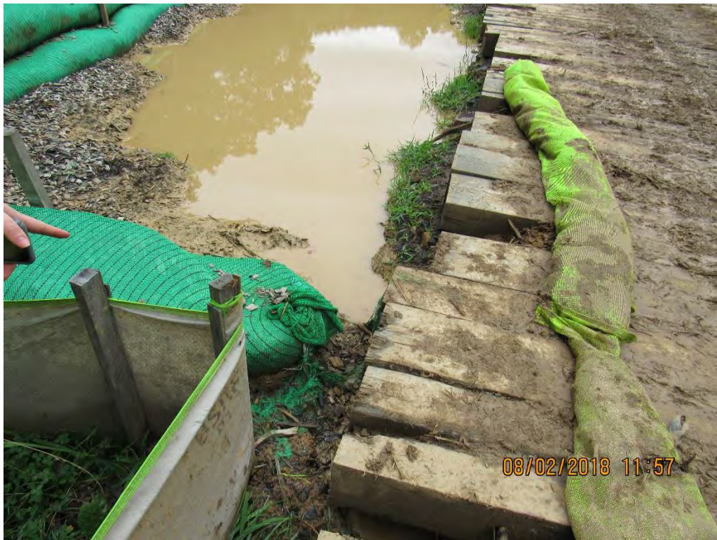
Photo 20: Source of sediment laden water in Slate Run-
