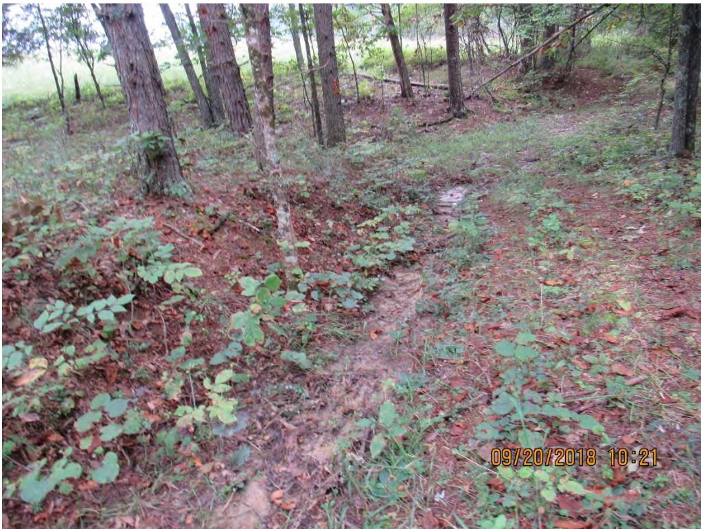
Photo 8: Downslope of historic release of controls near station 9617+75 above Slate Run.
