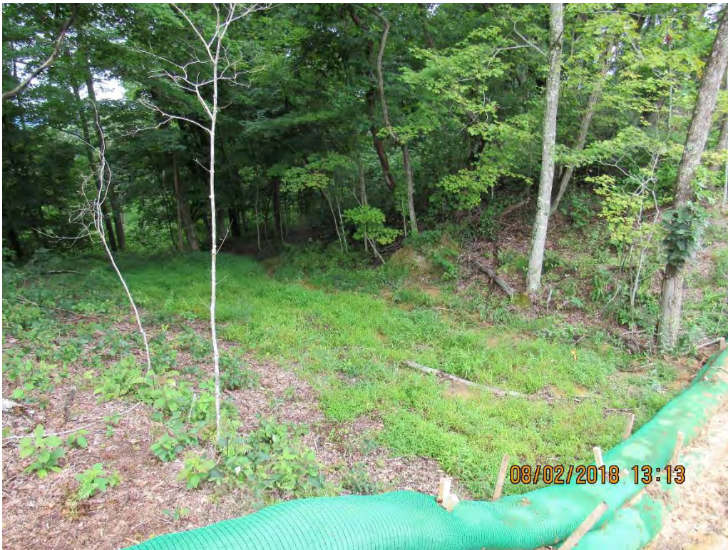
Photo 33: Down gradient of previous control failure in Photo 32.
