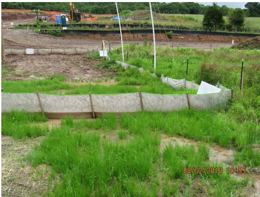
Photo 11: Installed silt fence is releasing filtered water.
