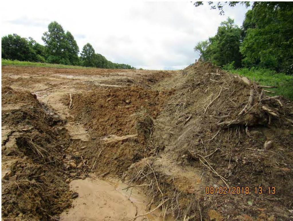
Photo 30: Additional sump installed above control failure near station 9961+00 (off access road 227)
