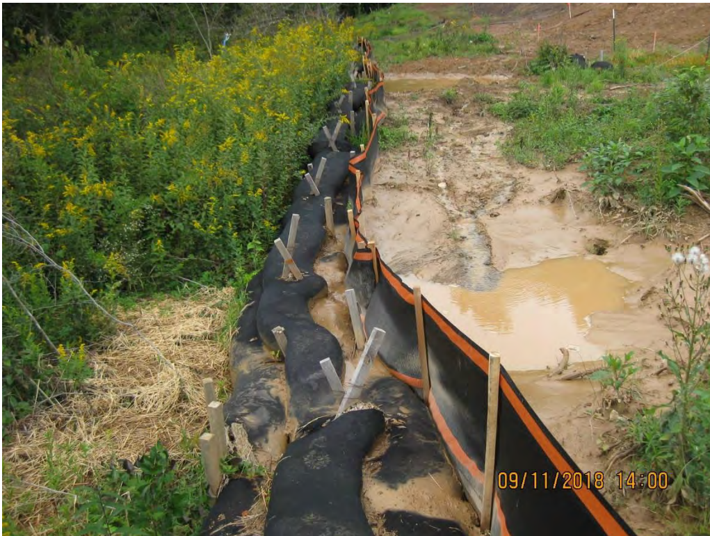
Photo 5: Station 150 (approximately)- controls maintained abating NOV issued 8/13/2018.
