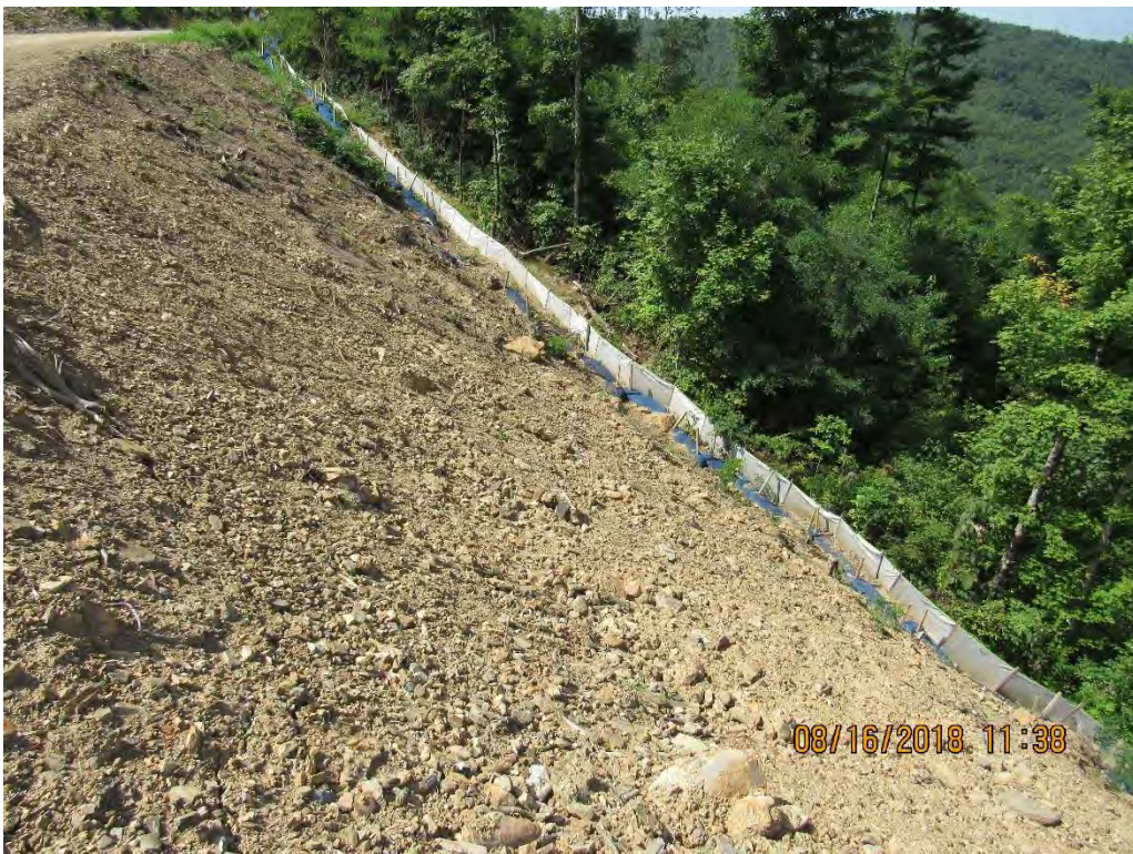
Photo 16: Southern view of Bamboo Road near Station 7158+00 without fill slope protection and temporary stabilization.
