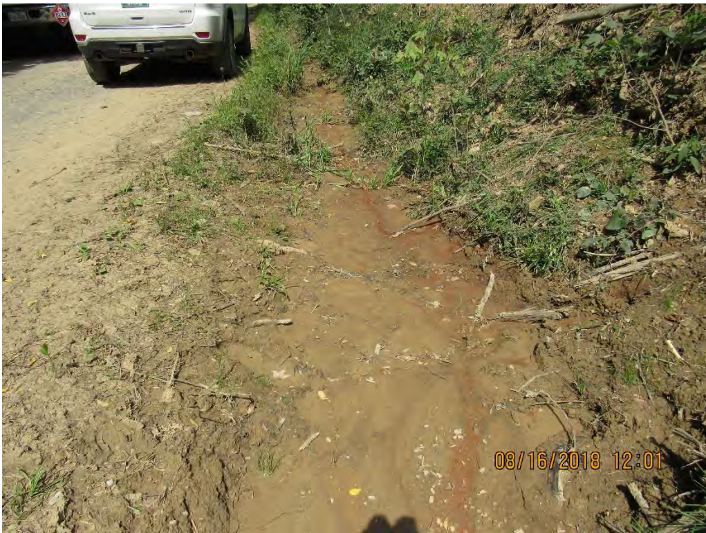
Photo 26: Road side ditch below water bar terminus in photos 23-25 conveying sediment laden water to installed culvert.
