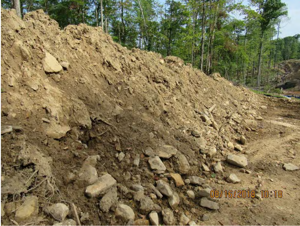
Photo 19: Northern view of waste pile with inadequate stabilization. (Photo taken near Bingham Road station 7450+00)
