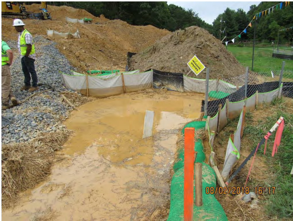
Photo 36: Station 10270+00, sump is full.
