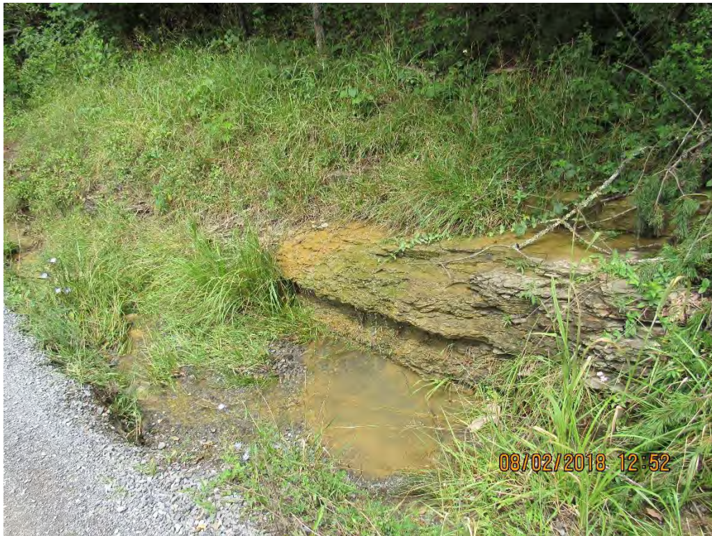
Photo 23: Entrance to UNT of Hans Creek several days after control failure on ROW-view downstream.
