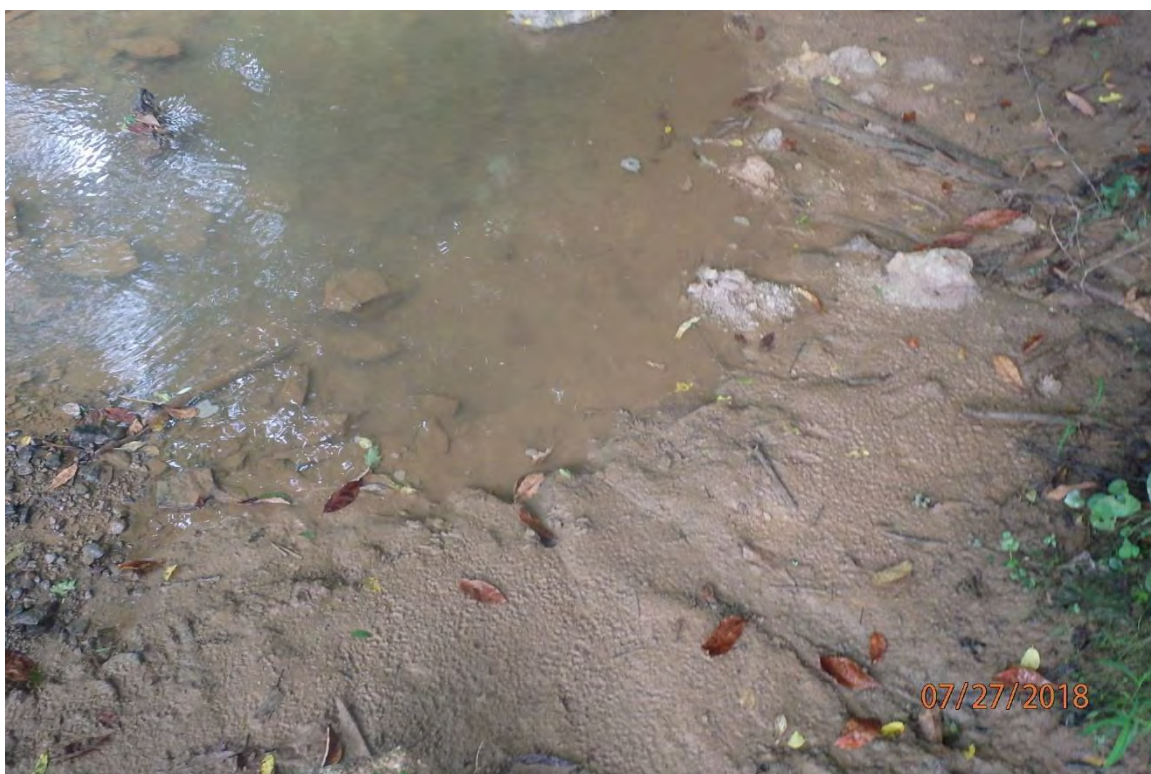
Offsite sediment deposits in Grass Run (S-A11a) that originate from site. Deficiencies in site evaluation item numbers 15, 19, 20 & 21 pictured.
