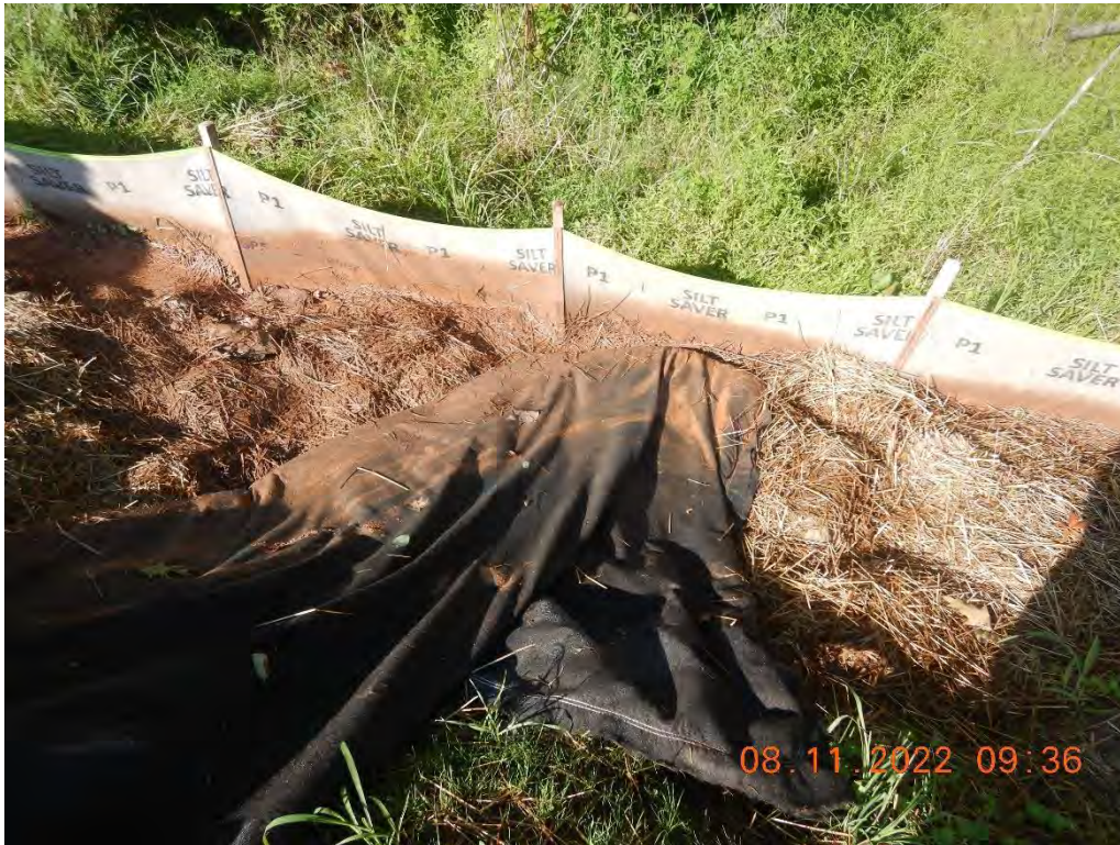
Photo # DSCN2184 – View of the filter bag after the pump had been shut down.
