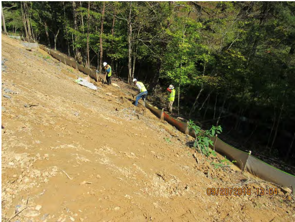
Photo 5: Repairs in progress along access road 231.01 near station 10270+49 Painters Run.
