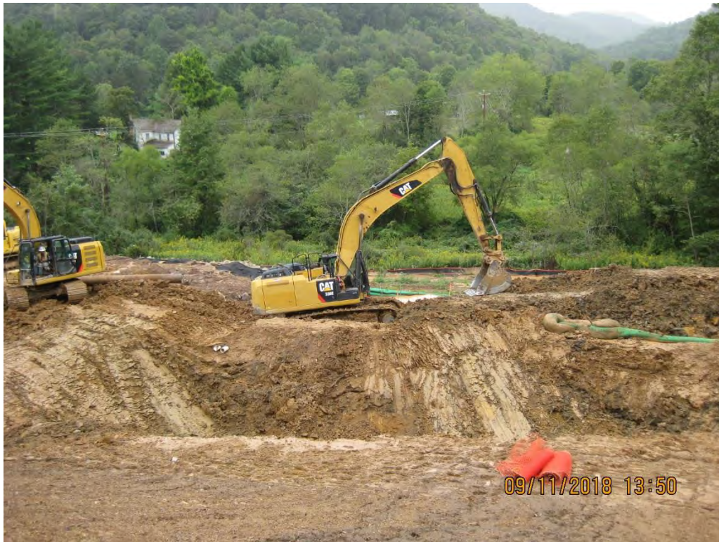
Photo 3: Station 150- Construction of temporary basin in preparation for Hurricane Florence.
