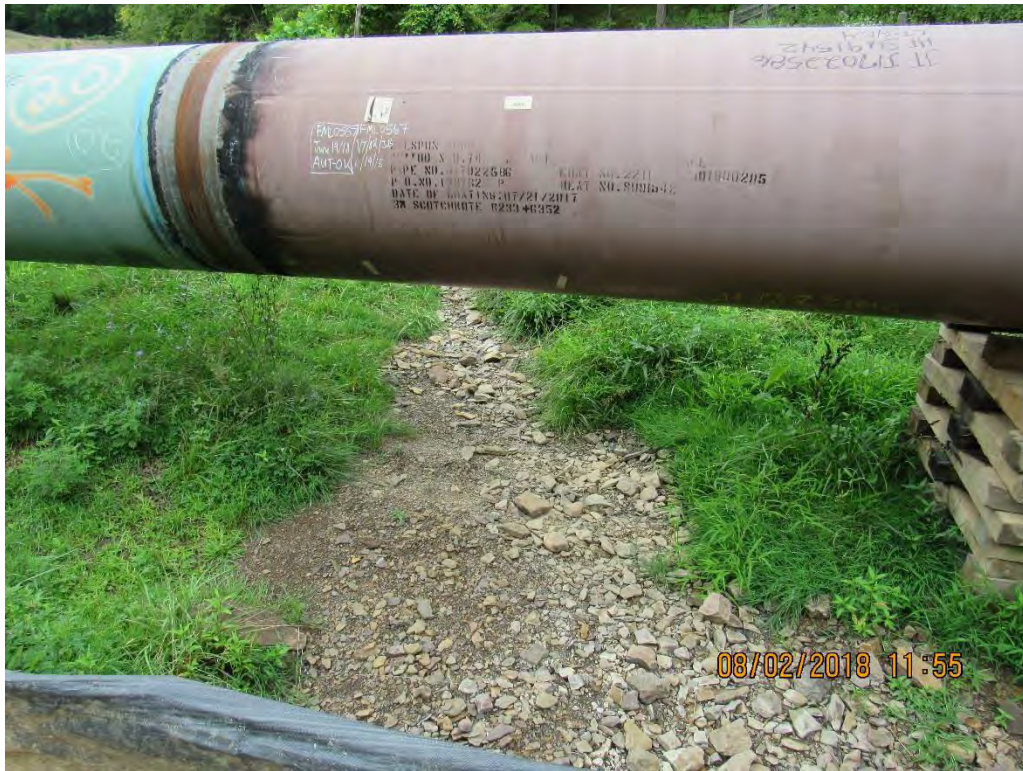
Photo 17: Upstream of last bridge over Slate Run.
