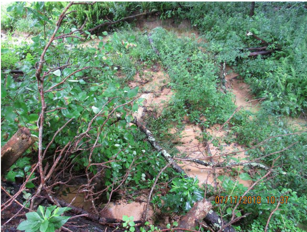
Photo 8: Sediment deposits below temporary tree dam.
