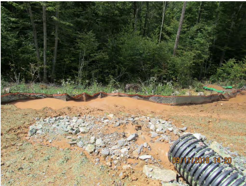
Photo 6: Station 900- Culvert outlet concentrating flow from diversion ditch.
