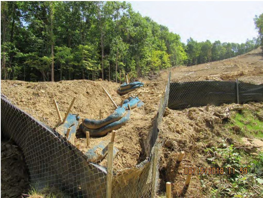
Photo 23: Water bar terminus at station 7084+00 with ROW slope of Photo 21 in background.
