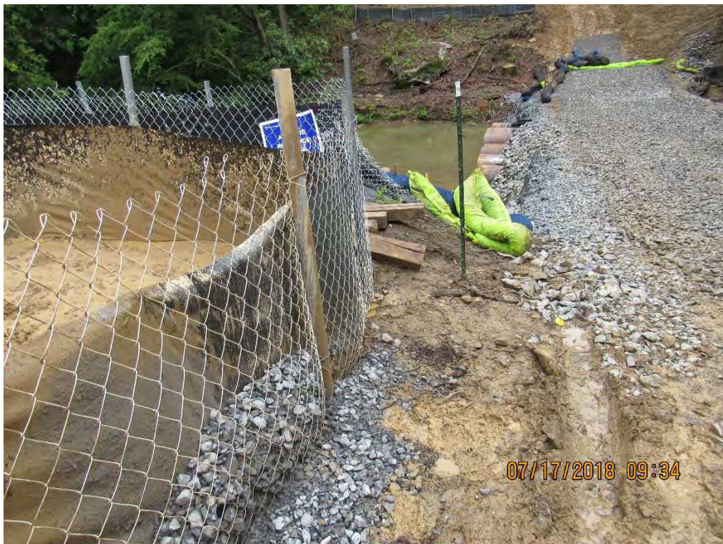
Photo 2: Proximity of outlet of sump and amount of accumulated sediment creates an area of concern.
