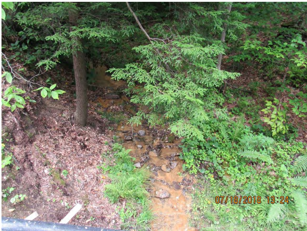
Photo 8: Sediment deposits in UNT of Harmony Creek below 1 st water bar failure
