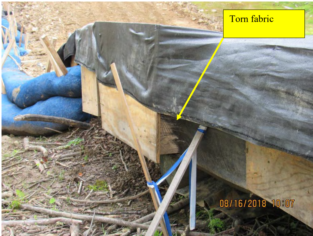
Photo 10: Exterior view of punctured fabric in Photo 9.
