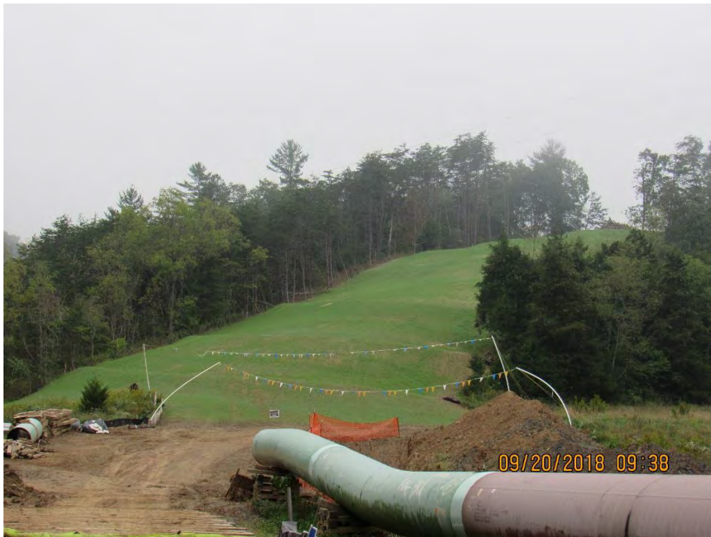
Photo 6: Slope above Slate Run near station 9624 has been reclaimed with some growth.
