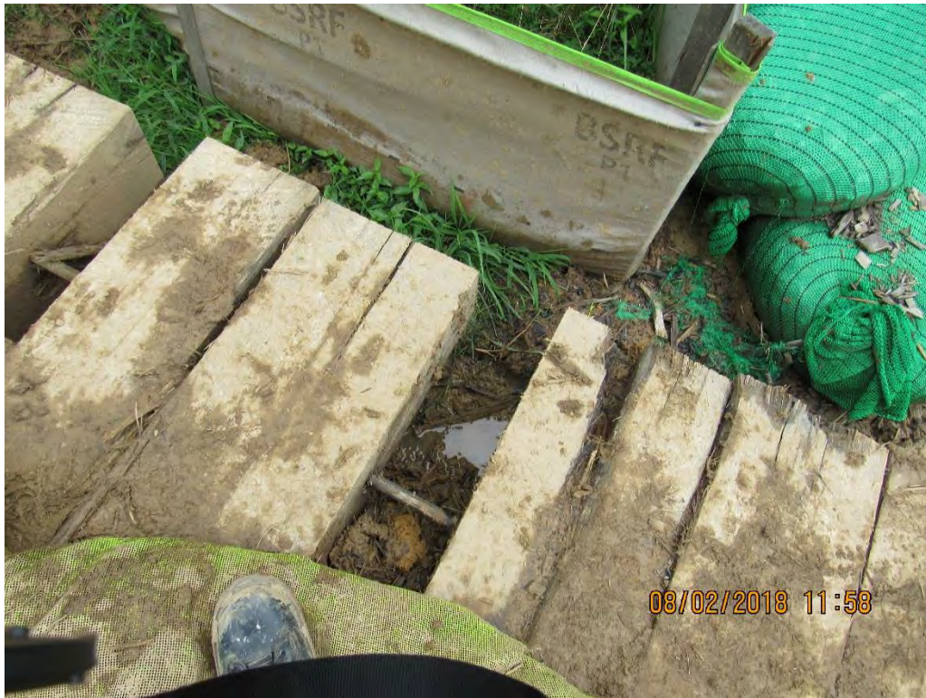
Photo 19: Sediment laden water traced under bridge matting.
