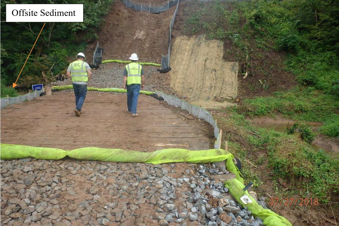
Overview of Grass Run crossing.
