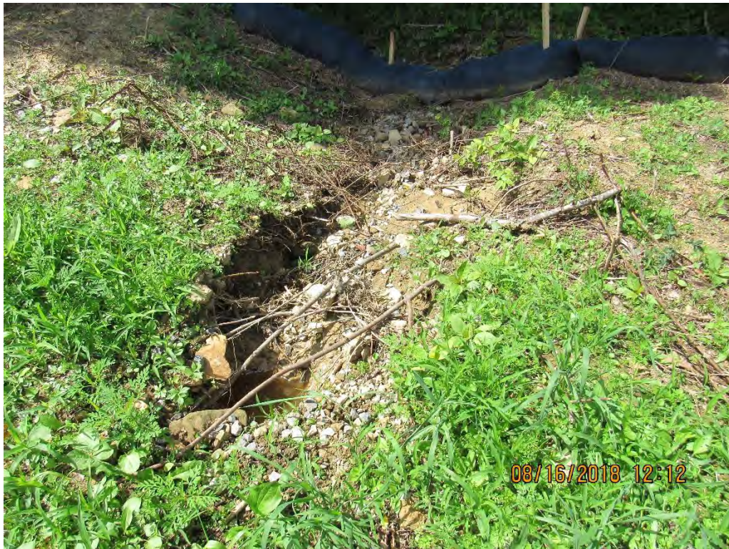
Photo 29: Outlet to SR culvert connected to installed culvert in photo 27.
