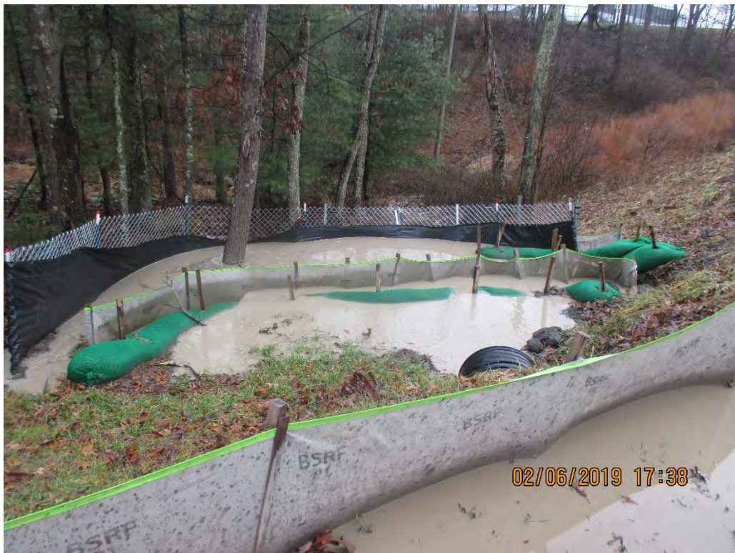
Culvert outflow into multiple controls with SLW present.
