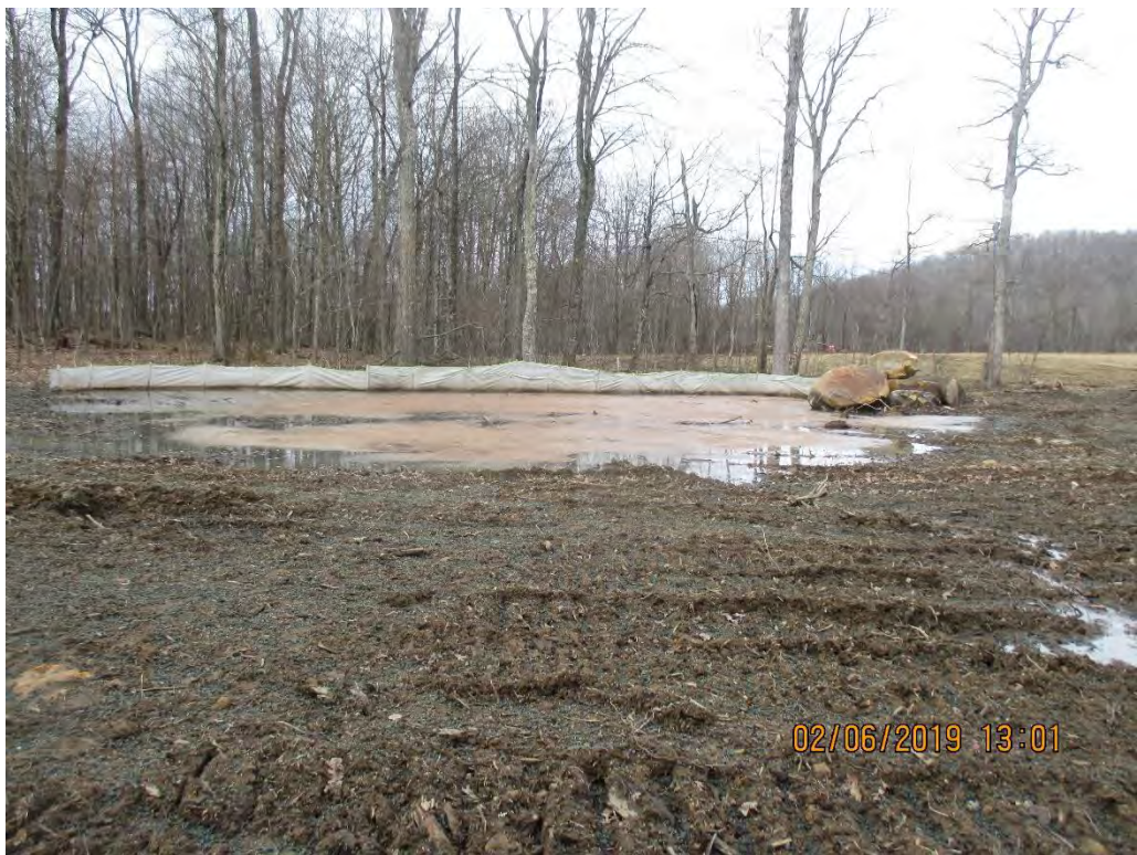
Low lying saturated area in ROW at station #8784+00.
