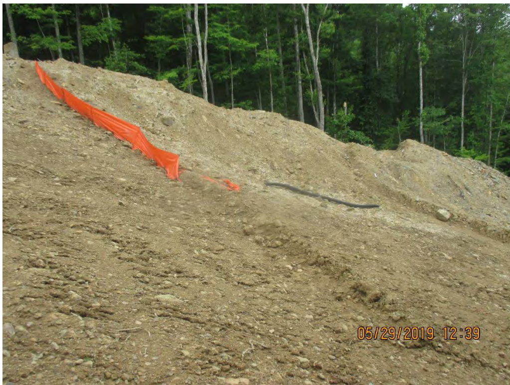
Trench drain outlet terminating onto ROW above Waterbar near station No. 3973+00.
