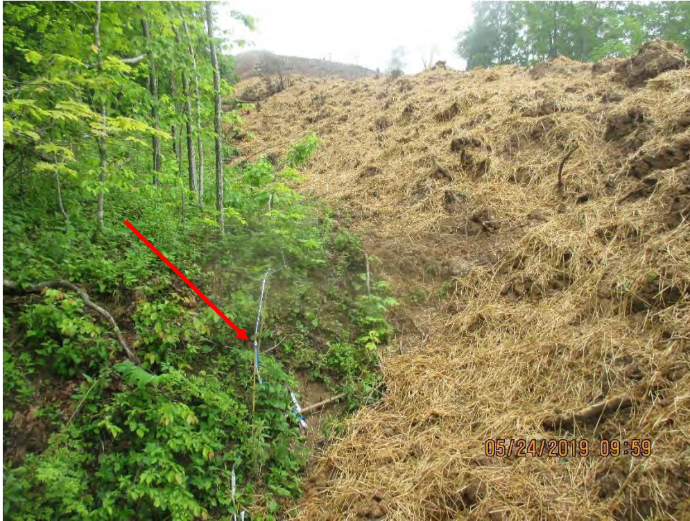
Topsoil pile near station No. 8387+96 facing South at MVP ROW LOD. Arrow depicts LOD.
