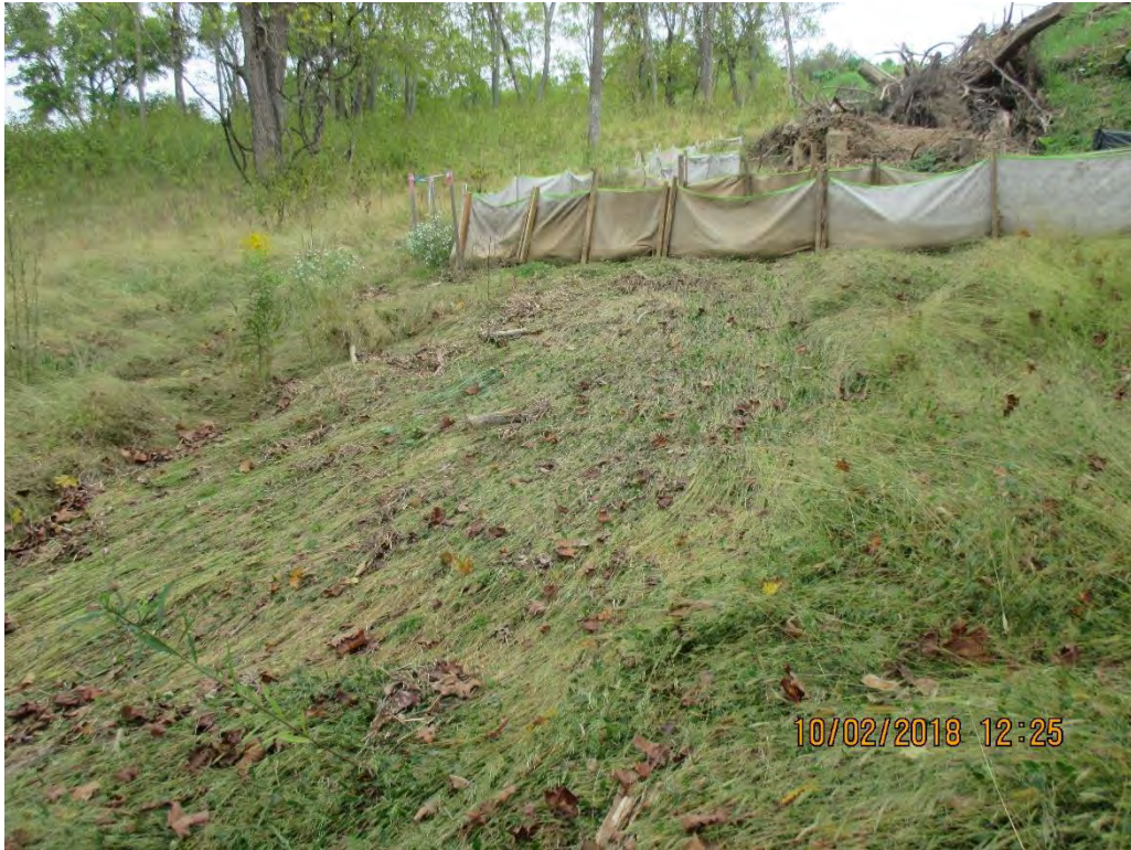
BMP above pond receiving concentrated flow.
