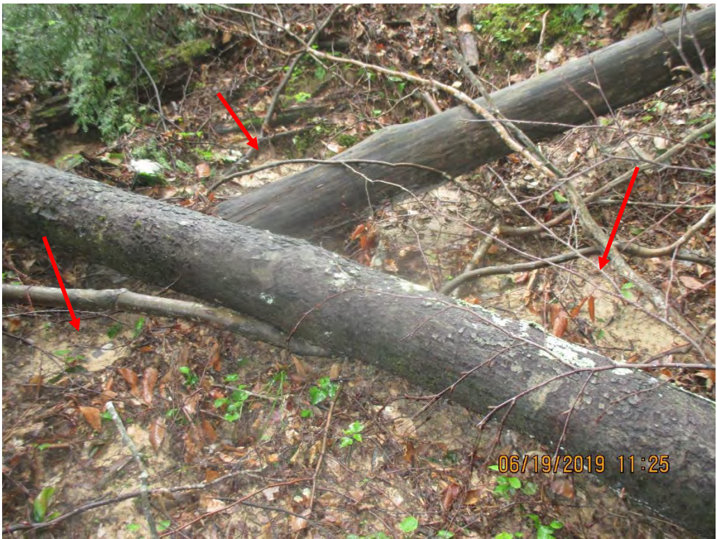
Sediment deposits below scouring on stream bank of S-L38 and below controls approximately 75 feet downslope of Station No. 6587+00. Arrow depicts sediment deposits.
