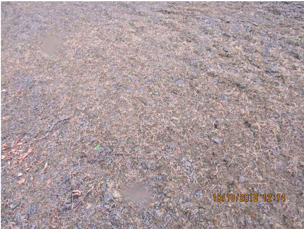
Photo 13: Slate Run station 9624 close-up of root system and remains of vegetation.
