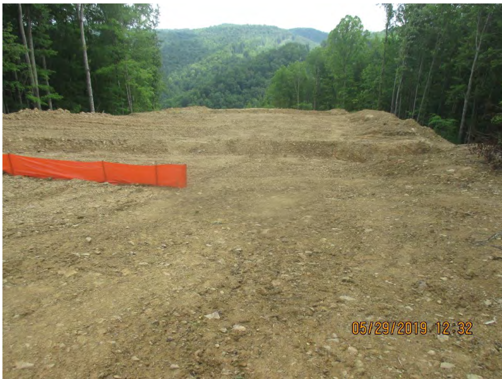
Silt fence installed above Waterbar at station No. 3977+00.
