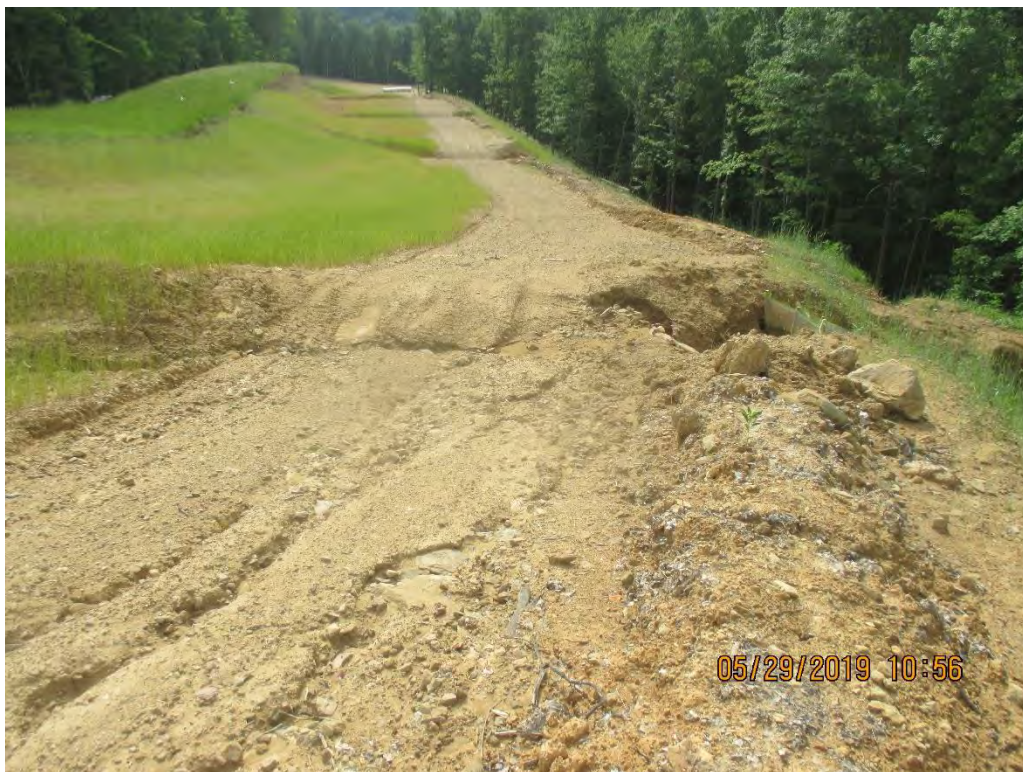
Standing above Waterbar outlet terminating onto fill slope at station No. 4031+00.
