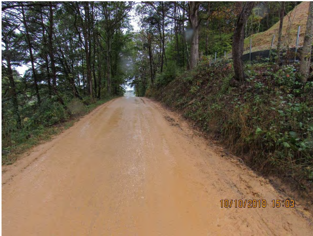
Photo 5: Painter's Run Road station 10270 upgradient of access road crossing.
