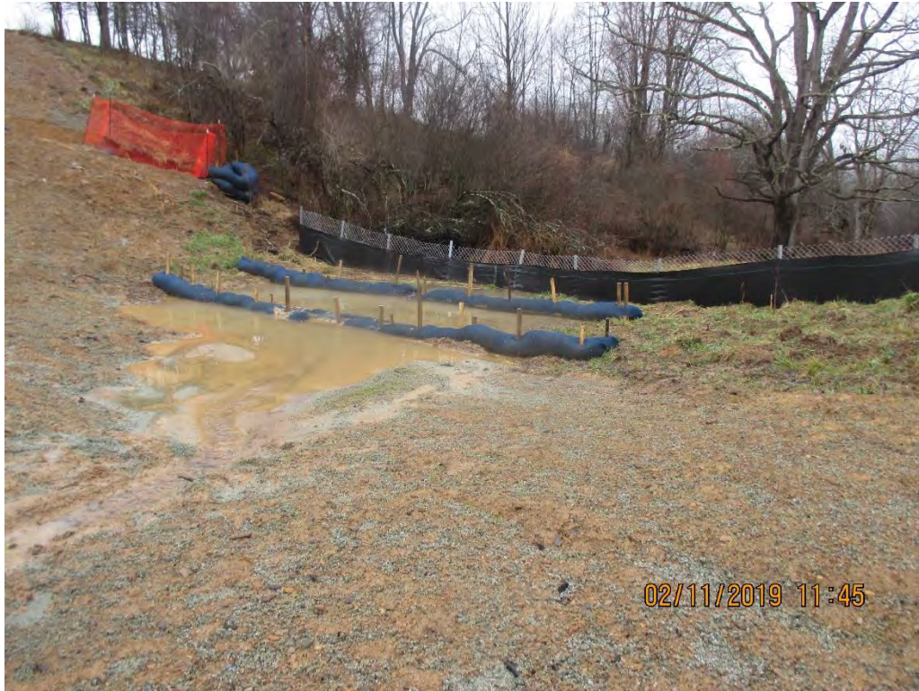
Facing upslope at waterbar terminus near station 5999+50.
