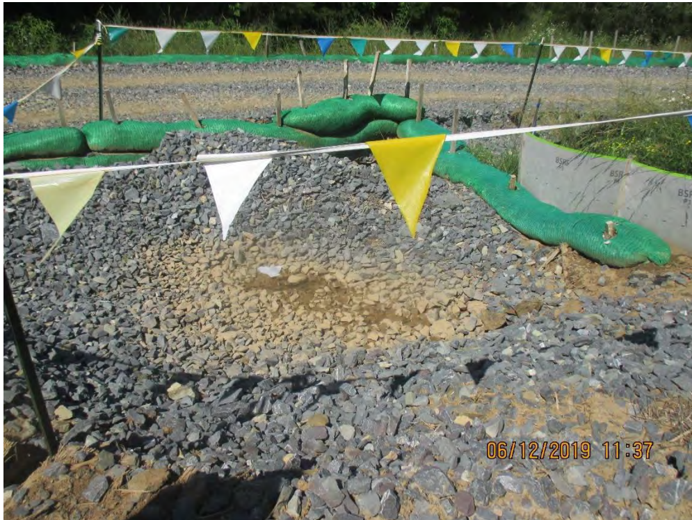
Culvert outlet terminating in sump along AR 227.
