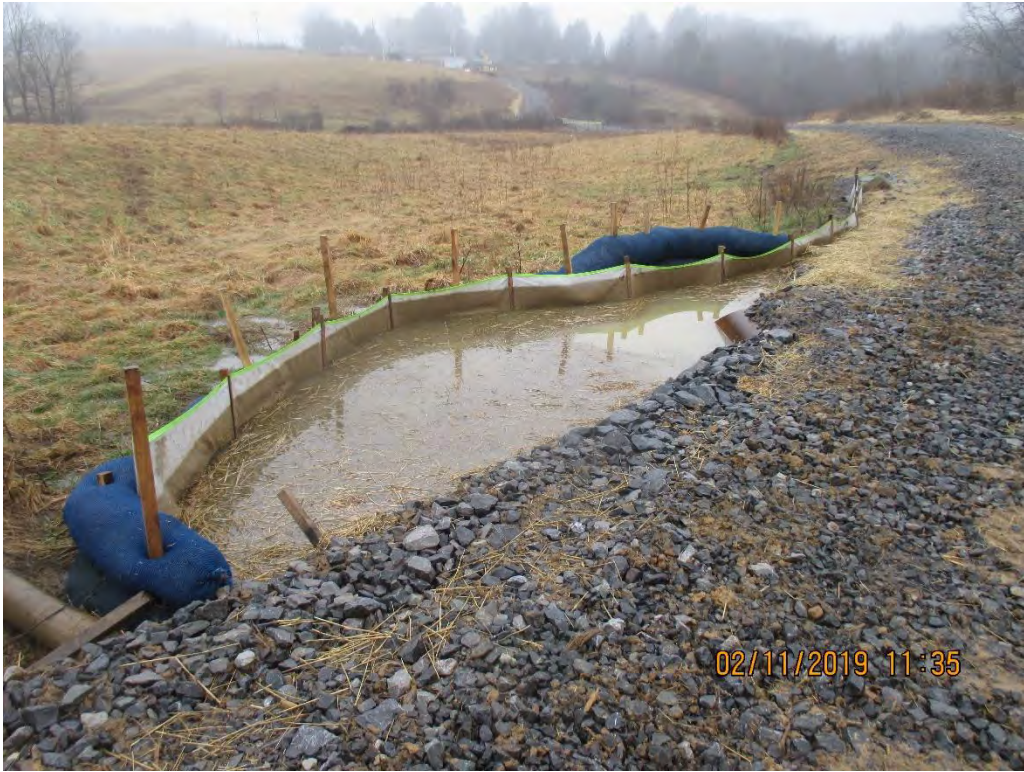
Culvert terminus on Access Road MVP-IN-141.01.
