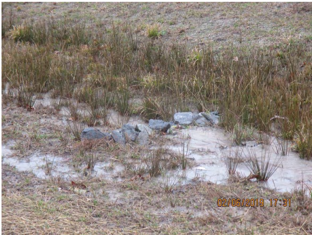
Rock check in ditch with SLW present draining towards culvert.
