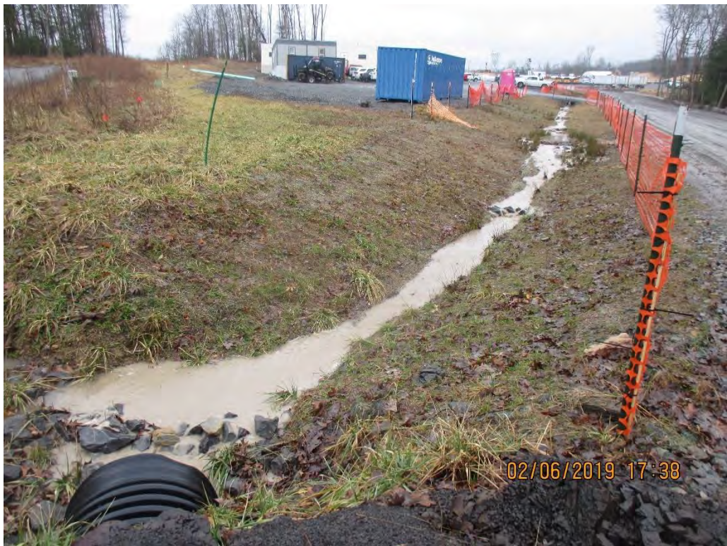
View of ditch facing west (upslope) towards culvert and wetland.
