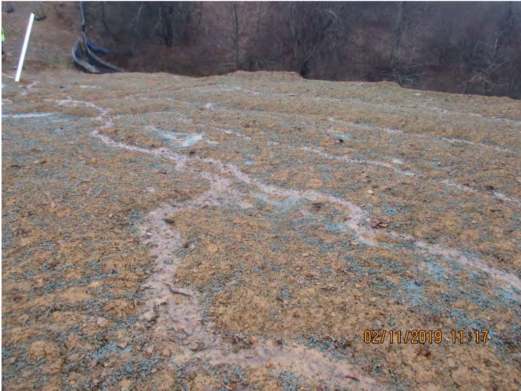
North side of slope leading to outlet near station 6017+50
