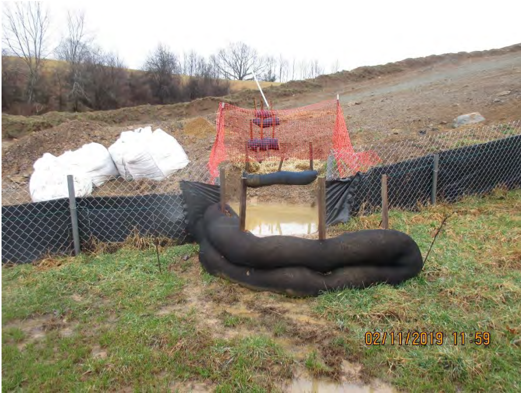
Waterbar terminus near station 5985+50 facing upslope
