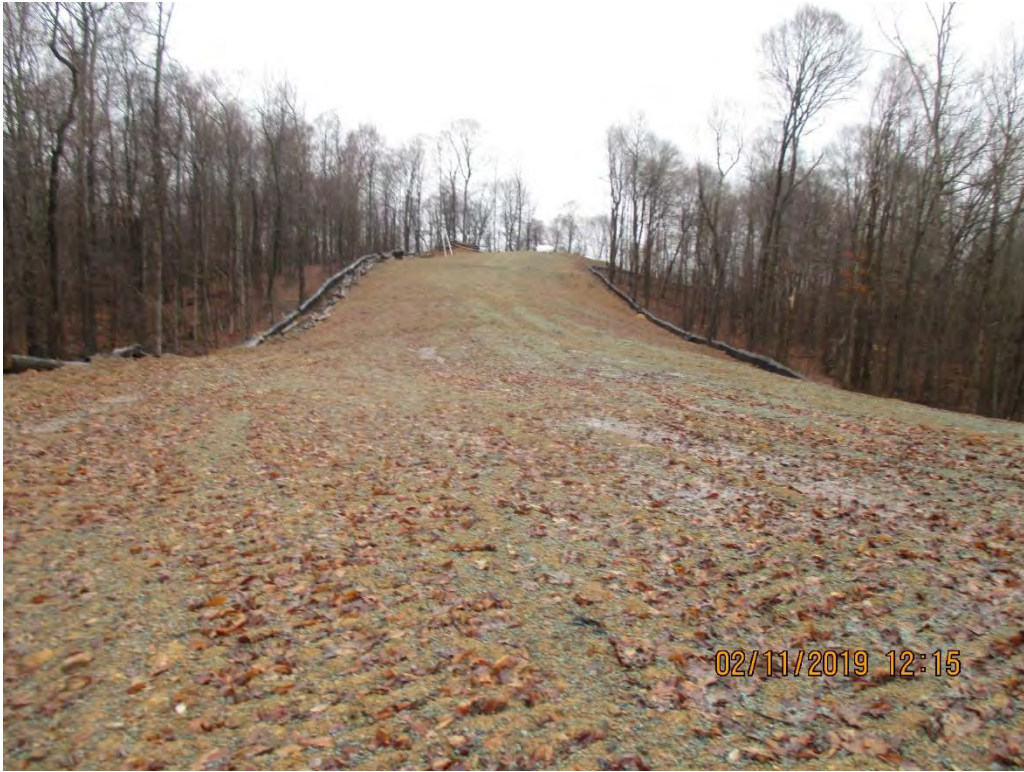
Slope at station 5966+50
