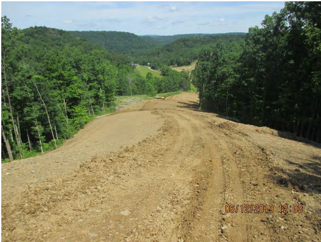
Facing North towards Anne's Branch at station No. 9745+00.
