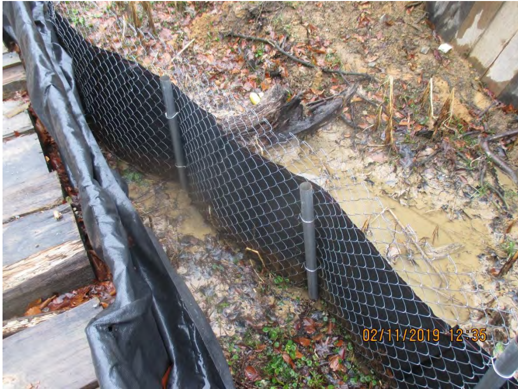
Super Silt fence present in Wetland W-IJ-55
