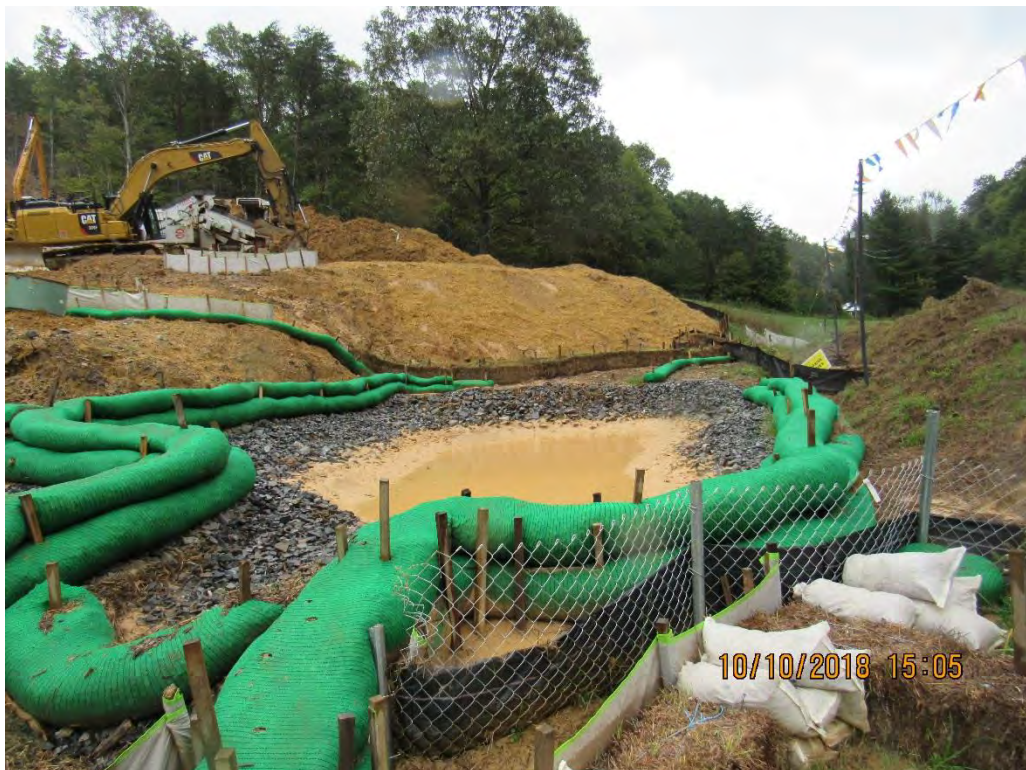
Photo 20: Painter's Run Road station 10270- maintenance performed abating NOV# W18-52-012-CP.
