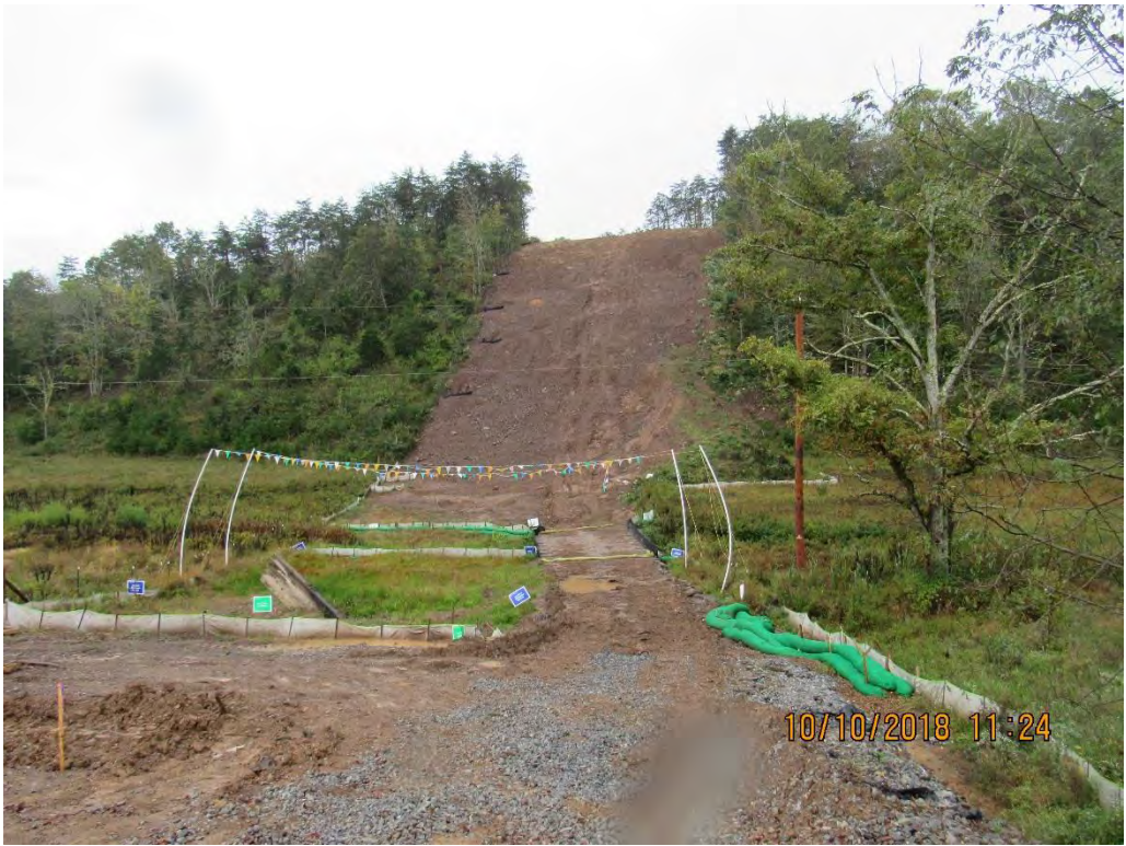
Photo 10: Wayside/Talcott station 9466 with rough grading completed awaiting final grade and restoration.
