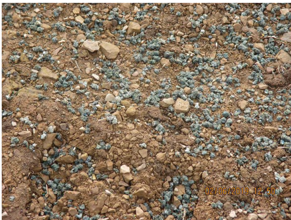
Aerial Pellets present on MVP ROW. Typical coverage observed during inspection.
