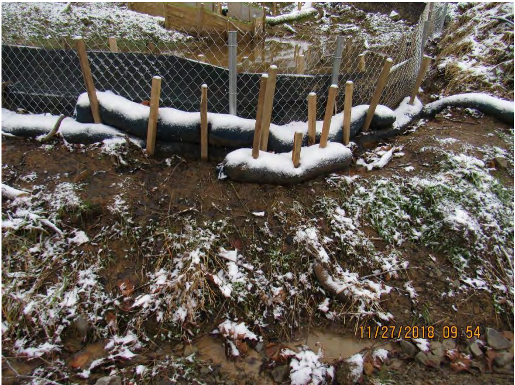
Photo 2: Clear water release from additional controls near station 3634 abating NOV# W18-52-010-CP.
