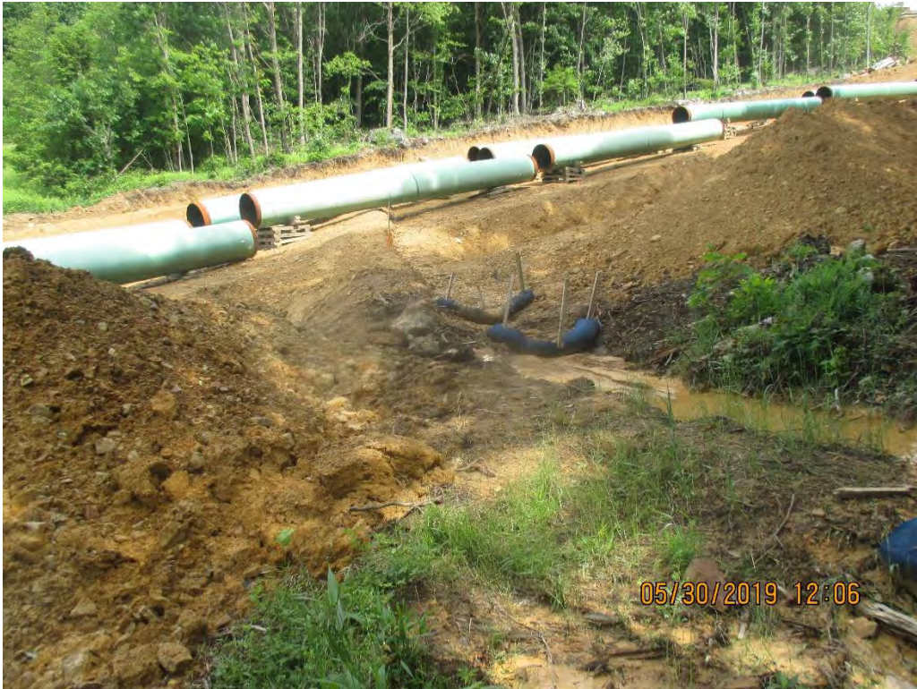
Waterbar at station No. 6510+40 facing upslope.
