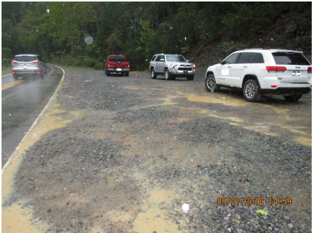
SLW accumulating and draining towards roadside ditch that intersects with S-A60 along Route122.
