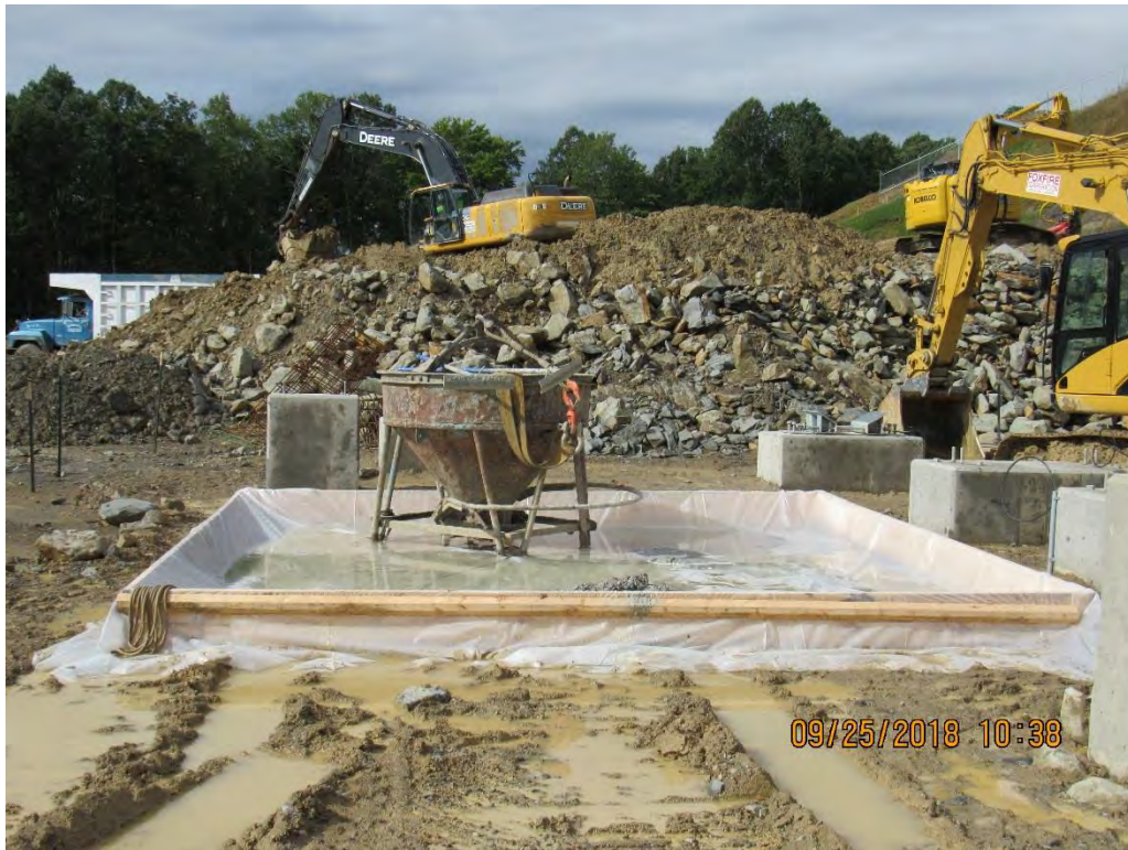
Photo 9: Properly installed concrete washout device abating NOV# W18-52-007-CP.
