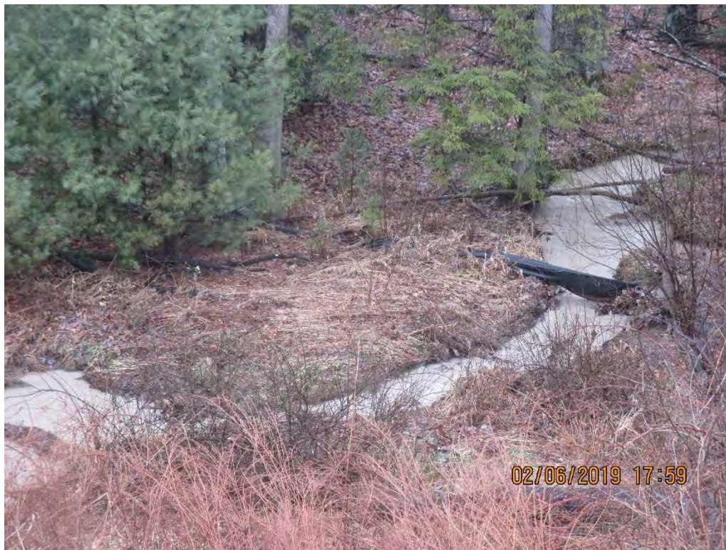
UNT of Brammer Branch downstream of culvert that conveys under MVP construction yard entrance.
