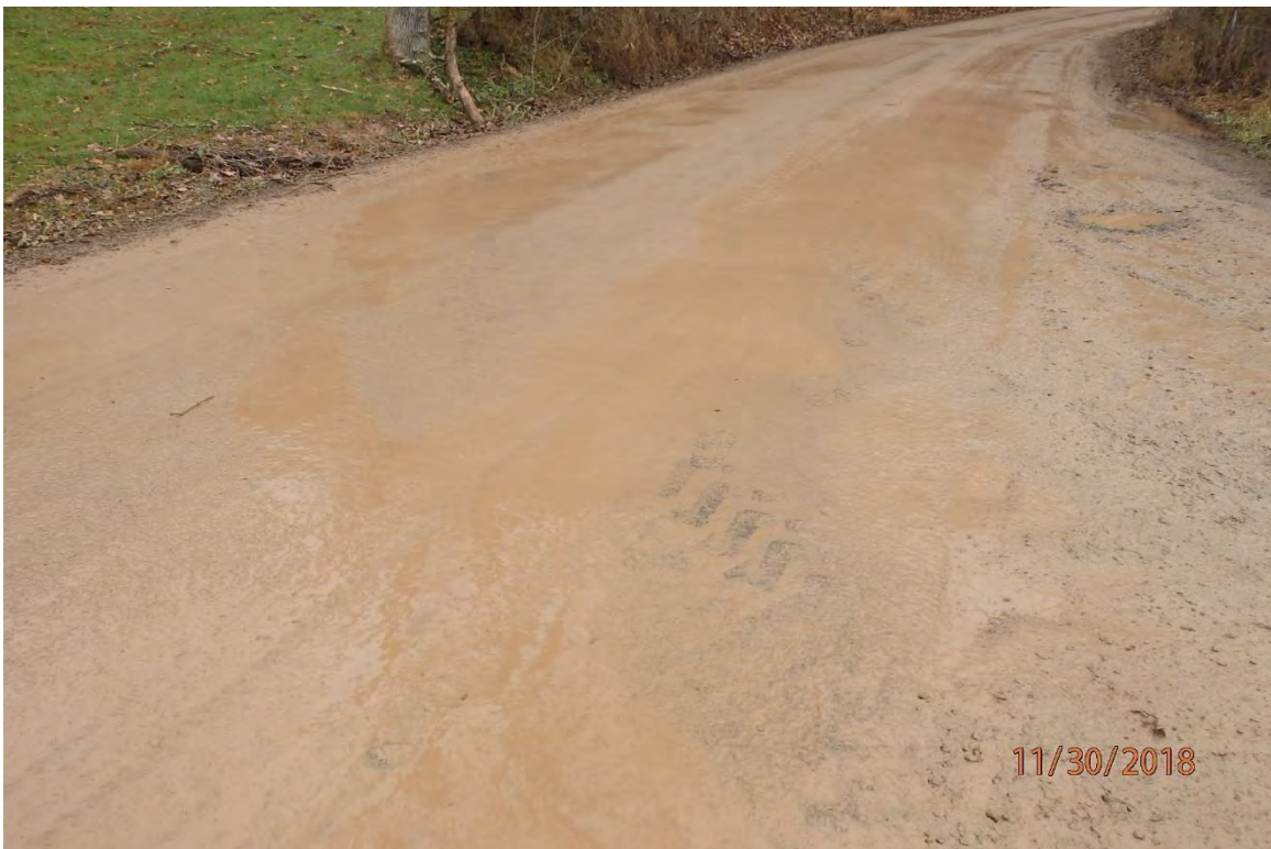
Access Road WV-HA - 29.04 off CR 50/5 showing the lack of an adequately stable construction entrance and the associated track out onto the public road.
