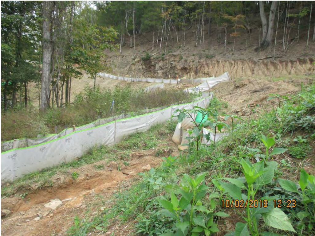
Lack of fill slope protection and channel stabilization enhancing erosion and causing BMP to be overwhelmed at station 9687.
