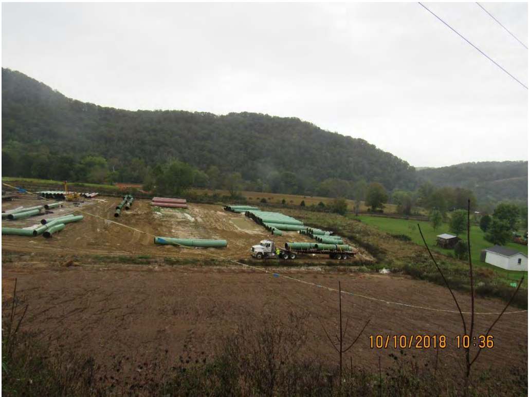
Photo 7: Lowell Road station 9087 laydown yard.
