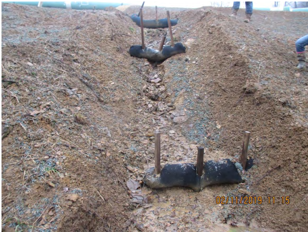
Waterbar on steep slope leading to outlet near station 6017+50
