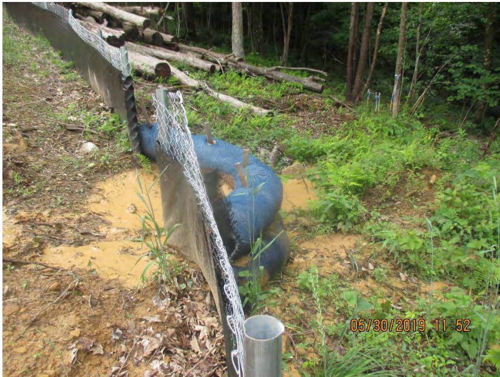
Waterbar outlet near station No. 6508+30. Sediment deposits past controls and LOD observed.
