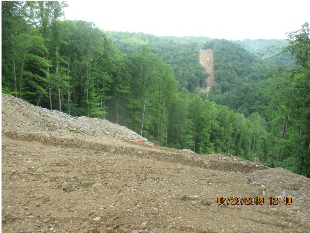
Facing Little Kanawha river basin and crossing near station No. 3973+00.
