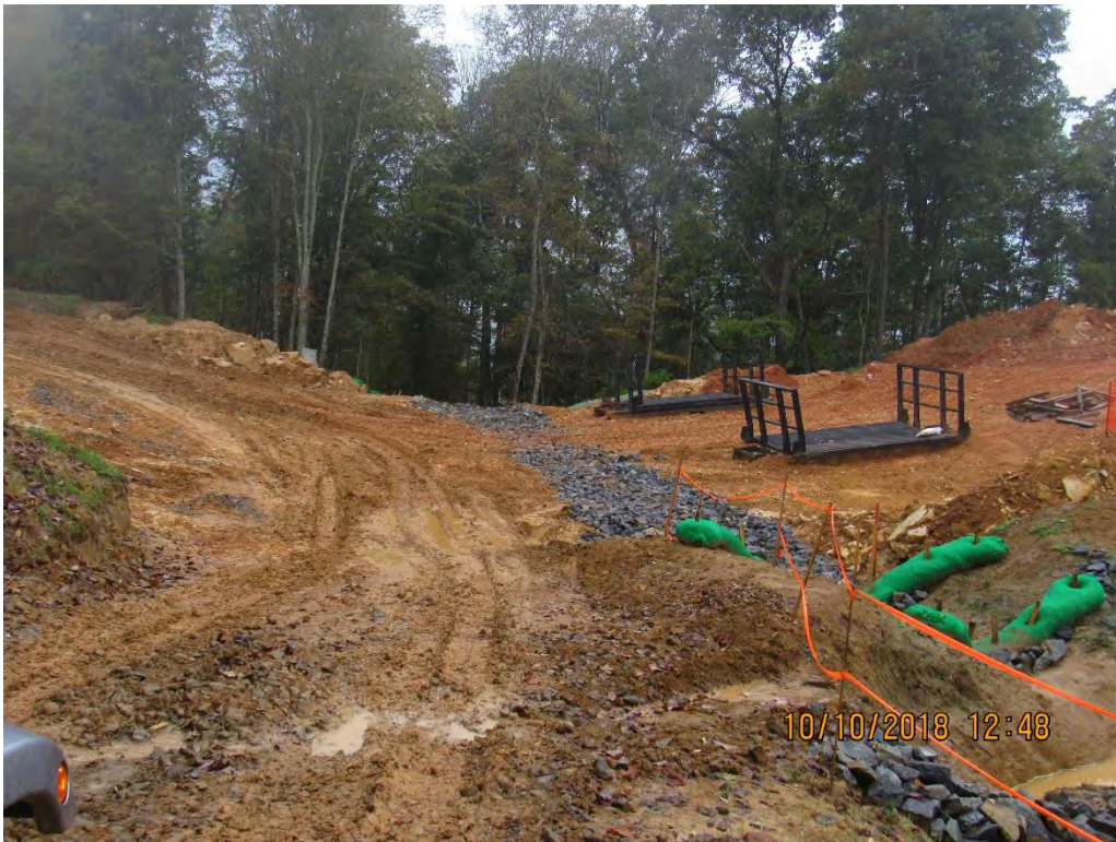
Photo 15: AR 224 at ROW station 9850+50 with diversion ditch across ROW.
