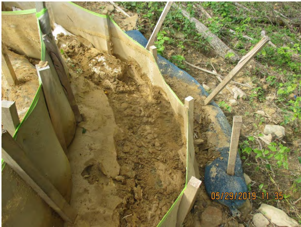
Perimeter outlet control's below Waterbar terminus at station No. 4027+00.
