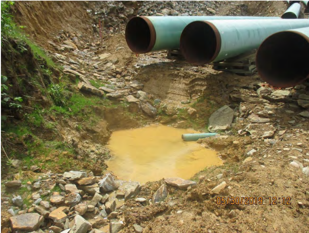
Sump with slope drain inlet for seep at station No. 6510+40.
