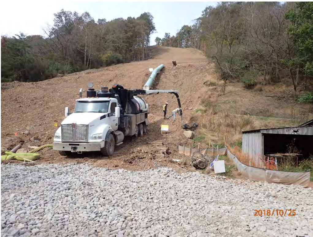
Contractors cleaning out sump near staging area off Sams Run Road.
