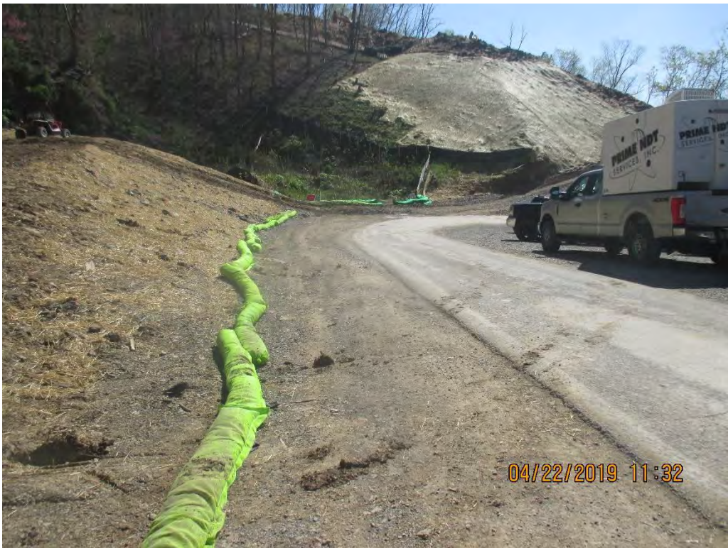
ATWS along Clayton Road/Fisher Hill Road with perimeter controls in place.
