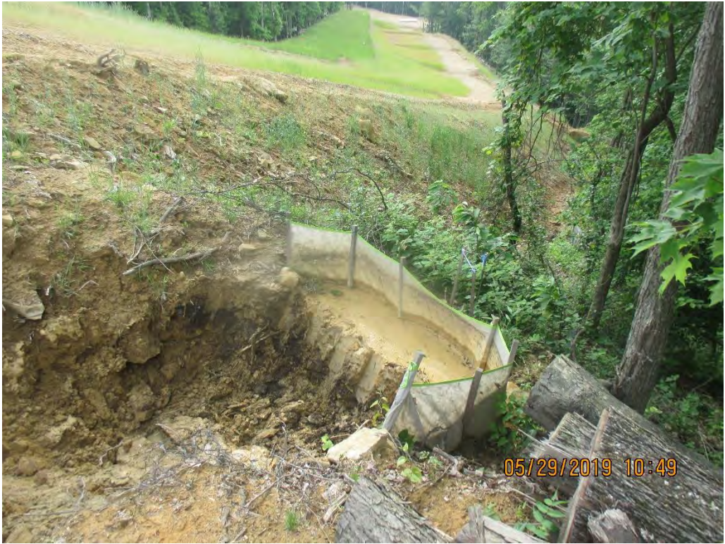
Waterbar outlet above fill slope at station no. 4031+00 facing downslope.
