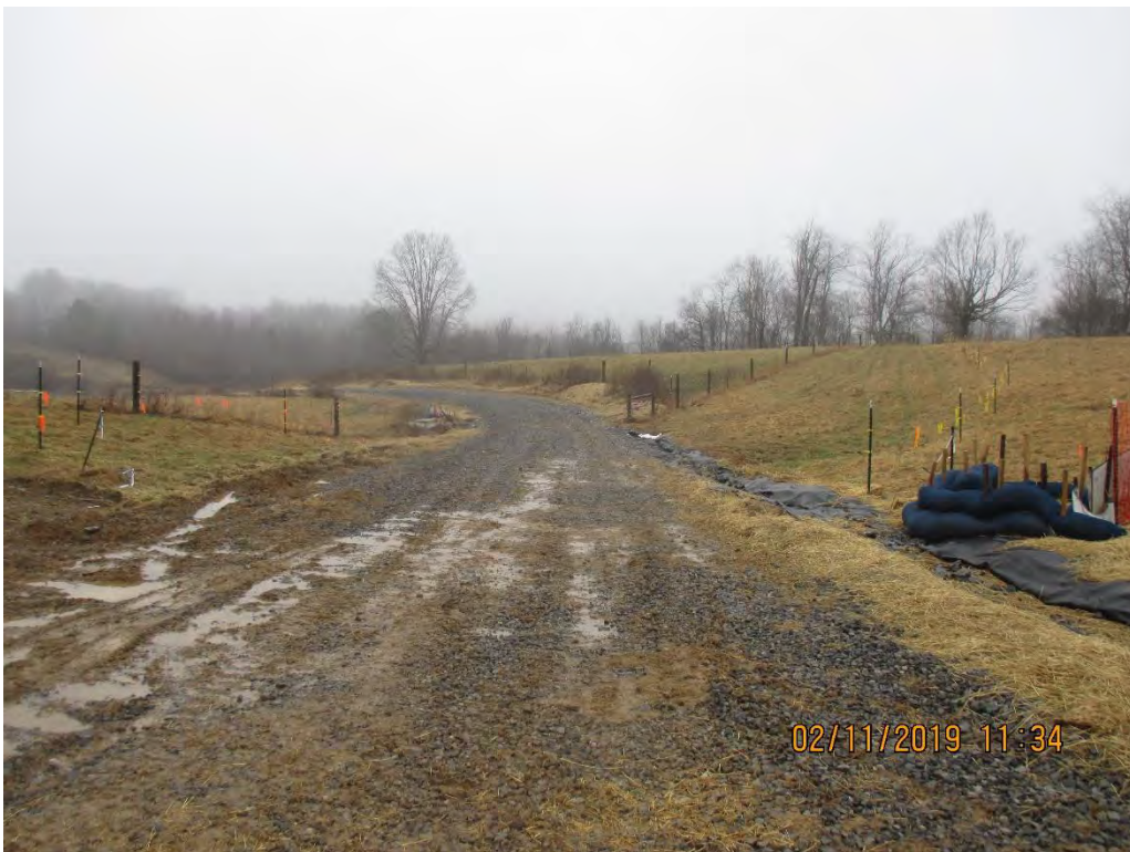
Access Road MVP-IN-141.01 facing West at station #5993+00
