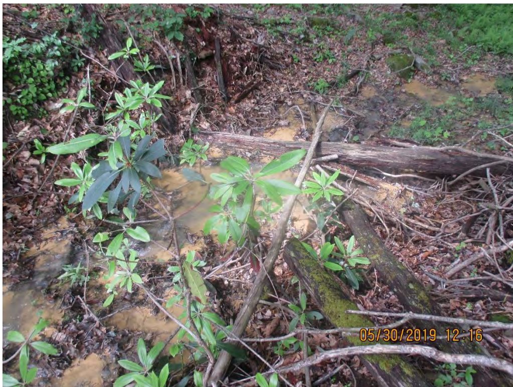
Sediment deposits and SLW observed past controls and LOD at station No. 6510+40.
