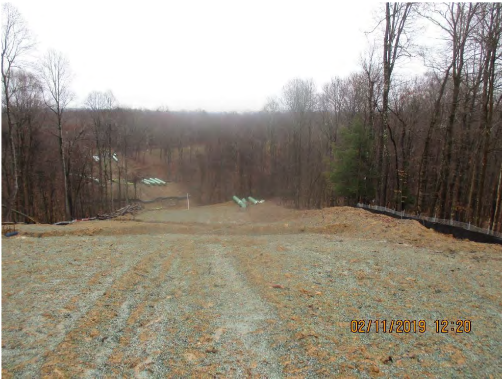
Facing North at Wetland W-IJ-55 and Stream Crossing W-QQ2
