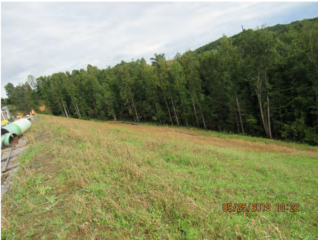
Photo 8: Re-vegetated slope on north eastern side of site abating NOV# W18-52-007-CP.
