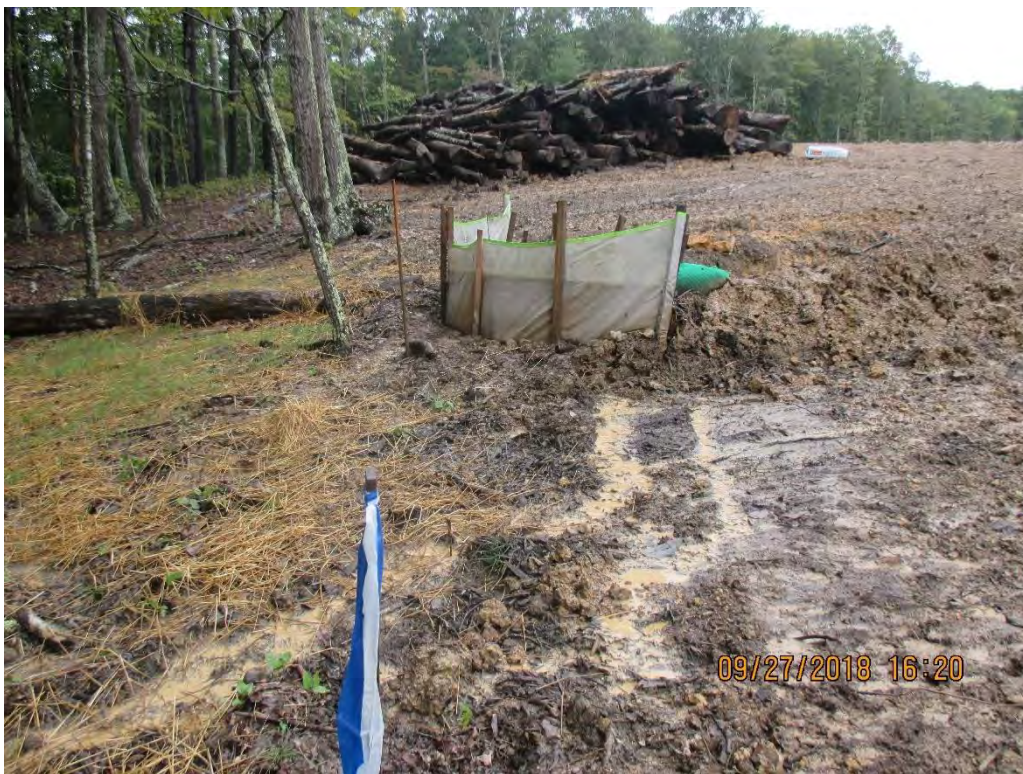
SLW flowing past BMP near Station #9417+75
