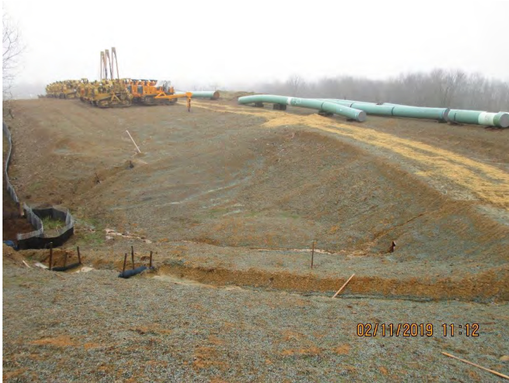
MVP ROW facing North standing at Rt 55 crossing at station #6017+50
