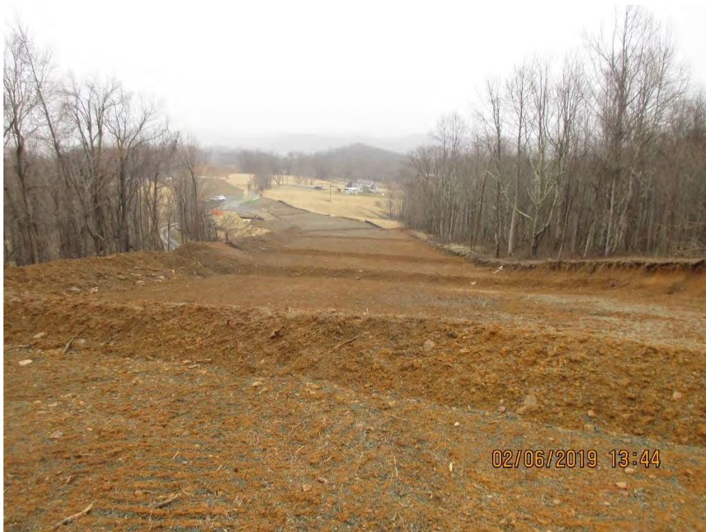
Facing South at MVP ROW and Access Road 202 at station #8816+00.
