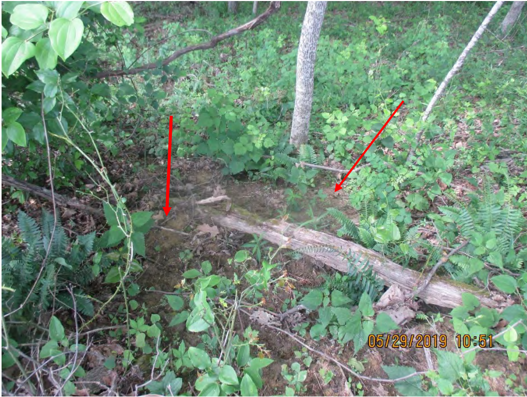
Waterbar outlet above fill slope at station no. 4031+00 facing downslope. Sediment deposits observed past LOD. Scouring from concentrated flow present.
