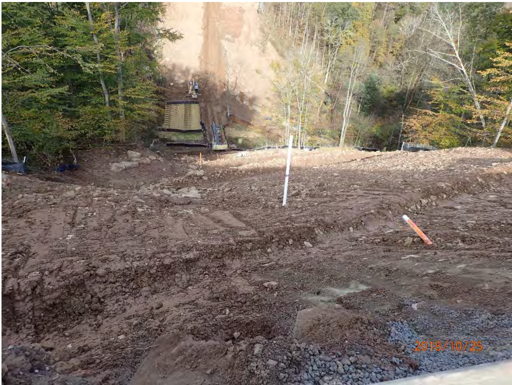
UNT to Mobley Run Waterbars had been reworked since last inspection.
