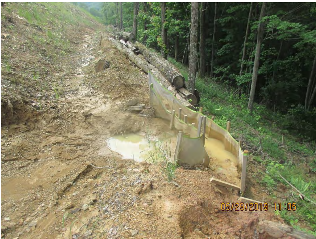
Standing further below diversion berm outlet No. 2 near 4031+00. Scouring of vegetation present below control. Sediment deposits were observed approximately 150-foot downslope of controls.
