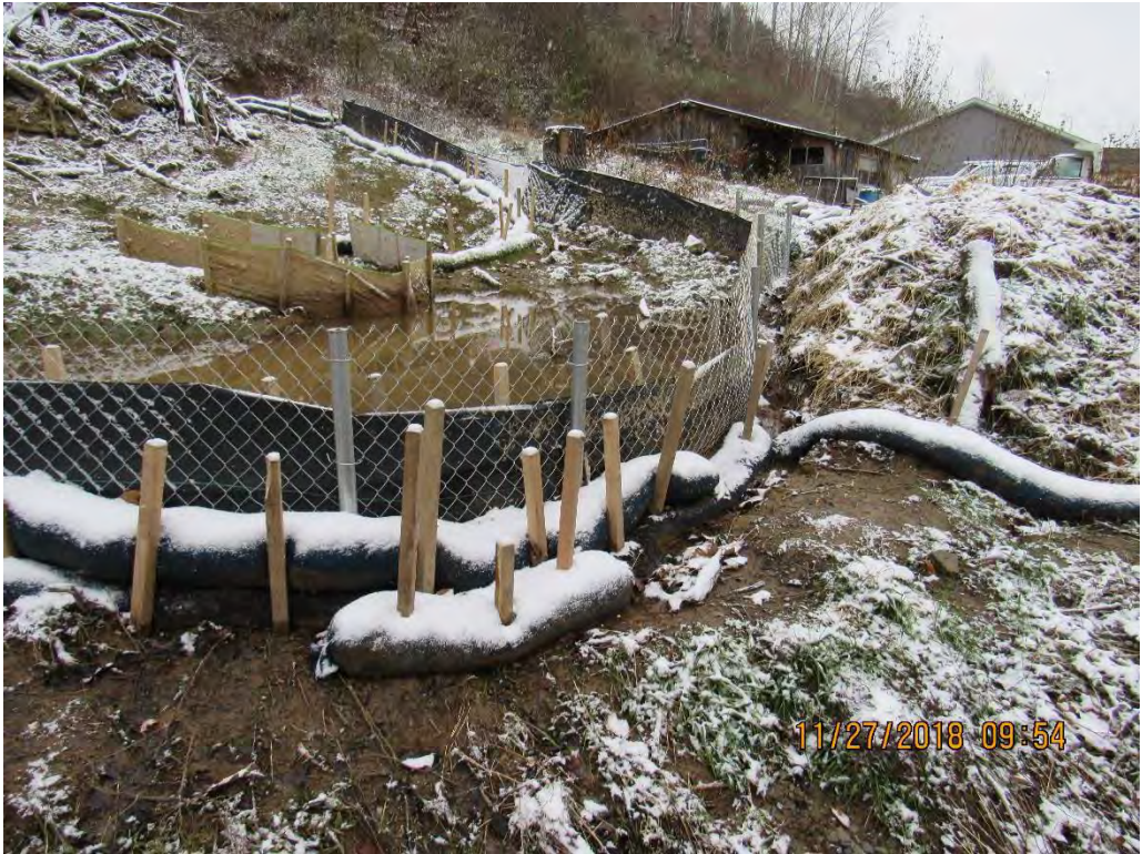
Photo 1: Near station 3634 location of NOV# W18-52-010-CP- additional controls added.
