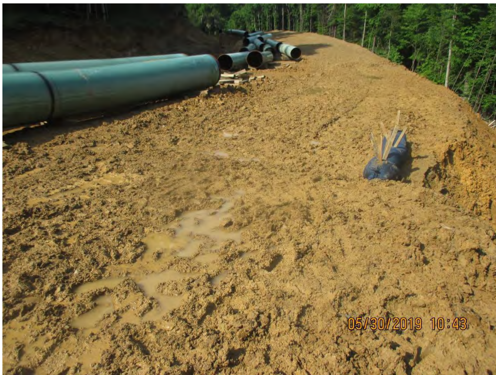
Waterbar outlet terminating onto slope near station No. 6485+10.
