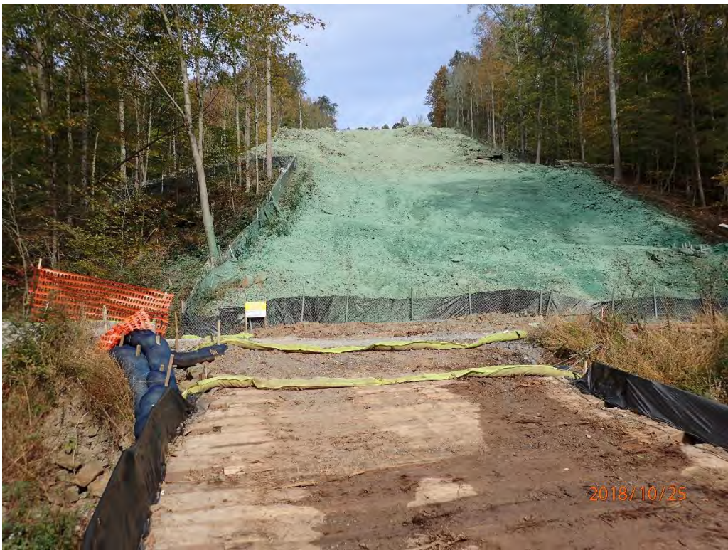
Fallen Timber crossing has been hydroseeded.
