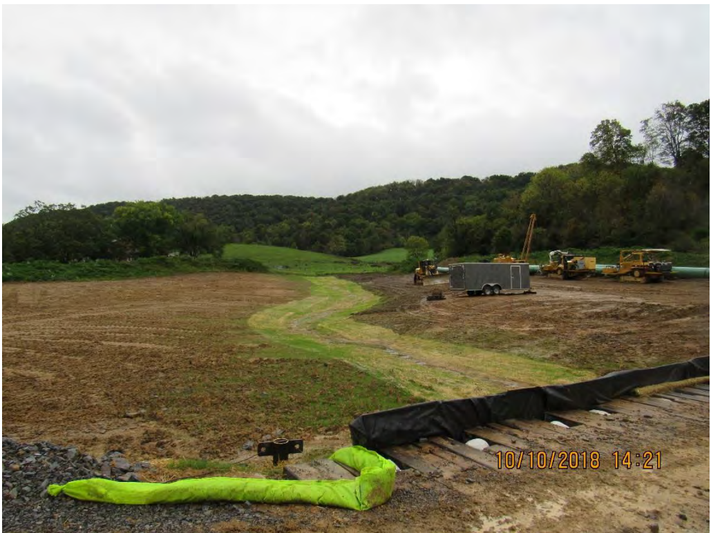
Photo 18: Established diversion for run-on from farmer's pond at Lindside Methodist Church station 10116.
