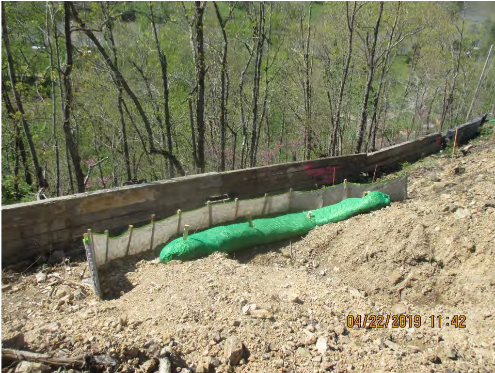
Waterbar outlet above clayton road crossing near station #9045+00
