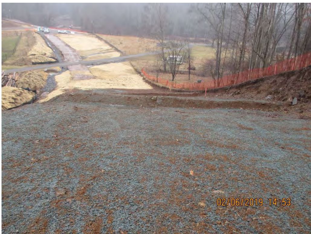
Facing North at MVP ROW near station 8966+00.
