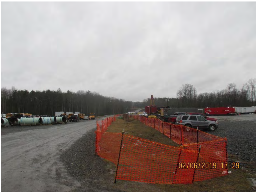
MVP contractor yard facing West towards drainage ditch and entrance.
