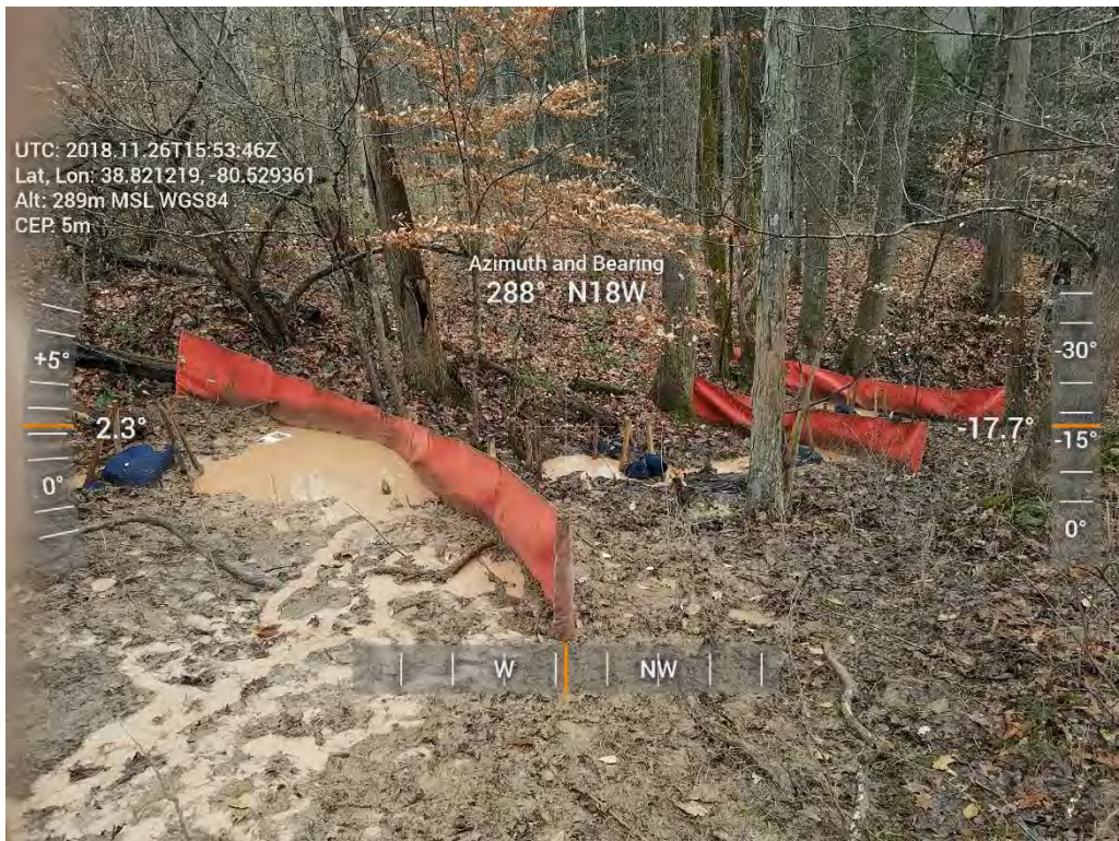
Photo 6: Receiving stream (UNT of Knawl's Creek) below release of slip with additional controls. Photo supplied by EI Andy Pauley.
