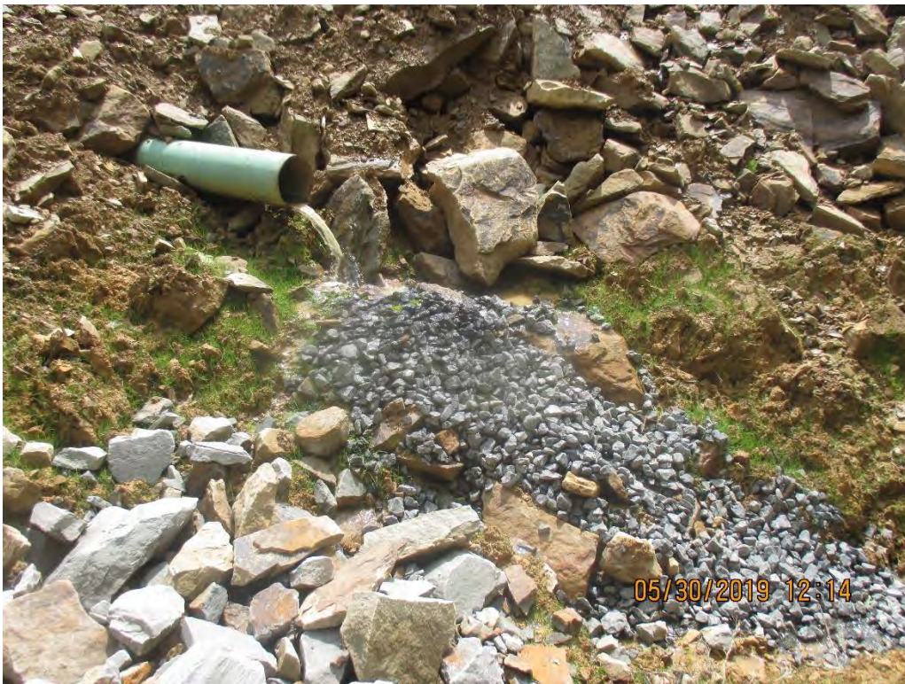
Seep slope drain outlet. Rock apron present.
