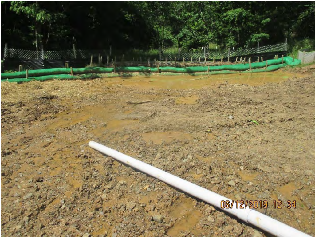
Pipe slope drain terminating onto ROW above controls (Dargo silt fence).
