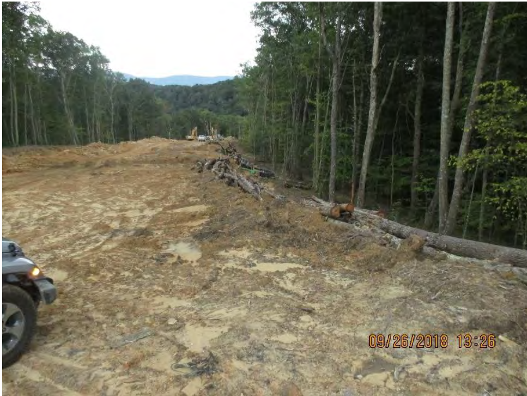
Area of ROW near Station #9897+00 looking towards Hans Creek drainage.
