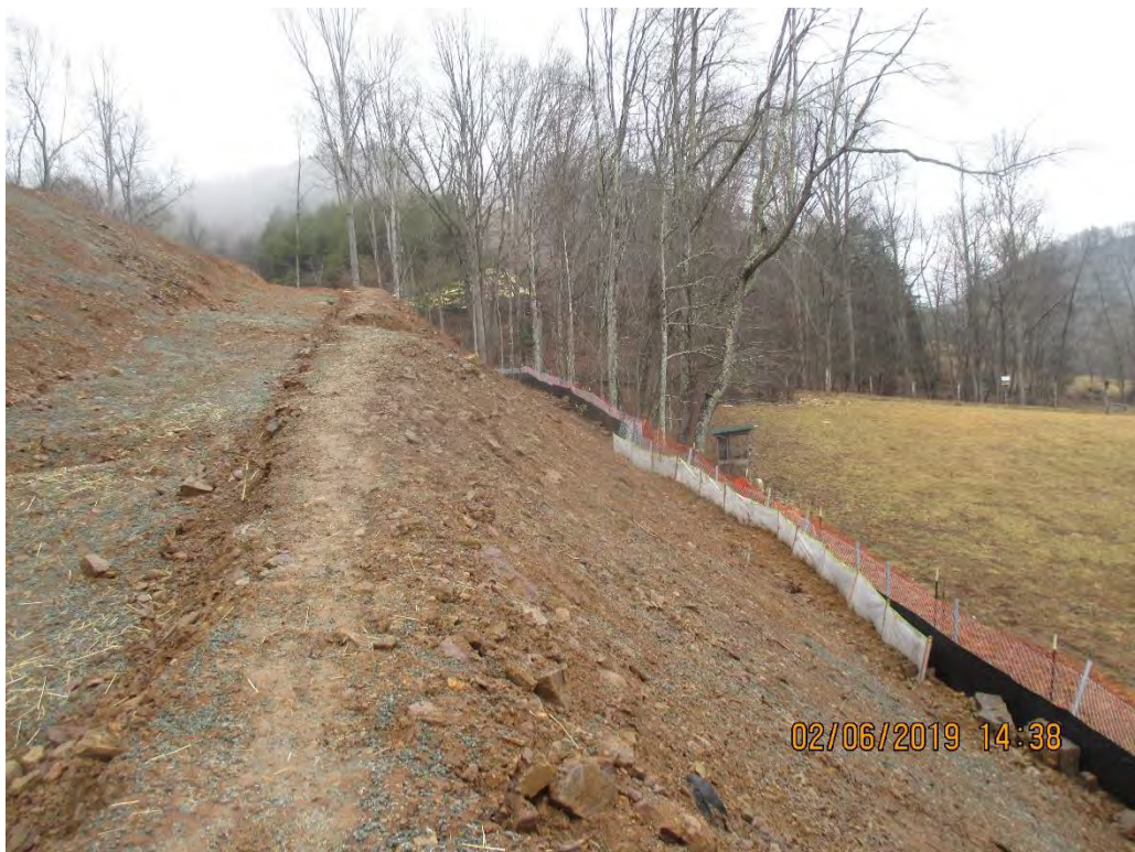
North of station #8966+00 looking at East side of MVP ROW.
