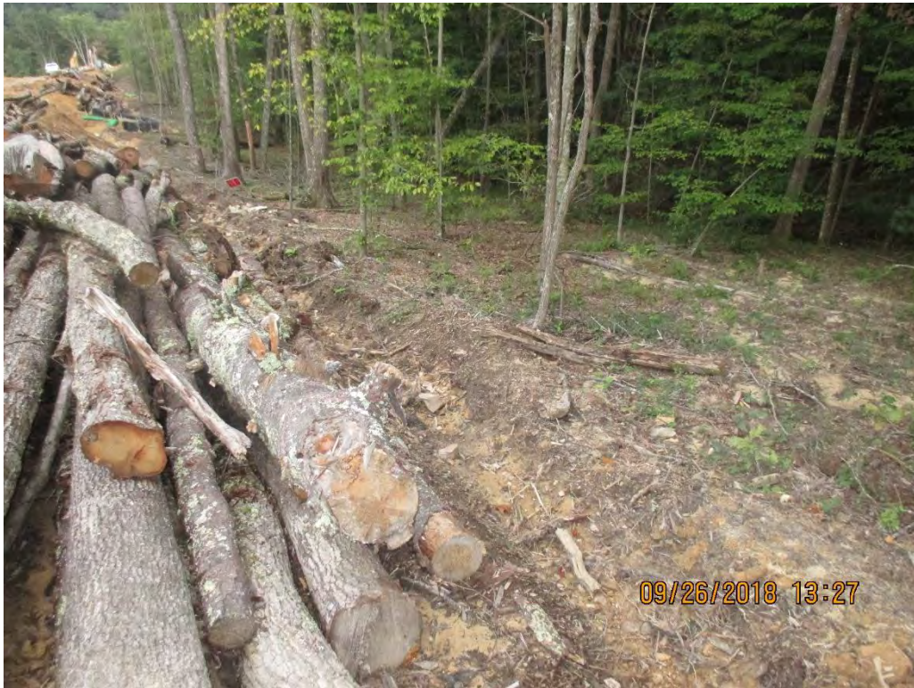
Off-site sediment deposits near Station number 9899+00.
