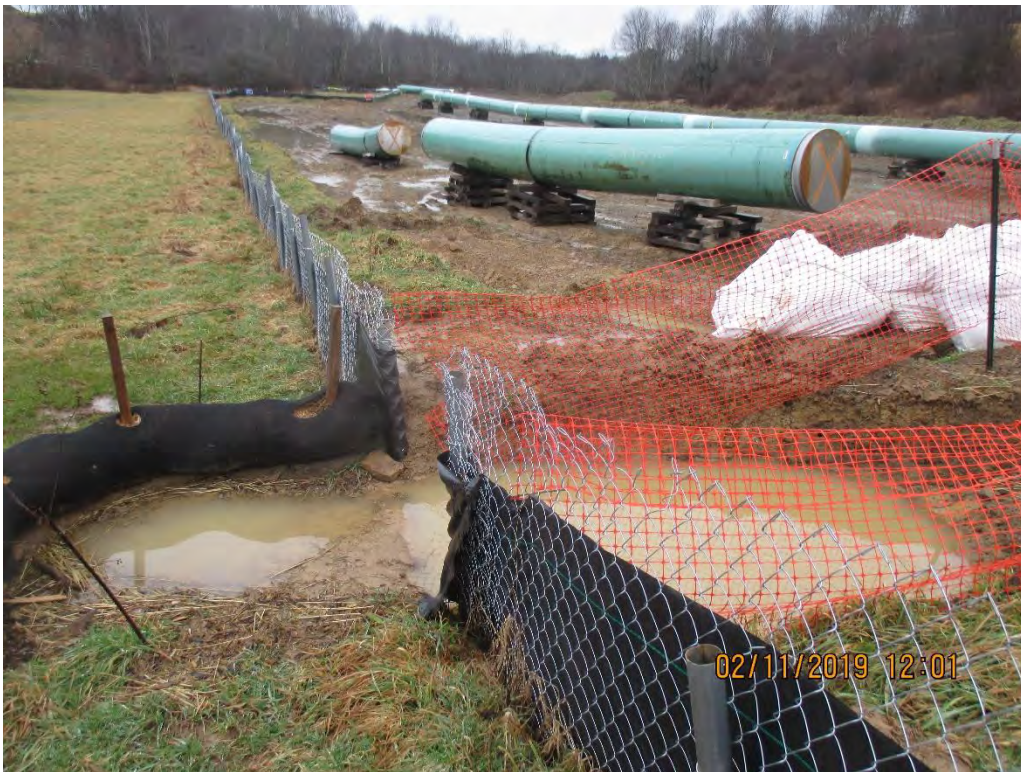
Waterbar terminus near station 5985+50 facing towards Stream crossing S-B28
