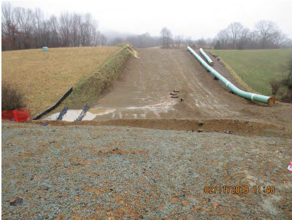
Facing North at MVP ROW near station #5999+50
