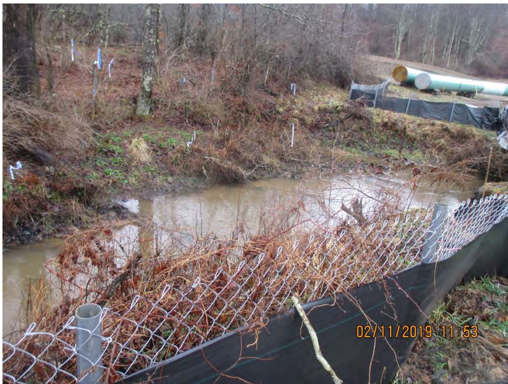
Stream S-B28 adjacent to Wetland B-27 near station 5981+90 (per SWPPP)
