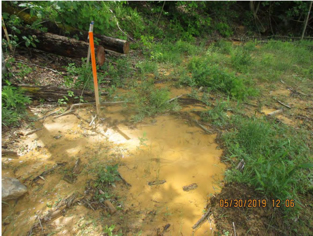
Sediment deposits downslope of Waterbar outlet at station No. 6510+40.
