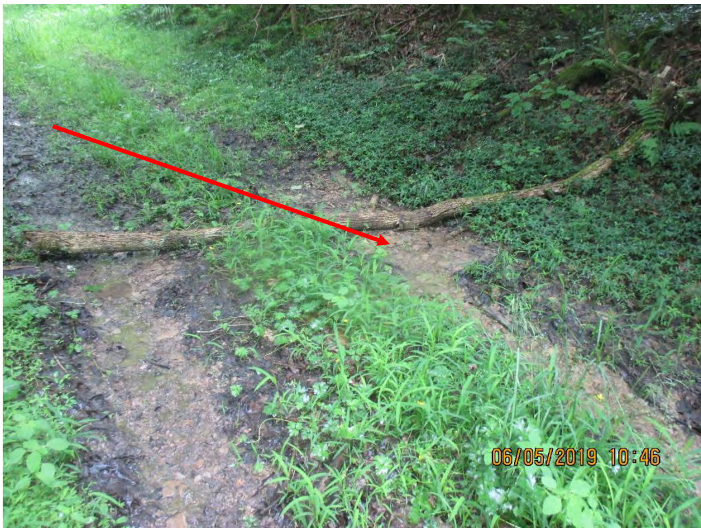
Sediment deposits approximately 500 feet past the LOD downslope of construction entrance.
