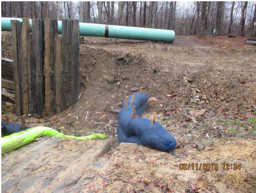
Facing upslope above wetland W-IJ-55
