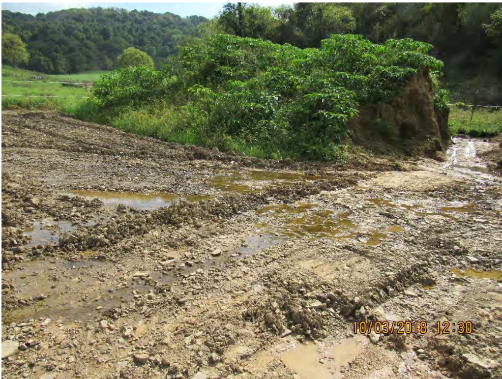
Photo 6: Run on water lacks an established channel through site at Lindsie Methodist Church station 10116+49.
