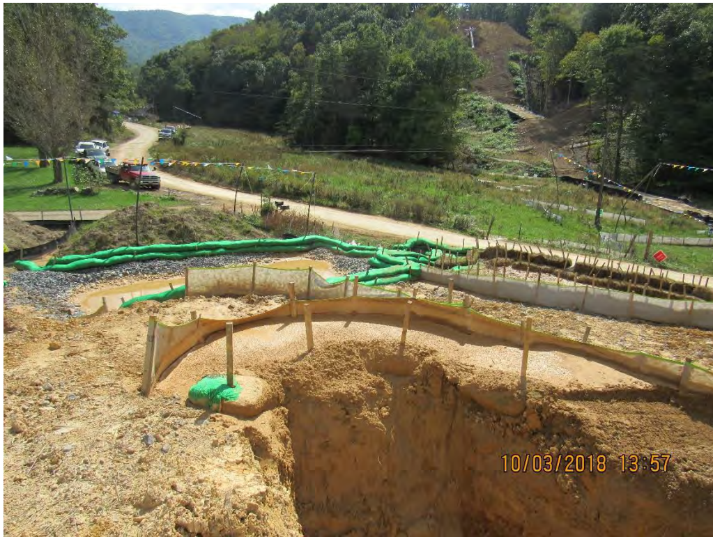
Photo 3: Front of control on right in Photo 2 after maintenance performed at Painter's Run station 10270.
