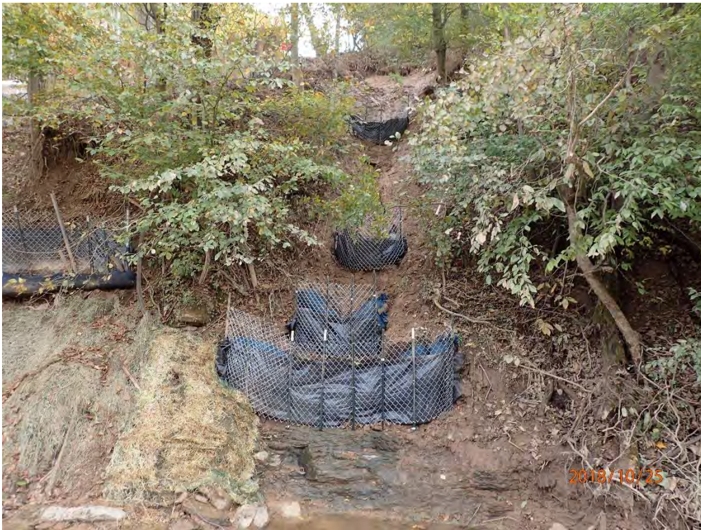
Slip off Sams Run with controls in place.
