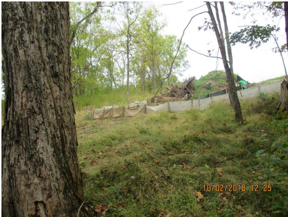
Opposite side of slope where BMP is being overwhelmed.
