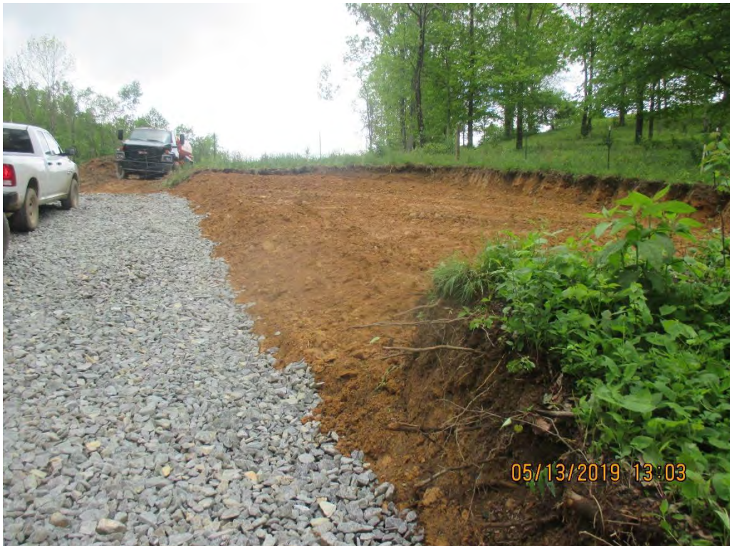
Construction entrance and additional parking space adjacent to Duncan Branch Road.
