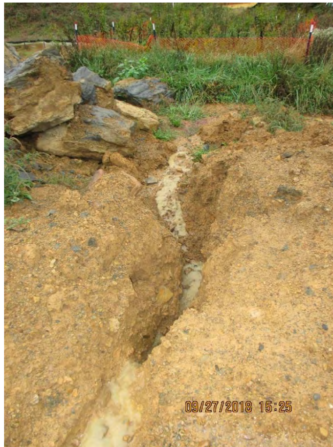
Water bar terminus leading to BMP. Erosion occurring due to channel not being stabilized.
