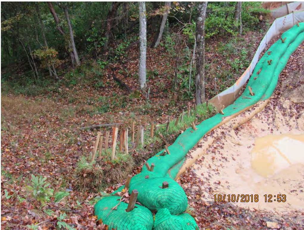
Photo 16: AR 224- sump at end of diversion ditch across ROW station 9850+50 and down slope/outlet of sump.
