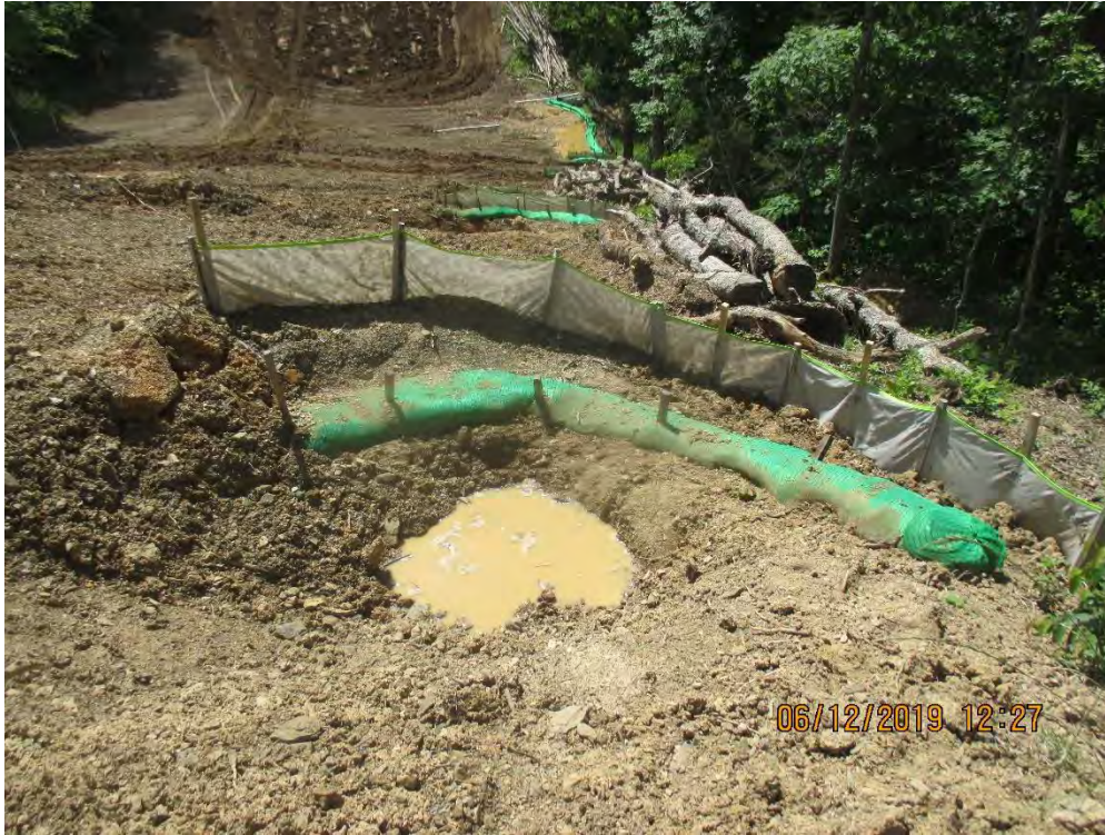
Facing Downslope at Dargo silt fence. Waterbar outlets in place with controls in foreground.
