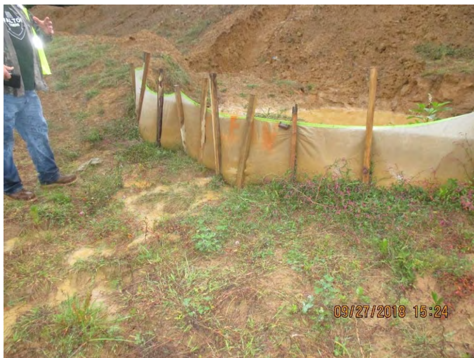
Sediment Laden water passing through/Under BMP.
