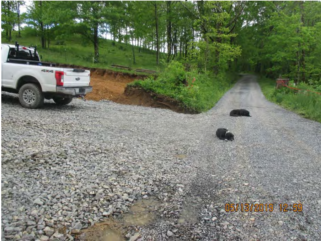
MVP ROW crossing with Duncan Branch Road near station #8399+10
