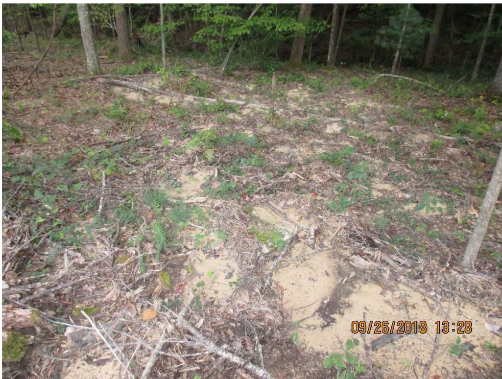
Off site sediment deposits located past LOD and being transported towards Streams S-H58 and TTWV-S-E58 near Station number 9899+00.
