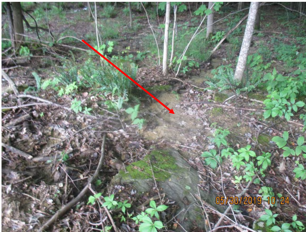
Sediment deposits past LOD and controls at station No. 6474+16. Arrow depicts deposits.
