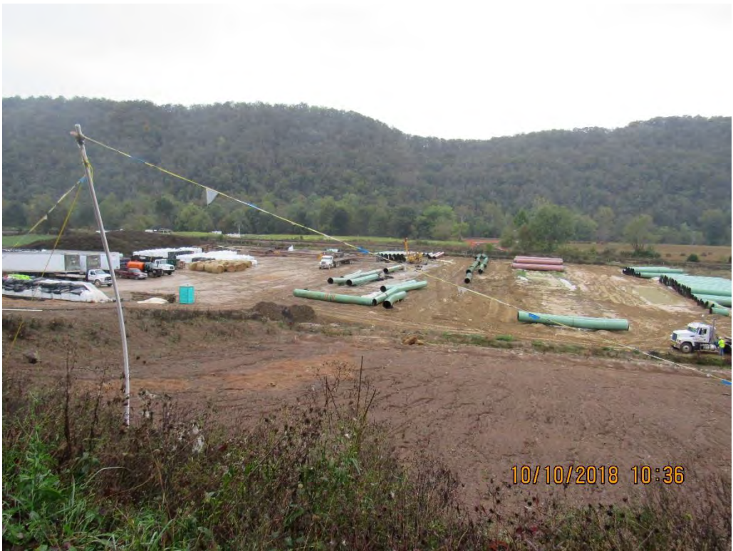
Photo 8: Lowell Road station 9087 laydown yard.
