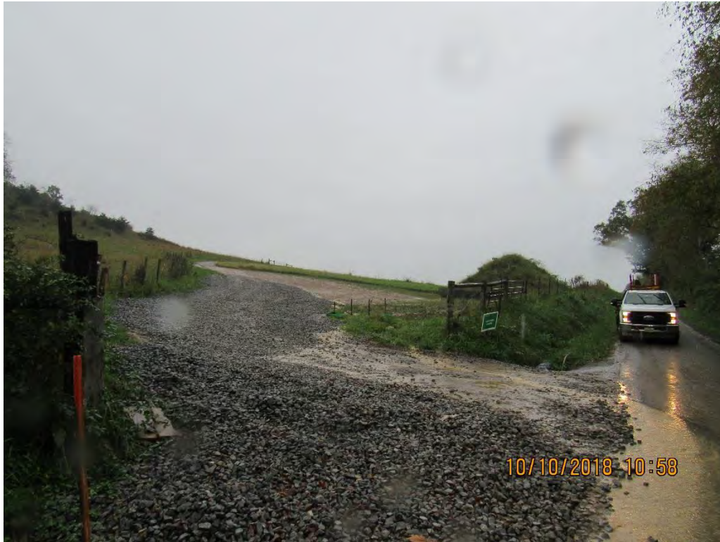
Photo 1: AR 210- sediment laden water leaving site.
