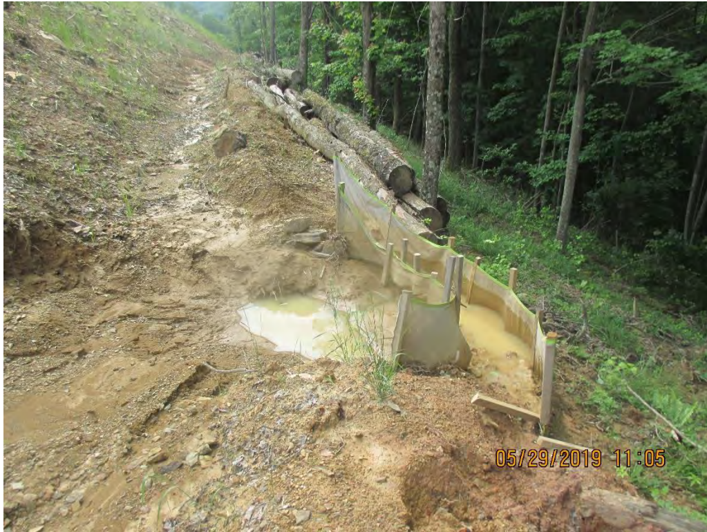
Diversion berm outlet No. 3. Sediment being deposited behind controls.
