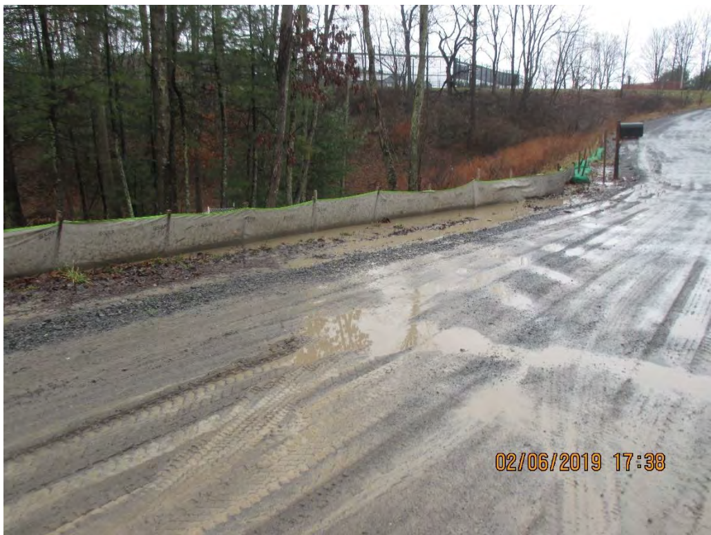
View facing towards culvert outflow and MVP yard entrance.
