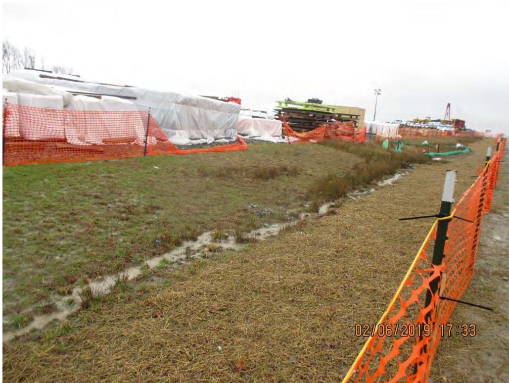
View of drainage ditch and wetland facing upslope (west).
