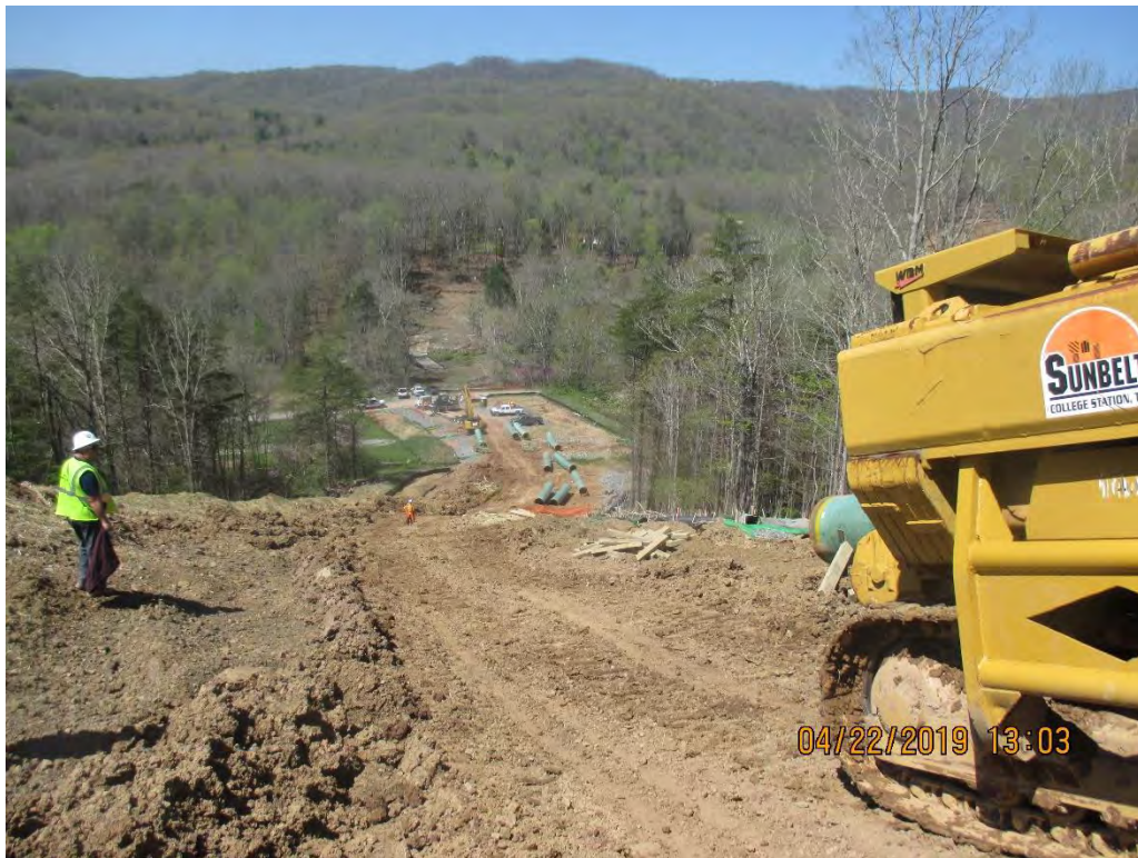
Standing above West Clayton Road facing North near station #9004.
