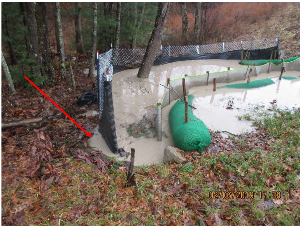
Controls downstream of culvert. SLW present going around controls.
