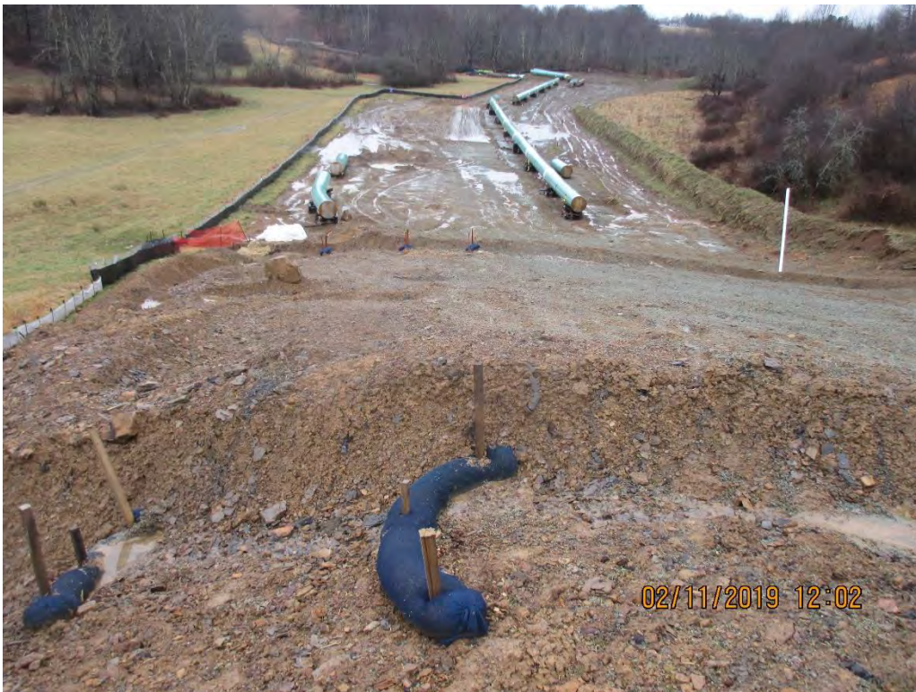
Facing West towards Stream Crossing S-B28 near station 5985+50
