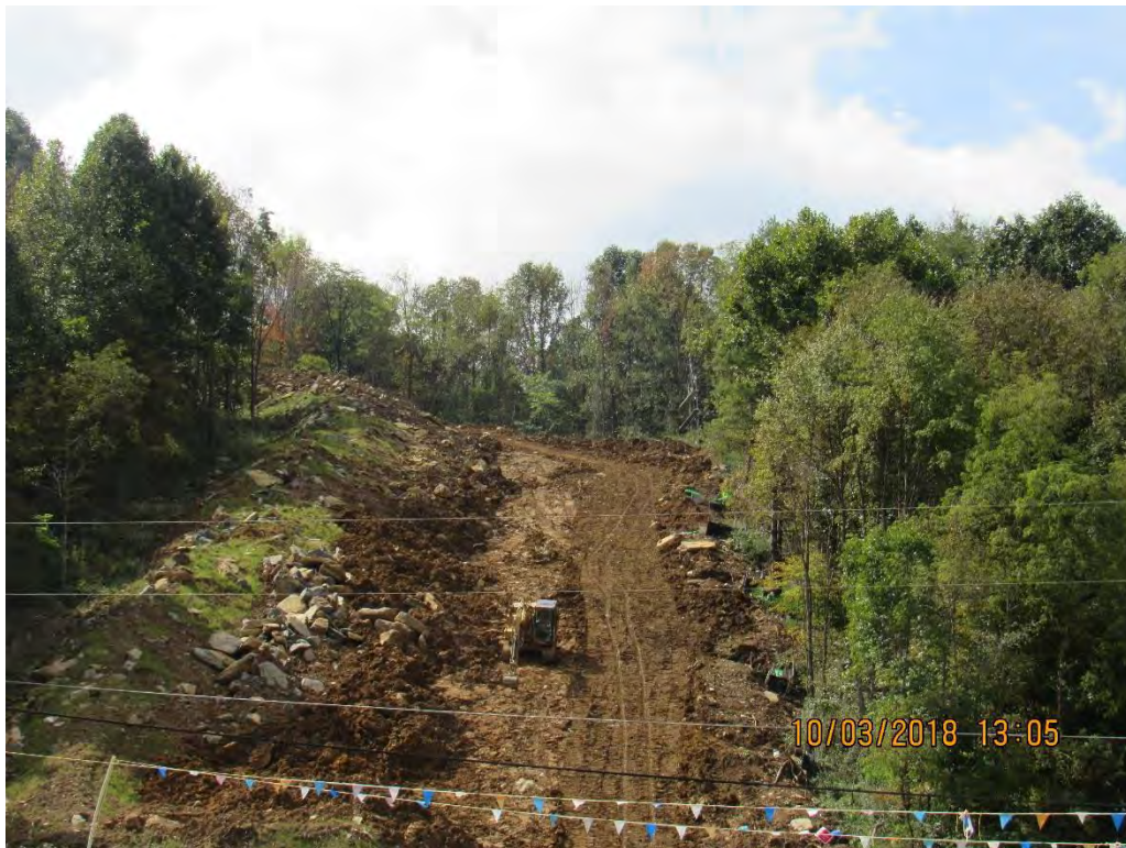
Photo 10: Back Valley Road station 10146+32- trenching/ditching has not started.
