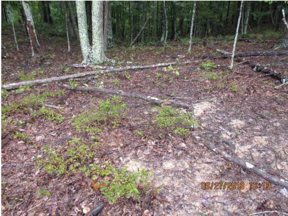
Area above spring/seep where off site sediment deposits were observed past LOD.
