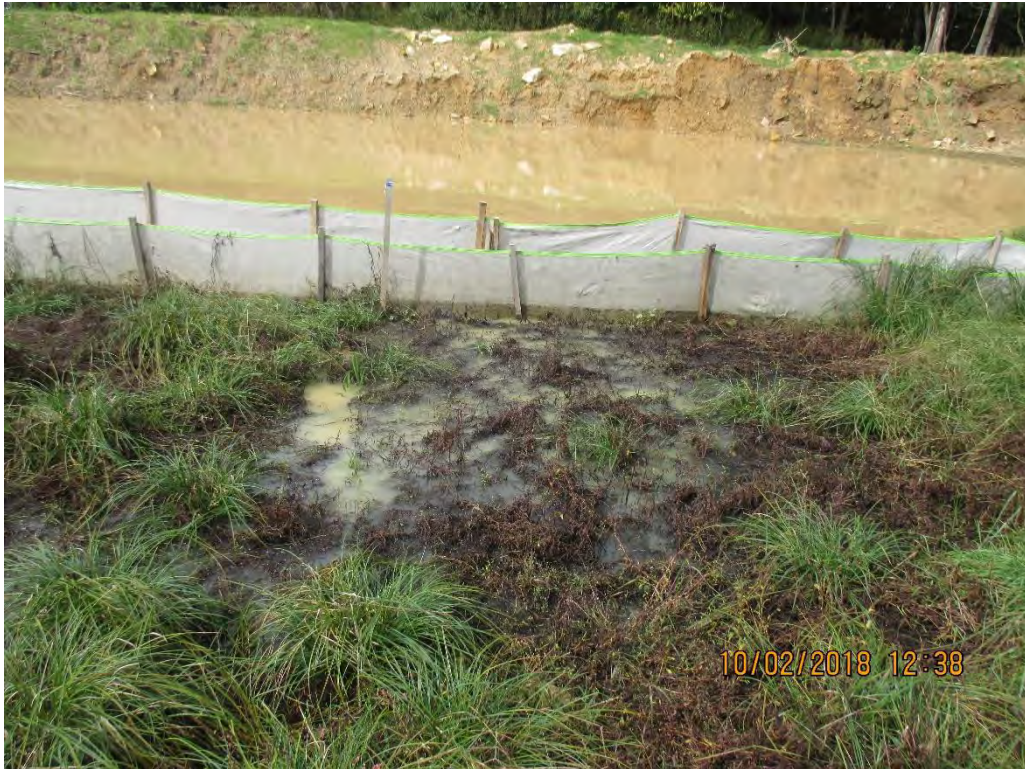
Sediment laden water infiltrating pond P-D2.
