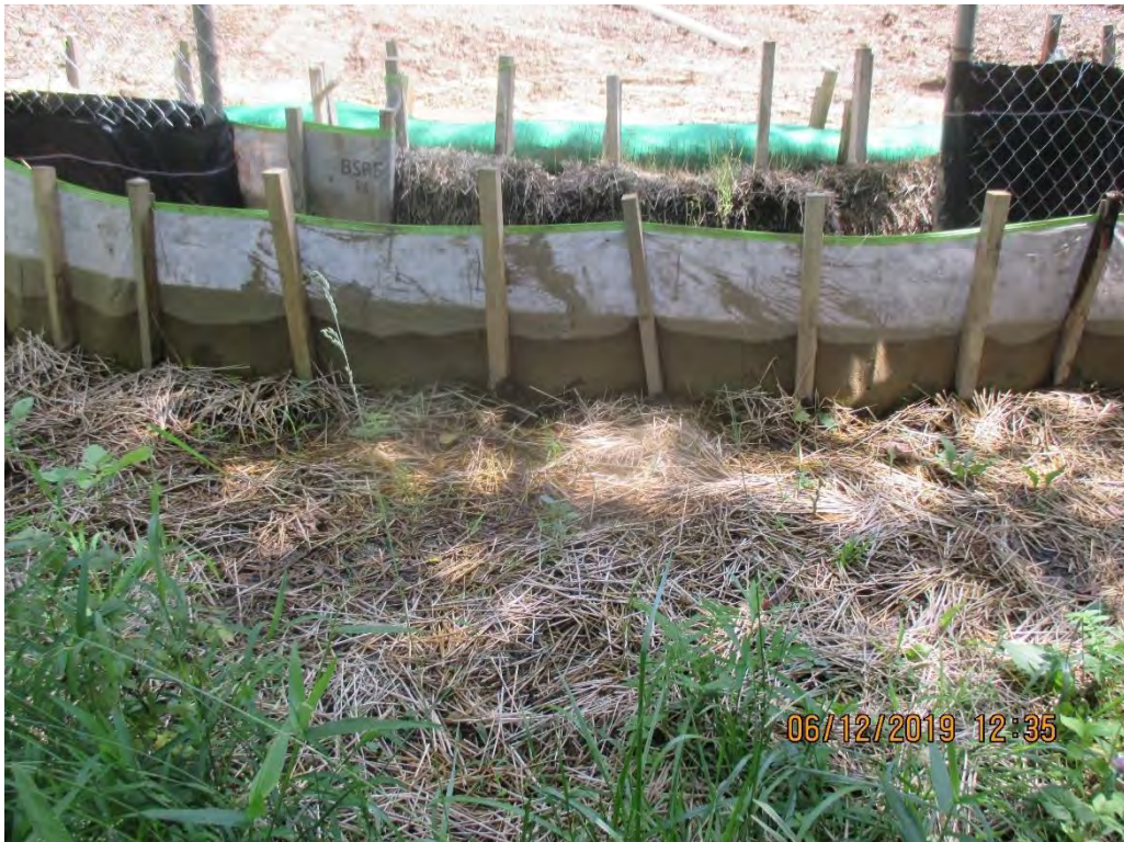
Standing below Dargo Silt fence facing upslope at controls.
