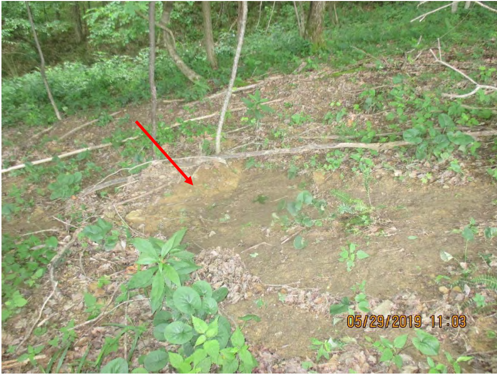
Standing further below diversion berm outlet No. 2 near 4031+00. Scouring of vegetation present below control. Sediment deposits were observed approximately 150-foot downslope of controls.
