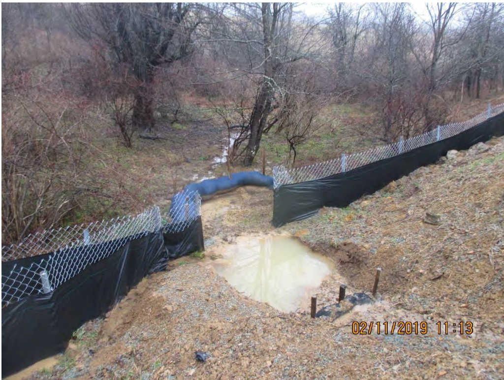
Outlet along perimeter control near station 6017+50
