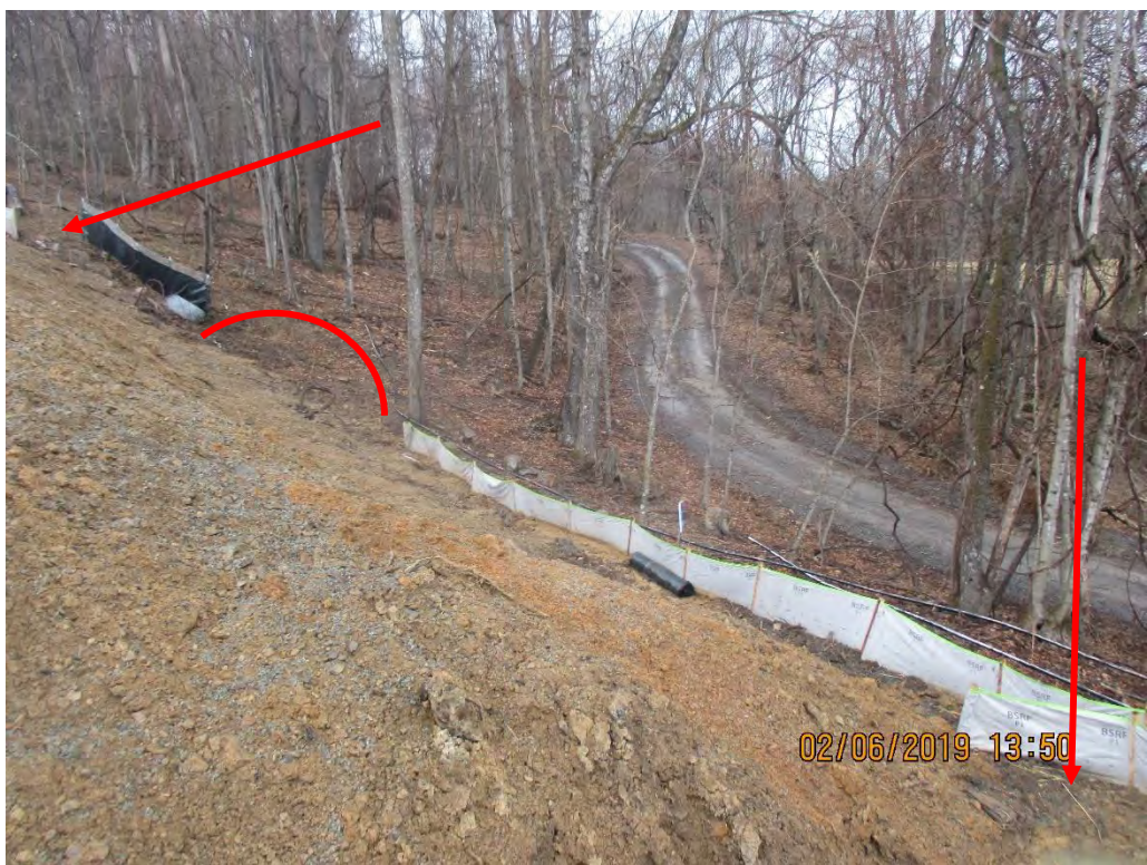
Waterbar outlet at station number 8816+00.
