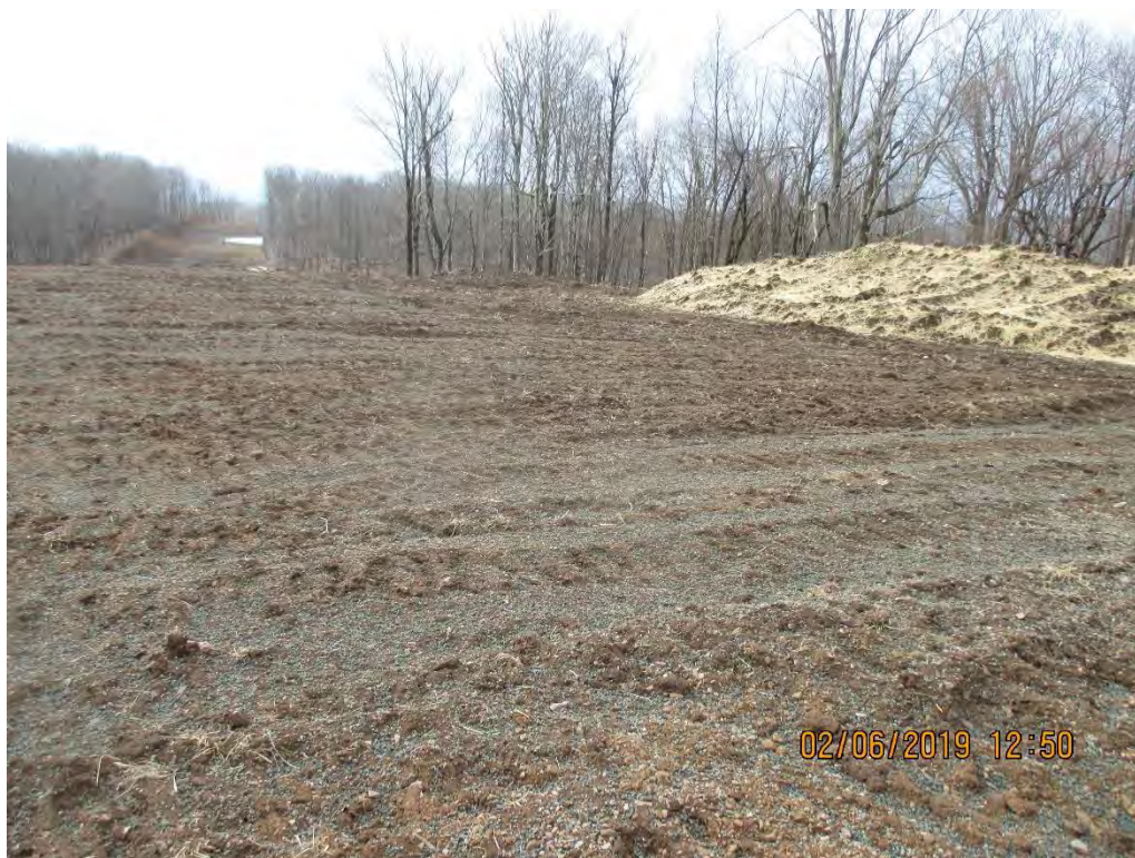
Facing South at ROW from ATWS 304A at Station #8776+03
