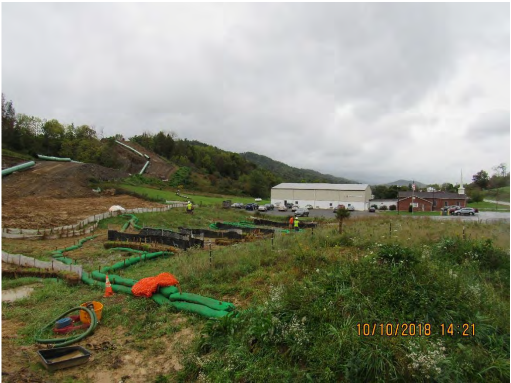
Photo 17: Lindside Methodist Church station 10116 with workers performing maintenance on controls below bridge.
