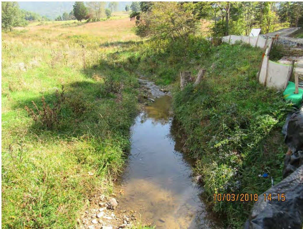
Photo 12: UNT of Painter's Run clear after repairs made. Abates NOV# W18-52-009.
