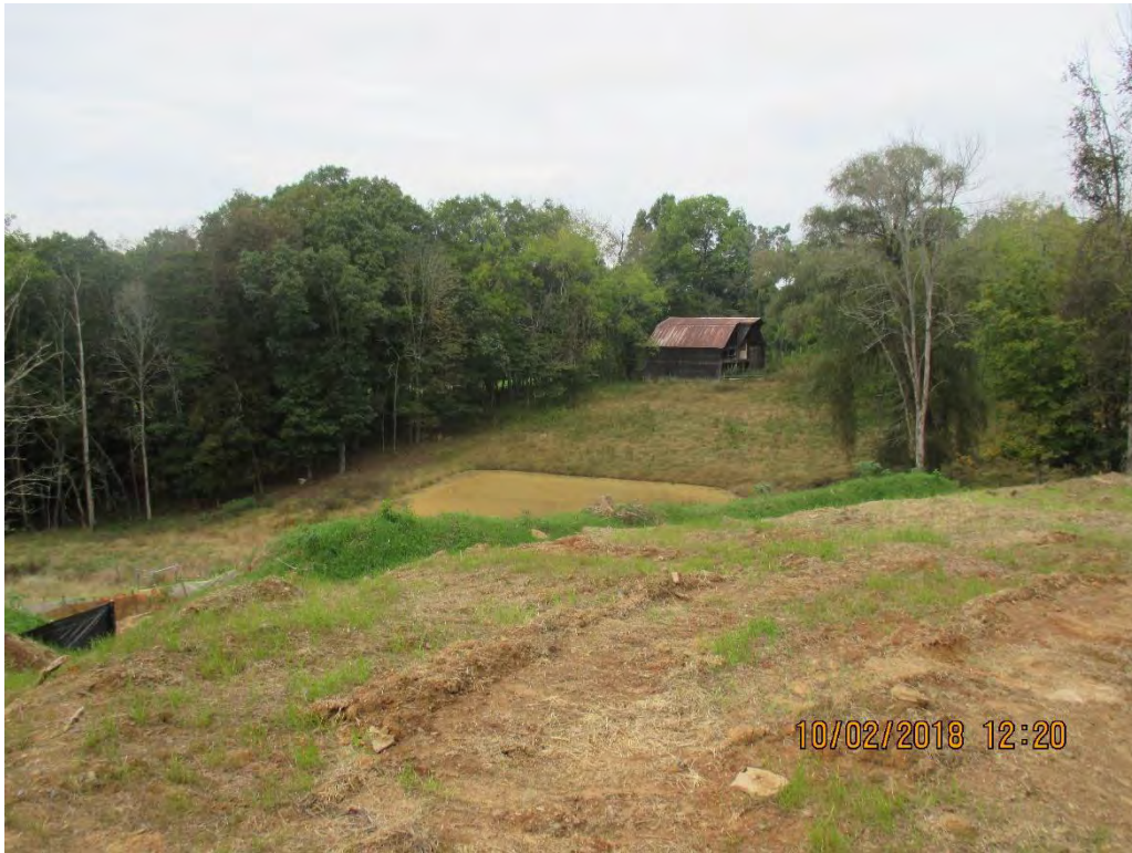
Pond (P-D1) impacted by visible settleable solids.
