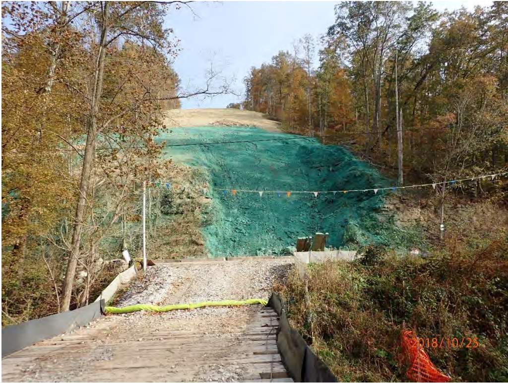
North Fork Road Crossing. Slope has been hydroseeded.
