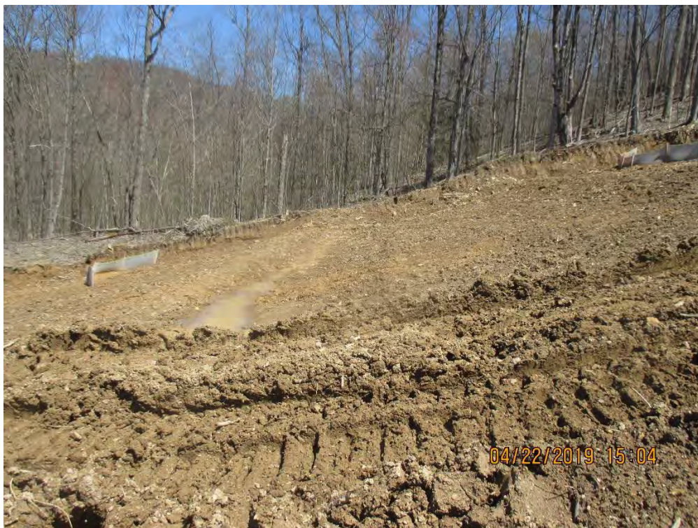
Facing towards cut slope and where waterbars terminated onto ROW.
