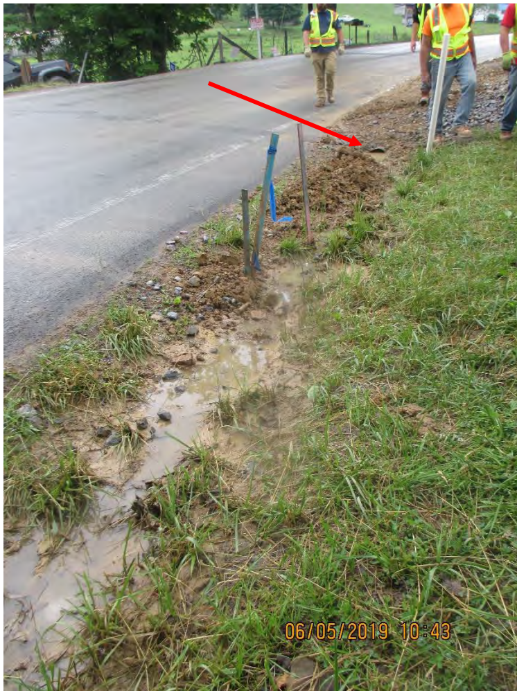
Roadside ditch and culvert outlet. Sediment laden water being conveyed downslope.
