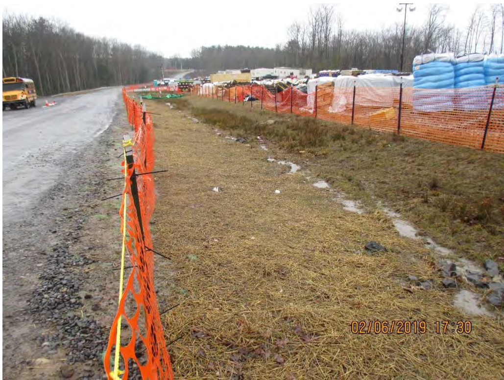
Facing West towards entrance and wetland located in ditch.
