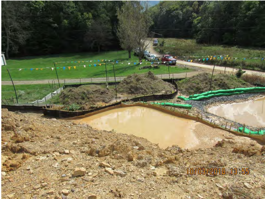
Photo 1: Sump after maintenance performed at Painter's Run Station 10270.
