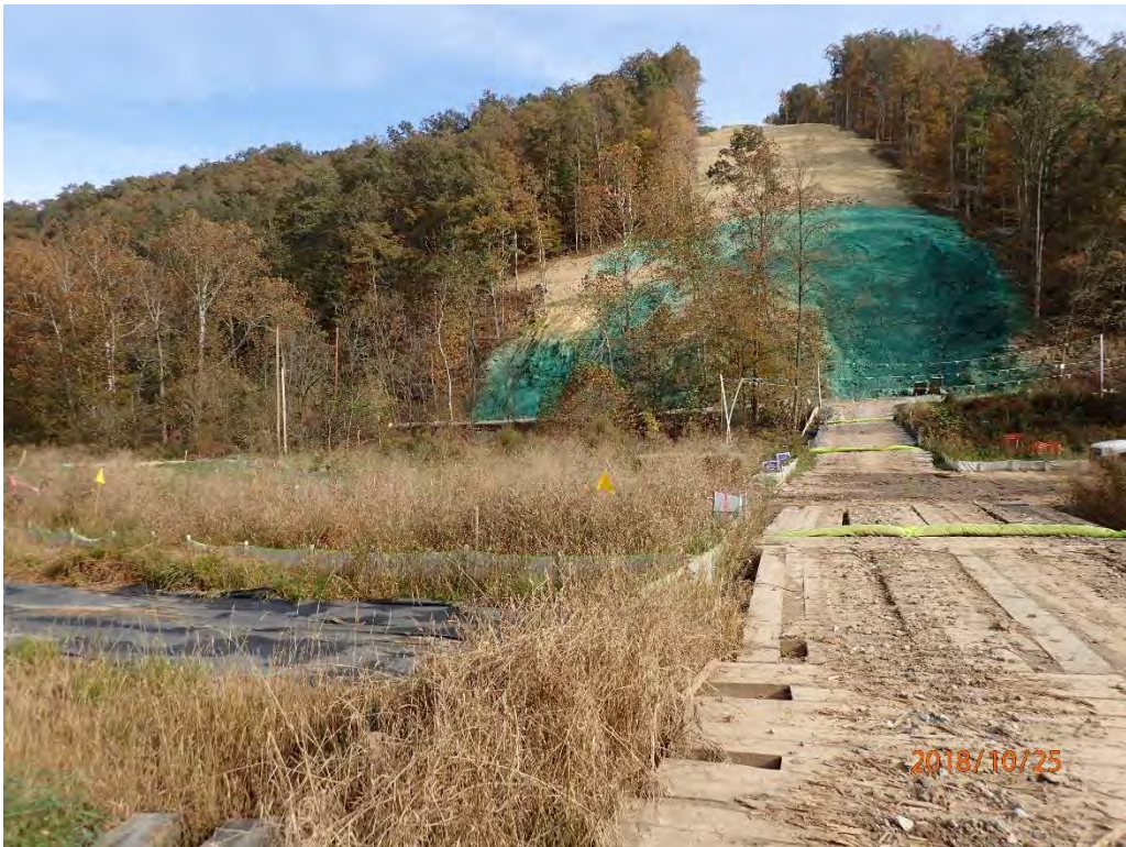
Wetland near 39.55401, -80.54555 has controls in place.
