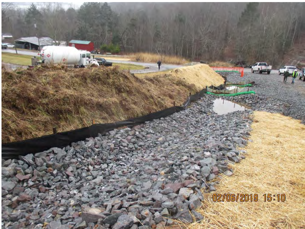
Rock lined channel facing North on West side of slope heading towards Stream S-KL29.
