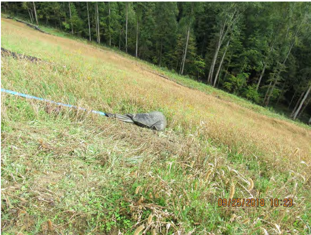
Photo 4: 1 of 3 improperly installed filter fabric bags still in use on north eastern side of site.
