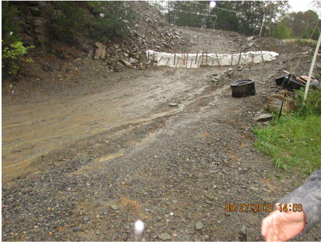
Area where SLW was leaving site and being intercepted by road side ditch along Route 122.
