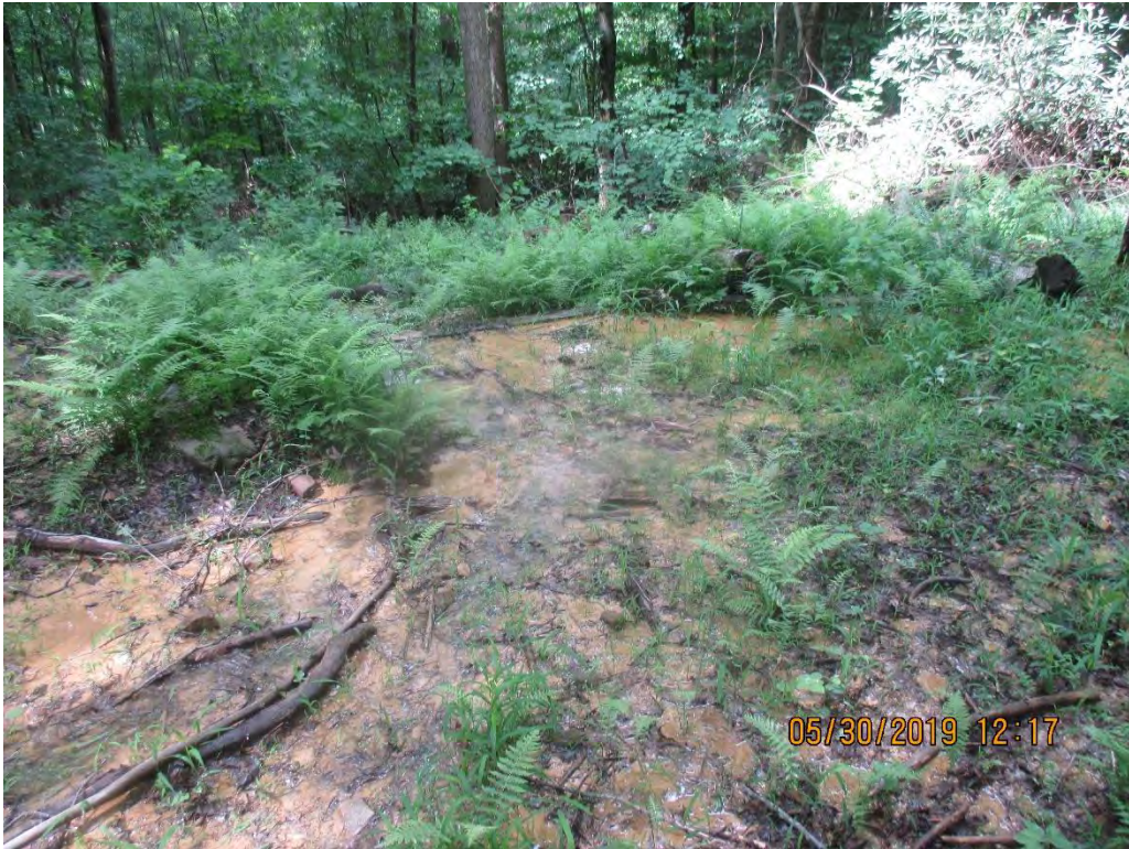
SLW and sediment deposits observed past controls and LOD near station No. 6510+40 approximately 200 feet past LOD.
