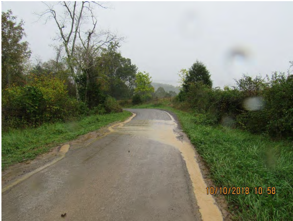
Photo 3: AR 210 sediment laden water crossing county road- down gradient view.
