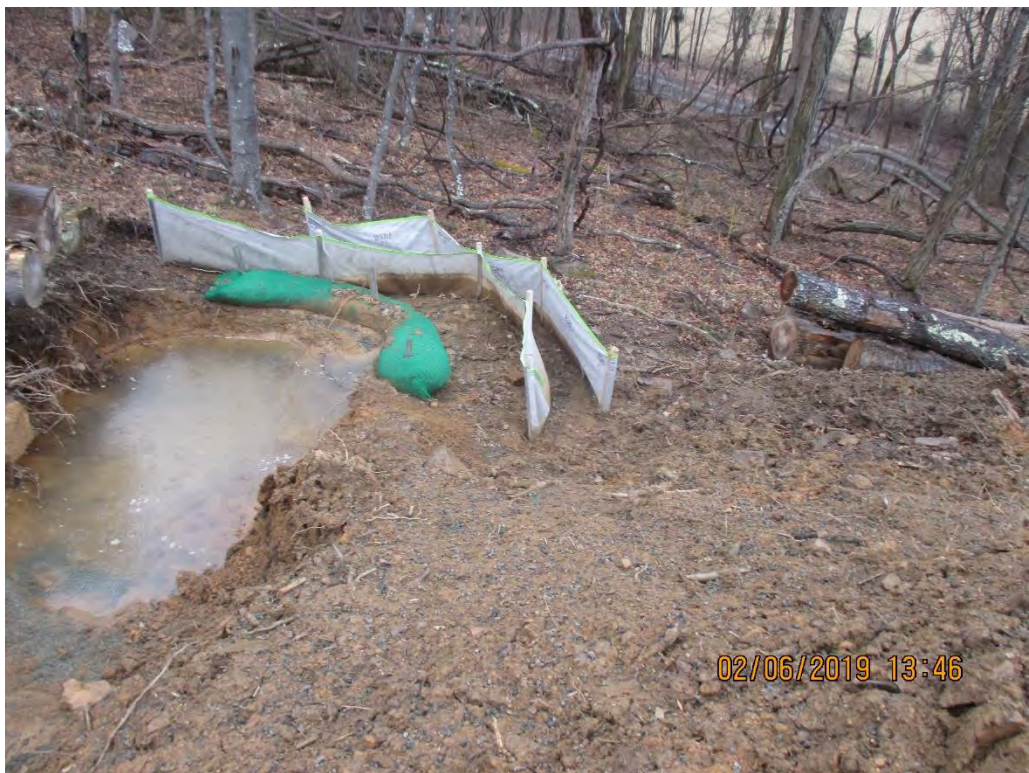
Waterbar outlet at station number 8816+00.
