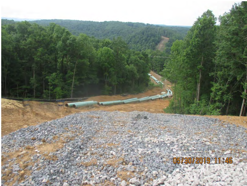
Construction entrance at Deepwell road crossing facing South at station No. 6504+20.
