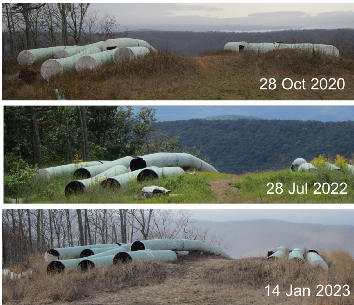
Figure 21. Photos of pipes in the Jefferson National Forest adjacent to the Forest Service’s Brush Mountain Road on three dates. Photos were taken from the road looking northwest. Visual observation provides no evidence of any maintenance over this period; while the sole evident protective measure applied originally, fabric cappings, has fallen into and remained in disrepair. Graffiti is visible on pipe near the center of 14 Jan 2023 photo, further indicating lack of pipe maintenance.
