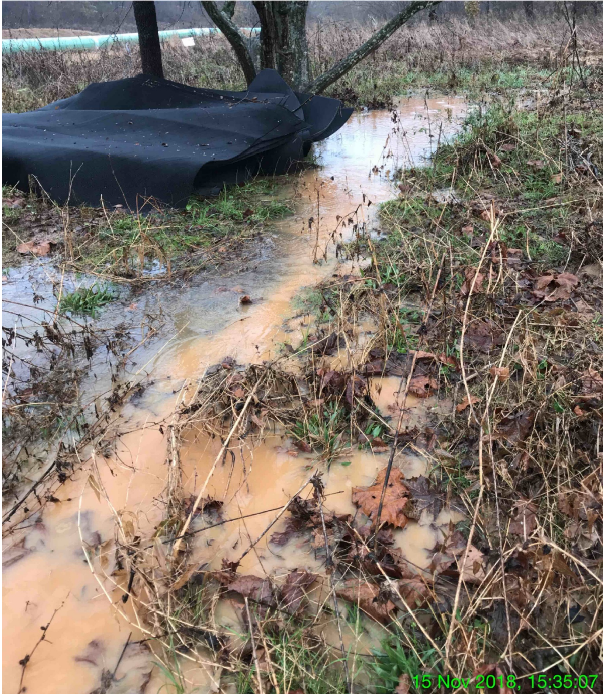
EXHIBIT B – Sediment-laden stormwater that was flowing out the gusher on the creek bank when the gusher was discovered on November 15, 2018. The black matting against the tree washed off the corridor and is a point of reference in these photos.
