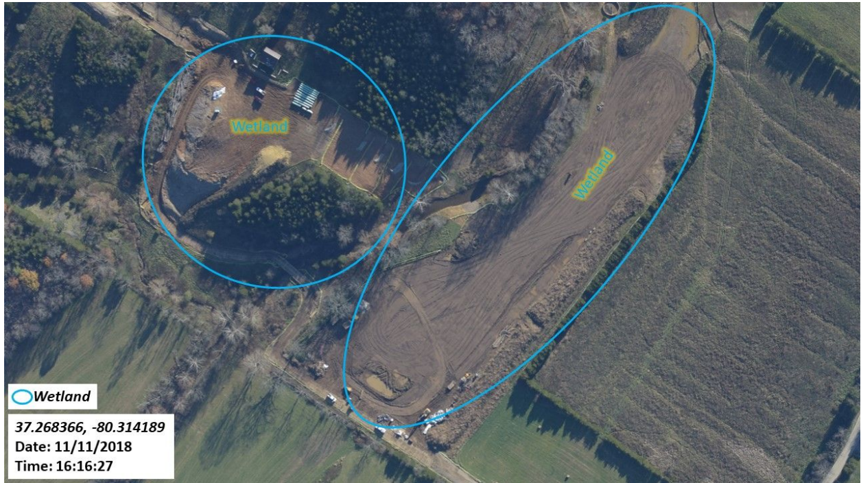
Figure 36: Wetlands area encroachment. Sediment flowing into North Fork Roanoke River.
