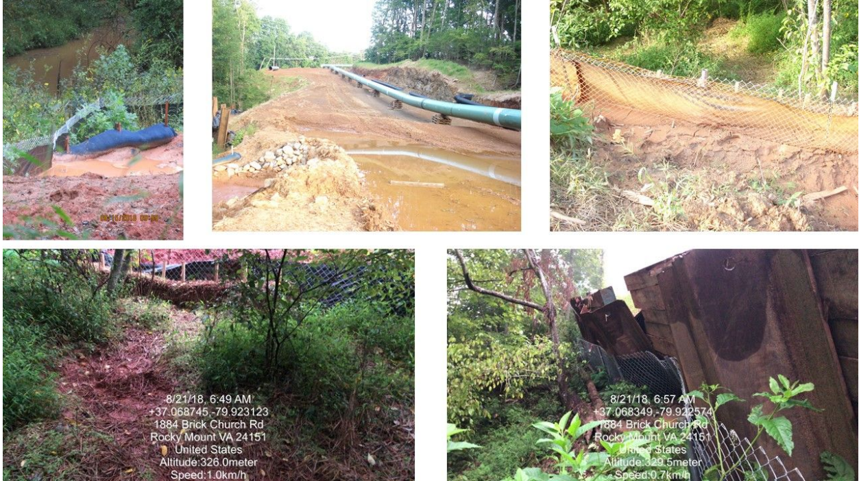
Figure 5: Ground support images. Pallets and plywood sheeting used as sediment barriers.
