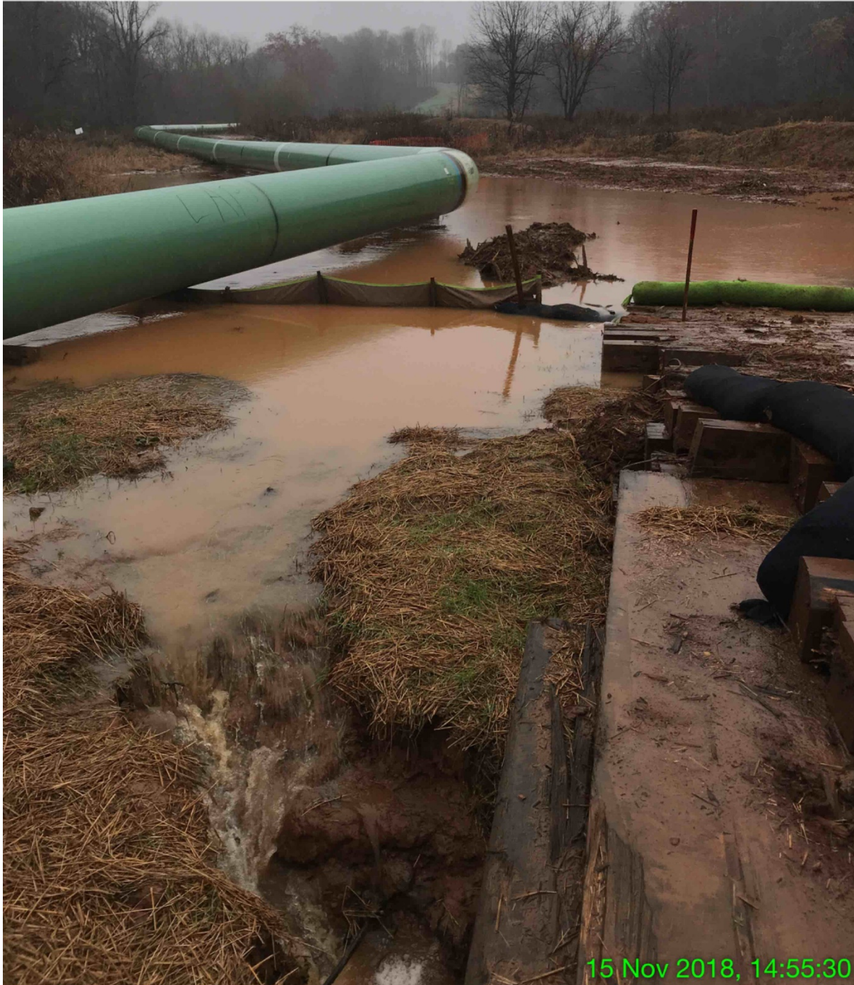
EXHIBIT I – The upstream side of the bridge over Little Creek. Muddy water flows under the bridge and out the downstream side of the bridge before entering the creek, seen in Exhibit J.
