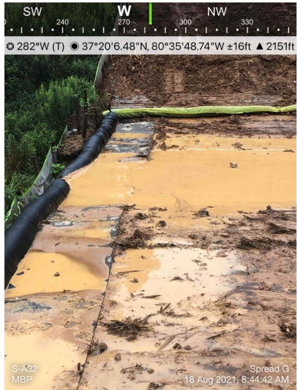
Figure 31 - Sediment deposited in UT to Doe Creek, August 18, 2021, Action Log ID 5065, Source: MBP
