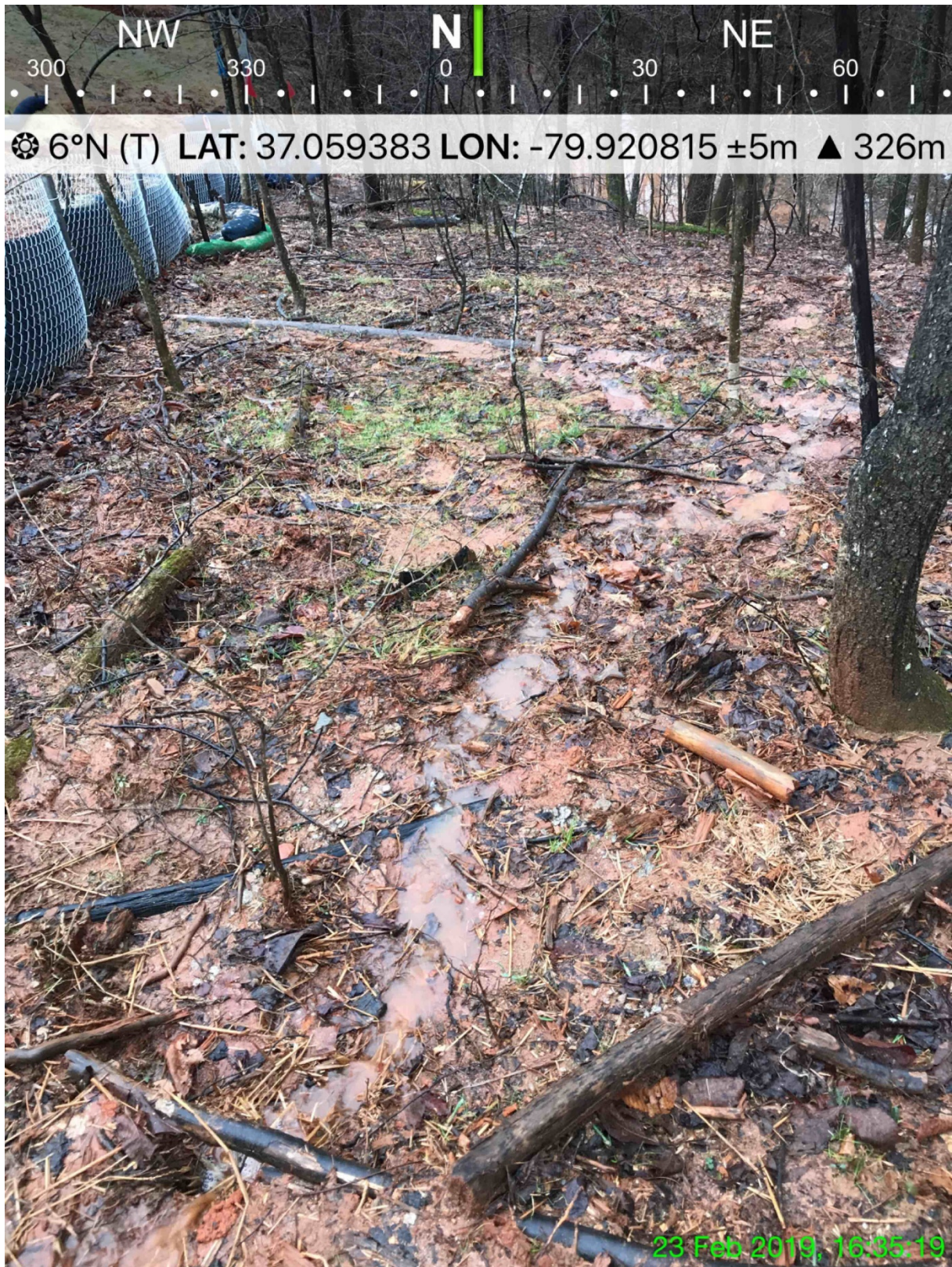
EXHIBIT R – Sediment-laden runoff has flowed from the construction corridor.
