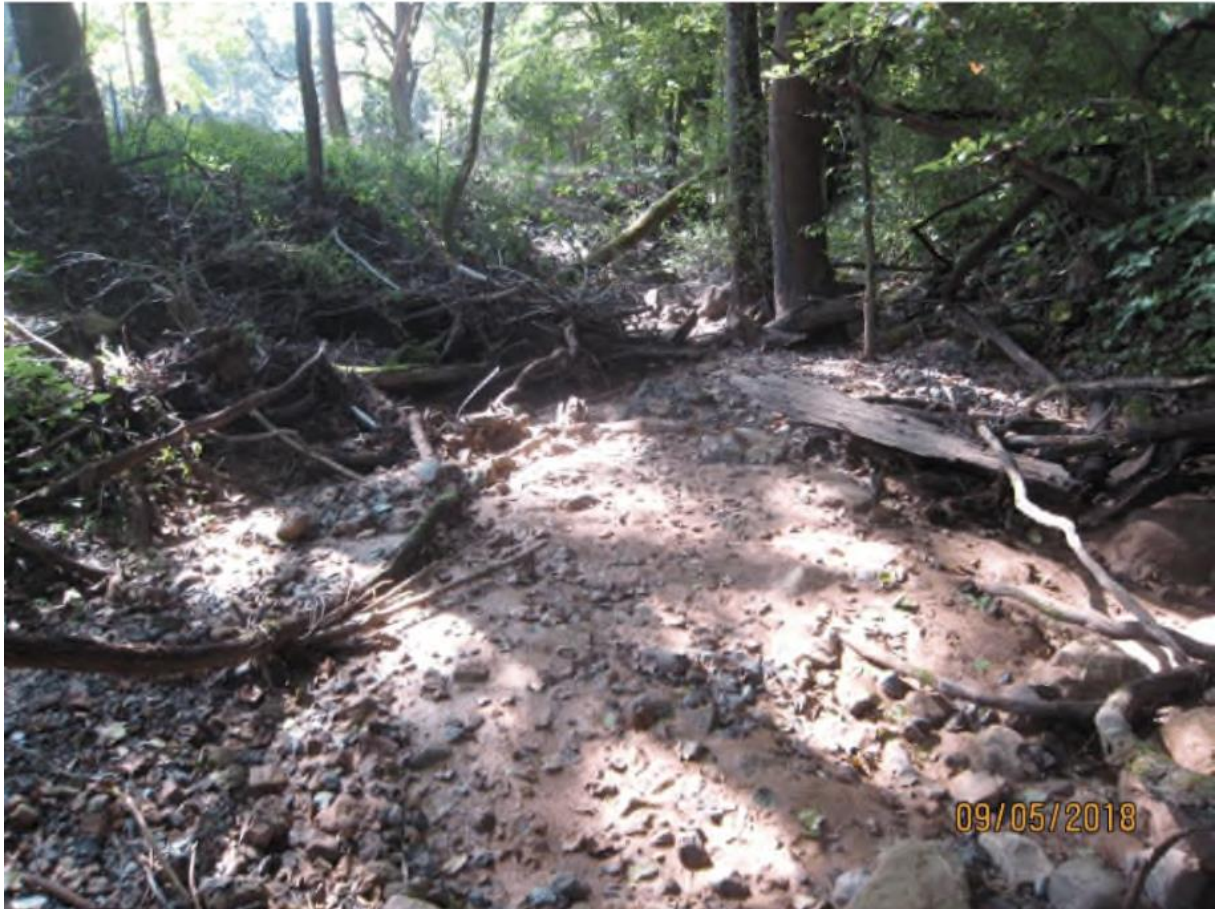
Figure 34 - Sediment deposited in Kimballton Branch, September 5, 2018, VWP inspection report, Spread G, Source: DEQ [Approx. 630 linear feet of Kimballton Branch stream channel impacted by sedimentation. Deposits up to 9 inches depth. Report indicates that aquatic life movement substantially disrupted.]
