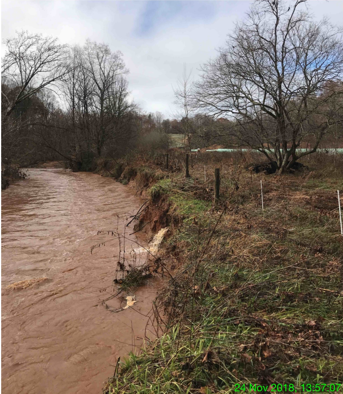
EXHIBIT C – Water gushing out of bank of Little Creek. Note the location of the cattle fence on the creek bank. Black matting against the tree and pipe on ground in background.
