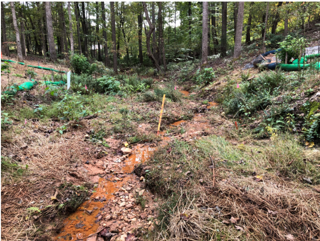
Photo 2: View downstream from bridge in Photo 1
