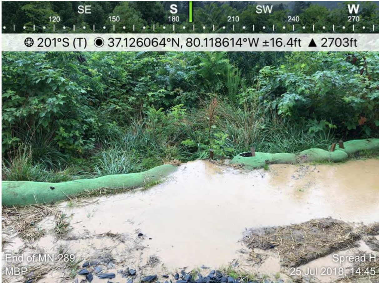
Figure 46 - Sediment-laden water overtopping perimeter control, July 25, 2018, Action Log ID 458, Source: MBP [an additional compost filter sock was added 10 days after this situation was observed]
