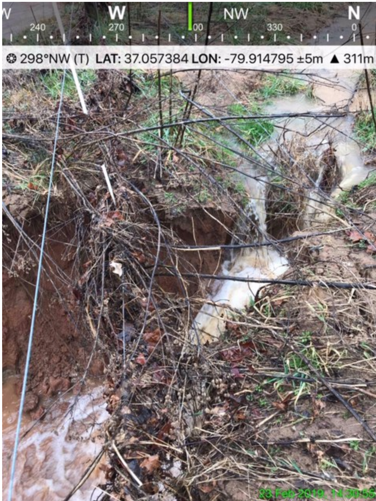
EXHIBIT F – A close-up view of the gusher eroding the creek bank on February 23, 2019. Notice the fence wire.
