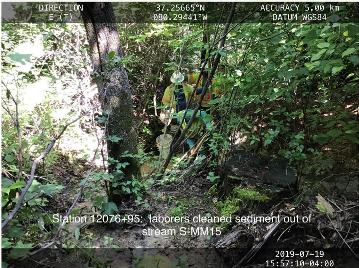
Figure 38 - Sediment deposited in UT Flatwoods Branch, July 19, 2019, Action Item Log ID 3248, Source: MBP [This is an example of what inspectors often term "remediation" through physical removal of sediments from the stream, using shovels and buckets.]
