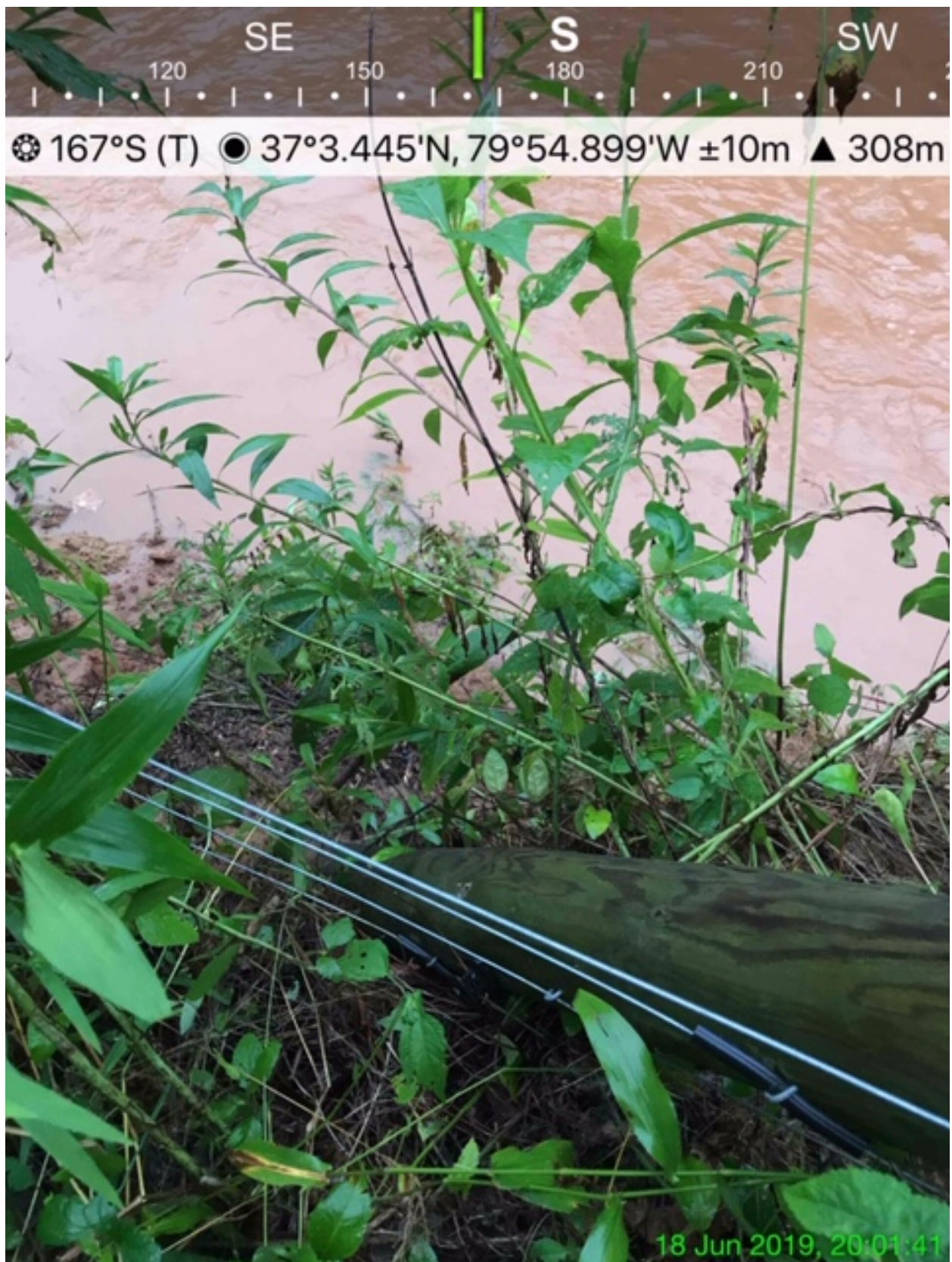
Exhibit RR – By June 18, 2019, the creek bank has eroded away from a fencepost that was at least six feet from the creek bank before construction started.
