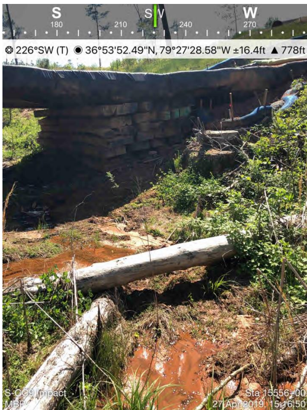
Figure 48 - Sediment deposited in UT to Cherrystone Creek, Action Item ID 2646, Source: MBP
