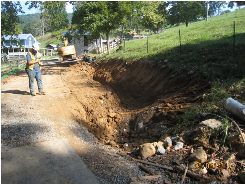
Photo 2: Access Road construction/maintenance near Photo 1 Orientation: Upslope
