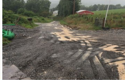
Ineffective gravel placement – now protecting stream crossing to left, but sediment is being channeled to the right side of the road into a recently dug ditch to move it offsite. No BMPs in place here to reduce sediment load within the ditch
