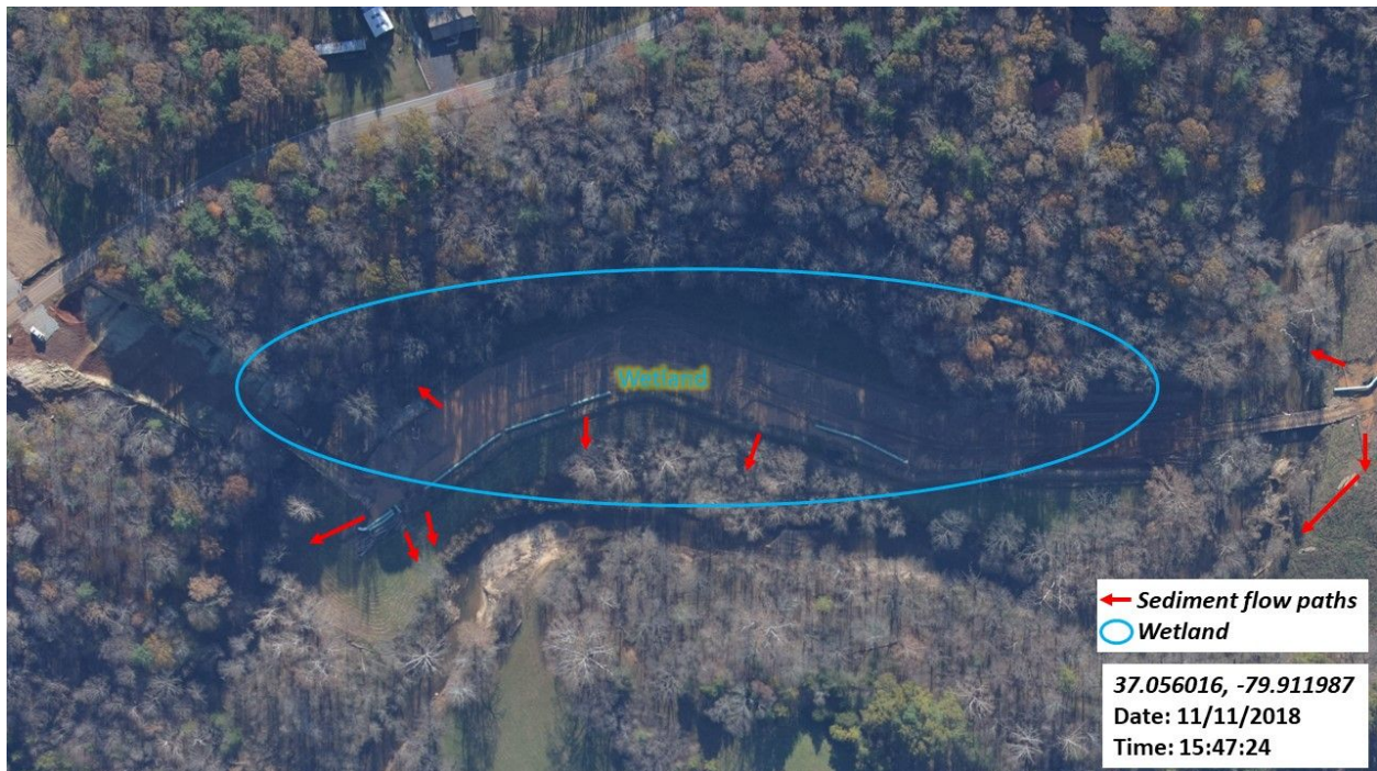
Figure 25: Sediment flowing off right of way into adjacent stream. Sediment deposits may be seen along stream.
