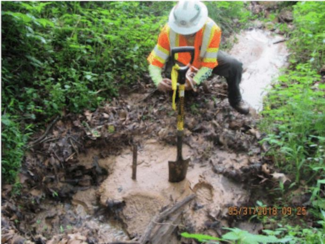
Figure 9 - Sediment deposited in UT to Blackwater River, May 31, 2018, DEQ VWP inspection report, Source: DEQ [sediment covered approx. 1,110 linear feet of streambed, up to 7 inches deep]
