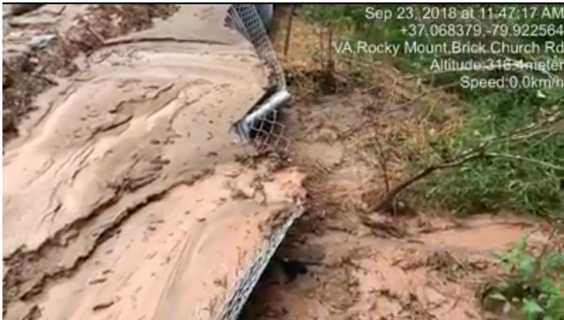
Figure 39 - Sediment deposits off ROW, at UT to Teels Creek, September 23, 2018, Source: citizen monitor
