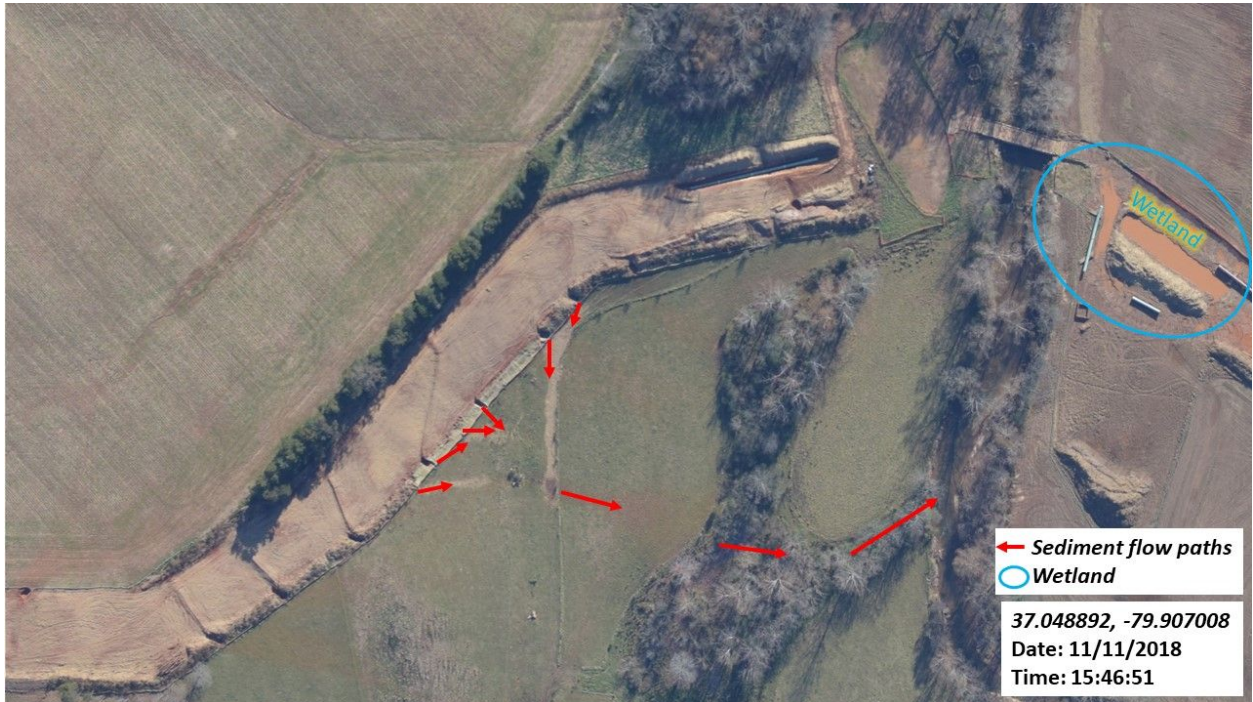
Figure 22: Sediment flowing into adjacent fields and drainage channels flowing to stream. Sediment ponding in delineated wetlands.
