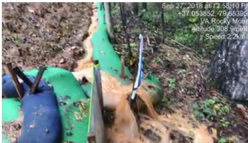
Figures 13 - 15 - September 27, 2018 Sediment-laden water overflowing compost filter socks and leaving the MVP ROW, several hundred feet upslope of the Blackwater River. Taken from a video accessible at Virginia Pipeline Violations Facebook page
