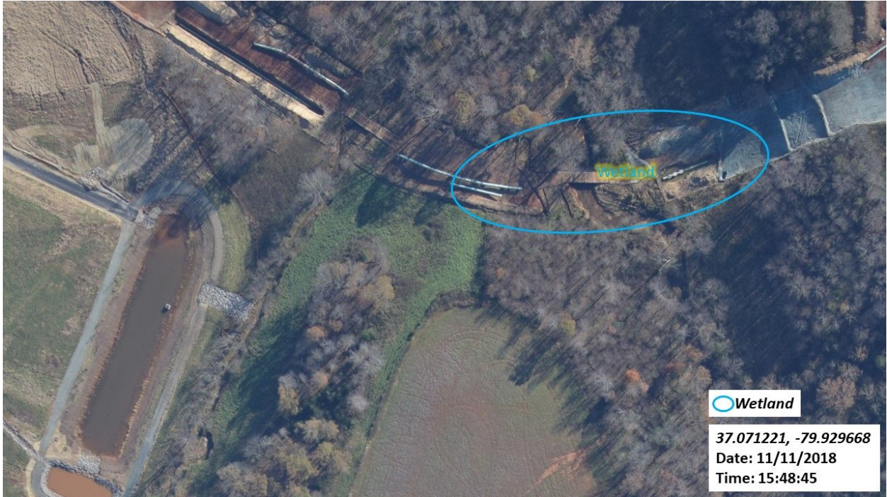
Figure 28: Wetlands and stream show evidence of sediment contamination.
