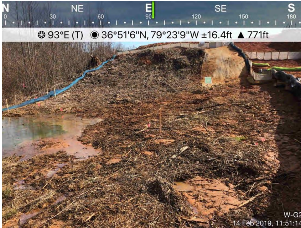
Figure 3 - Sediment deposited in wetland W-G2, adjacent to Little Cherrystone Cr., February 12, 2019, Action Log ID 1888, Source: MBP [deadline for removal of sediment extended "due to wet ROW conditions," removed after 10 days]
