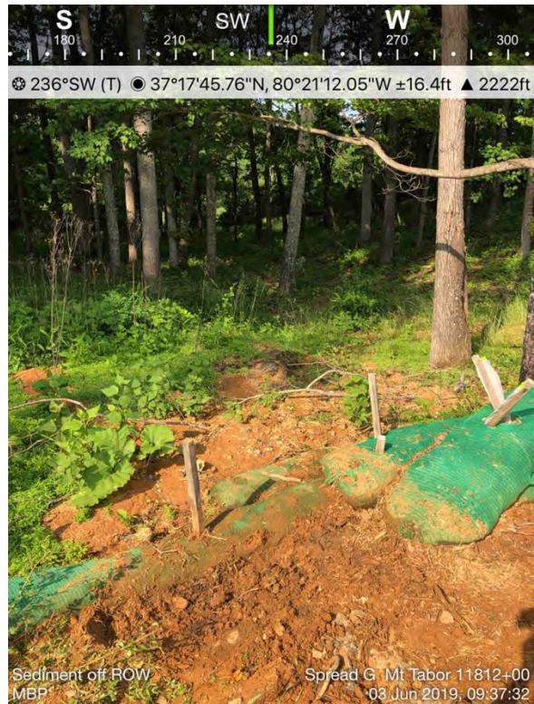
Figure 11 - Sediment deposited off ROW, June 3, 2019, Action Item ID 2844, near Dry Run, Source: MBP
