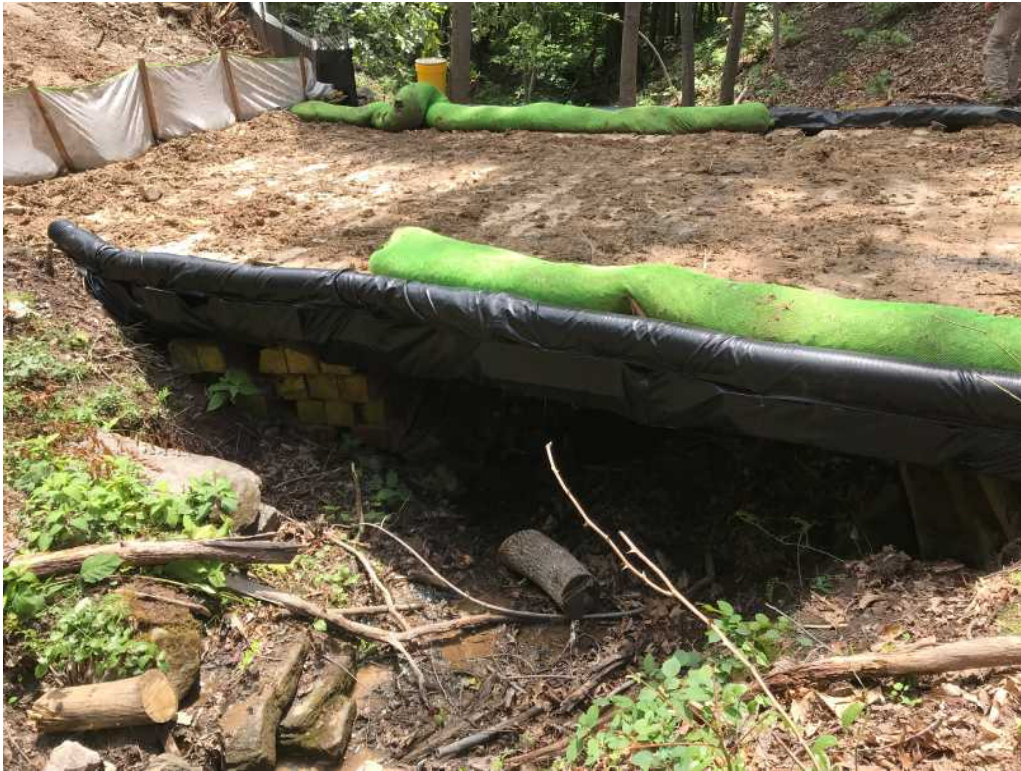
Photo 1: Sedimentation and woody debris within Stream MN-513 at bridge crossing Orientation: Downstream
