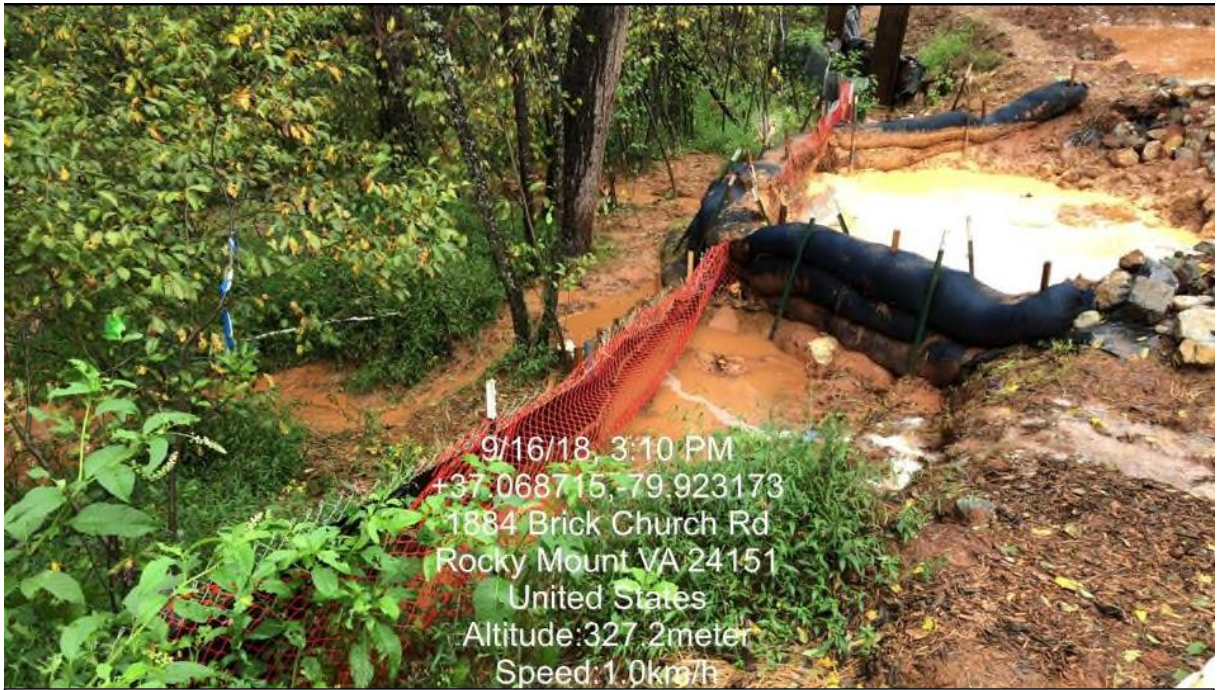
Figure 41 - Sediment deposits off ROW, at UT to Teels Creek, September 23, 2018, Source: citizen monitor.
