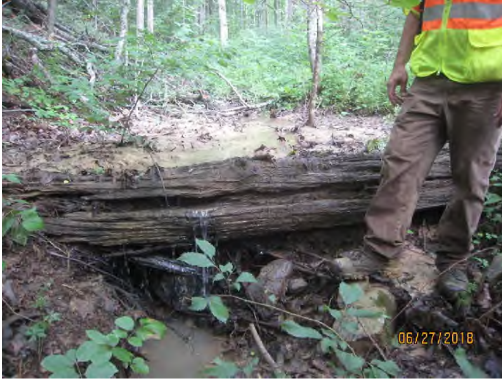
Photo 3: Sediment in stream at debris dam ~1,690' downstream of LOD; Depth = 2-7" Orientation: Upstream
