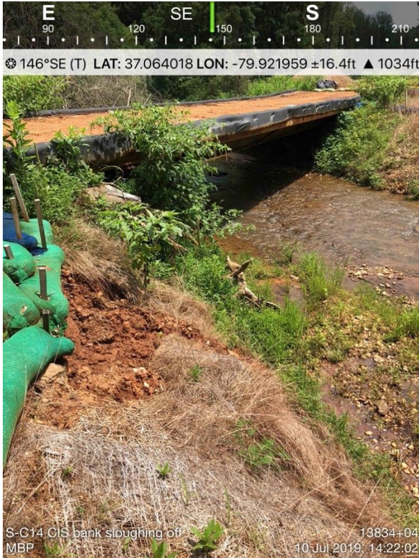
Figure 42 - Stream bank eroded at MVP site, Teels Creek, July 10, 2019, Action Log ID 3187, Source: MBP
