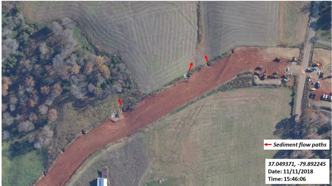
Figure 18: Sediment flowing off pipeline corridor onto adjacent properties.
