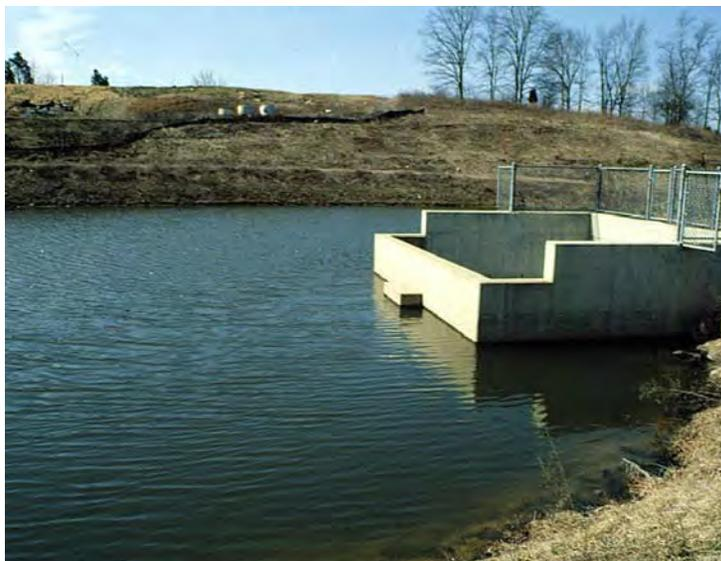
Principal Spillway multi-stage weir. Note low flow/extended detention orifice protected by “hood” draws water from approximately 18” below pool surface.
