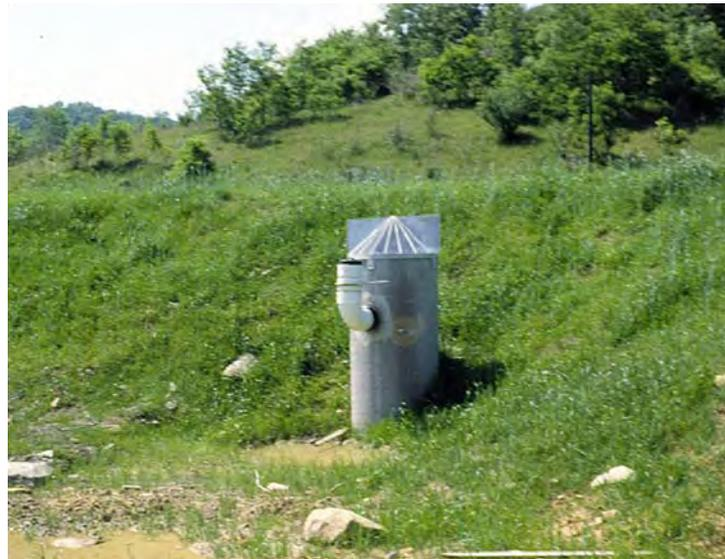
Principal Spillway multi-stage riser configured for temporary sediment basin function. Note anti-vortex plate and inclined trash rack to prevent clogging.
