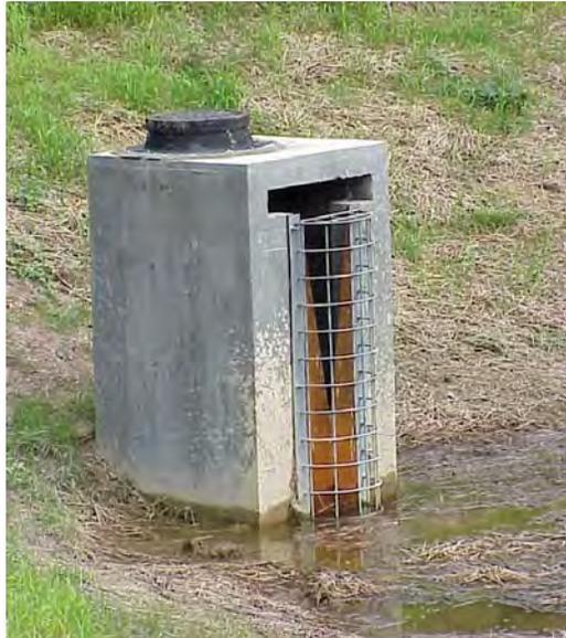
Principal Spillway multi-stage riser – “V” shaped weir protected by trash rack.
