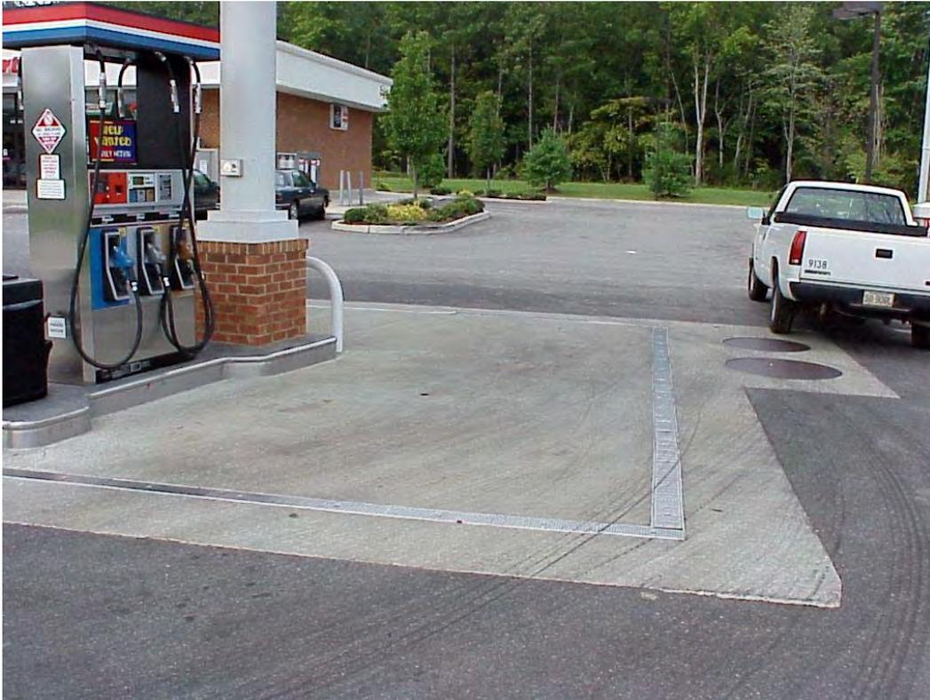
Manufactured BMP Systems. Manufactured systems can be selected to address specific pollutant sources. This trench drain surrounds fuel handling area of a service station to direct any spills or other identified petroleum based contaminants to a manufactured system designed specifically for fuel or hydrocarbon containment. Note: fuel area is under cover which serves to limit the design flow entering the system.
