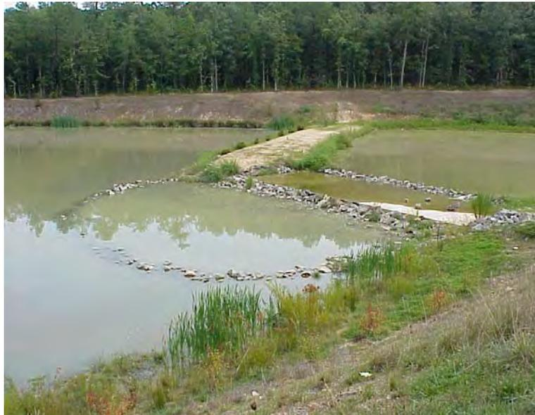
Sediment Forebay constructed with submerged rip-rap weir.
