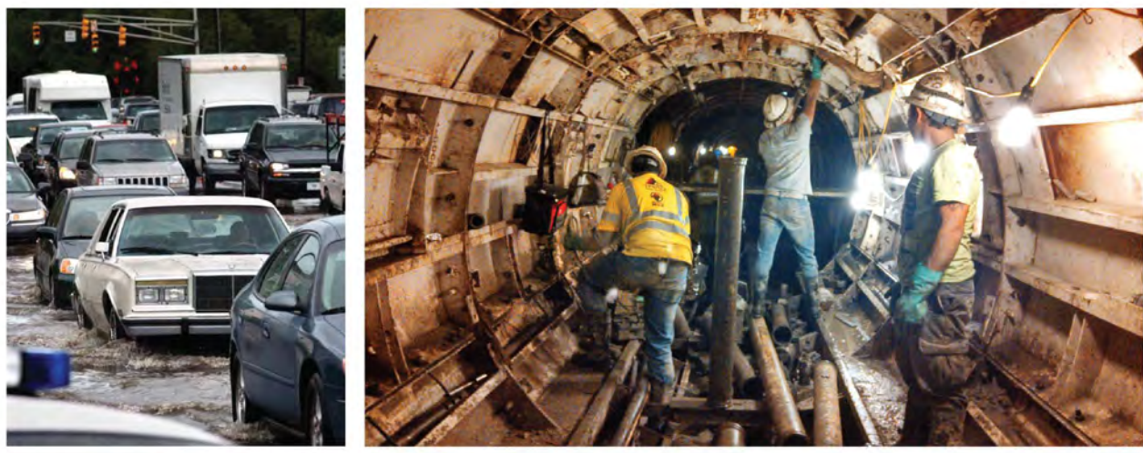
Figure 19.9: (left) U.S. Highway 17 (Septima Clark Parkway—crosstown) in Charleston, South Carolina, during a flood event. Floodwaters can get deep enough to stall vehicles. (right) Market Street drainage tunnel being constructed in Charleston, South Carolina, as part of a drainage improvement project to prevent current and future flooding. This tunnel crosses a portion of downtown Charleston 140 feet underground and is designed to rapidly convey storm water to the nearby Ashley River. Photo credit: City of Charleston 2015. 45
