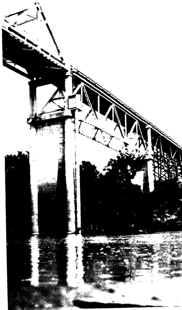
FIGURE 28.—Corrugated-steel-pipe well and wooden shelter attached to bridge pier.
