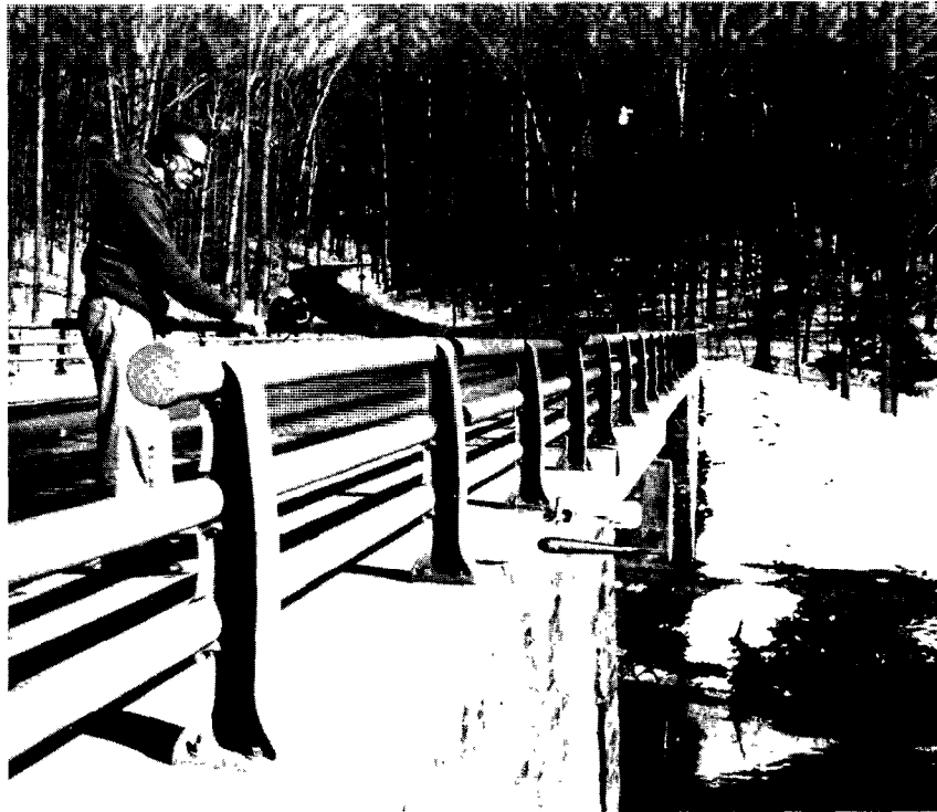
FIGURE 76.—Bridge board in use.
