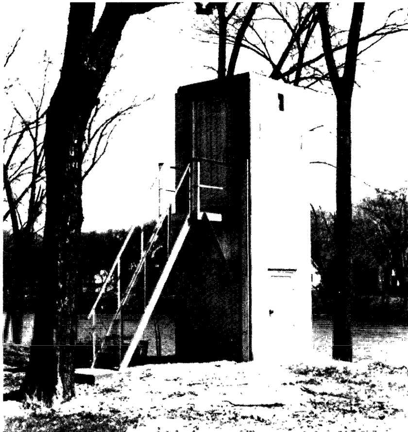
FIGURE 22.—Reinforced concrete well and shelter. (Note clean-out door.)
