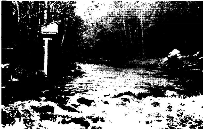
FIGURE 2.—Gage and natural control, Little Spokane River at Elk, Wash.
