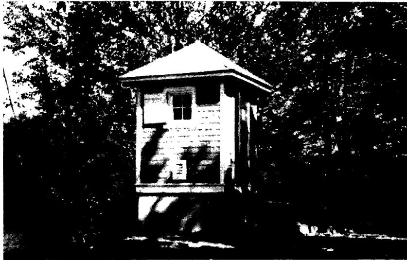
FIGURE 23.—Concrete well and wooden shelter with asphalt-shingle siding.
