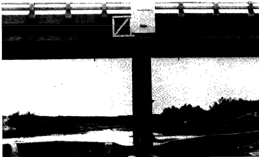
FIGURE 7.—Artificial control on Delaware River near Red Bluff, New Mex., with shallow V notch in the broad-crested weir.
