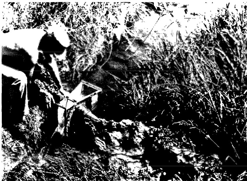
FIGURE 131.—Modified 3-in Parshall flume installed for measuring discharge.
