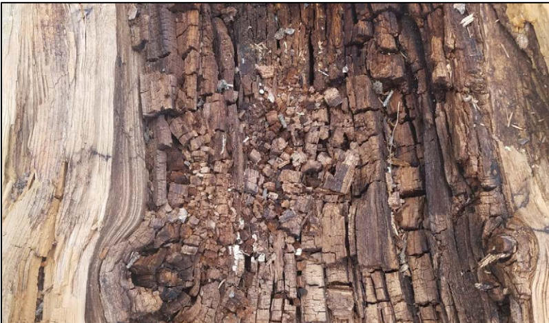
Figure 28. Cubical, crumbly brown rot.
