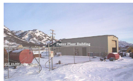
Power plant facility in Ivanoff Bay.
