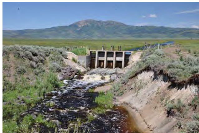
Clark's Cut water control structure at Grays Lake, southeast Idaho © FWS
