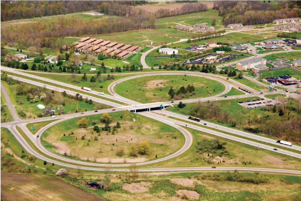
Figure 10-32. Four-Leg Interchange (Partial or Two-Quadrant Cloverleaf with Ramps before Main Structure)
