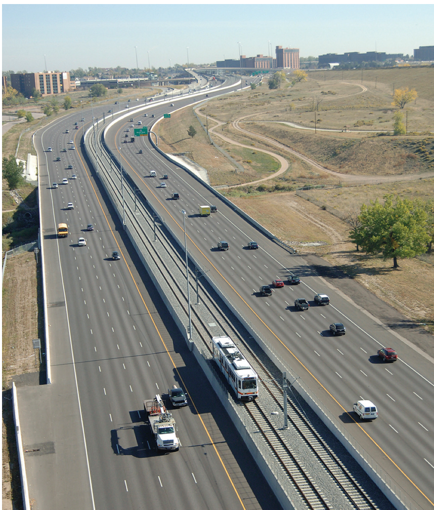
Figure 8-30. Freeway with Rail Rapid Transit in the Median
