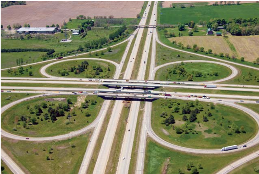
Figure 10-29. Four-Leg Interchange, Cloverleaf with Collector-Distributor Roads
