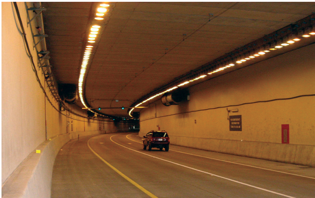
Source: Missouri DOT Figure 4-16. Interior of a Two-Lane Directional Tunnel
