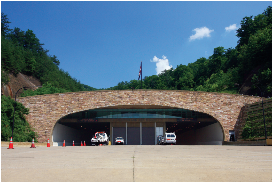
Source: Kentucky Transportation Cabinet Figure 4-15. Entrance to a Freeway Tunnel
