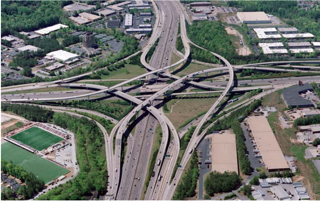
Figure 10-37. Four-Level Directional Interchange
