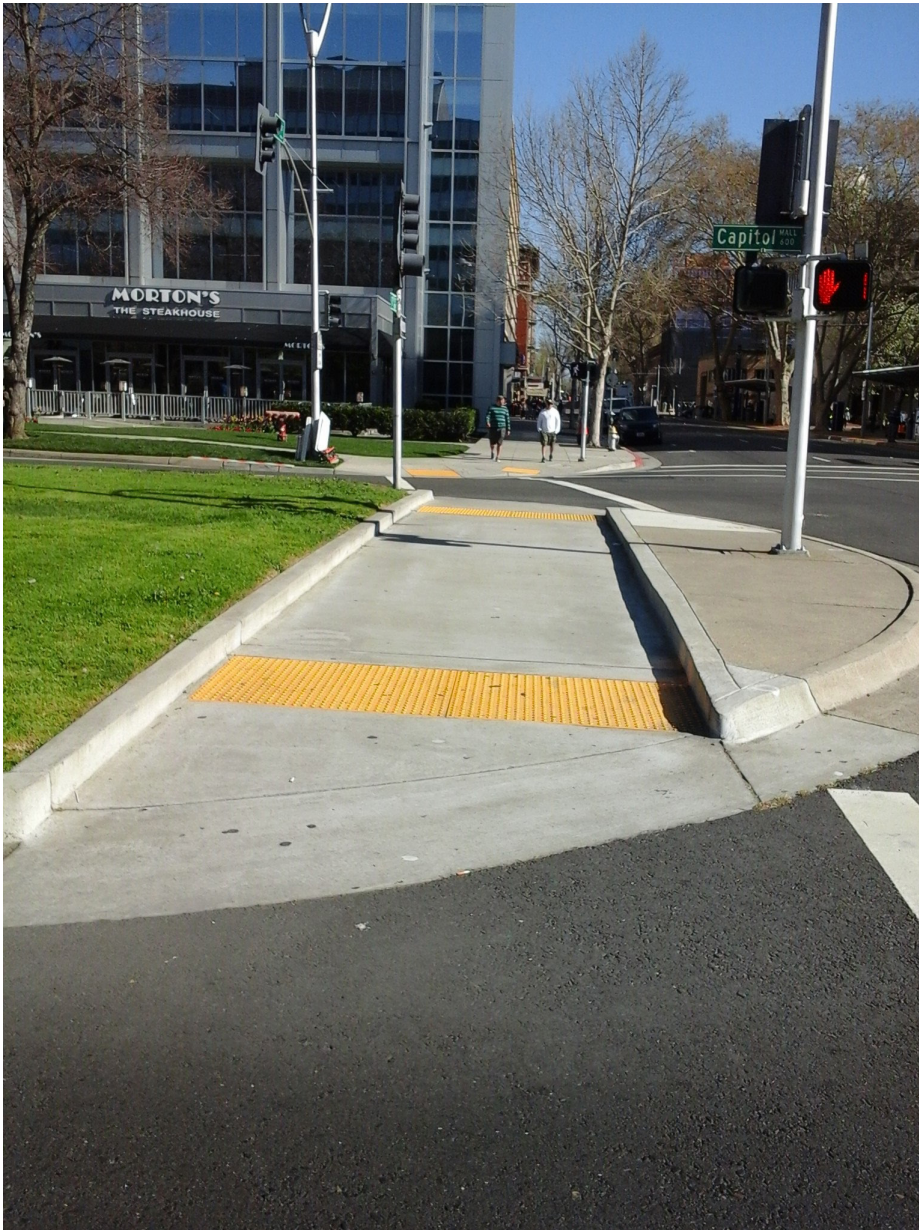
Figure 4-20. Examples of Sidewalk Curb Ramps
