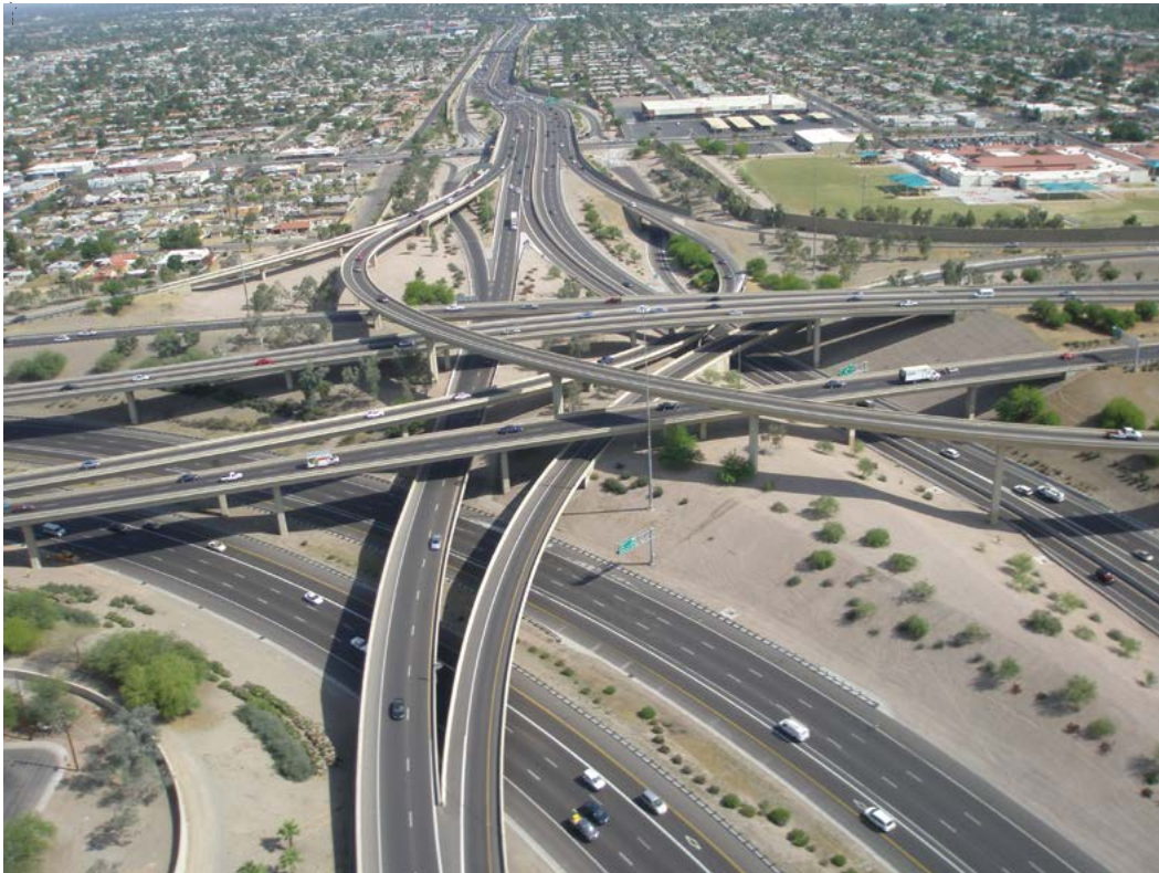
Figure 10-37. Four-Level Directional Interchange
