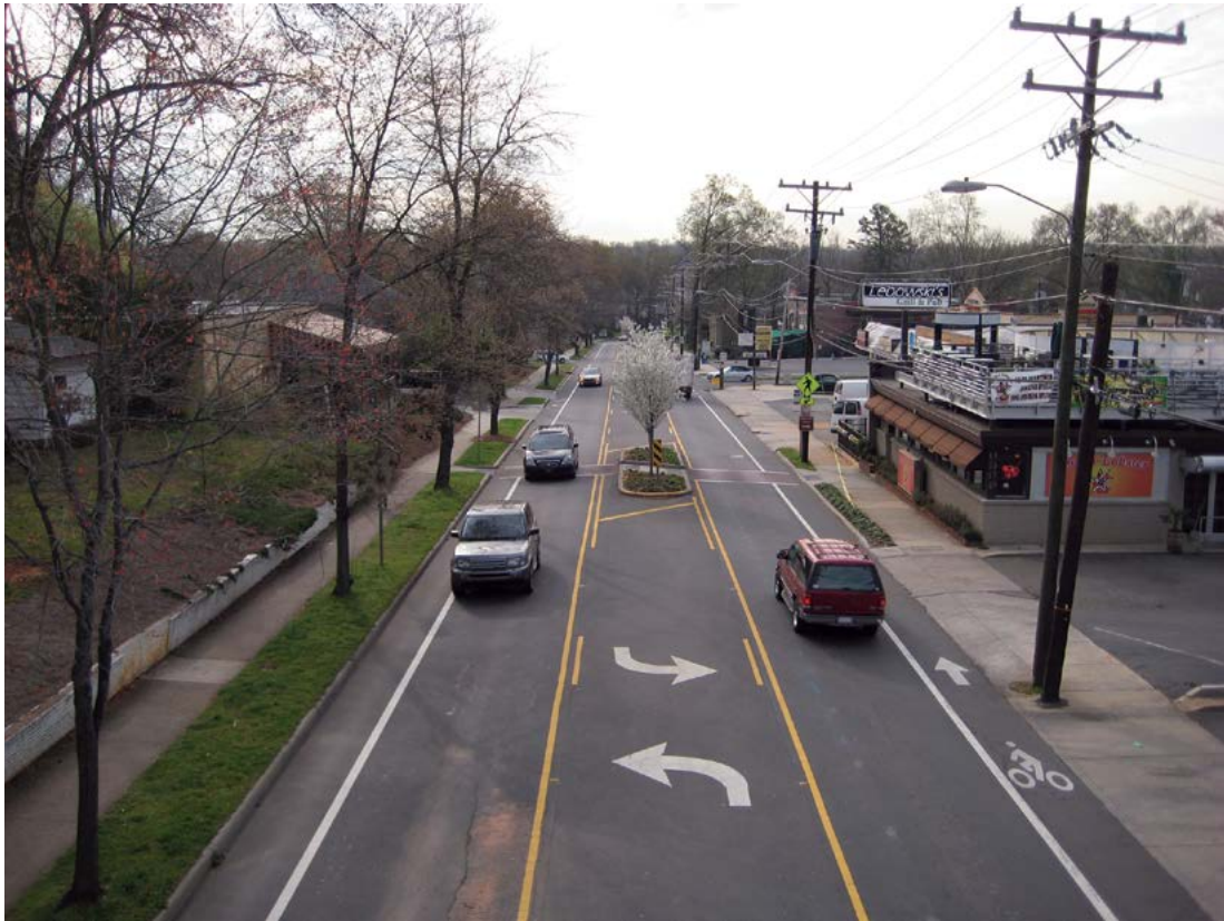
Figure 7-8. Continuous Two-Way Left-Turn Lane
