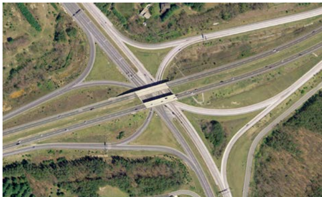
– B – Overpass SPDI
