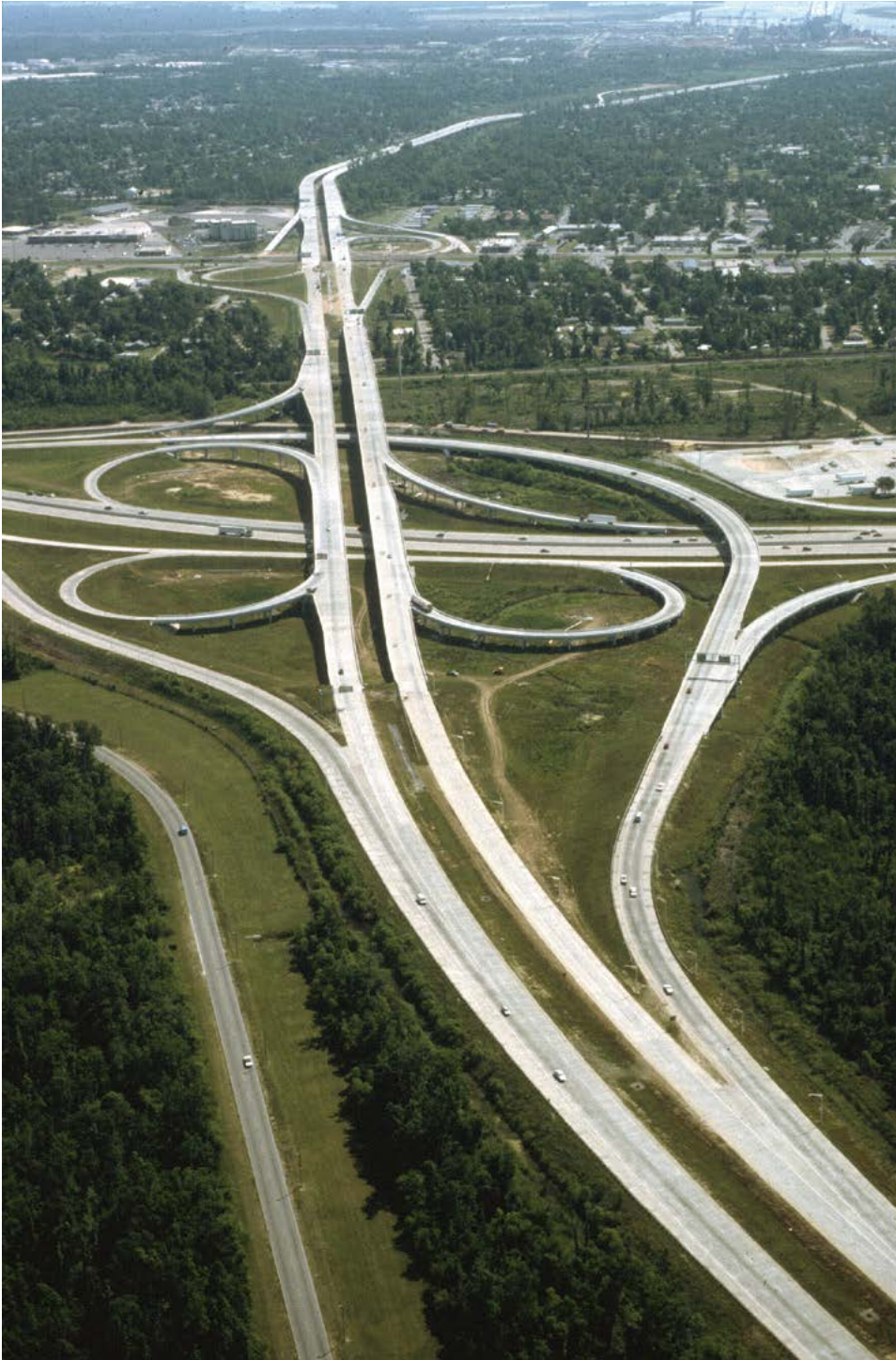
Figure 10-43. Cloverleaf Interchange with Semidirect Connection
