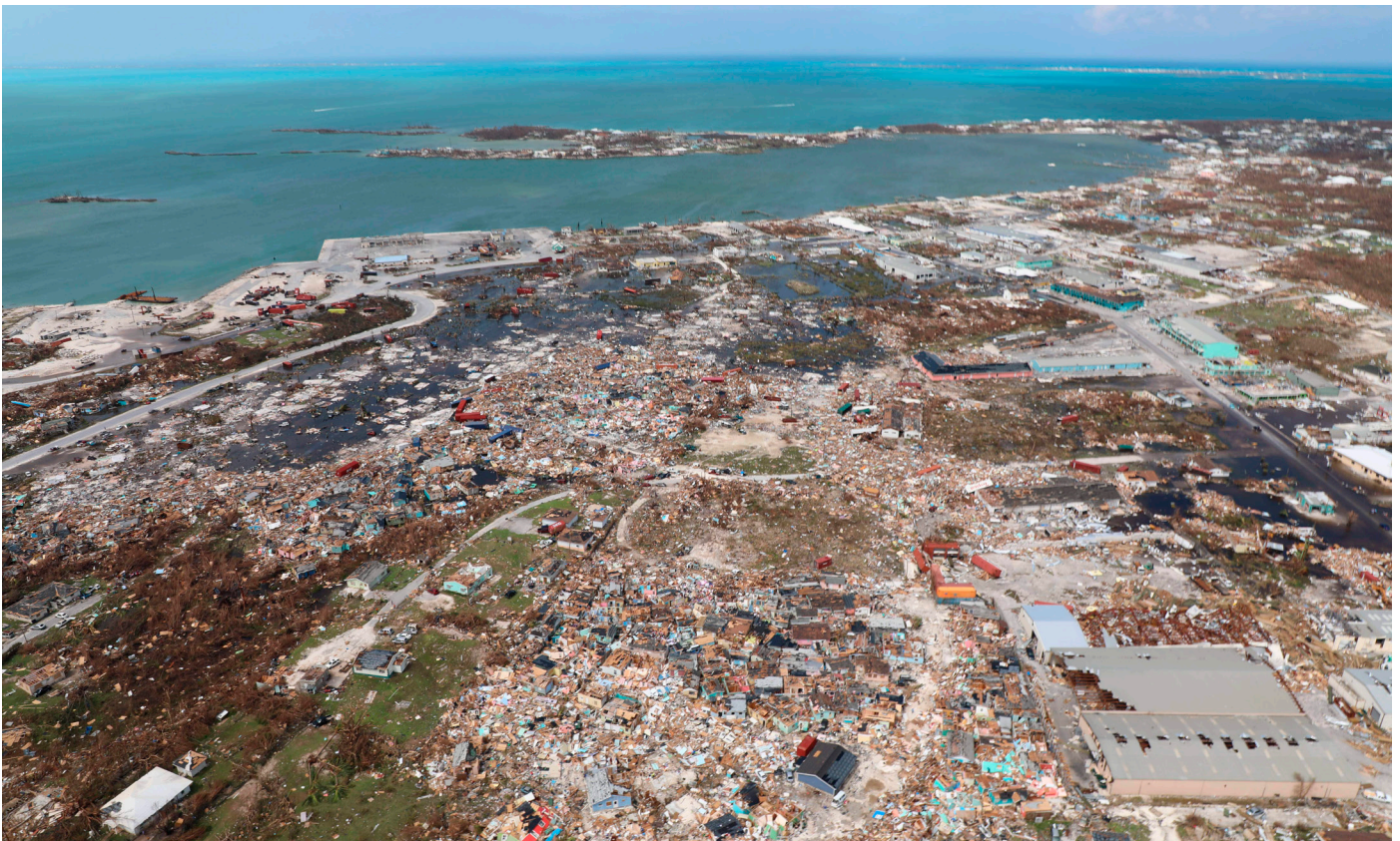
Widespread destruction caused by Hurricane Dorian is seen from the air, above Marsh Harbour, Great Abaco island, on 4 September 2019. (Gonzalo Gaudenzi/AP)
