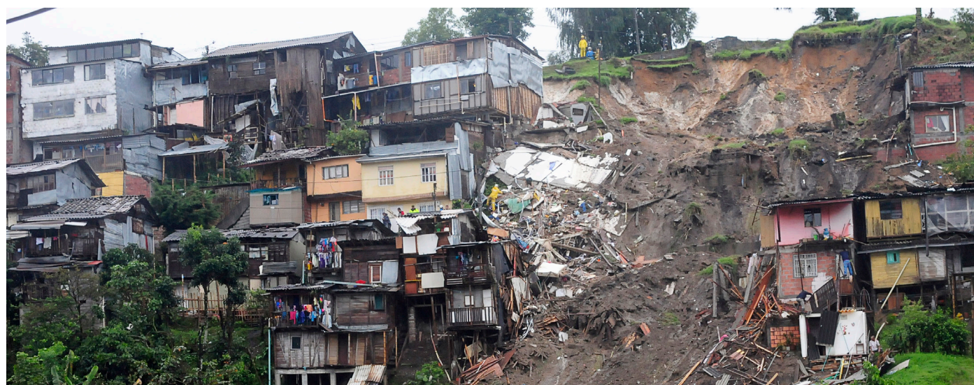
View of a landslide that destroyed several houses in Manizales, Colombia, Wednesday, 19 April 2017. At least seven people were found dead after intense rains provoked several landslides in a mountainous, coffee-growing part of Colombia. (AP Photo/Maria Luisa Garcia)
