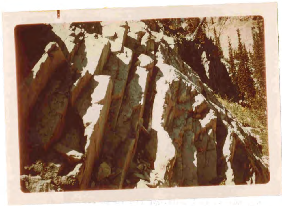
Competent bedrock with fracturing perpendicular to the slope gradient leads to the stability of the slope with disturbance.
