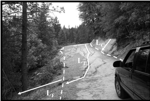
Figure 1. A picture of a reconstructed outsloped native surface road on a highly erodible, weathered granodioritic hillslope in northern California, USA. The road prism is comprised of the cutslope, travelway, and fillslope, and the arrows show the potential length of overland flow for each of these pathways. Note how the rill networks on the travelway concentrate the road surface runoff before it is discharged onto the fillslope. The extensive rilling is due to poor compaction during road reconstruction.
