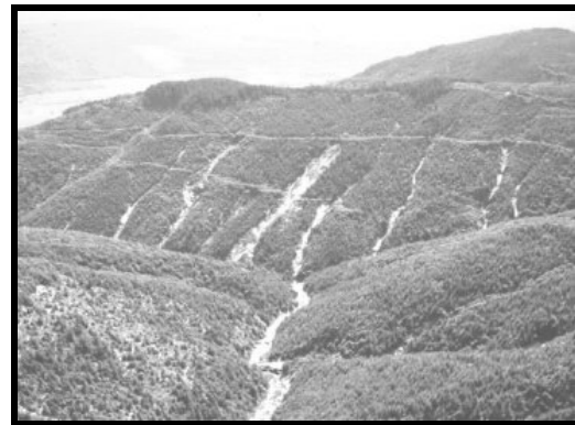
Figure 6. Road-induced debris flows in northwest Washington state, USA. The debris flows initiated in the colluvial hollows on the upper road were triggered by road runoff, and these triggered the failures at the road-stream crossings on the lower road. This sequence has been defined as a “disturbance cascade” (Wemple et al., 2001). The road was built prior to the implementation of best management practices and large fill volumes were placed within colluvial hollow and inner gorge landforms (WA DNR, 1983).
