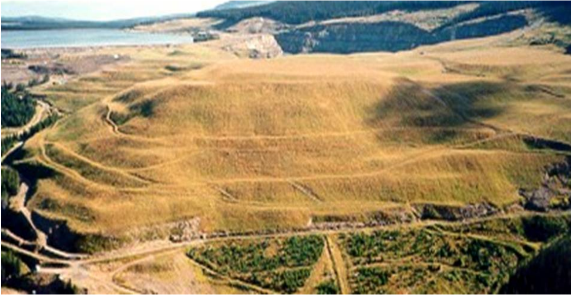
Figure 3.9 Many key properties and processes, such as weathering of mine wastes under this soil cover at the Equity Silver Mine, are difficult to measure let alone predict. (photo of Equity Silver Mine in northwest British Columbia from Mike Aziz, Goldcorp Canada Ltd.).
