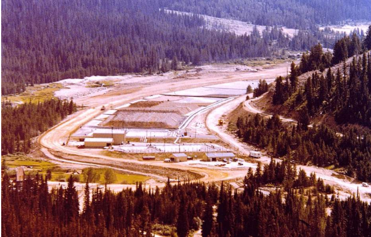
Photograph 6-3: Canadian Superior Mining (U.S.) Ltd. Heap Leach Processing Facility
