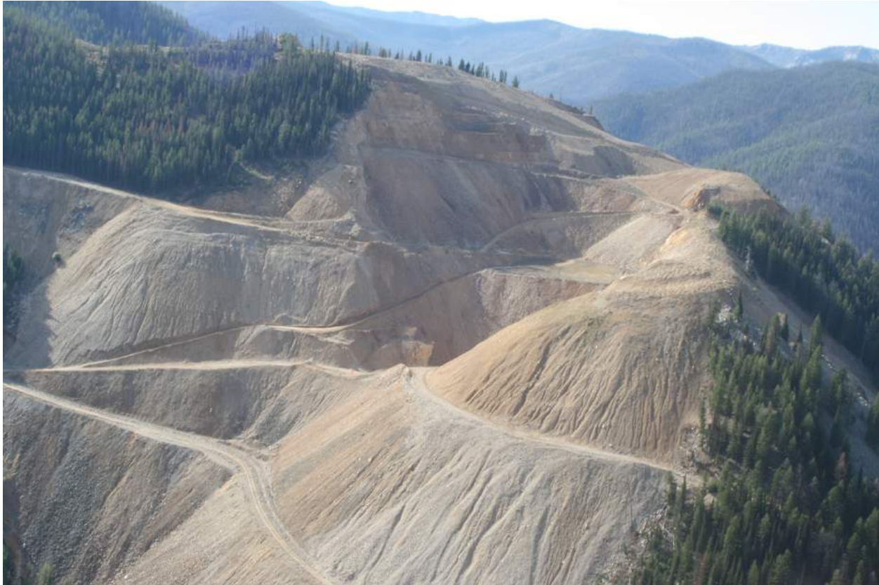
Photograph 6-4: West End Pit showing Partial Backfill
