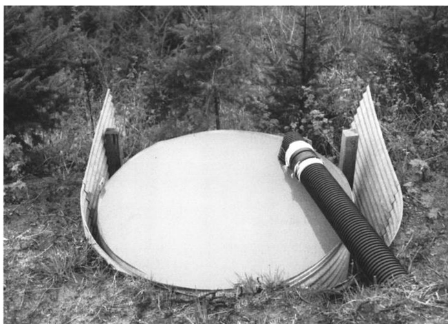
Figure 3. Photograph of sediment trap with crossdrain outlet.
