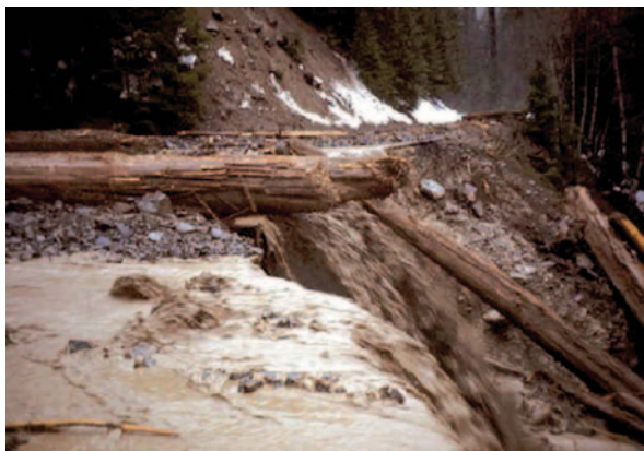
Fig. 16.9 Road in H. J. Andrews Experimental Forest rapidly eroding because of flow diversion. (Grant and Swanson 2007)
