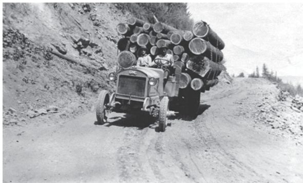
Fig. 16.7 Logging road in the 1930s. Note the lack of an inside ditch and the eroding ruts on the road surface. (Potlatch Corporation: Historical Photographs © 1999)
