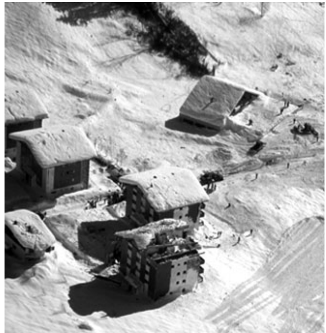
Fig. 4. Aerial picture of residential houses in Leukerbad that were damaged by a powder-snow avalanche. In the background, trees are visible that were destroyed by the avalanche.
