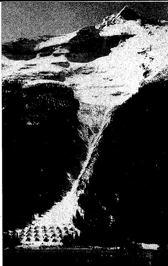
Figure 9.50. Earth mounds to retard flowing snow at the end of a runout zone. (Photo by P. Schaerer)
