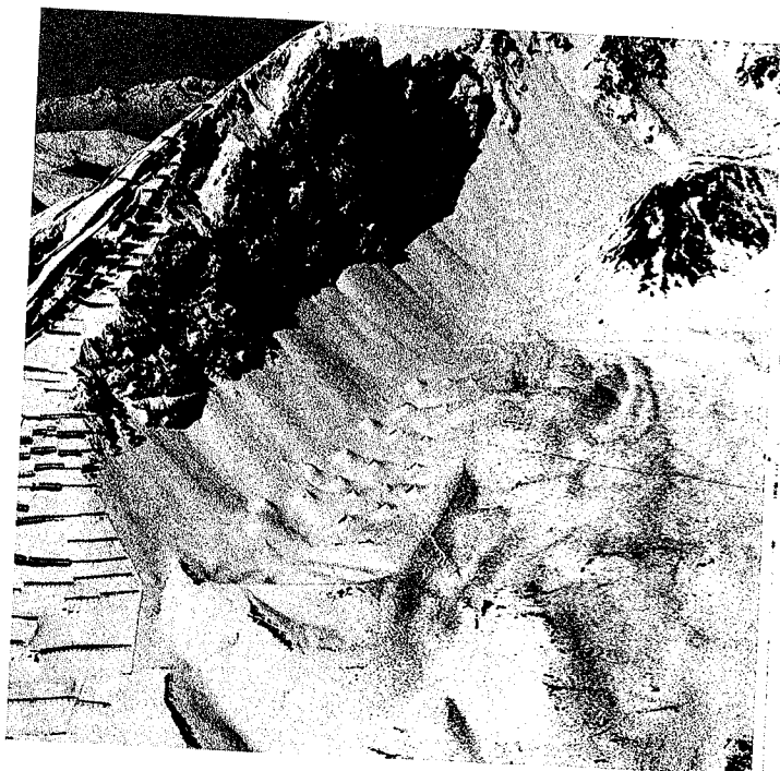
Figure 9.33. The left side shows supporting structures in avalanche starting zones. In the center of the picture, mounds and arrester dikes are visible. (Photo by E. Wengi)
