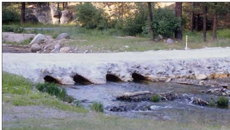
Figure 6.—A vented ford. From Keller and Sherar (2003).
