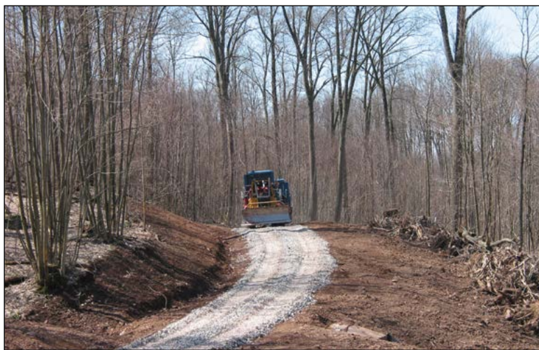
Gravel application on a new cut-and-fill forest road, and woody material from the right-of-way positioned as a windrow on the fillslope. (Photo by U.S. Forest Service, Northern Research Station.)
