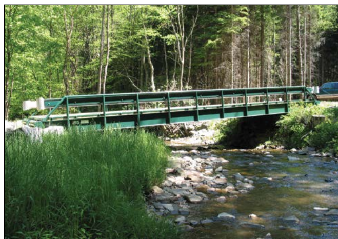
A temporary bridge installed over a perennial stream to reach a timber harvest area. (Photo by U.S. Forest Service, Northern Research Station.)
