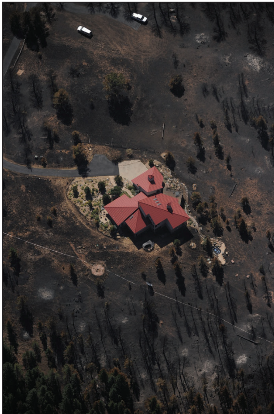
Figure 55. This is an example of a home ignition zone (HIZ) and how it reduces ignition potential within 100 feet of a home. Home construction was nonflammable or ignition resistant. Areas adjacent to the home were irrigated plantings or nonflammable materials. Firebrands landing on and around the home had few flammables to ignite. Surface fires were not eliminated within the HIZ but importantly, were restricted by the landscaping design from burning to contact the home. Trees that would produce high intensities were separated, thereby reducing the chances of canopy burning and, when not prevented, the burning canopies produced significantly less radiant heating to the home (photo: Joe Amon).
