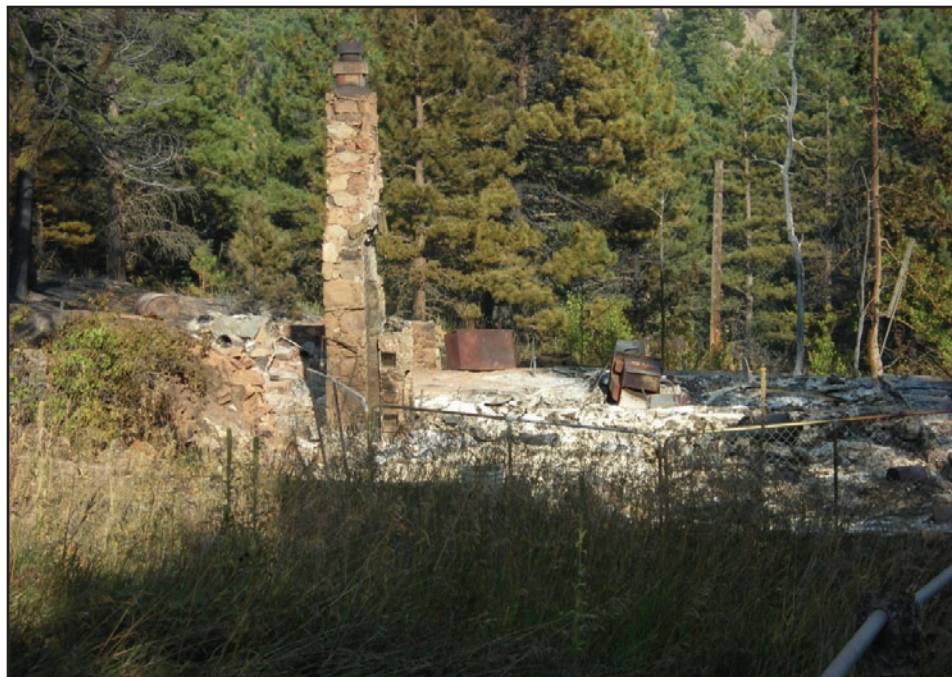
Figure 53. An example of total home destruction surrounded by unconsumed vegetation indicates the ignition was associated with a low intensity fire exposure (photo: Boulder County Sherriff Office).
