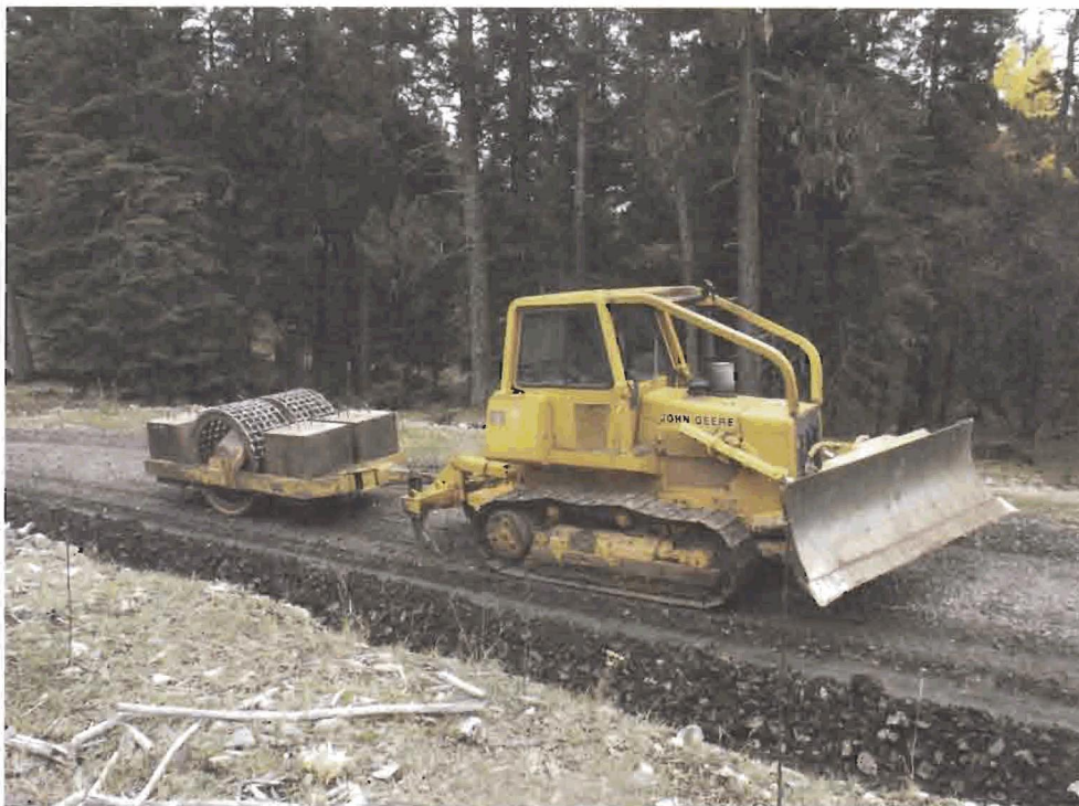
Figure A 3. Dozer and grid roller equipment used during sound testing on the Lincoln National Forest, NM, 22-23 October 2002.
