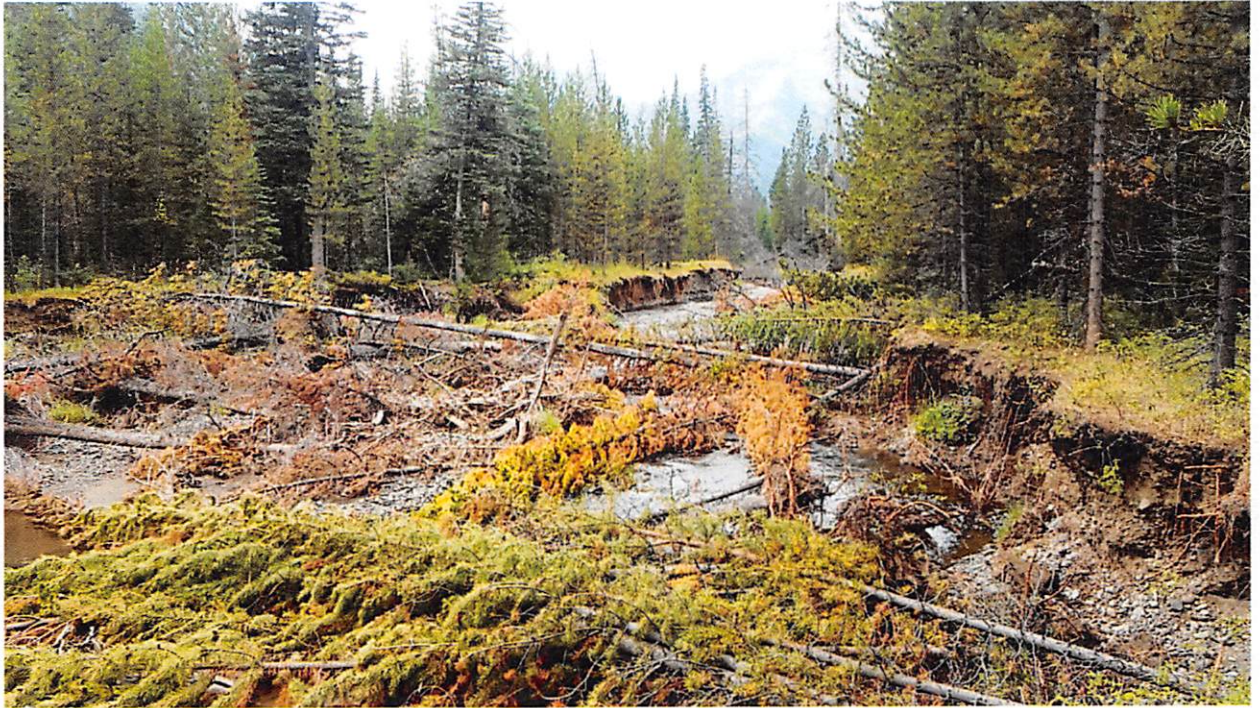
Figure 1. Erosion of FS D101.1D by Sunlight Creek. The main channel of Sunlight Creek now flows down this decommissioned, but unreclaimed access road. Photo taken August 18, 2015 at 44.662266 -109.685702.
