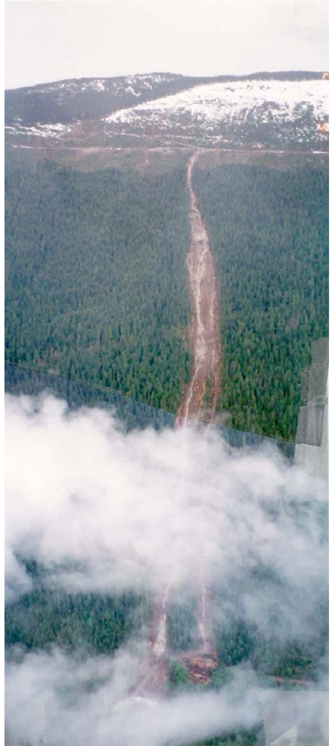
Fig. 6 May 31, 1997 Gowan Creek debris flow initiated as failure of road-fill slope about 80 km southeast of Pemberton, British Columbia (Bartle et al. 1997)
