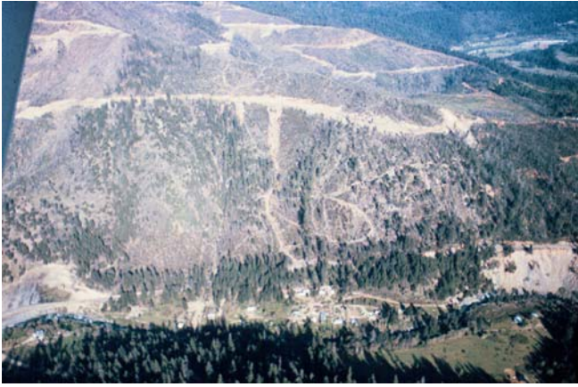
Fig. 1 Debris flows from fill-slope failures of road and log landing on Klamath National Forest near Happy Camp, California
