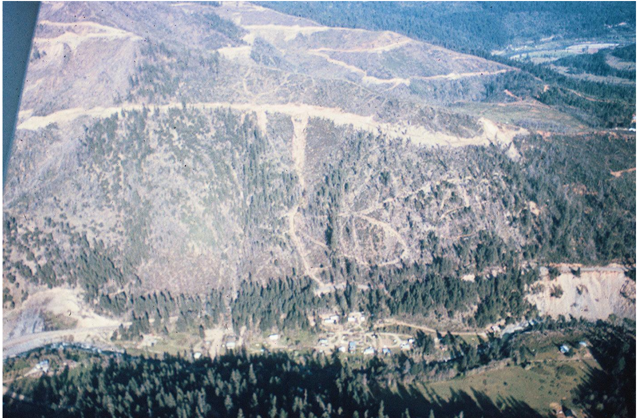
Figure 1 - Debris flows from fill-slope failures of road and log landing for timber salvage in the aftermath of 1960s Indian Ridge wildfire on Klamath National Forest near Happy Camp, California. Debris flows endangered community living along Indian Creek. The same area burned in the Slater fire September 2020. (1971 photo, view toward east; Happy Camp is next to right side of photo)
