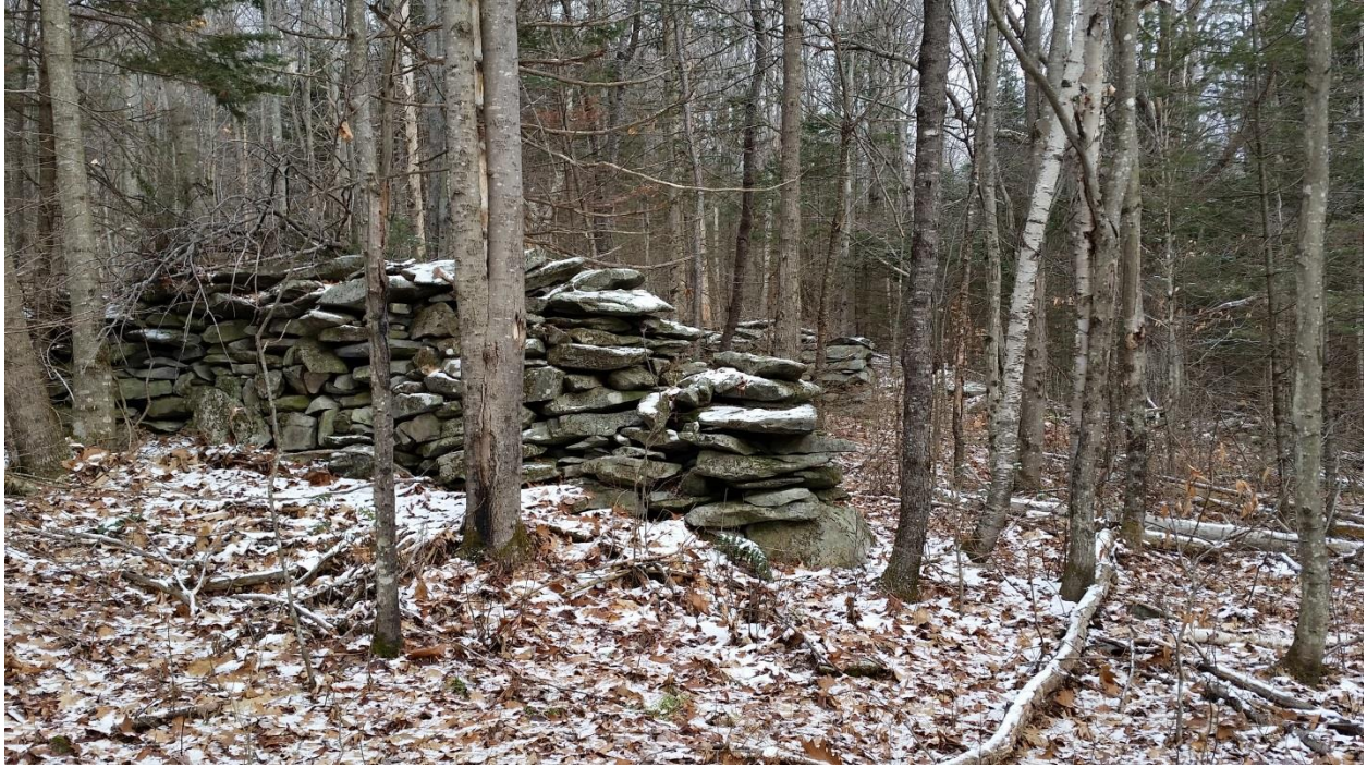
Two supporting walls, most likely from a barn or other farm structure
