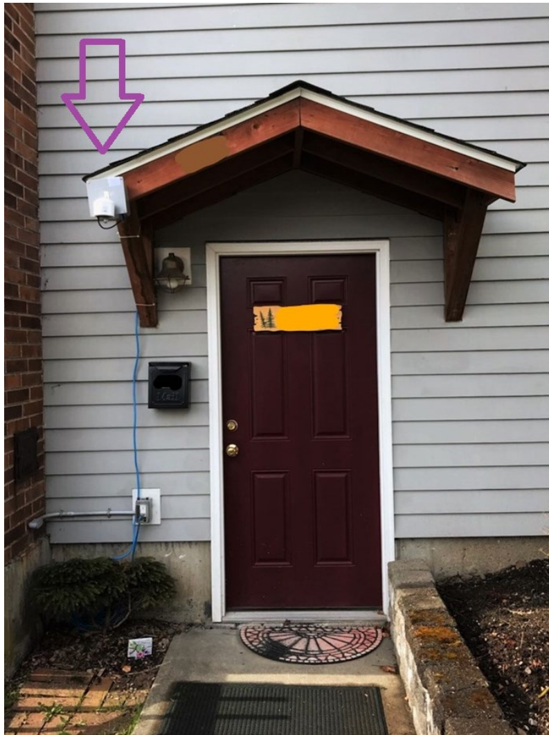
Figure 3. Example of PurpleAir site set up. The PurpleAir unit attached to the junction box is indicated by the purple arrow.
