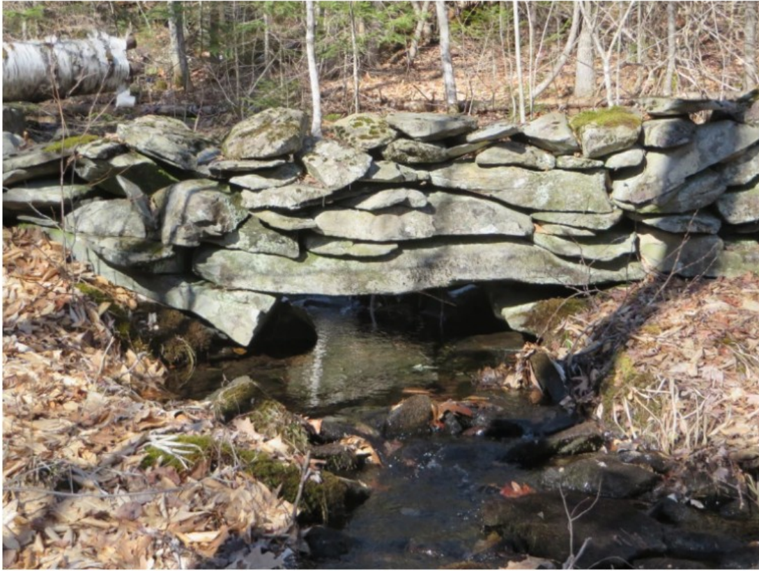
This section of wall was carefully built to span this small stream.
