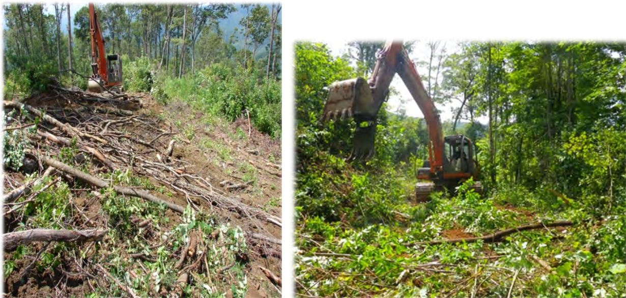
Figure 26. Farmers Branch Timber Sale in harvest unit 4 (left) and Eagle Fork Timber Sale unit 2 (right) subsoiling to reduce soil compaction and detrimental soil disturbance from skid roads and landings
