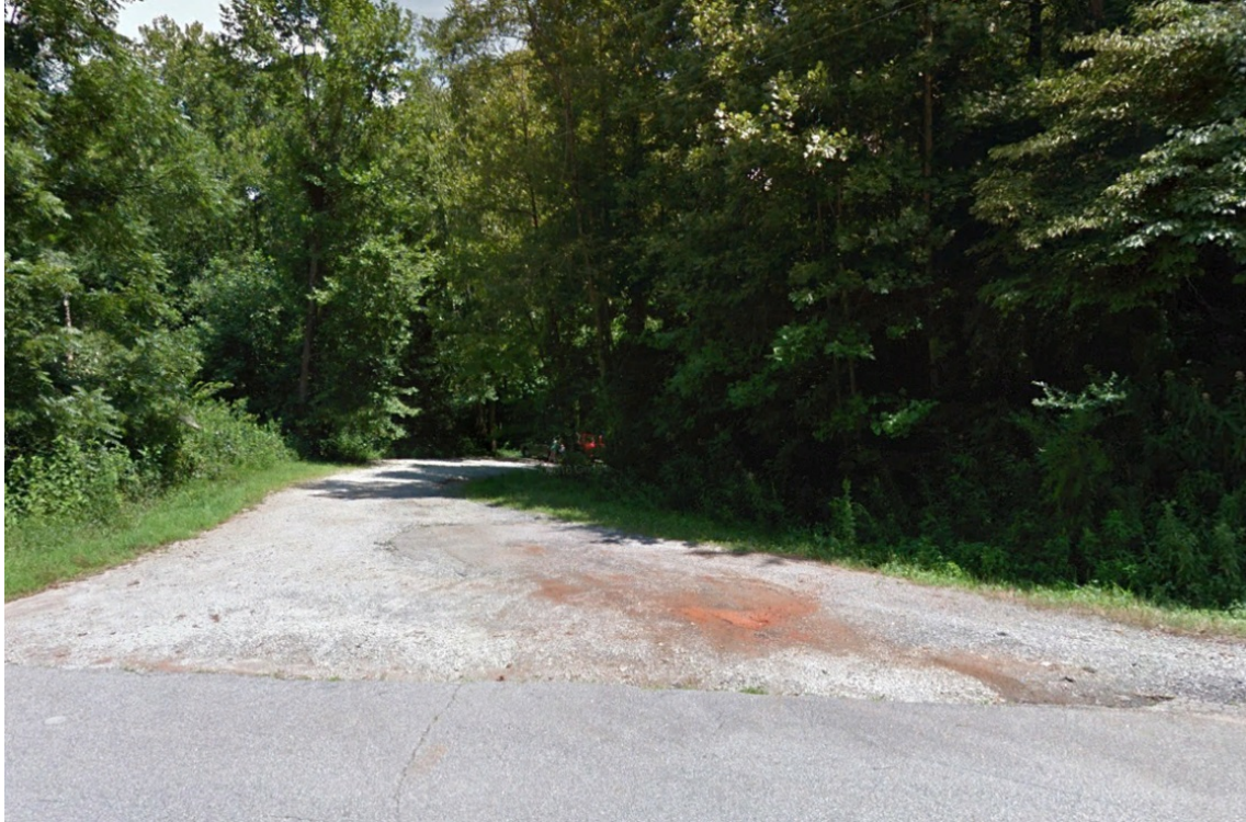
Figure 1.4-8. Ridley Fields Lot near the Hwy 28 Bridge.
