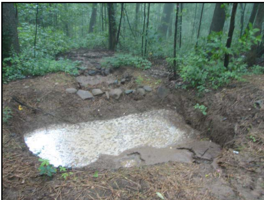
Figure 3.1.1.5 Photograph of a Constructed Sediment Trap Full of Sediment
