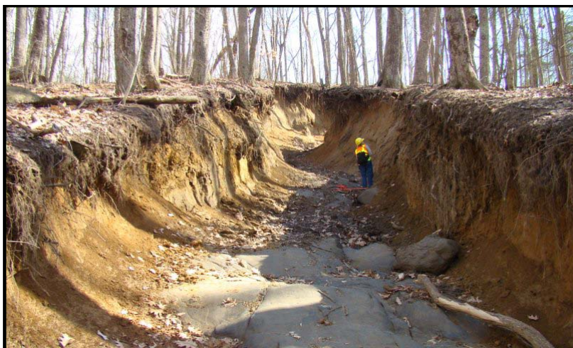
Figure 3.1.1.3. Example of trail entrenchment in the Upper Tellico OHV Area, where approximately 10 feet of soil has been lost, exposing large rock and bedrock.
