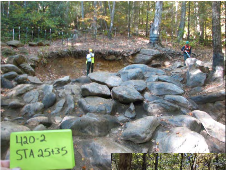
The “Rock Garden” on Trail 2 has deep entrenchment with eroding side walls and is a source of sediment to Jenks Branch.
