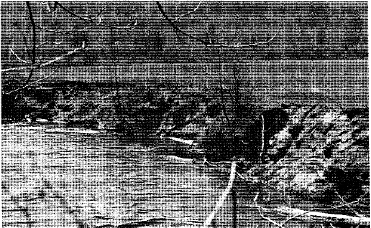
Eroding river banks along the West Fork.
