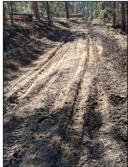
Road conditions during log hauling operations on the DLL2 project.
