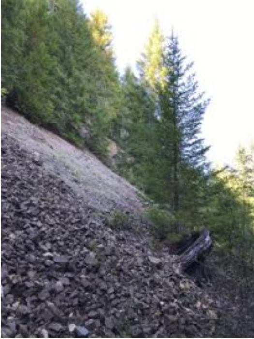
Figure 8: FSR2041515 at Unit 189- no sign of road
