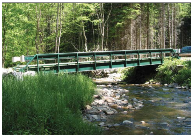
A temporary bridge installed over a perennial stream to reach a timber harvest area. (Photo by U.S. Forest Service, Northern Research Station.)
