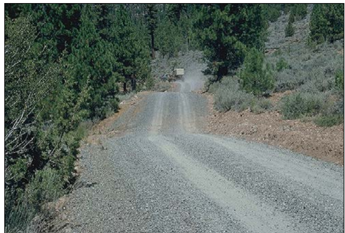
Figure 3.—A broad-based dip on a forest haul road. From Keller and Sherar (2003).
