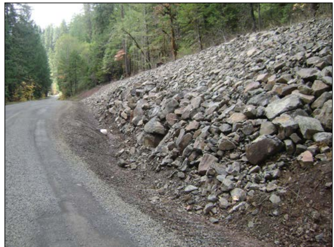
Riprap applied to a forest road cutbank for stabilization after initial erosion control measures following road construction were not adequate during winter storms. (Photo by U.S. Forest Service, Umpqua National Forest.)
