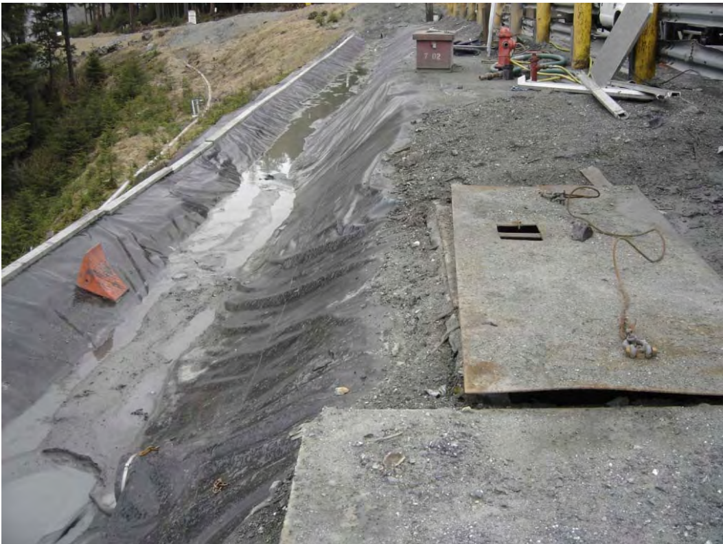
Photo 24: Ditch at 920 Area Looking West
