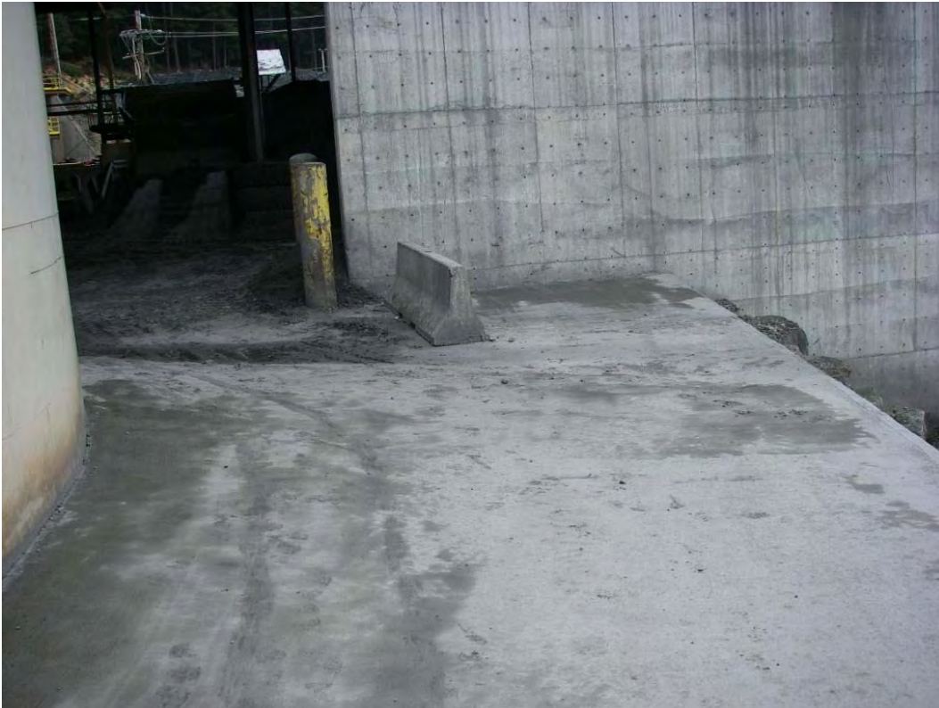
Photo 27: Tailings Thickener Concrete Containment
