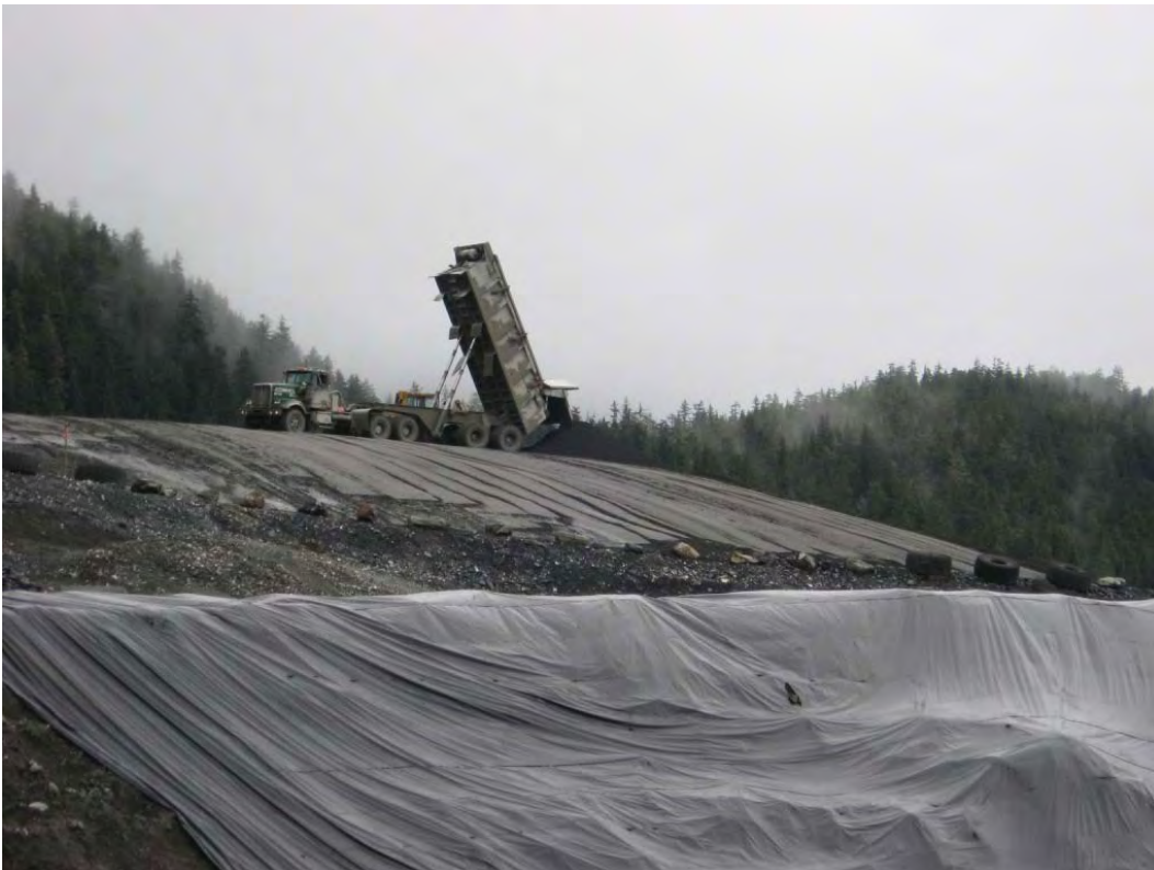
Photo 4: Haul Truck dumping tailings at the Tailings Disposal Facility
