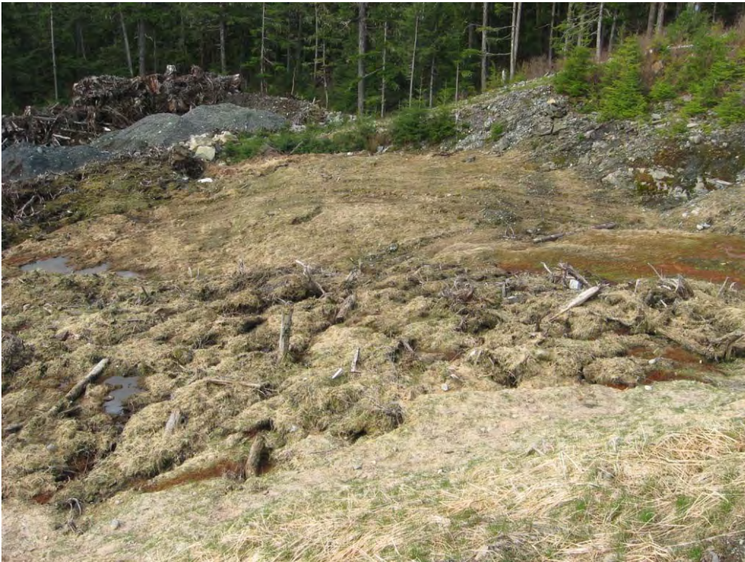
Photo 22: At Pit 7 looking downslope over the saturated toe of what is primarily overburden hauled from the quarry at 1.5 km on the A road
