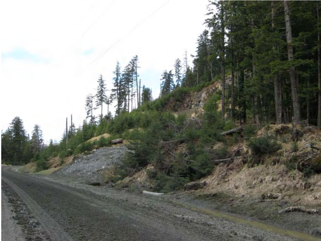
Photo 17: Side view of the access ramp and reclaimed and revegetated production rock in Pit 6
