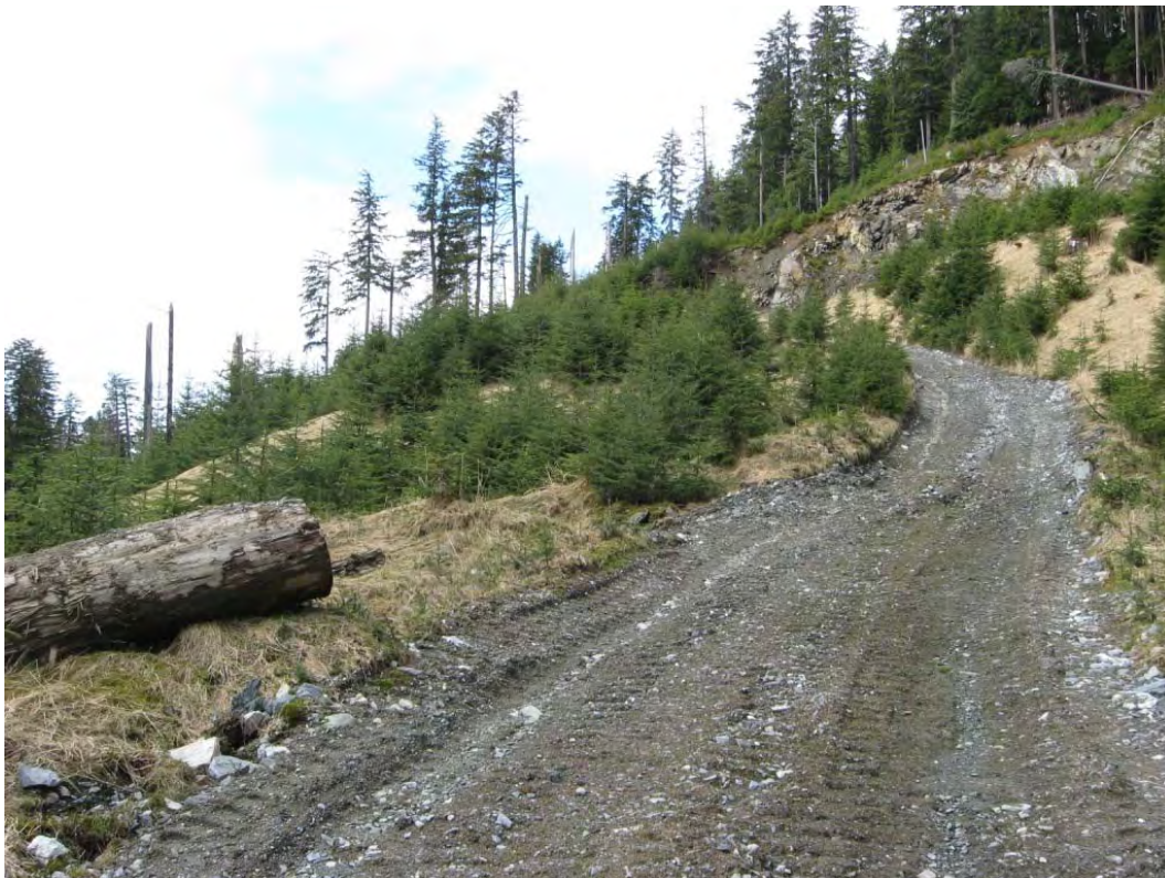
Photo 18: Looking up the access ramp that overlies reclaimed and revegetated production rock in Pit 6
