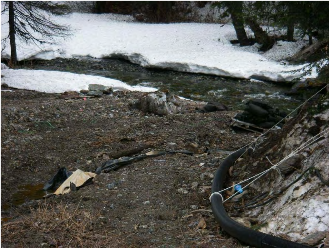
Photo 25: Construction Area near Freshwater Intake
