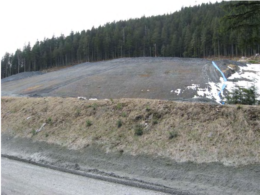
Photo 9: Groomed final slope on the lower portion of Site 23
