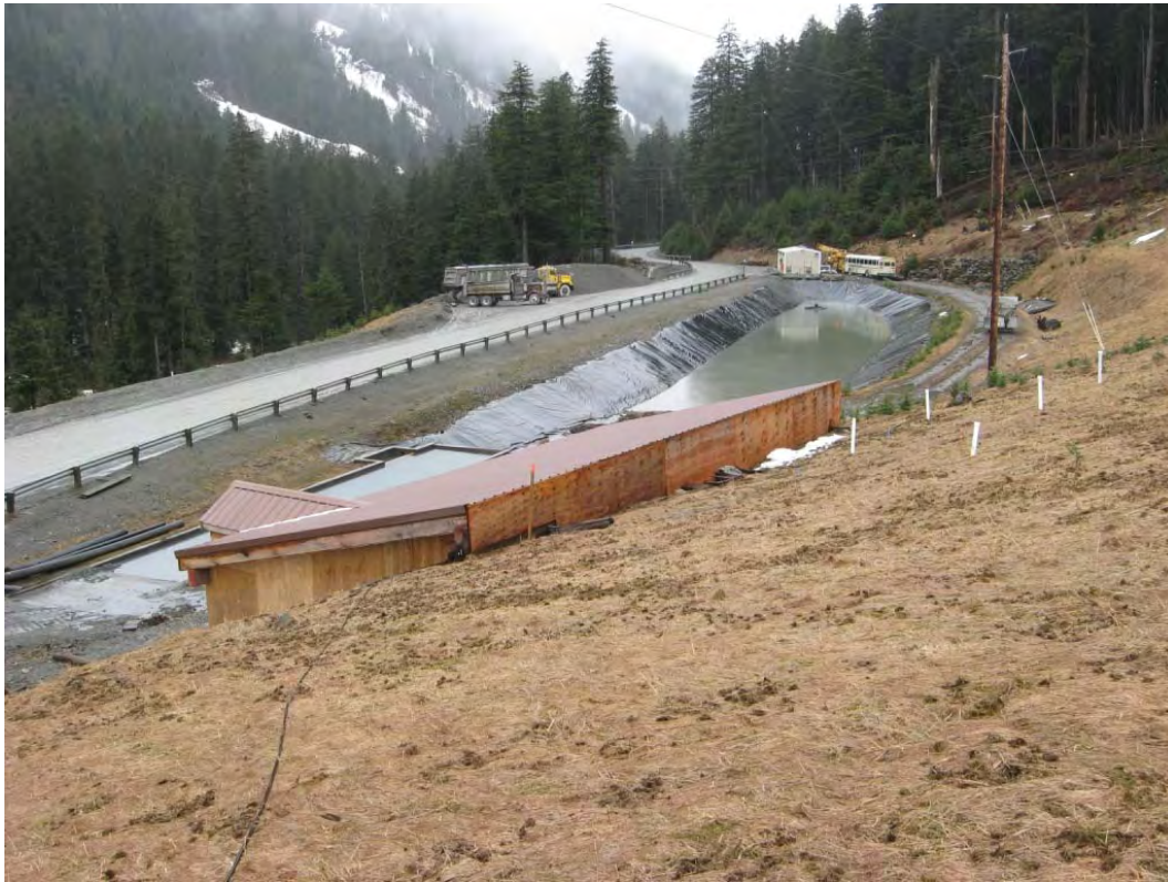
Photo 7: Side view of the cover (foreground) and wooden housing for seepage collection piping at Site 23; lined stormwater storage pond in background
