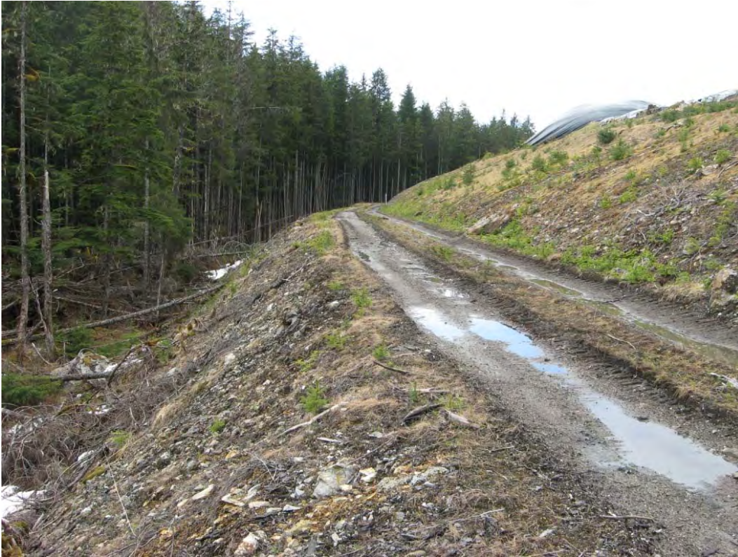
Photo 13: Perimeter berm constructed of production rock at Site E
