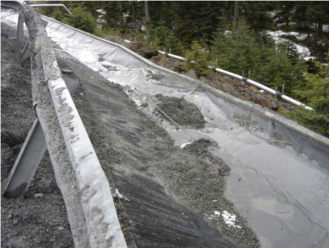
Photo 23: Ditch at 920 Area Looking East
