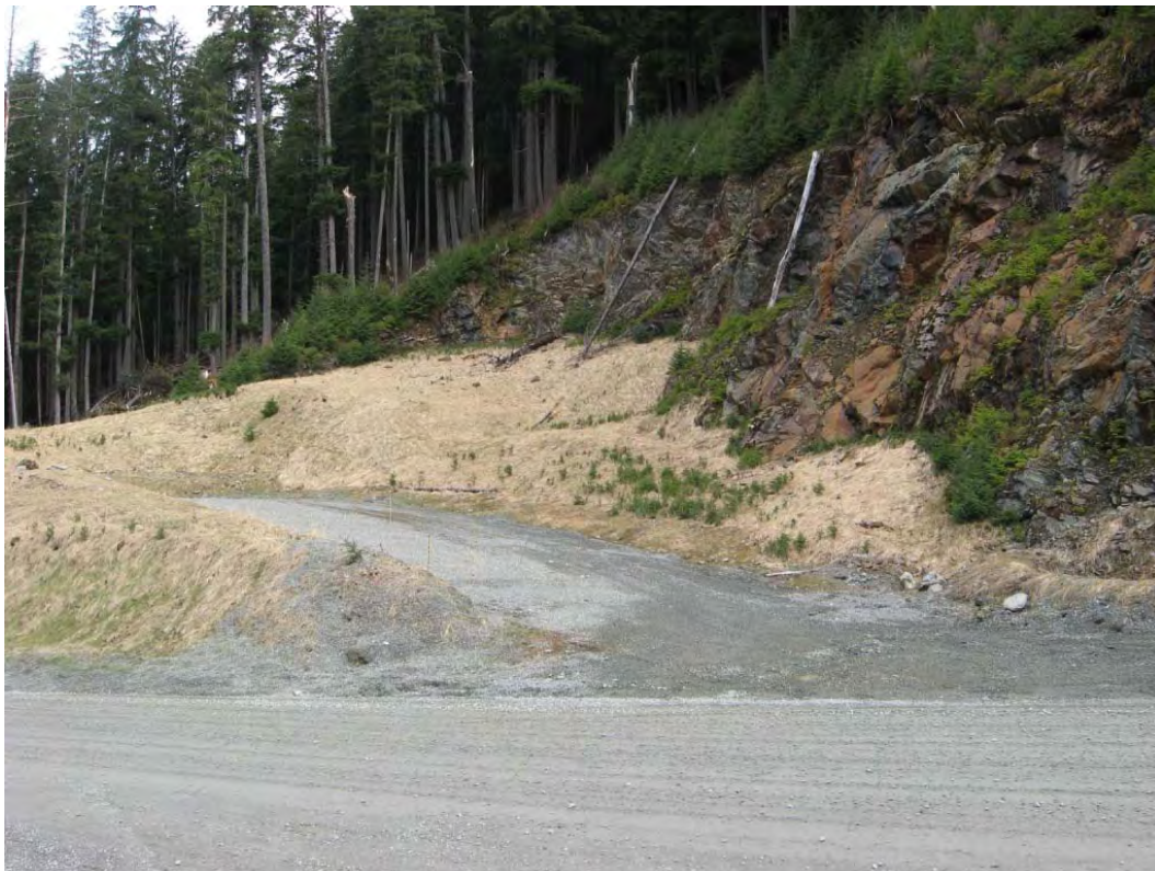
Photo 20: Side view of the access ramp and reclaimed and revegetated production rock in Pit 174
