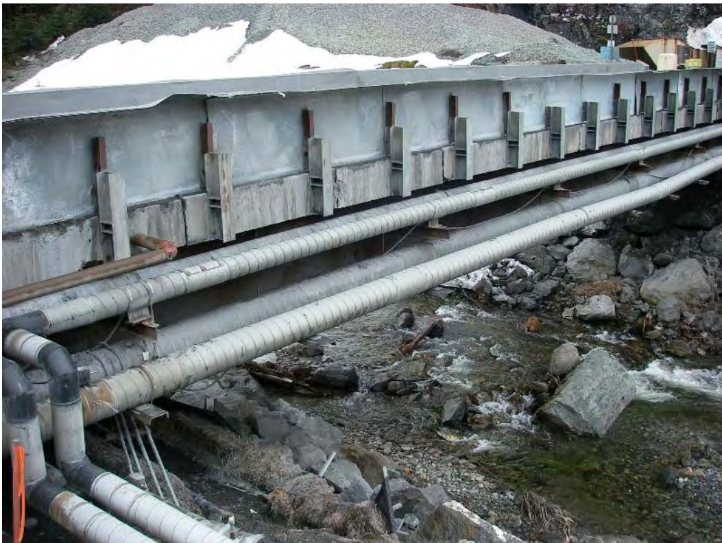
Photo 28: Pipelines attached to the bridge that crosses Greens Creek at the 920 Area
