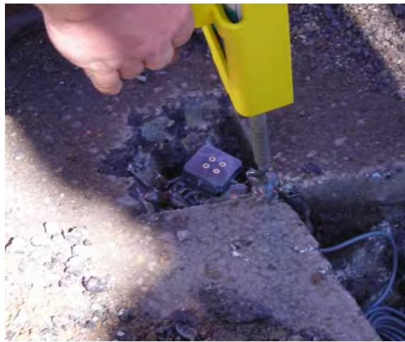
FIGURE 8 Sensor installation.
