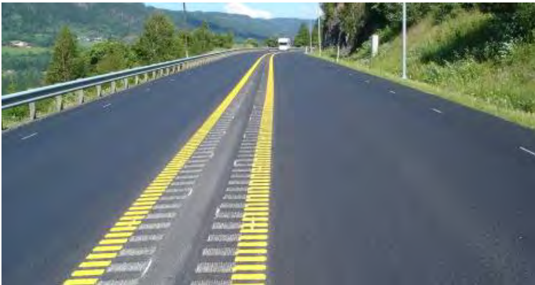
FIGURE 1 Visual central reserve with rumble strips.
