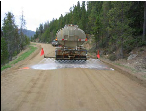
Figure 6.32. Magnesium chloride-based dust suppression product application.
