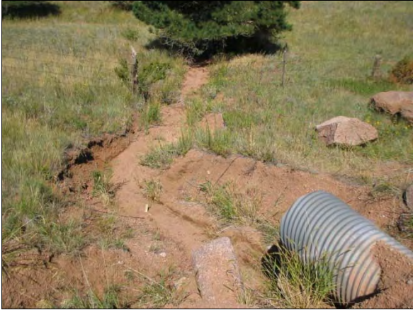
Figure 6.11. Non-forested, shrubland drainage plot with culvert.
