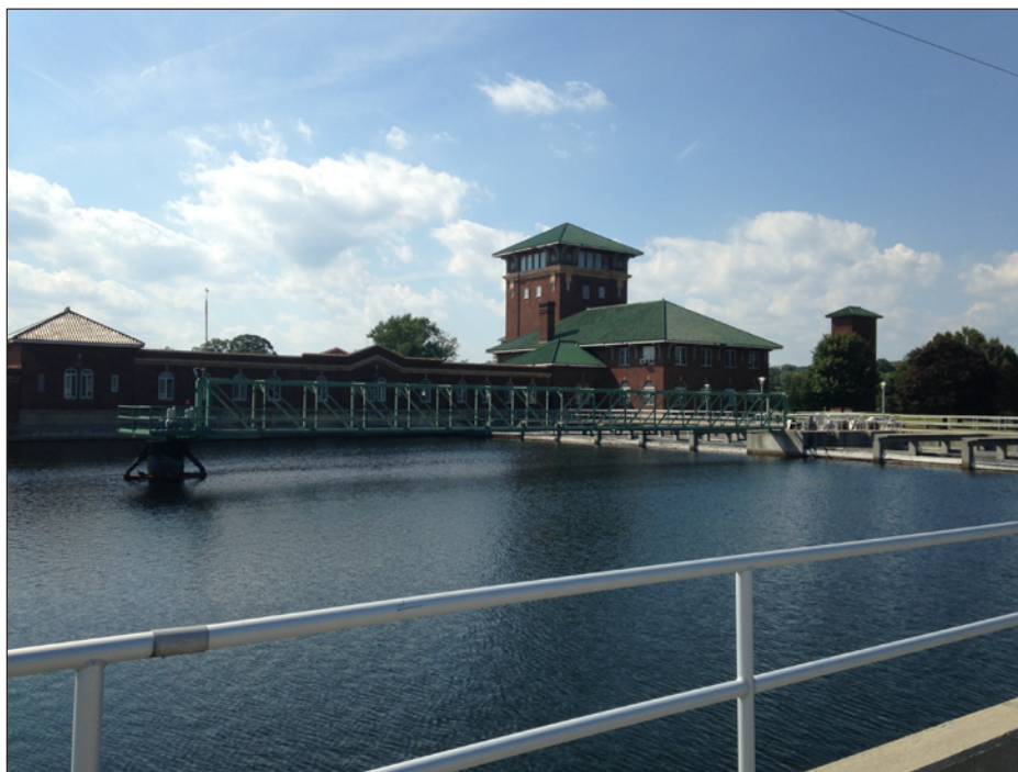
Water treatment plant, Baltimore, Maryland. Photograph by Cheryl A. Dieter, USGS.
