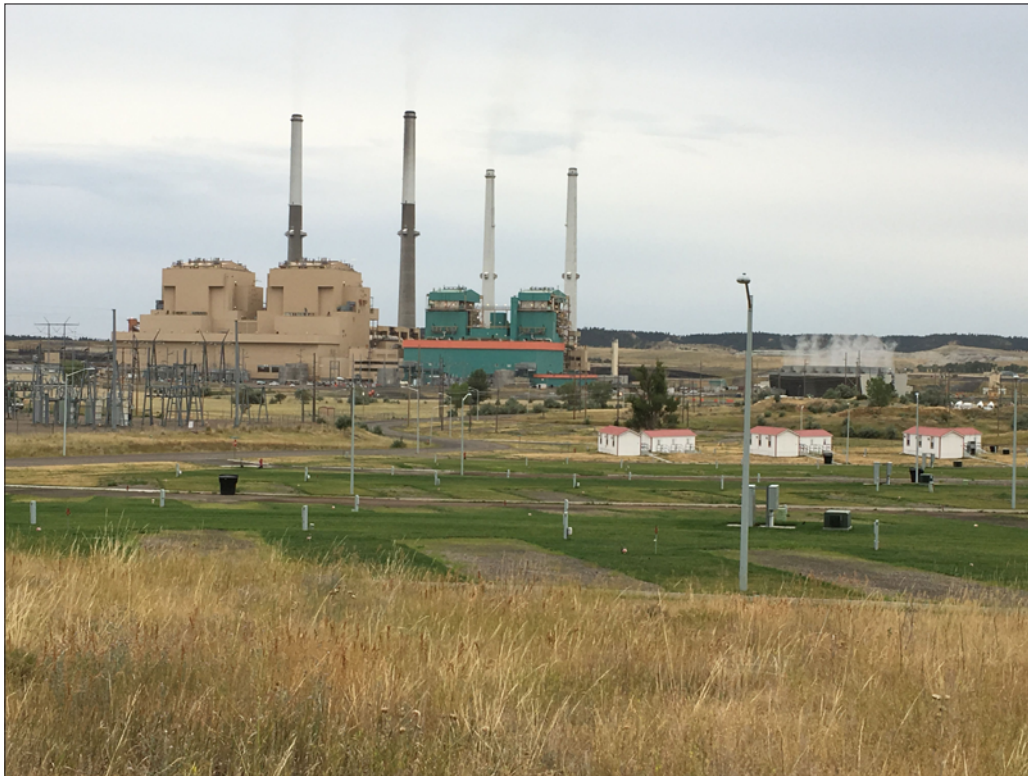
Thermoelectric powerplant in Montana. Photograph by Rodney Caldwell, USGS.
