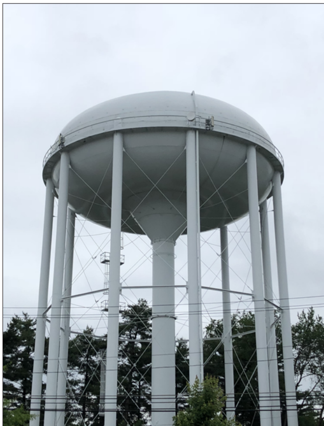
Public-supply water tower in Baltimore County, Maryland.
