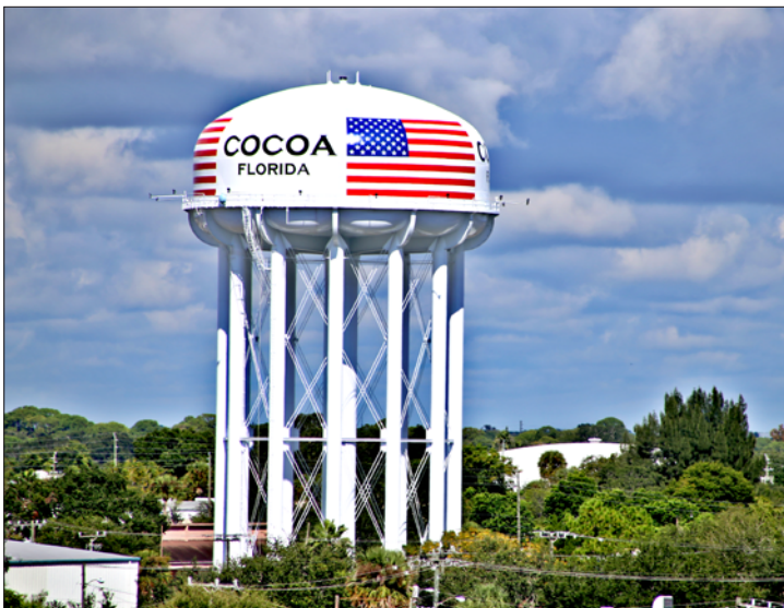
Public supply water tank, winner of the “2015 Tank of the Year” presented by Tnemec Company, Inc. Photograph provided by the City of Cocoa, Florida, used with permission.
