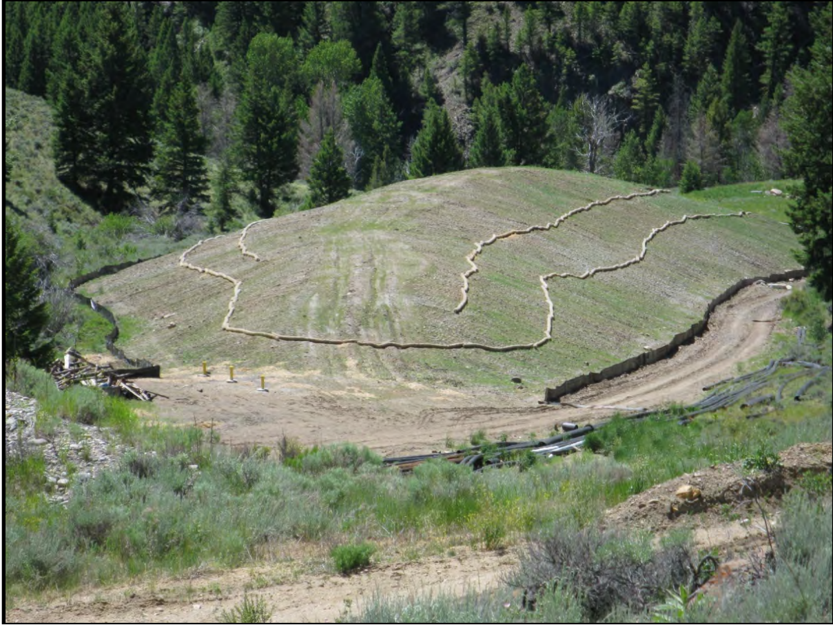
Photo 2.1-16. Salvaged topsoil storage pile.
