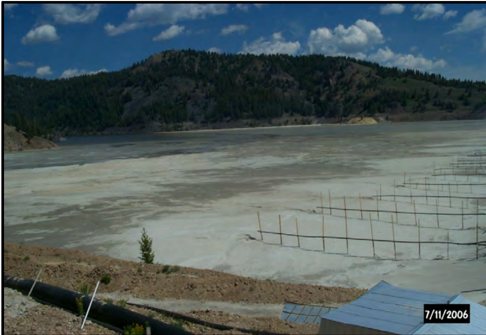
Photo 2.1-13. TSF impoundment, view to north up Bruno drainage (filled). Beach in foreground, tailings slimes pipelines at right.
