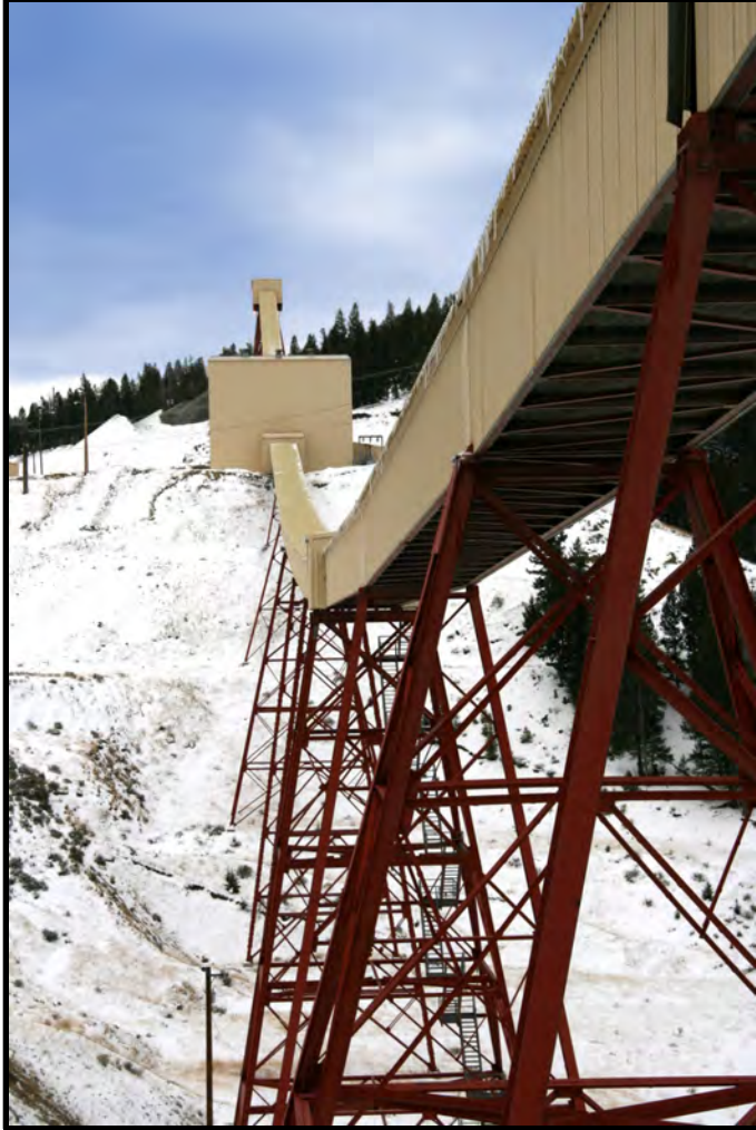
Photo 2.1-5. Overland belt conveyor to mill coarse ore stockpile, view to east.
