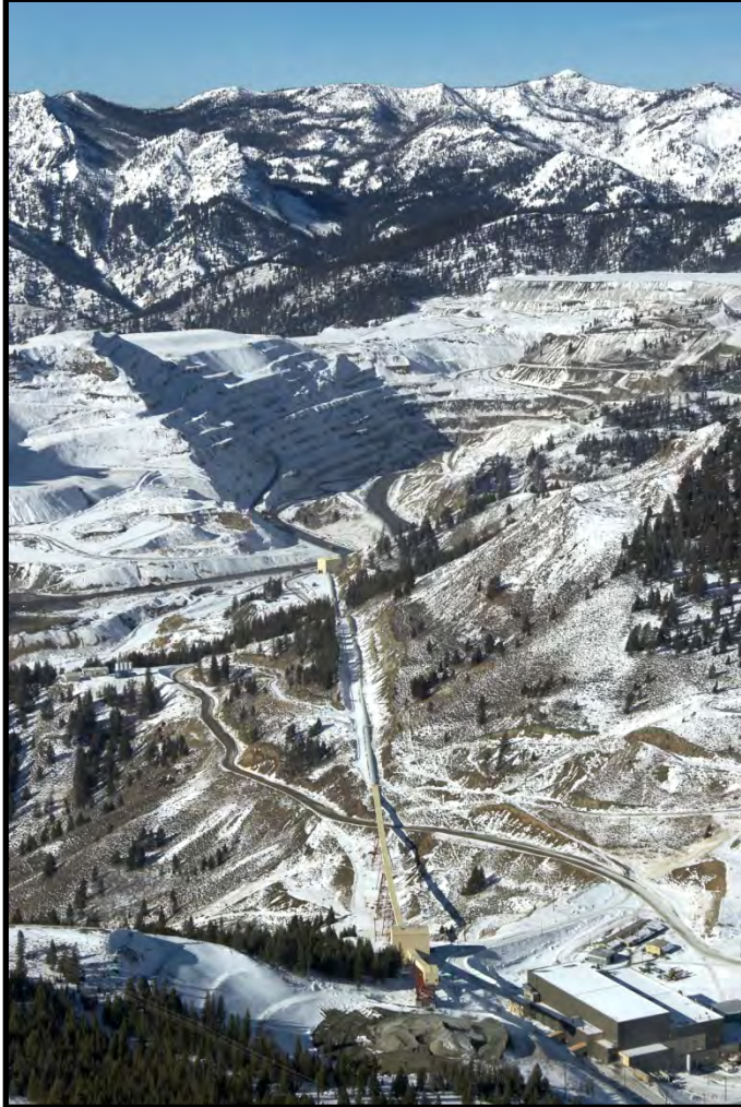
Photo 2.1-6. Conveyor and, in foreground, coarse ore stockpile and mill. Conveyor angles northward around hillside in photo center. View to west.
