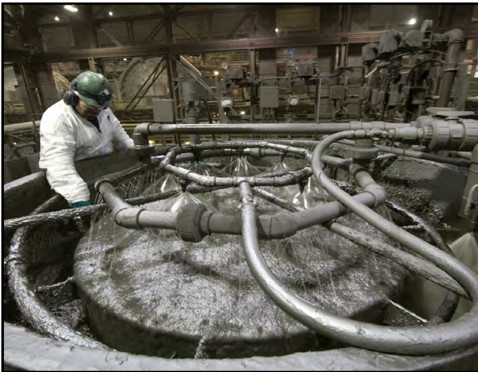
Photo 2.1-10. Column flotation cells.
