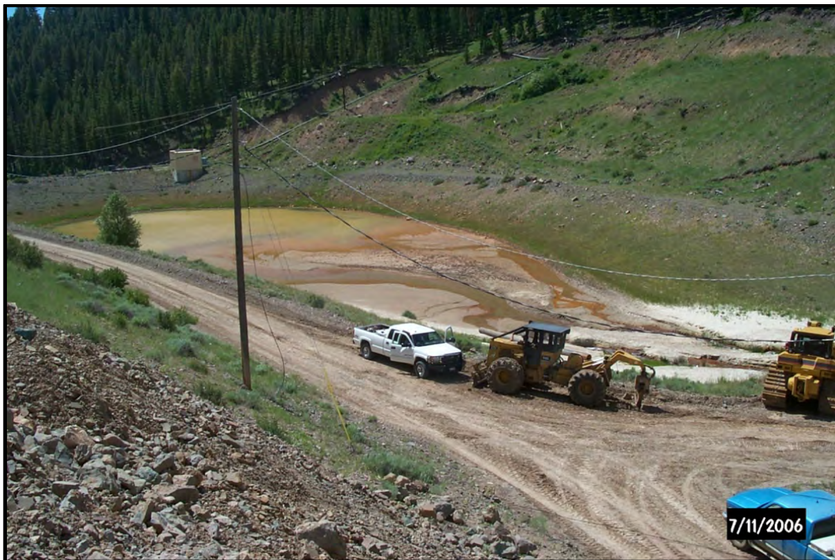
Photo 2.1-15. Sedimentation pond (SRD) below the TSF embankment. View to southeast.
