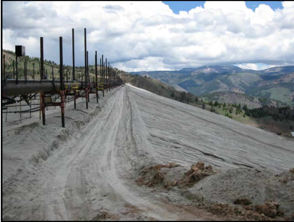
Photo 2.1-12. TSF embankment. Header pipeline, cyclones and embankment face, view to northeast.
