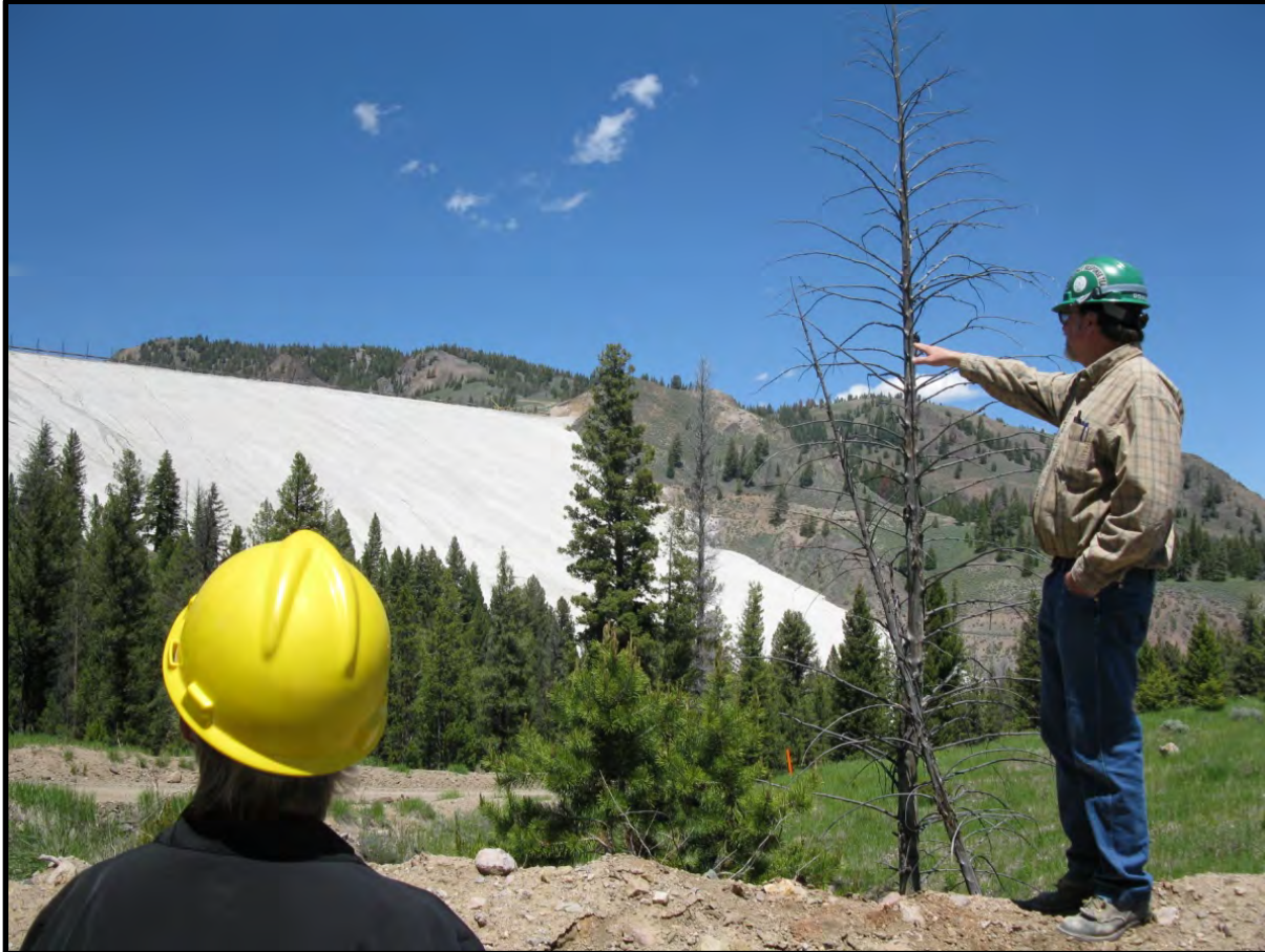
Photo 2.1-14. TSF embankment face, view to northeast.
