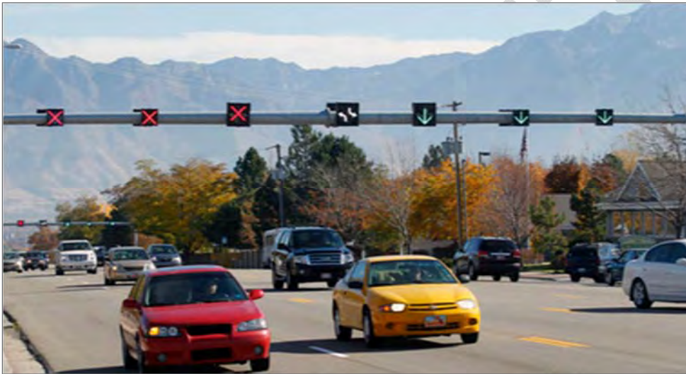
Figure 2-7. Changeable Lane-control Signals
